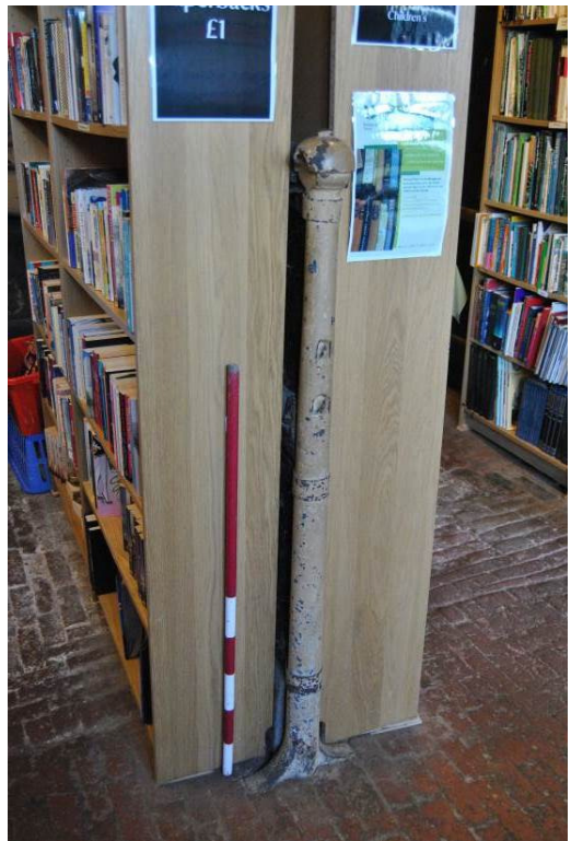
Plate 34: Cast iron heel-post.
