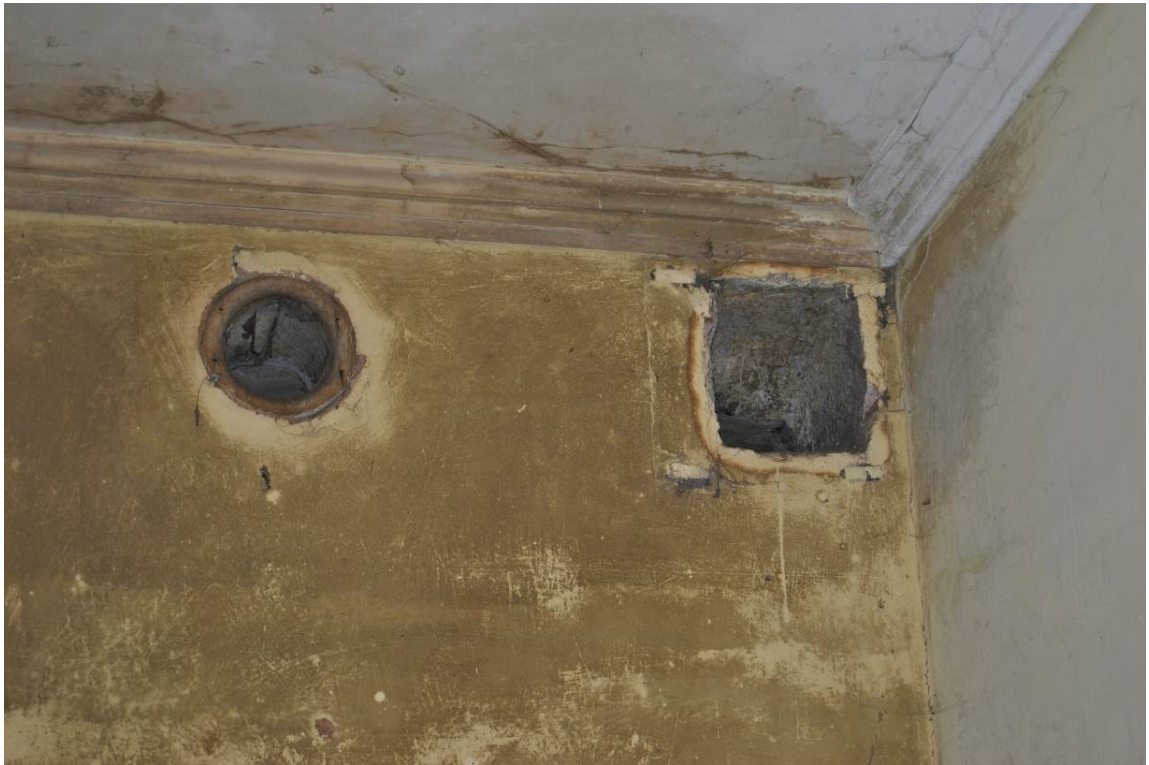
Plate 38: Pre- and post-conversion high-level ventilators (left and right respectively).
