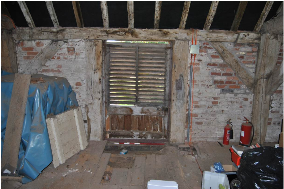
Plate 47: Surviving primary timber-framing at Bay 5 (east) with inserted, louvred door NB. double peg holes to inner edge of intermediate studs evidencing former mid-rail.
