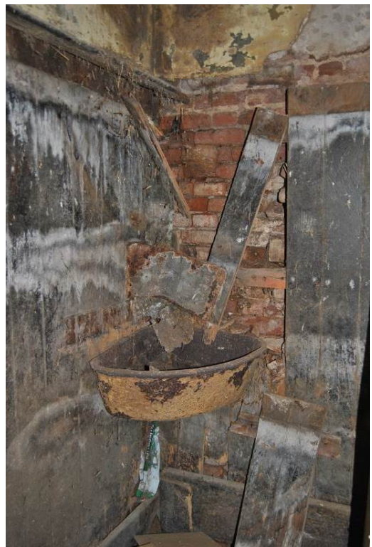
Plate 28: Early brickwork exposed behind T&G lining at south end of west wall (loose box 2).
