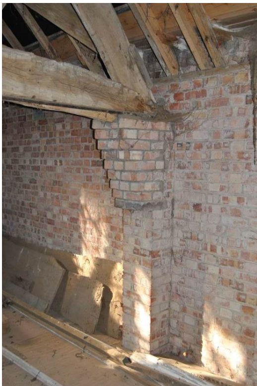
Plate 50: Corbelled brick pier at T2 (W) – 1940s.
