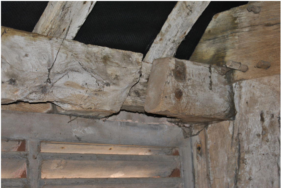
Plate 48: Primary wall plate; bridled scarf joint with splayed abutments.
