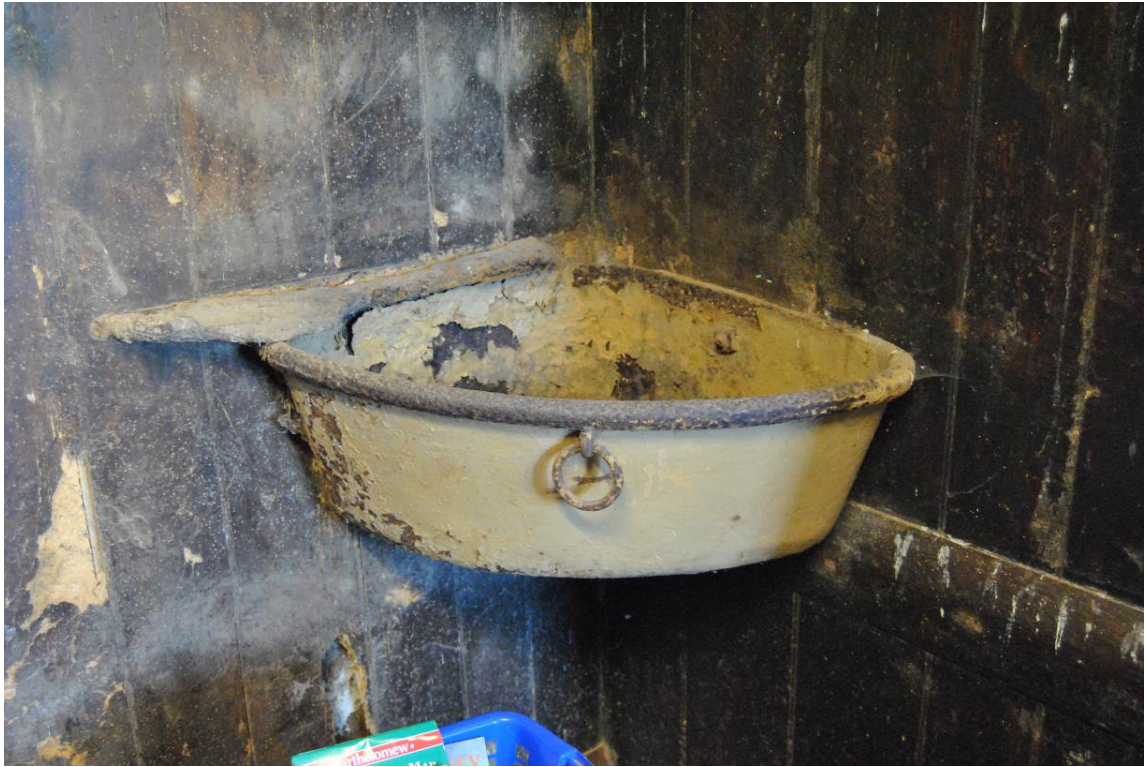
Plate 40: Typical manger with tethering ring, stable [G.02].
