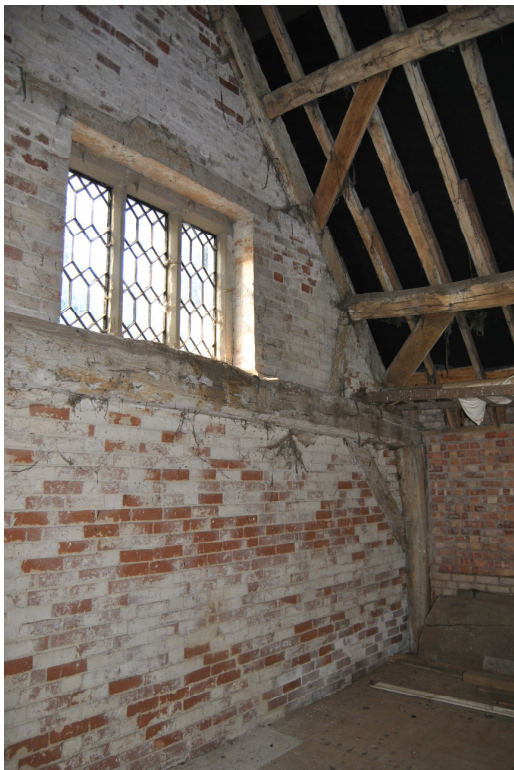
Plate 59: Truss T1 (south gable), formerly closed in wattle and daub, rebuilt in brick, mid-C19 th .
