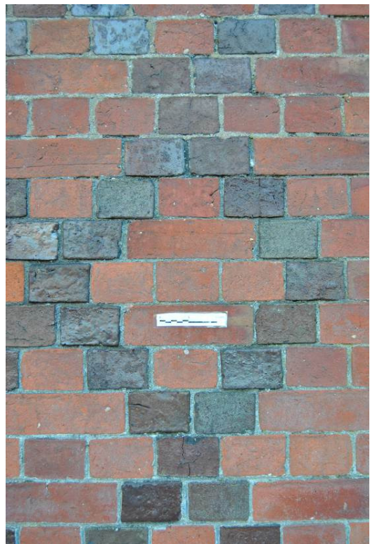
Plate 5: Detail of brown-glazed diamond pattern diaper-work (10cm scale).
