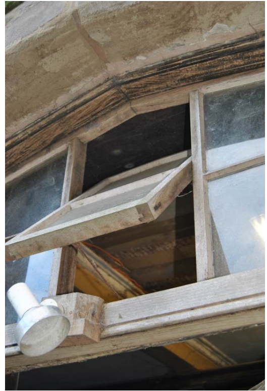
Plate 7: Overlight with central opening panel.
