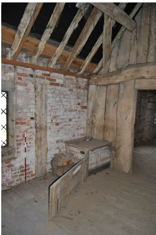
Plate 52: Feed bin at Bay 3 (NW) serving ground floor chutes within [G.02].
