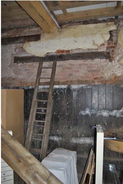
Plate 27: Blocked window below timber lintel in west wall of loose box 2.
