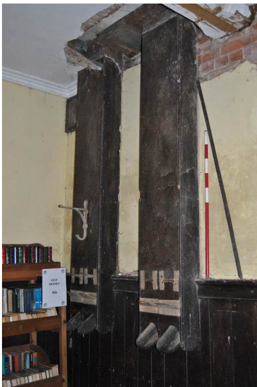
Plate 36: Feed chutes to west wall.
