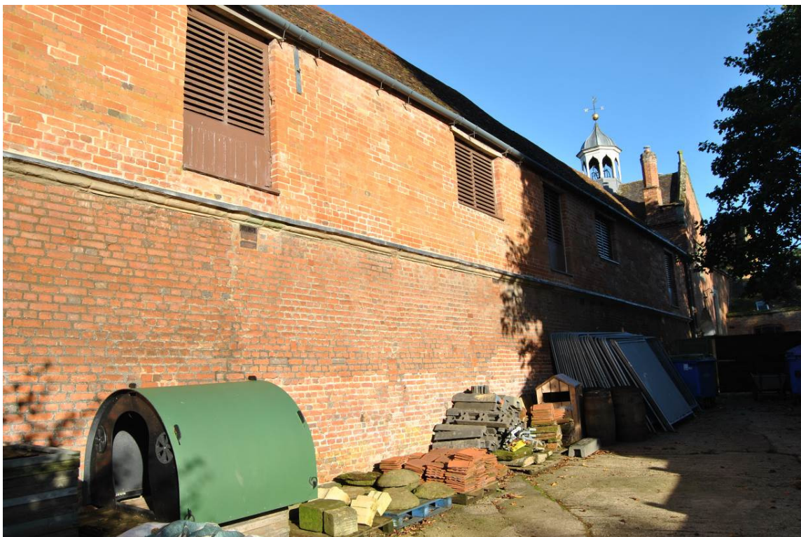
Plate 11: East elevation (oblique) looking north-west towards carriage entranceway (beneath cupola to right of photo); NB: first floor stone ogee-moulded string and corbelled brickwork to upper floor.
