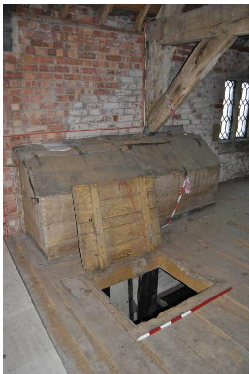
Plate 51: Floor hatch and feed bins at Bay 2/3 feeding ground floor chutes at [G.01].
