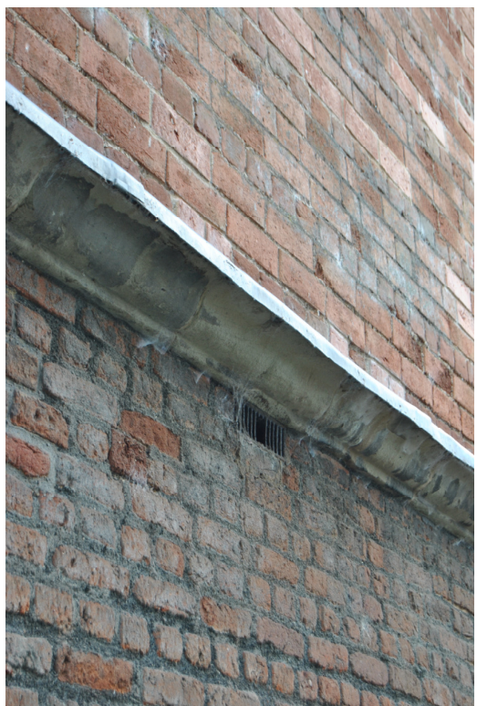
Plate 15: Detail of corbelled out first floor brickwork.
