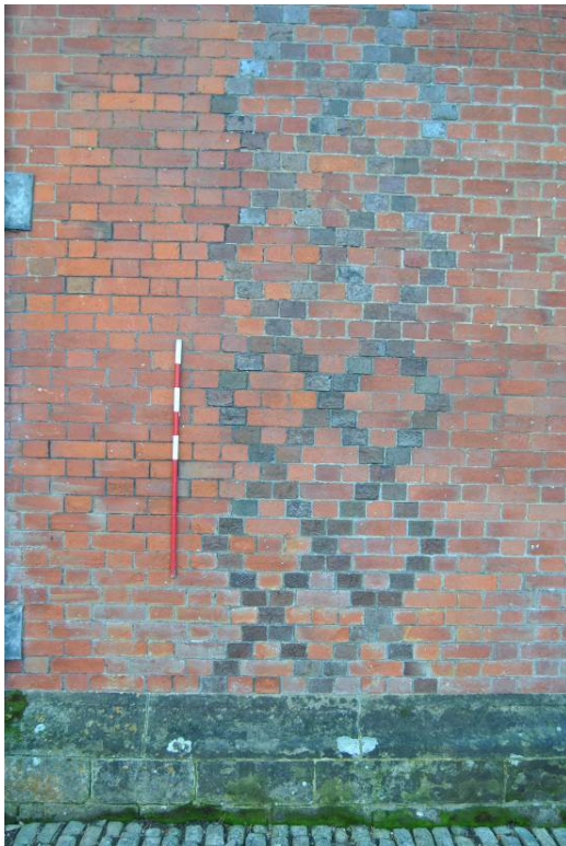
Plate 4: C19 th Flemish-bond refacing of west elevation with diaper work strips (1m scale).
