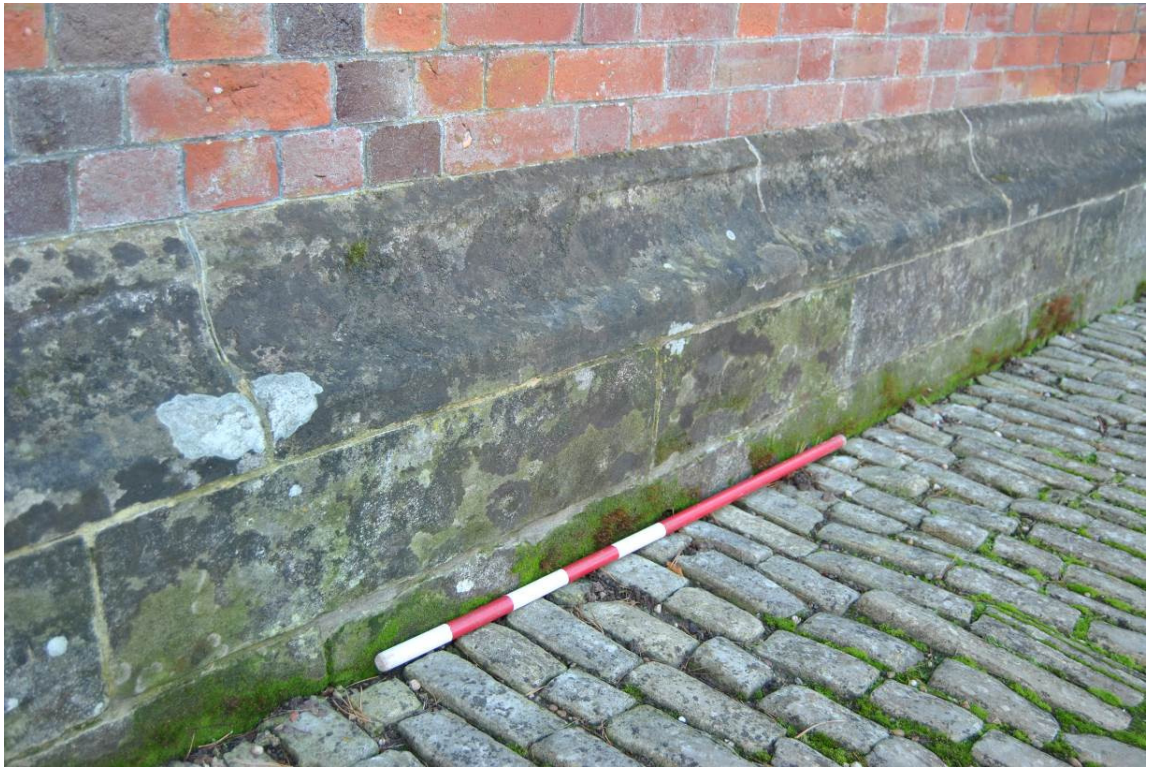
Plate 3: West elevation; stone plinth with moulded cap.
