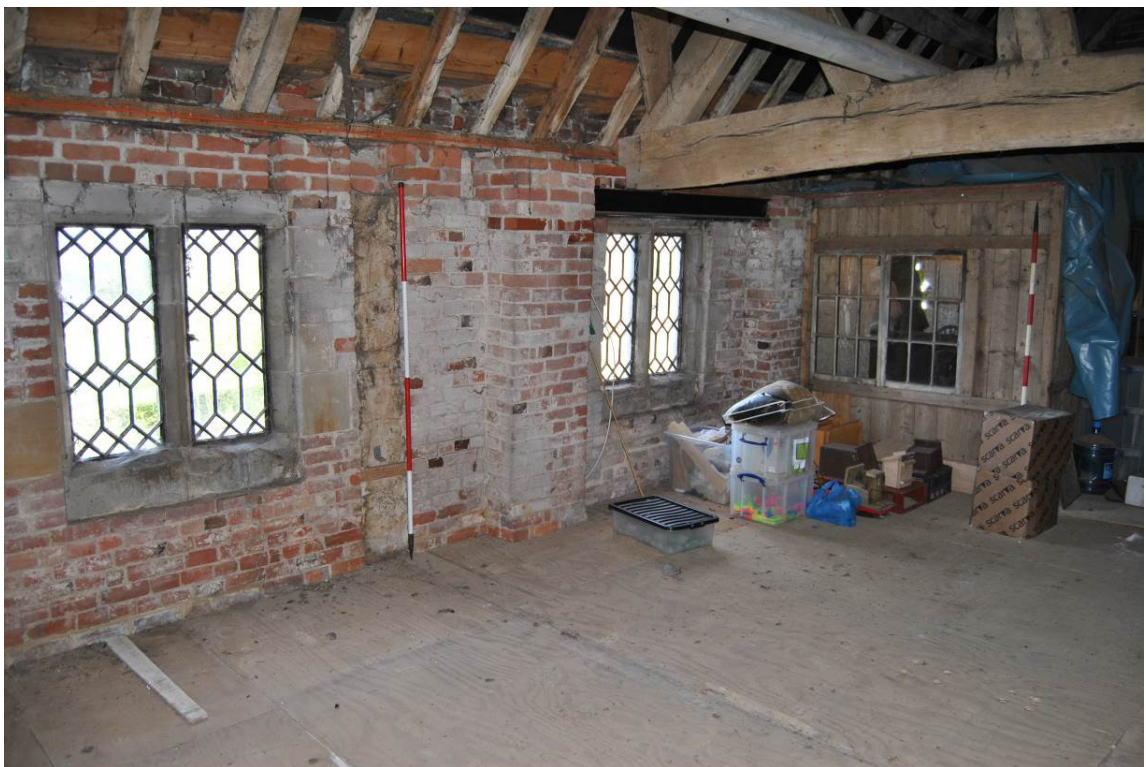
Plate 49: Rebuilt west wall at Bays 4/5; NB: surviving intermediate stud to left of photographic scale and tie of truss T5 supported on paired RSJs over inserted window.
