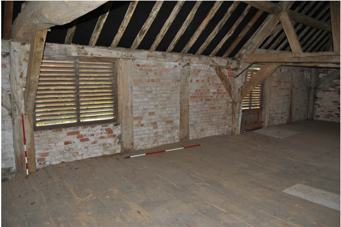
Plate 46: Surviving primary timber-framing at Bays 1-2 (east) with inserted, louvred door/window. Bay 2 (left) is wider at 17ft, Bay 1 (right) is 15ft in width.
