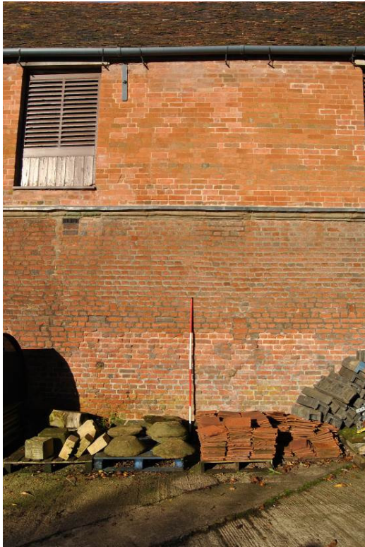
Plate 12: Representative section of east elevation brickwork; primary to GF, secondary facing to 1F.
