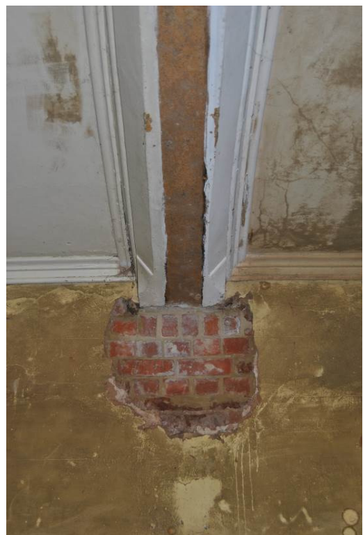
Plate 37: Principal ceiling beam with evidence of former, inserted steel supports (removed 2011).
