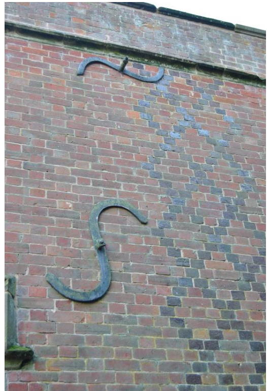
Plate 10: Tie-rod end plates at first floor level, south end of west elevation.
