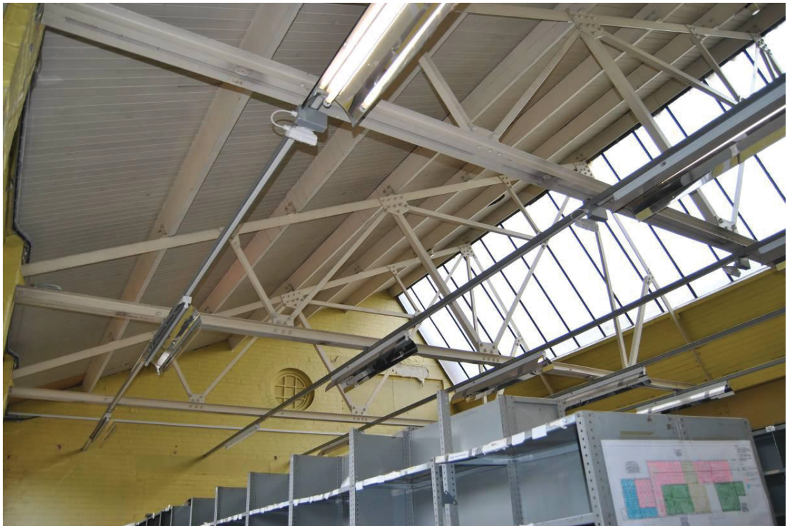
Plate 80: Asymmetrical steel truss to Phase IIIa extension [G.008], with glazed north-light.
