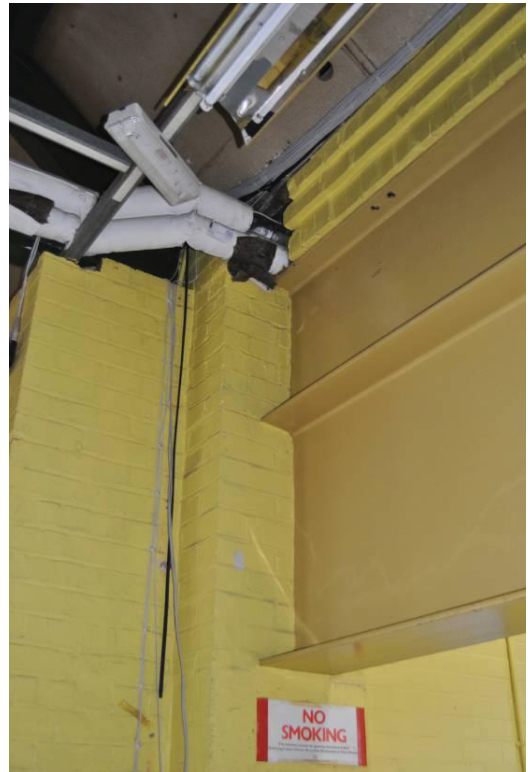
Plate 54: Doubled steel I-beam spanning opening to western Phase IIIa extension [G.006](b).
