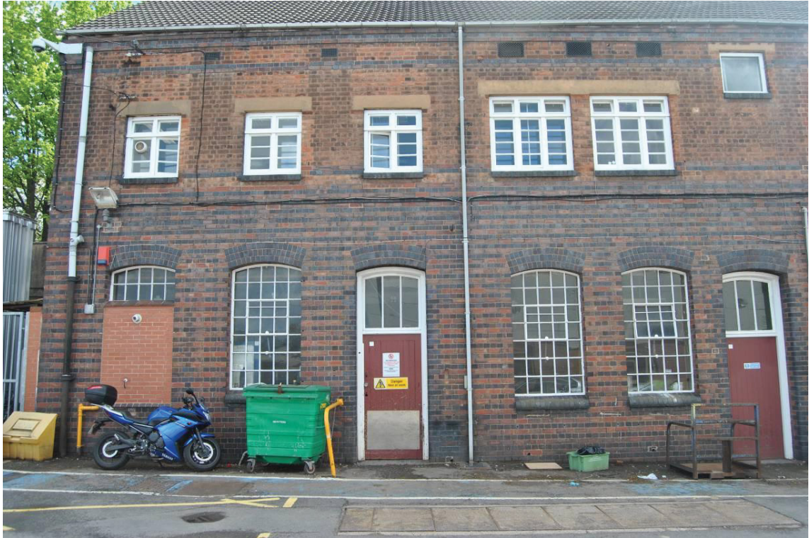
Plate 55: Phase II extension, north elevation. NB: clear disturbance to brickwork above three left hand windows.
