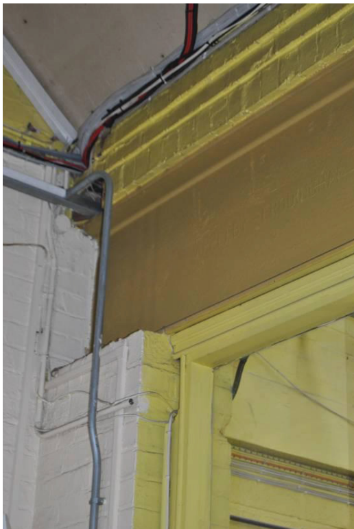
Plate 53: Steel I-beam spanning opening to eastern Phase IIIa extension [G.008].
