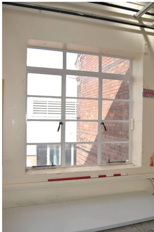
Plate 93: [G.003]; 3-light steel framed window to north elevation.
