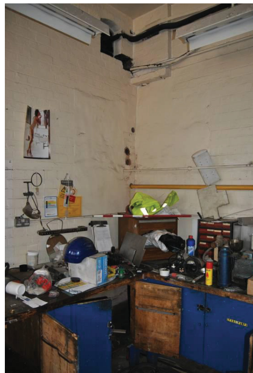
Plate 63: Patching to wall suggesting former fireplace (NB: angled wall shown in this location on supplied plans)
