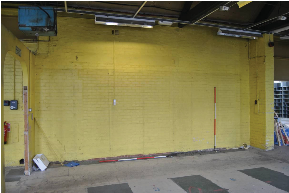
Plate 50: Section of primary south wall at Bays 10/11 with two blocked doorways.
