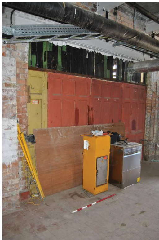
Plate 21: [B.010]; infill panelling of re-used doors (west wall).
