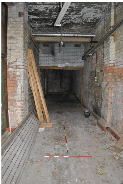
Plate 35: [B.007] looking south NB: high level glazed brickwork to middle distance
