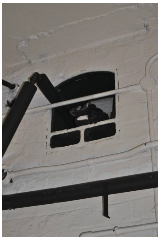
Plate 60: Workshop [B.015]; high-level wallbox in west wall indicating former line-shafting.
