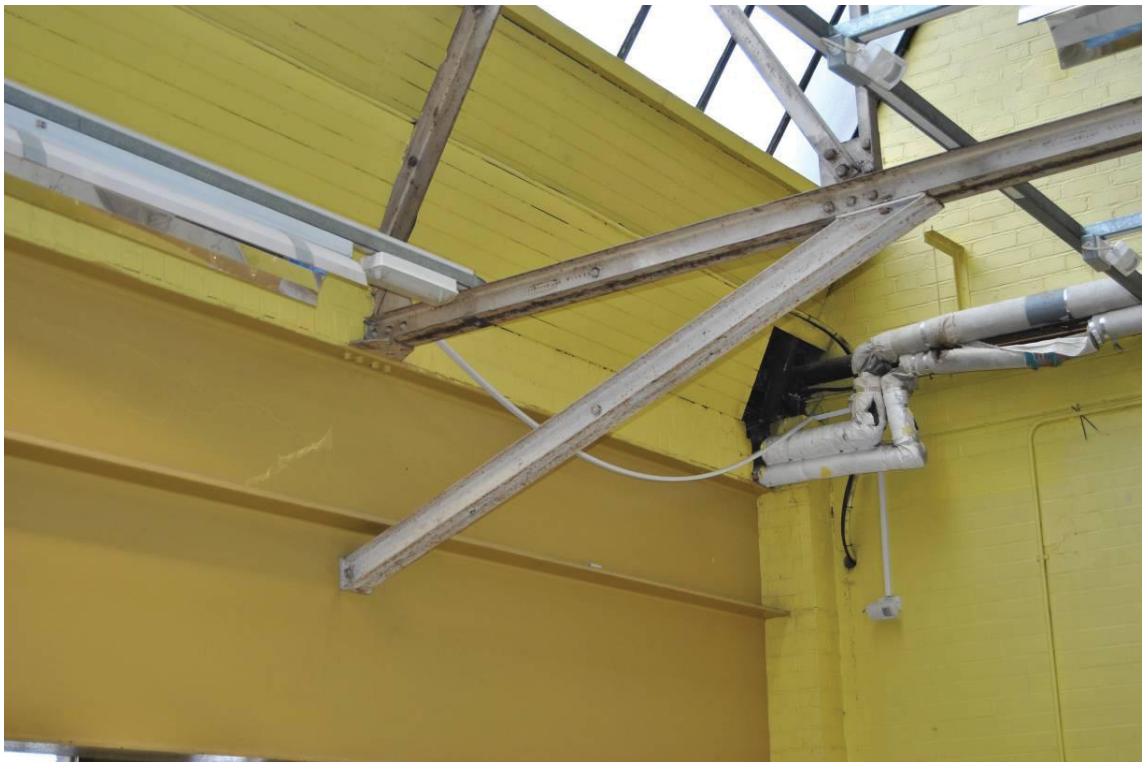
Plate 81: Additional brace to north end of steel truss within [G.006](b).
