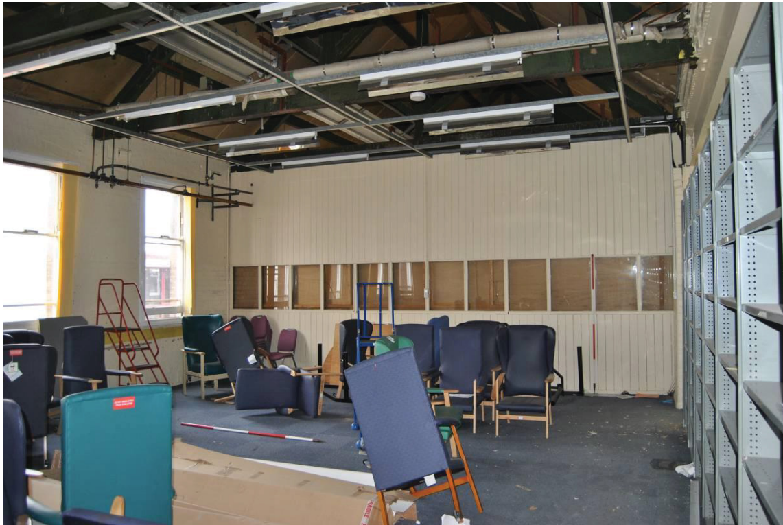
Plate 47: Primary range, west end; Room [G.005](a) looking east with inserted, part-glazed partition.
