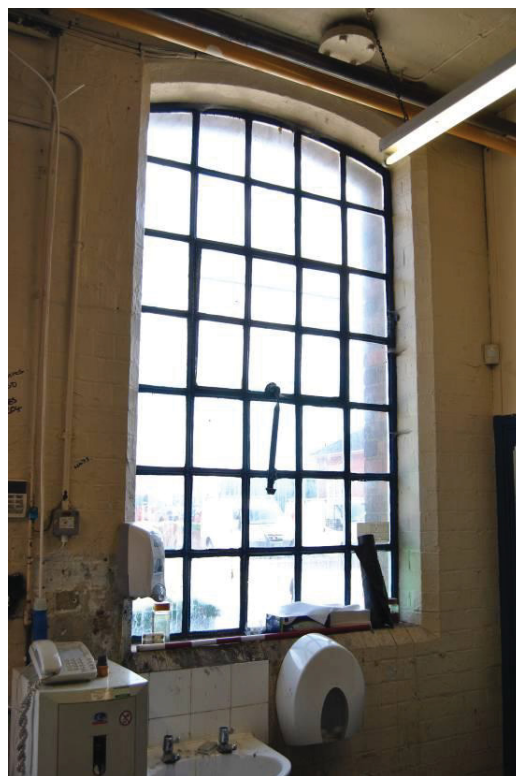
Plate 58: Workshop [B.015]; detail of iron multi-pane window.
