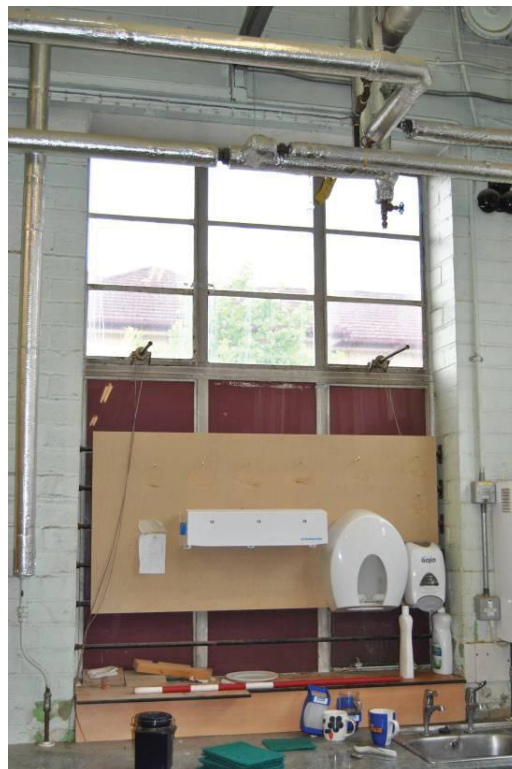
Plate 91: 3-light steel window frame, [G.002].
