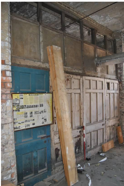
Plate 33: Infill panelling of re-used doors, [B.008].
