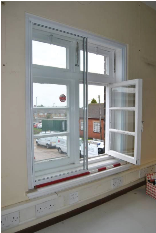
Plate 68: Inserted timber casement window to north wall of [G.010].
