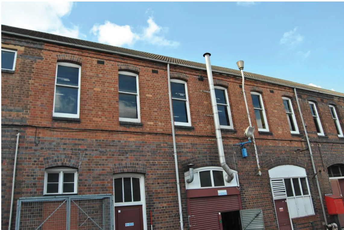
Plate 12: Renewed upper ground floor walling and windows at Bays 12 - 15 (see Figure 9a)
