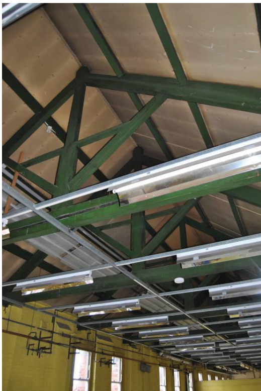
Plate 48: Primary range; king-post roof structure.
