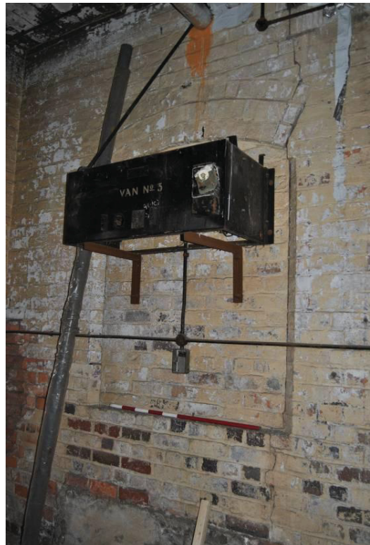
Plate 34: Wall-mounted 'Westalite' VR30/25 rectifier; NB: fixed to blocking of primary window opening.
