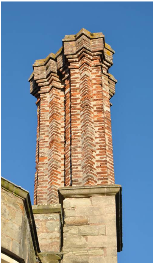
Plate 14: Star-form brick stack (east gable end)
