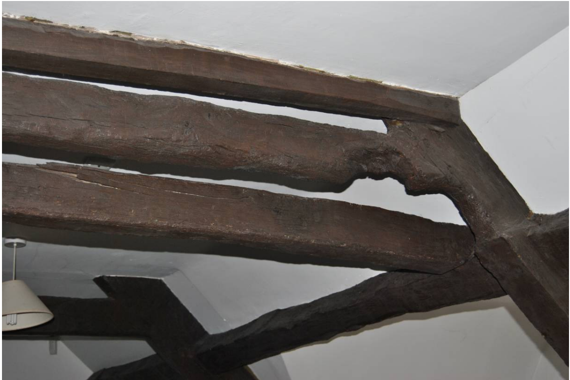
Plate 93: Fire damage to truss T8 [S.01].
