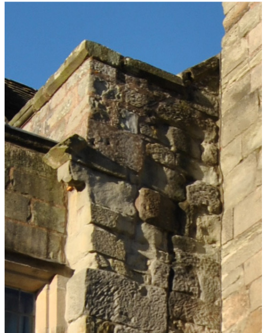
Plate 15: Rebuilt/raised eaves at SE angle; drip mould related to former Music Room extension.
