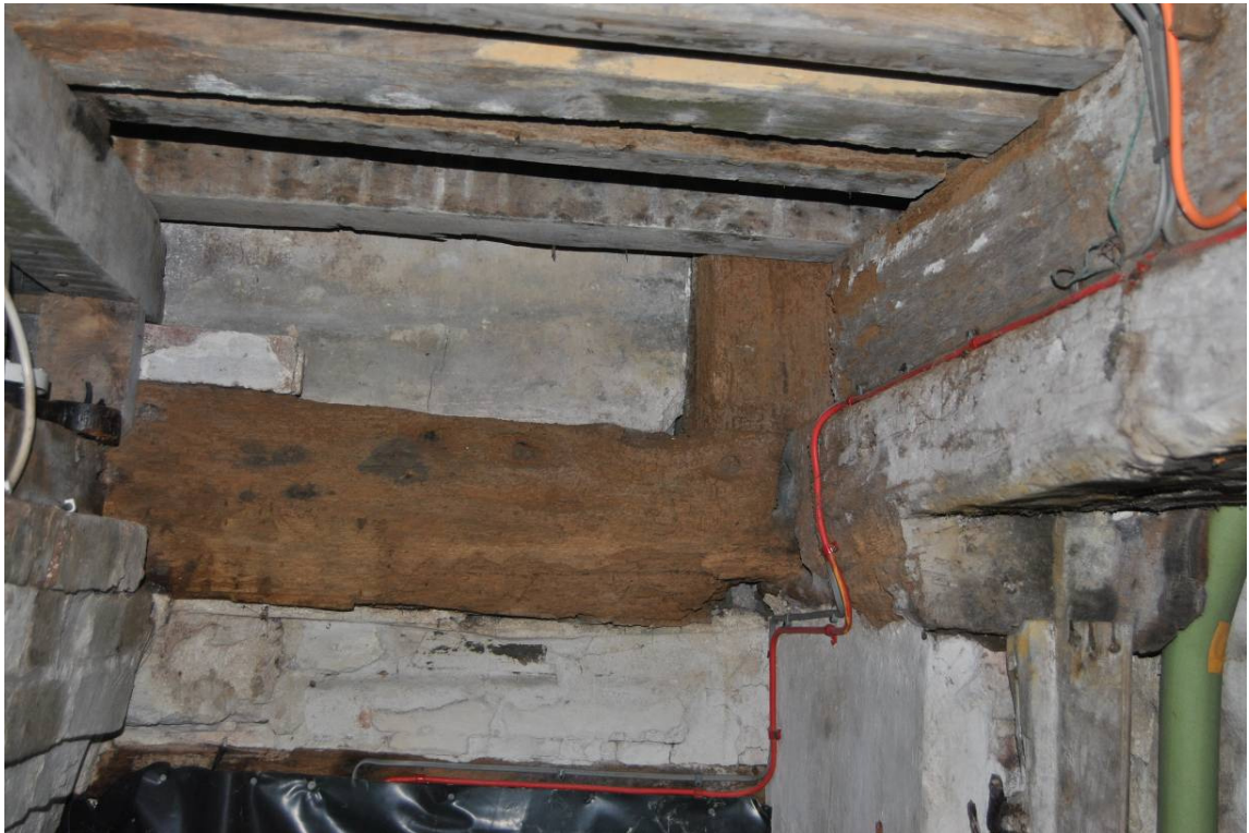
Plate 108: Fragmentary remains of PHASE I cross frame, [B.05].
