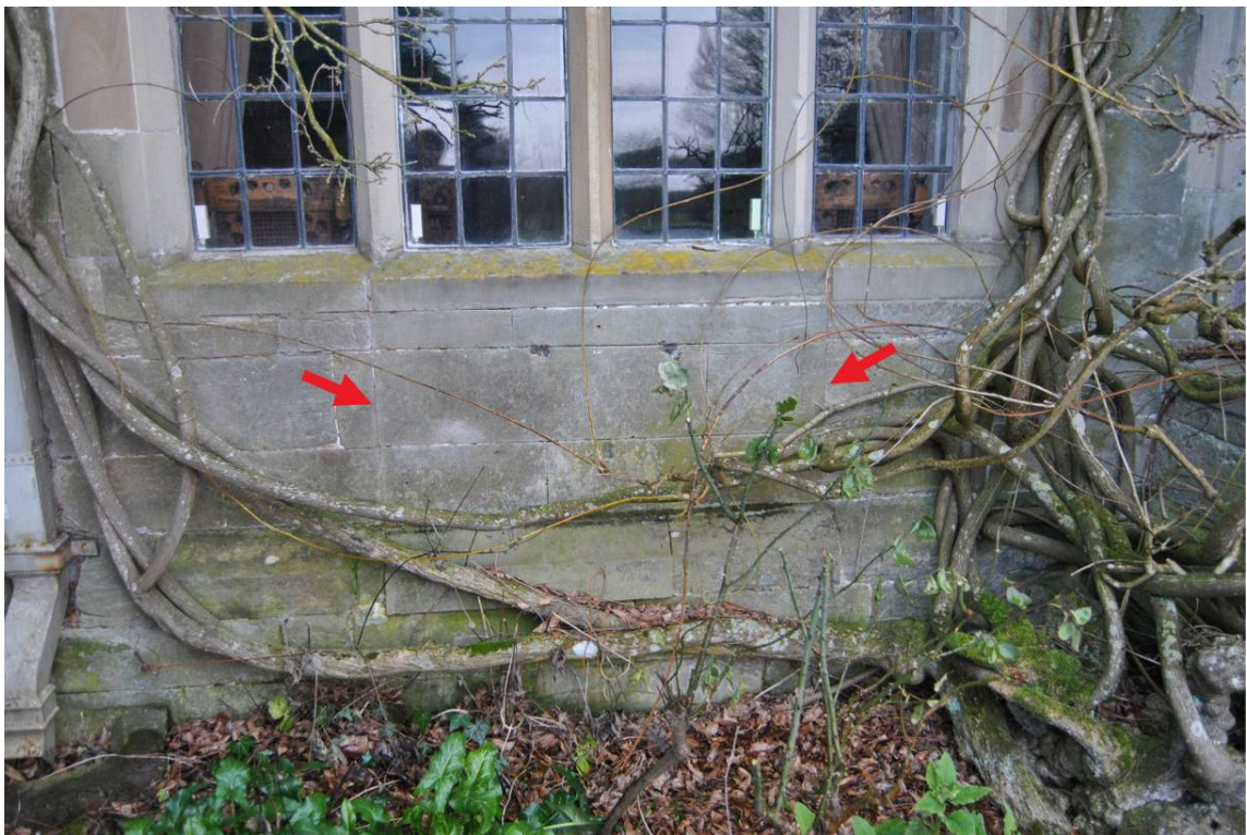
Plate 9: Detail of south wall between parlour wing and eastern canted bay showing paired straight joints (arrows) beneath window [w3] evidencing former doorway (See Figure 7a). Note also the three fixing points beneath central mullion possibly related to sundial shown in view of 1840 (Figure 7b).
