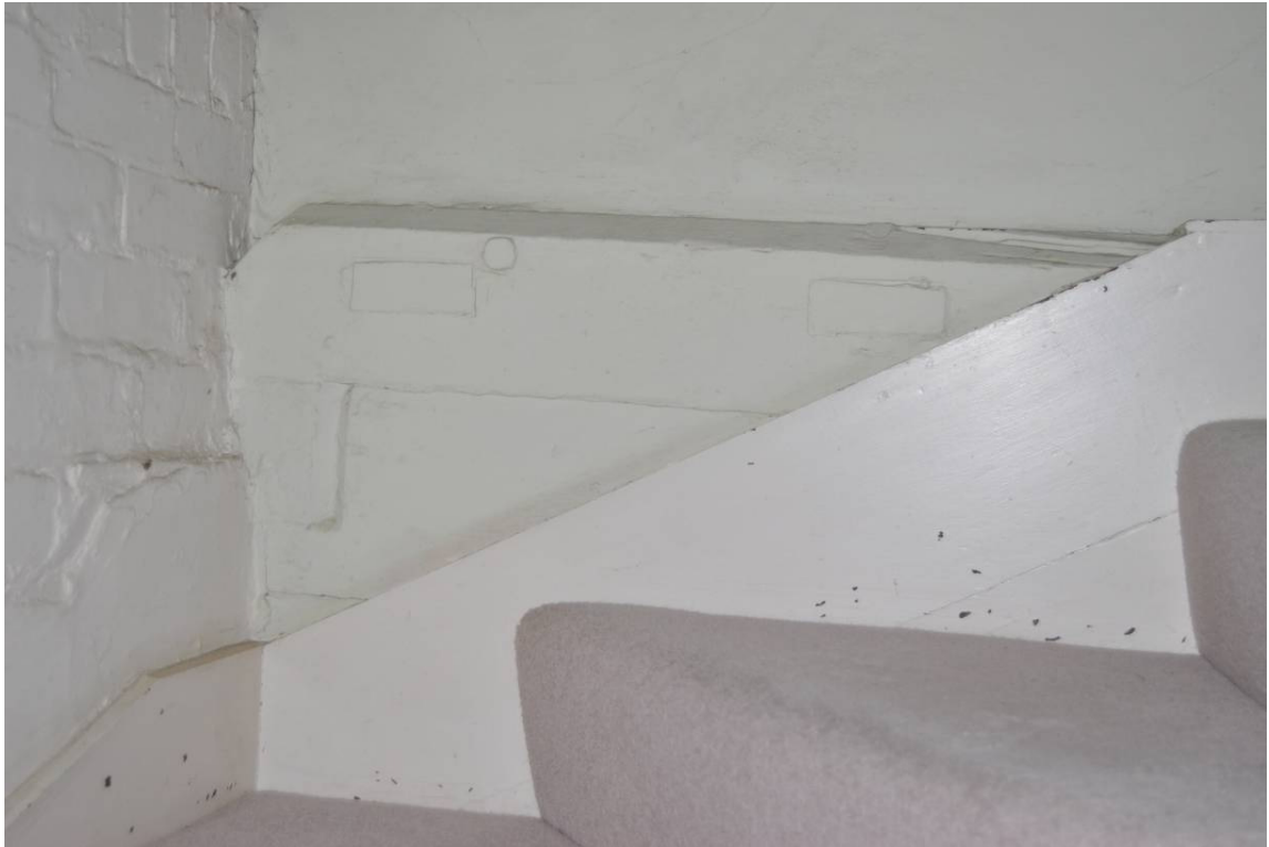
Plate 127: Cut-off joist tenons in PHASE I transverse beam at head of inserted stair.
