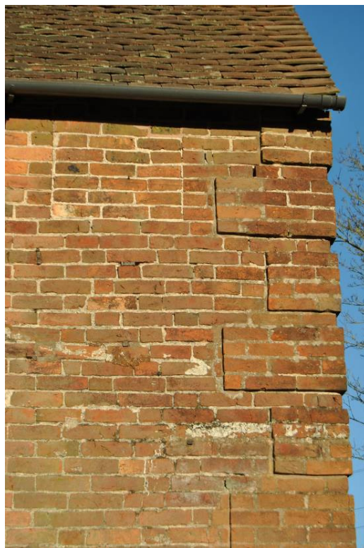
Plate 104: Detail of rusticated quoins and blocked opening to 1F level.
