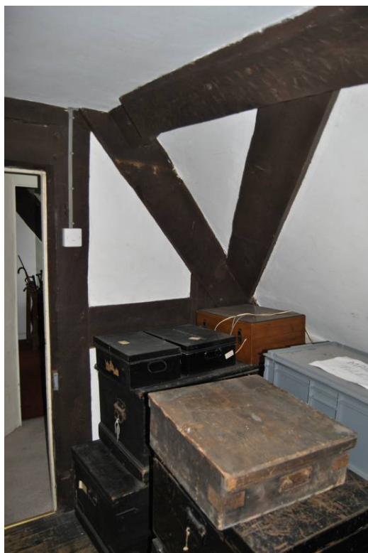
Plate 130: [S.06]; wind-bracing at Bay 2 (NE).
