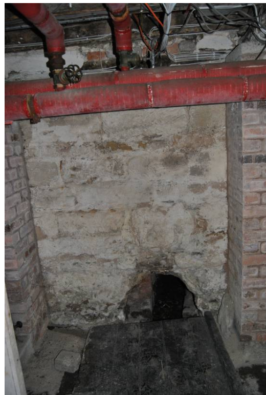
Plate 29: Basement [B.02]; drainage channel to base of east wall (extends under hall).
