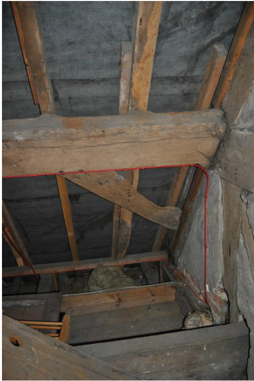
Plate 134: [S.10] (SW); butt-purlin and wind-brace.
