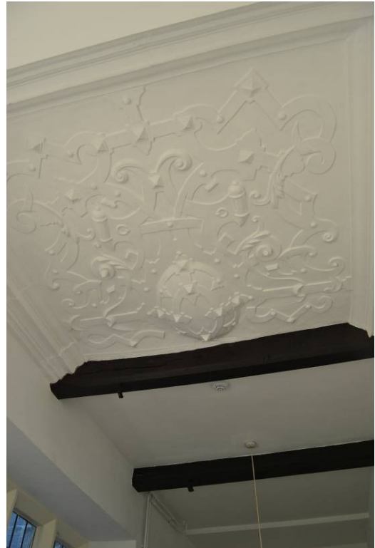
Plate 66: [G.06]; strapwork ceiling panel matching [G.05]. NB. transverse beams (?rel. C19 th inserted stair).
