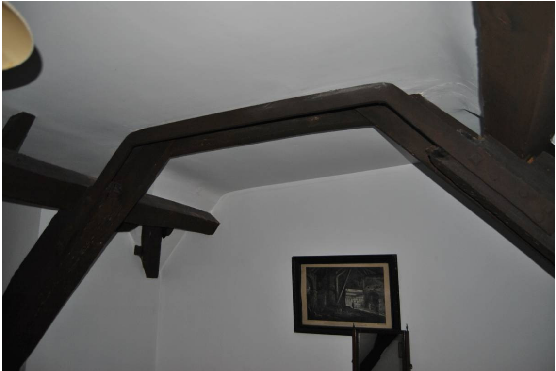
Plate 91: Fire-damaged principals and iron strapping to roof-truss T16 in [S.03].
