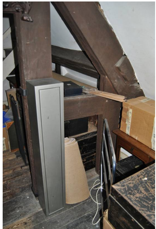
Plate 129: [S.06]; truss T1, queen-strut and princess-post with mid-rail.
