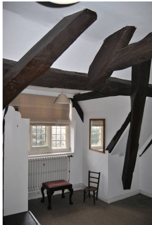
Plate 95: Inserted braces at T9, [S.01]
