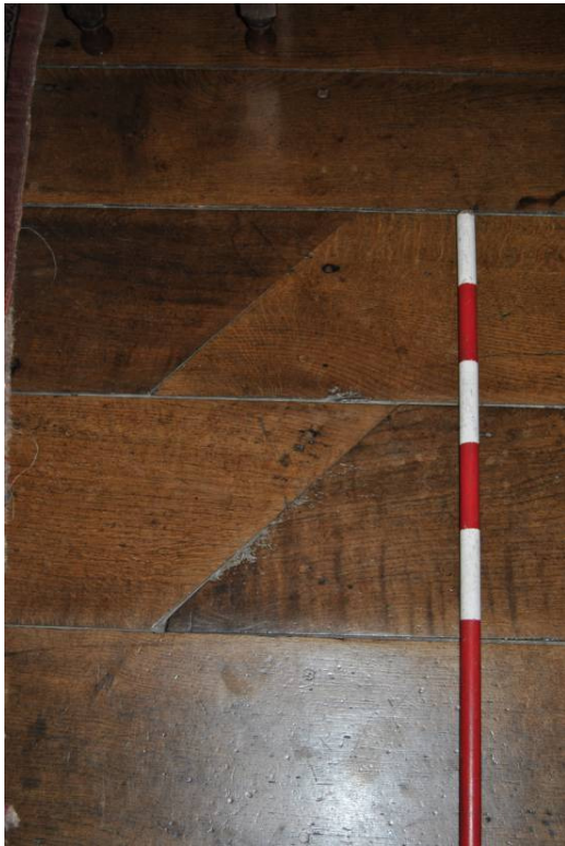
Plate 62: [G.05]; detail of angled butt-joints in floor.
