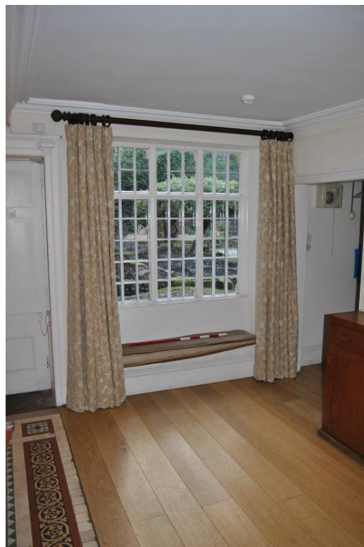
Plate 112: [G.08] looking north-west. NB: north edge of tiled floor respects line of former partition (Figure 14).
