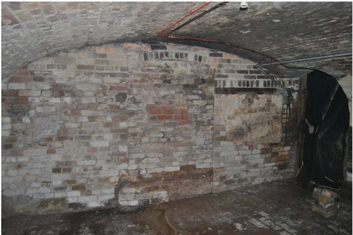
Plate 110: Blocked doorway and window openings in east wall of basement room [B.06].
