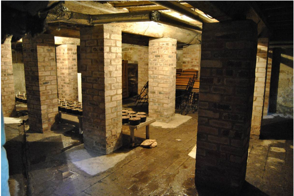
Plate 30: Cellar [B.01]; inserted brick piers (1960s) support re-used timber beams.
