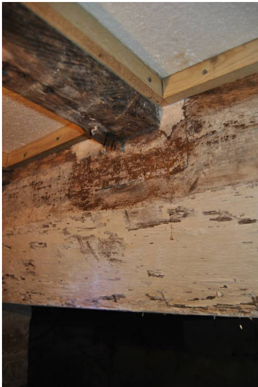
Plate 31: Deeply chamfered floor beam with ogee-stopped common joist (secondary).
