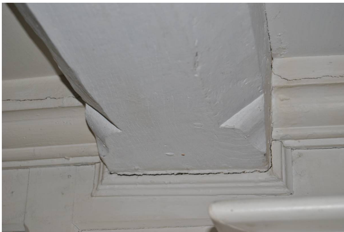
Plate 123: [F.11]; ogee-stopped ceiling beam.
