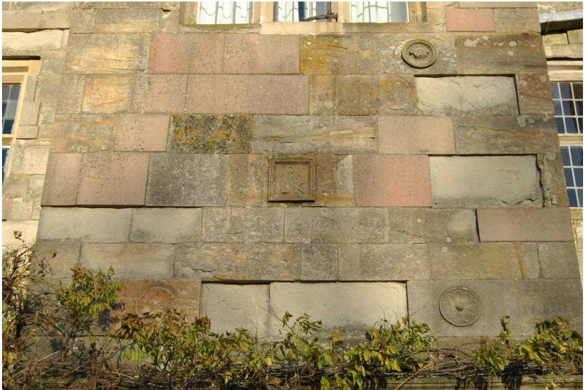
Plate 10: Moulded stones including rosettes and central initialled plaque 'BLK', arranged in form of 'quincunx', NB: top left stone missing.
