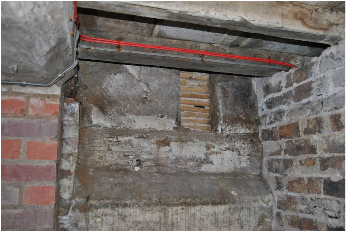
Plate 107: PHASE I framing exposed within [B.04] (west wall); cill beam, down braces and base of close-studwork.
