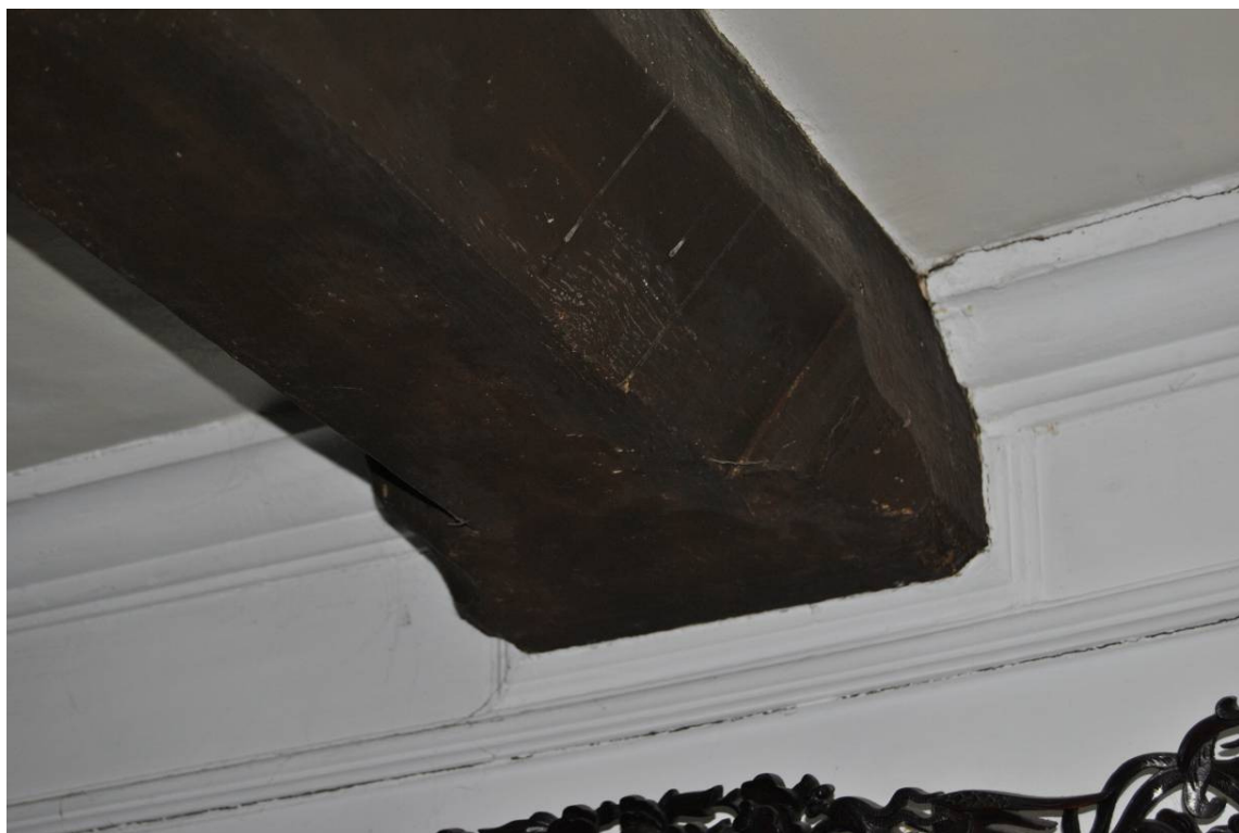
Plate 120: Detail of ogee-stopped ceiling beam to [F.09].
