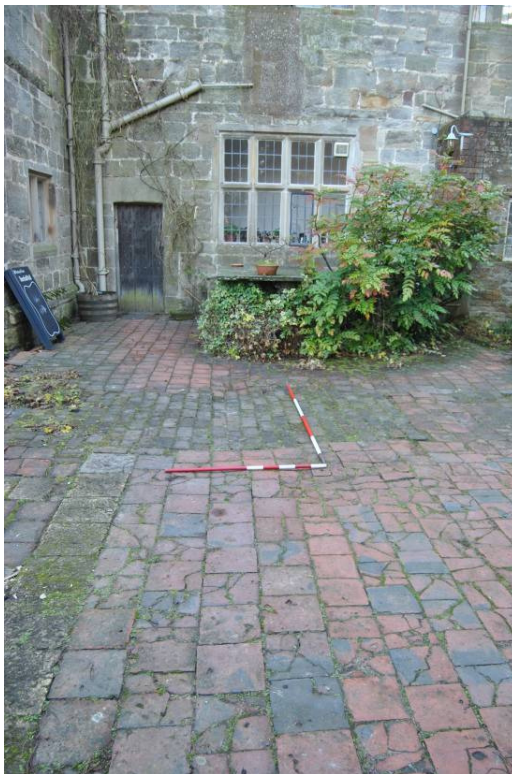
Plate 21: Quarry-tile and brick floor of former north-west range
