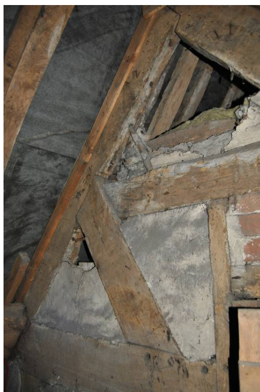
Plate 133: [S.10]; western truss T4 with v-strutting and wattle and daub infill panels
