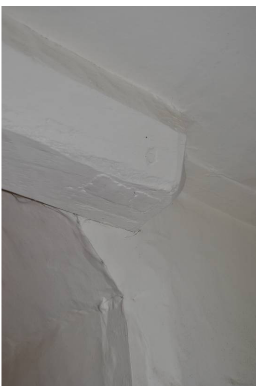
Plate 118: [F.10] primary beam truncated for insertion of stair.
