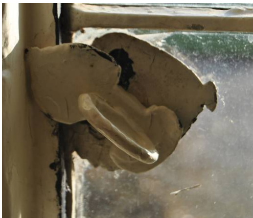
Plate 38: Standard primary turnbuckle catch.
