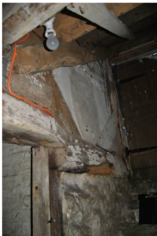
Plate 106: Relic PHASE I framing exposed in east wall of stair (cill beam and down bracing)
