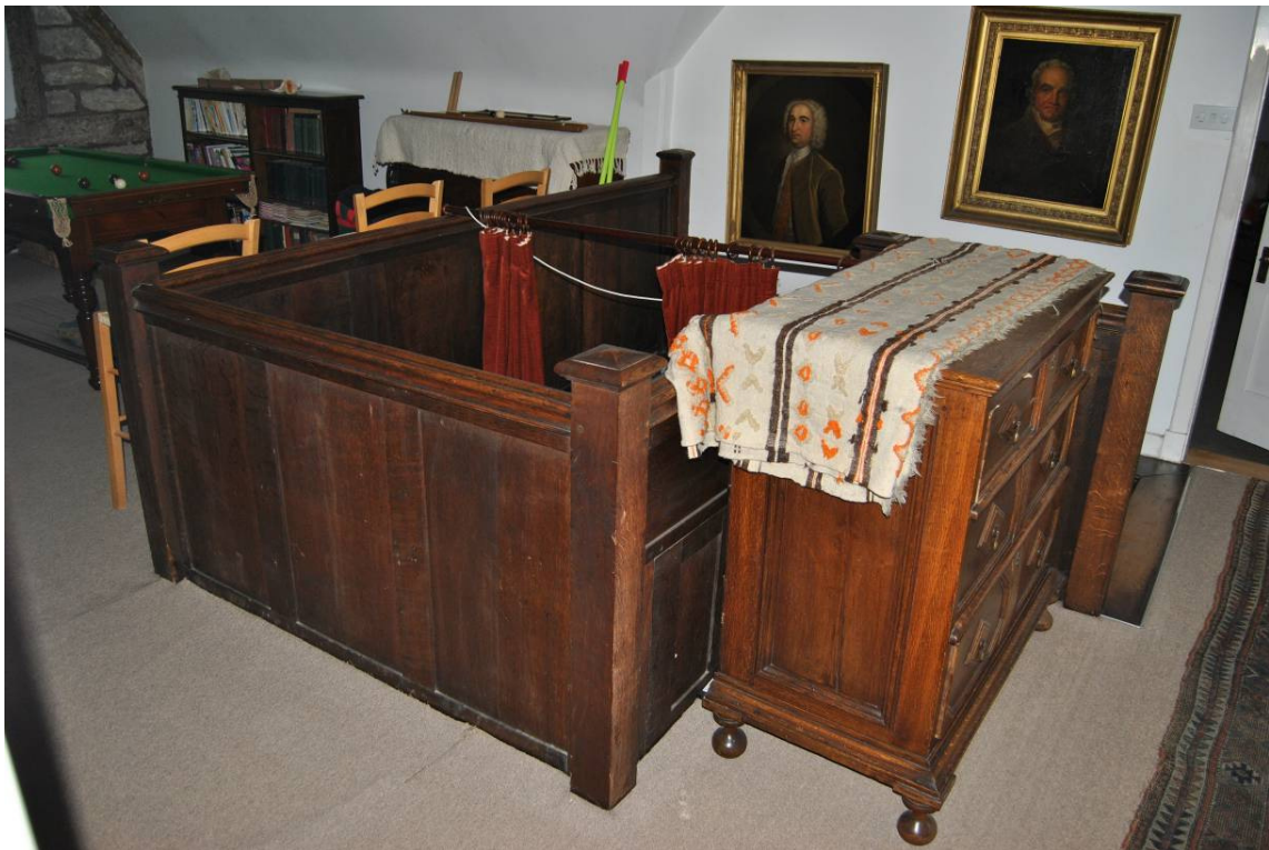
Plate 87: Rebuilt head (after 1818 fire) of principal stair at [S.02].
