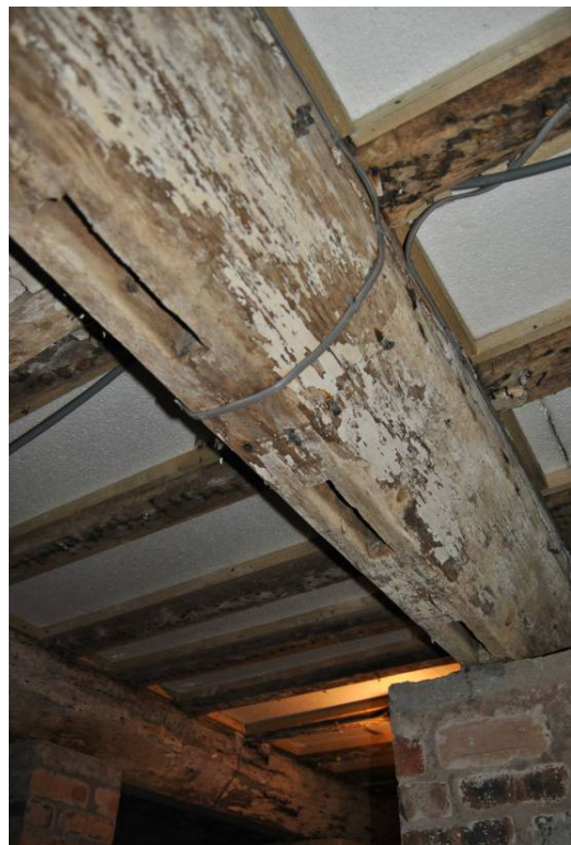
Plate 32: Redundant post-mortices to soffit of deeply chamfered floor beam (?part of screen).
