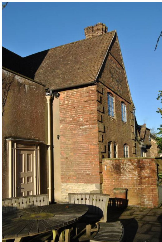
Plate 103: Phase II projection, encased in C18 th - brickwork.
