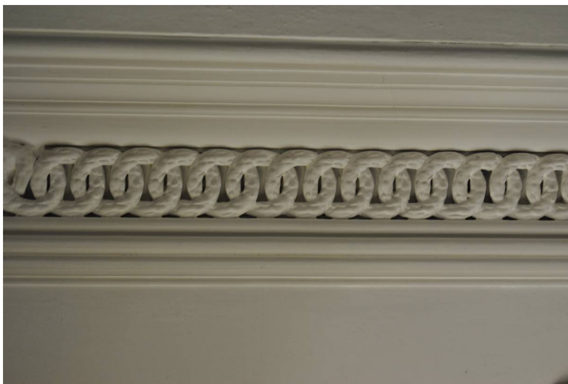
Plate 51: Plasterwork cornice moulding to [G.03].
