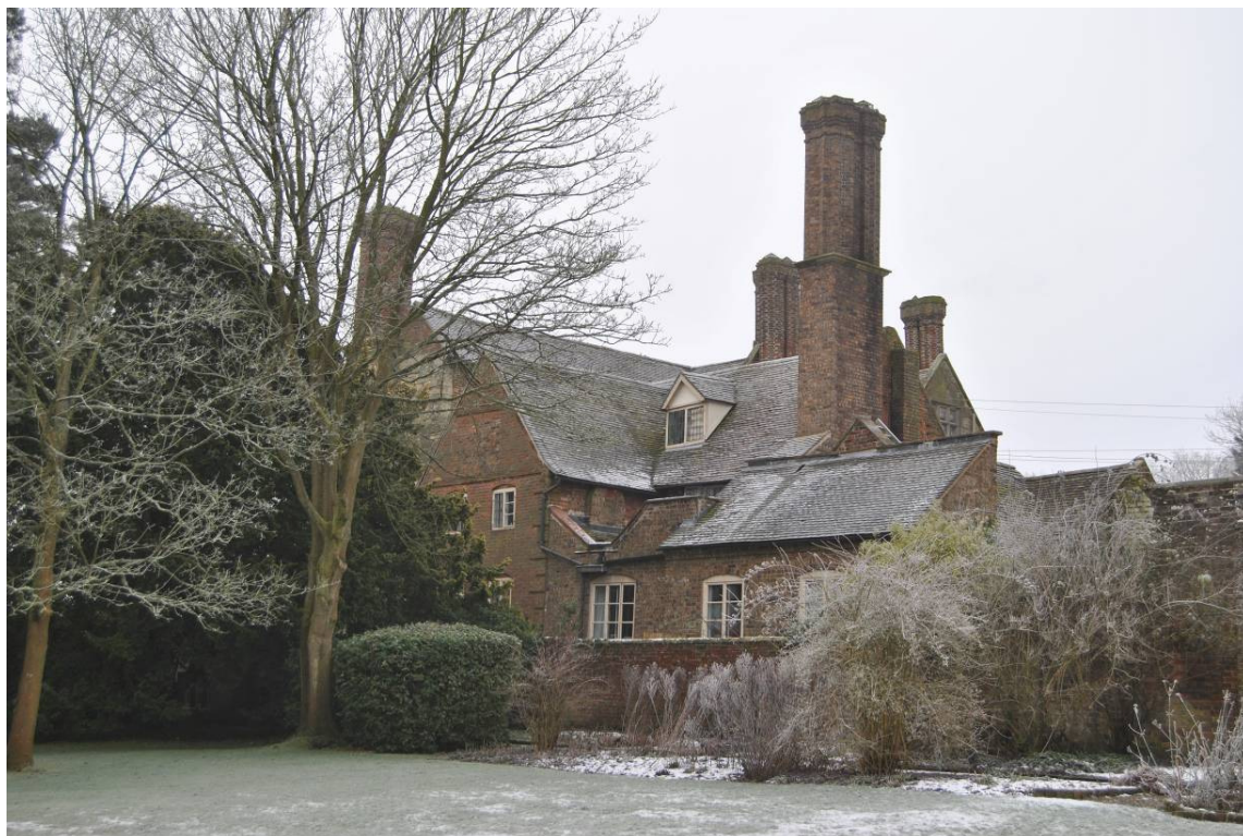
Plate 101: North-east range, east elevation, oblique looking south-west. NB: truncated stack to north elevation of projecting gable. Single-storey, Broseley-brick ranges date to later C19 th (Phase VIb).
