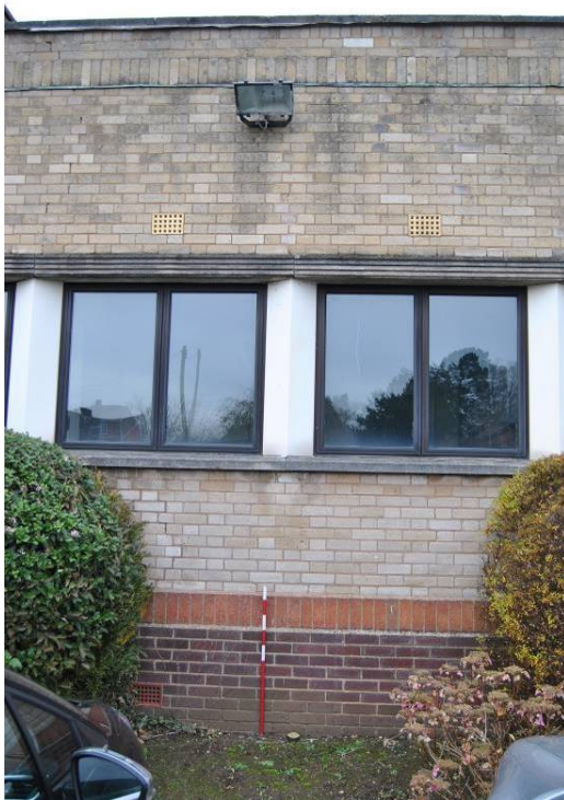
Plate 4: Representative section of walling with purple, stretcher-bond plinth.
