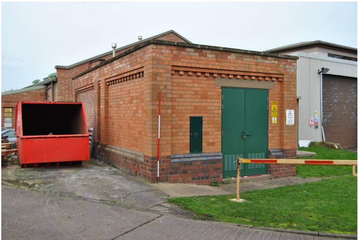
Plate 64: Electricity sub-station (Red Hill S/S 33497), 1935 extended 1942 (PA 7765).
