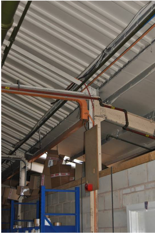
Plate 38: Secondary rakers (right) over 1944 extension to western side of print works.
