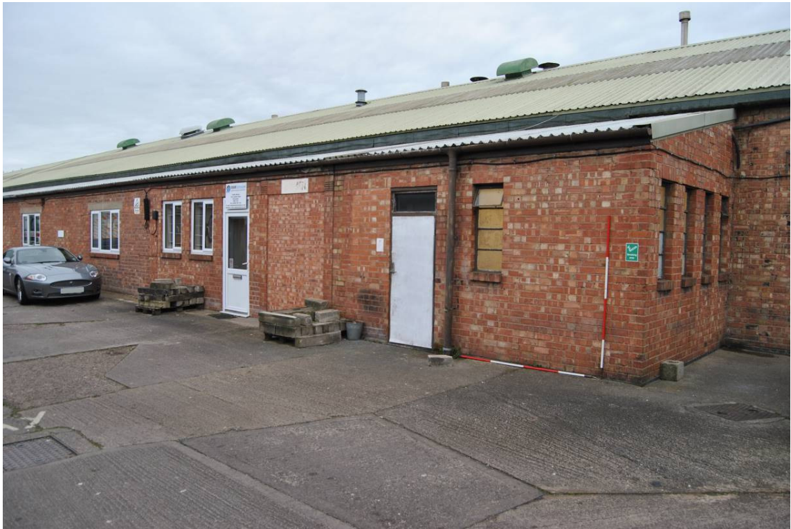
Plate 26: Primary female entrance and toilet/cloakroom block to west side of print workshops.
