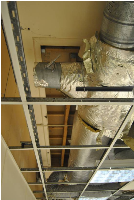
Plate 17: Original sky-light visible above inserted ceiling.
