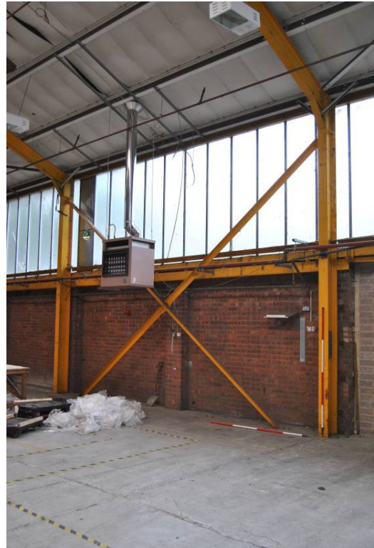
Plate 52: Interior of storage range K1; east wall with glazing above eaves level of adjacent range (G).
