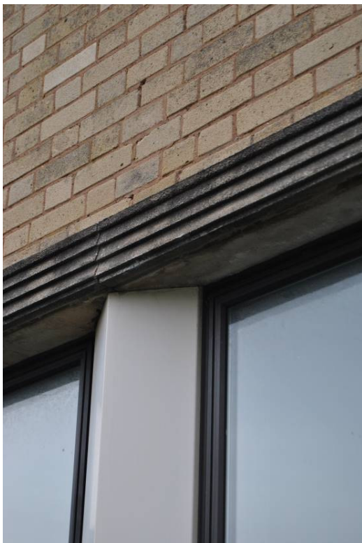
Plate 7: Detail of moulded, cast-concrete window head.
