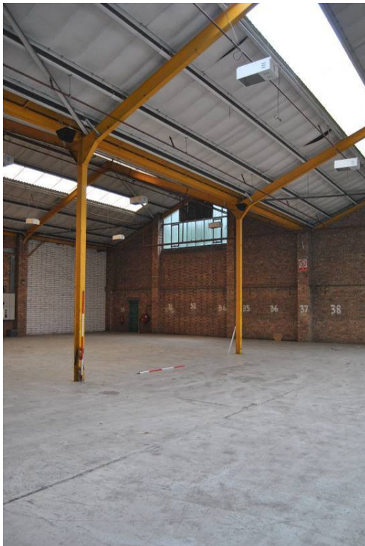
Plate 51: Interior of 1960s storage range K1 looking north-west.
