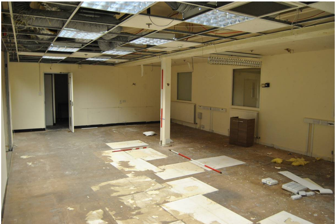
Plate 14: Former general office looking west (original north wall removed; supported by column).
