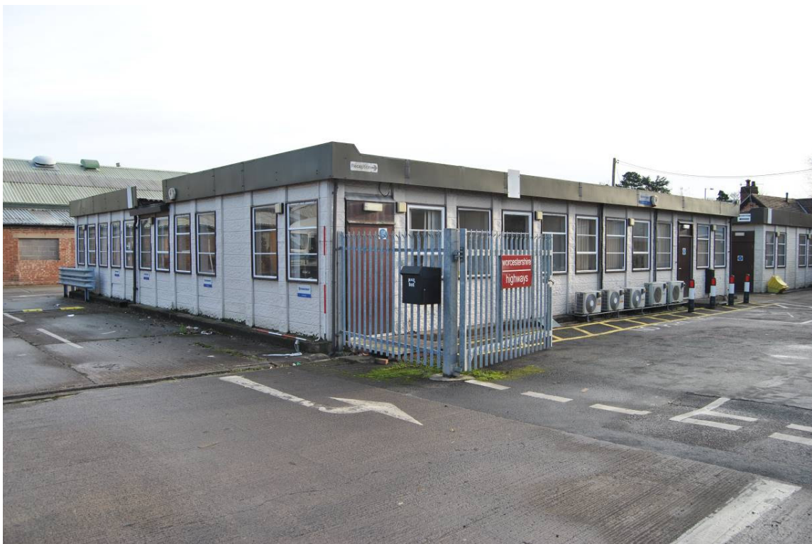
Plate 59: 'Ringway' building (M; Figure 10); modular, pre-fab 'Banbury superspan' construction (1964/69) looking south-east.
