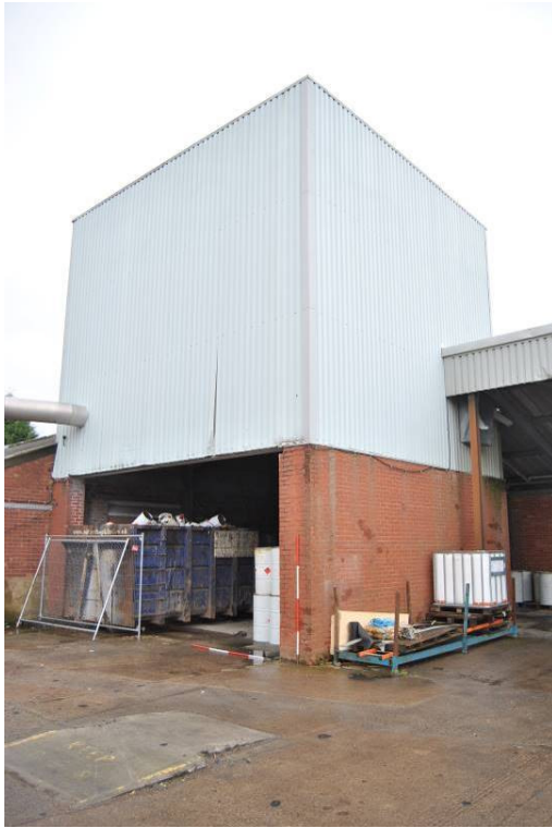
Plate 62: Housing for former cyclone extractor (N).
