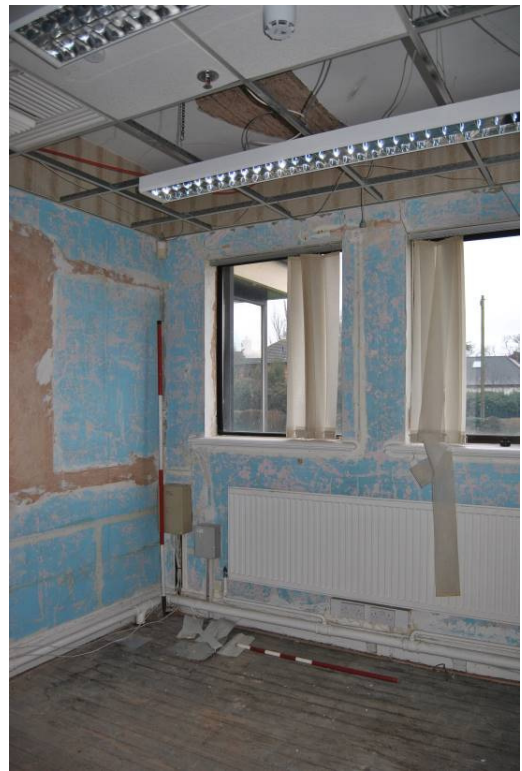
Plate 13: Primary office space, NB. original lath and plasterwork above inserted suspended ceiling.
