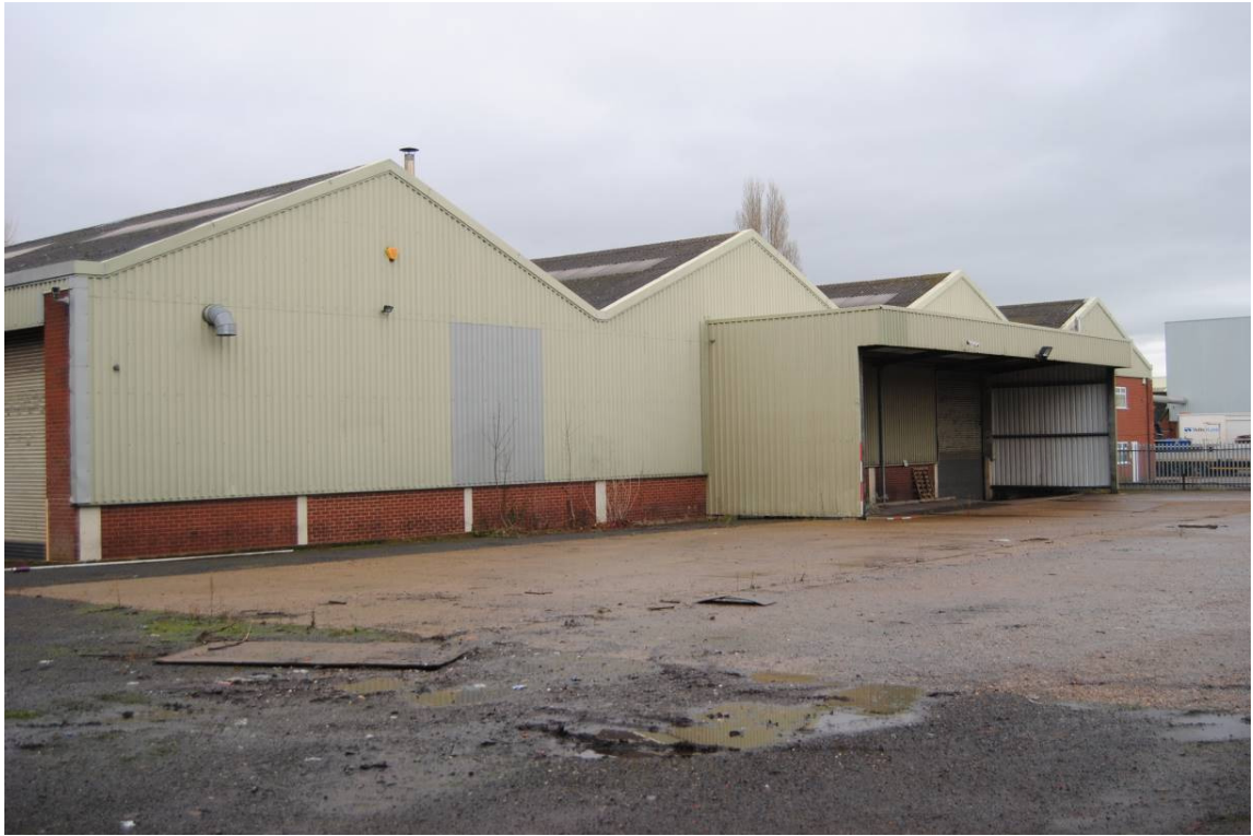
Plate 55: 1970s paper storage ranges (K2/3; Figure 10) looking north-east.
