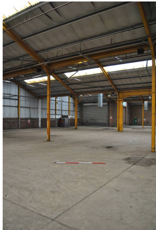
Plate 57: Interior of 1970s paper storage ranges (K2/3; Figure 10) looking south-west.
