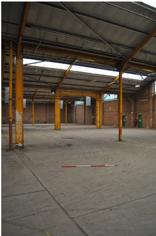
Plate 56: Interior of 1970s paper storage ranges (K2/3; Figure 10) looking north-west.
