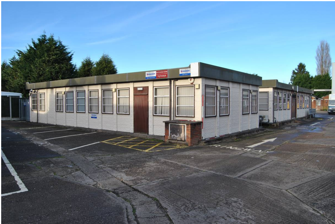
Plate 58: 'Ringway' building (M; Figure 10); modular, pre-fab 'Banbury superspan' construction (1964) looking north-west.
