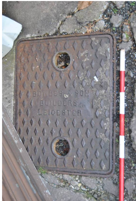
Plate 8: Inspection cover adjacent to office range, embossed 'Bowles and Son, Leicester' (original contractors - see Figure 7b).
