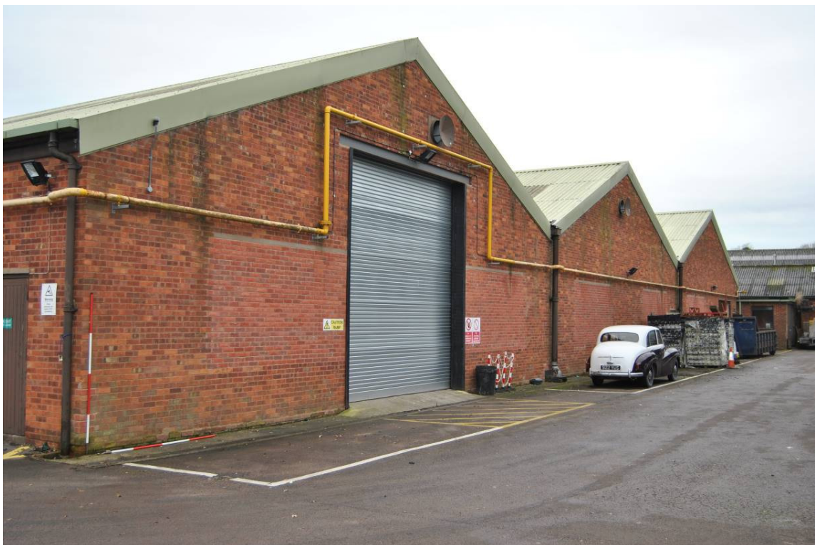
Plate 46: 1964 northern print shop extension (H; Figure 10) looking south-west, NB. inserted roller door (see Plate 44) and blocked primary windows.
