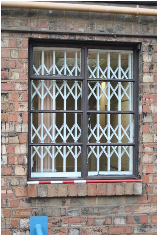
Plate 22: Original, steel-framed window.
