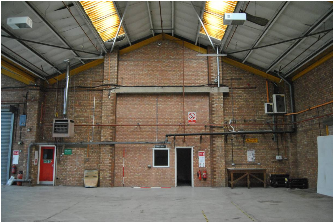
Plate 53: South gable of 1960s paper storage range; former loading door with concrete lintel, infilled for creation of two-story office (L; Figure 10).
