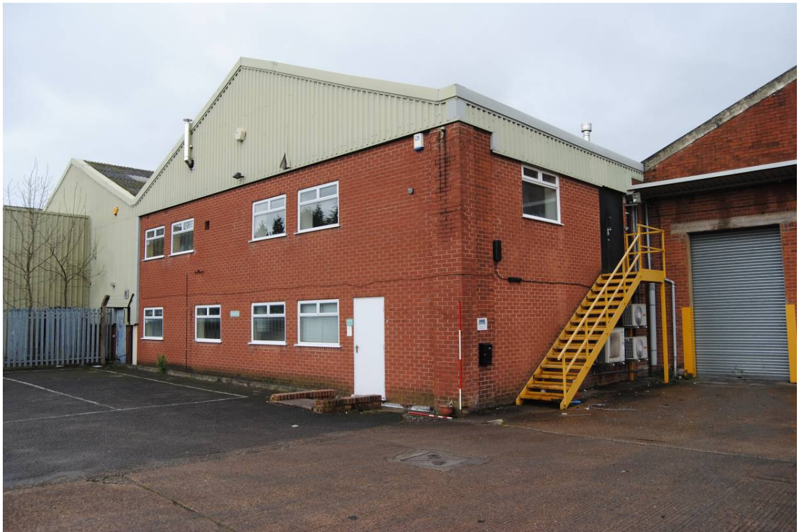
Plate 54: Two-storey office block (L; Figure 10) formed in angle of 1960s/70s paper storage ranges.
