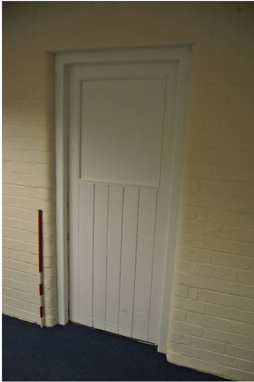
Plate 34: Primary door with bull-nose jambs opening onto corridor B1, formerly directly to main print works.
