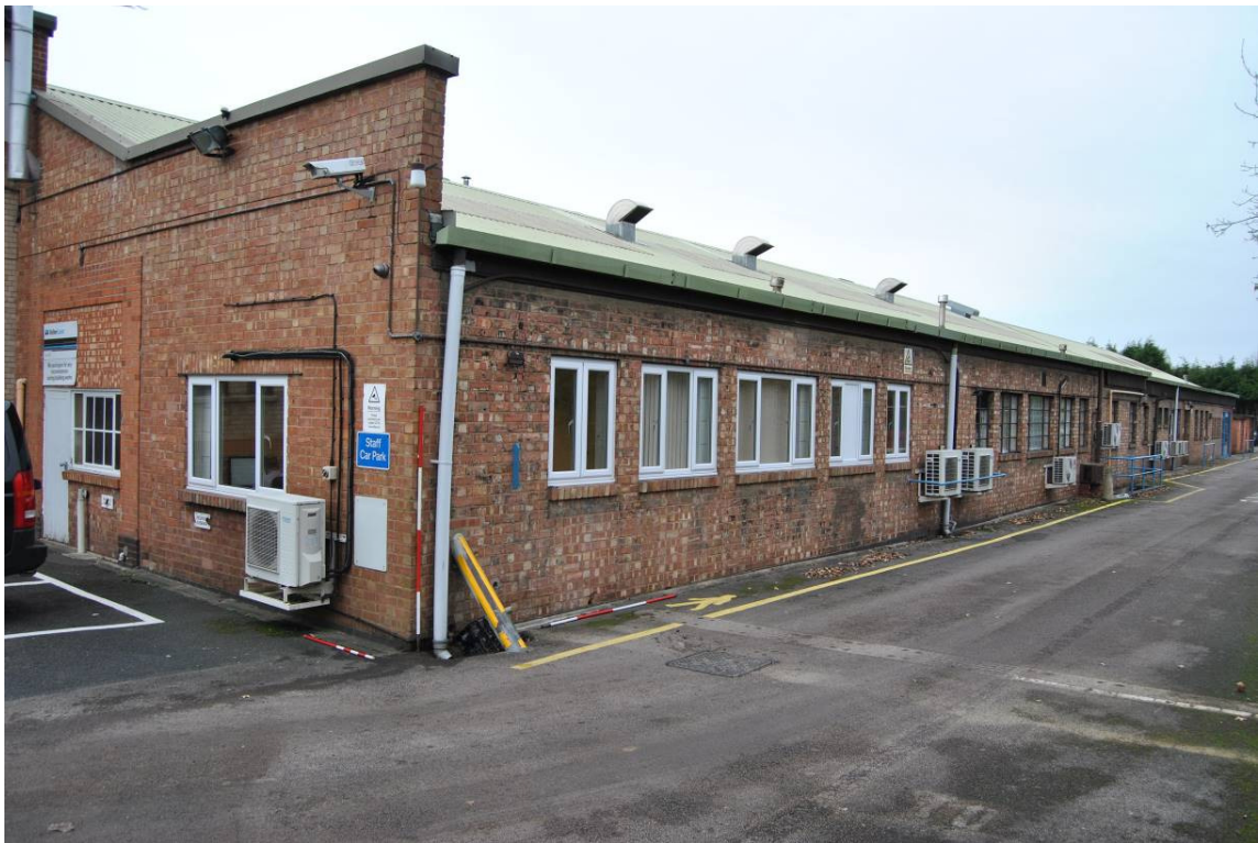
Plate 20: Range of offices etc. flanking eastern side of primary printing shops, looking north along eastern access road.
