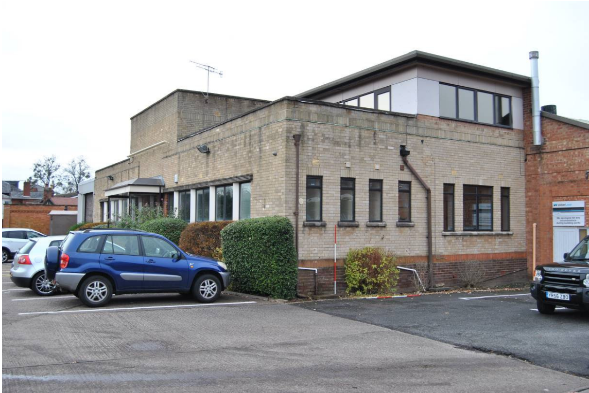
Plate 6: Oblique view of office range showing 1995 1F extension.
