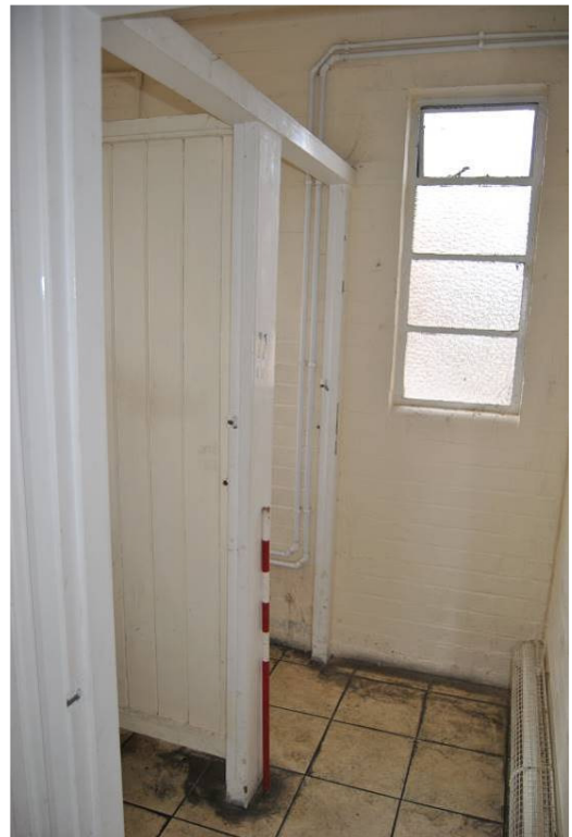
Plate 37: Primary timber partitions to original female toilet block.
