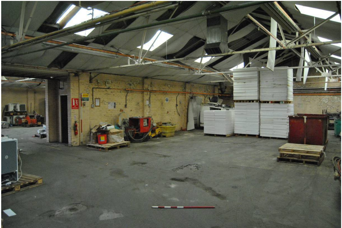
Plate 40: 1950s paper storage range (G; Figure 10); interior looking north-west.
