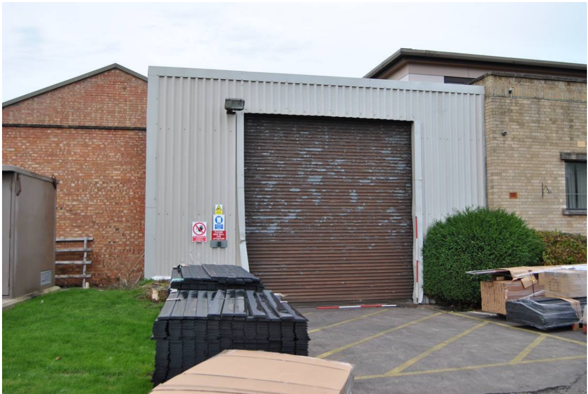
Plate 63: Covered loading bay (O) to west of office range.
