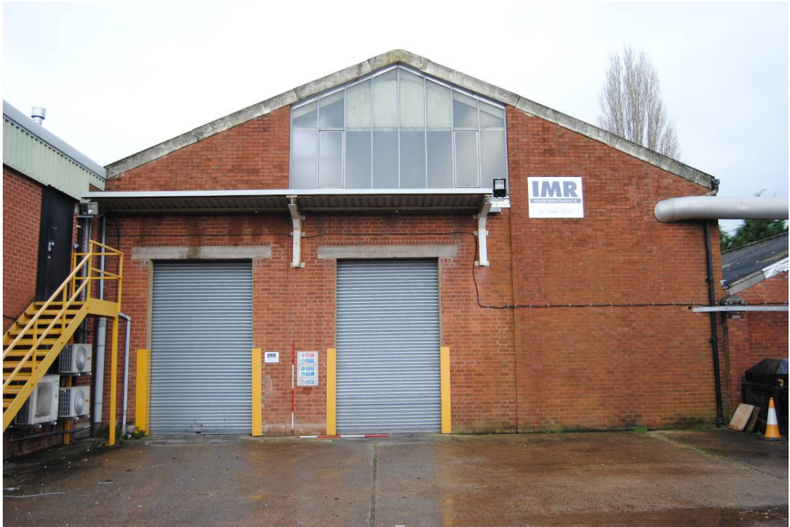
Plate 50: South gable end of 1960s paper storage range (K1; Figure 10).
