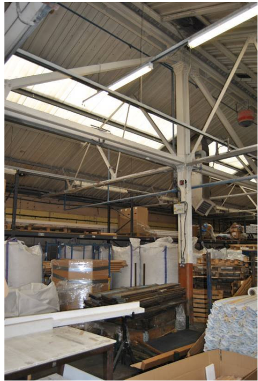
Plate 32: Longitudinal trussed-girder supported by primary steel stanchion.
