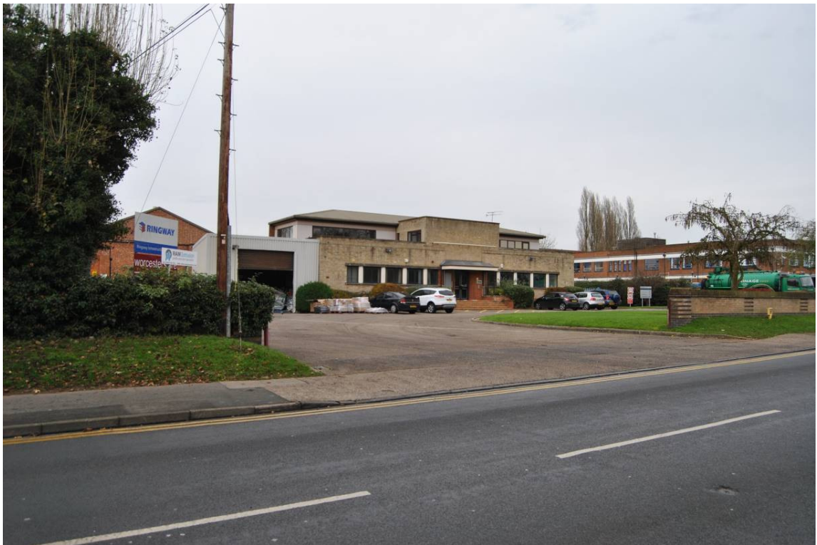
Plate 2: Contextual view of works from London Road, looking north-east (compare Figure 7b).
