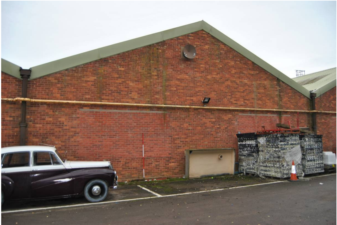
Plate 47: Detail of central range showing blocked windows x 2 (see Figure 15b).
