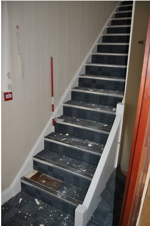
Plate 15: Stair rising to first floor offices (1955).
