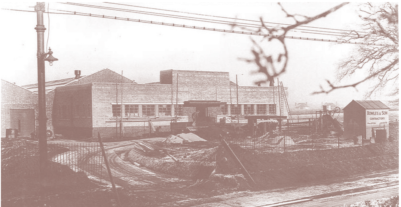
Trinity Press under construction, December 1935
