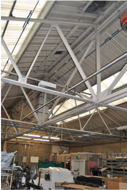
Plate 31: Detail of roof truss and longitudinal trussed-girder.
