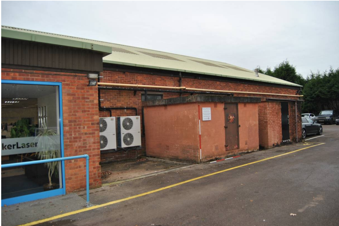
Plate 45: 1961/4 print shop extensions (F/H; Figure 10) and fuel/solvent stores.
