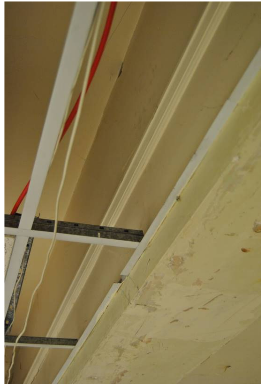
Plate 16: Picture rail and original ceiling visible above modern suspended ceiling.
