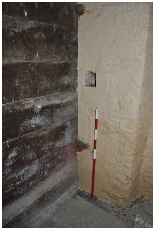
Plate 35: Hole for draw-bar within western jamb [d1].
