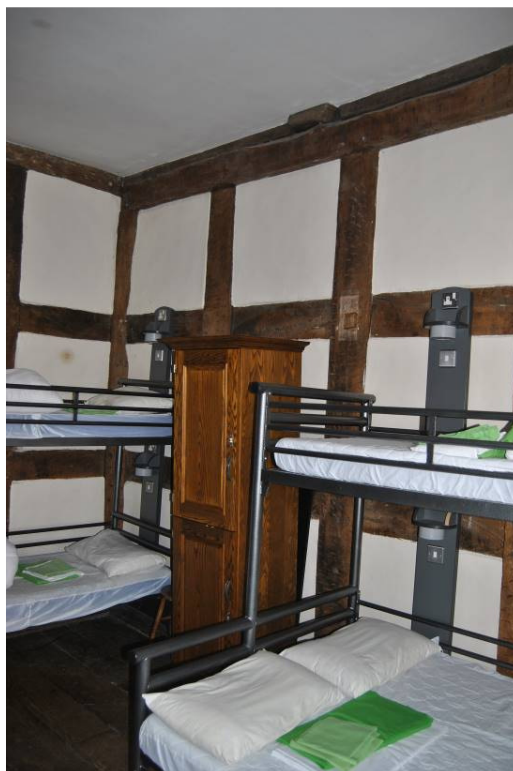
Plate 83: Room [F5], looking north-east, NB. transverse ceiling beam of parlour wing lodged over top-plate of wall frame.
