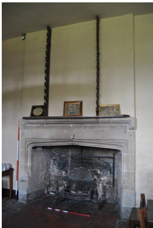
Plate 50: Main FP in lateral wall with bow-rack over and iron pot-crane.
