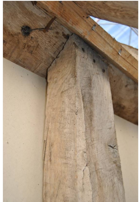
Plate f. stud nailed at upper purlin.
