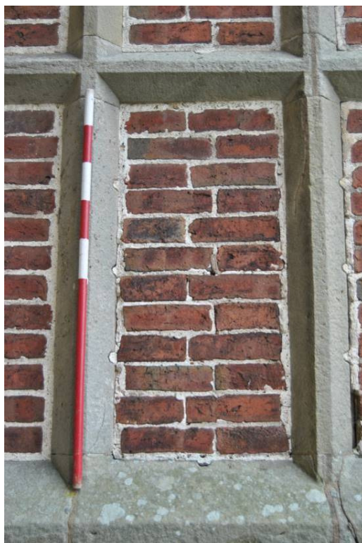
Plate 13: Detail of brick blocking showing evidence for former standard and saddle bars.
