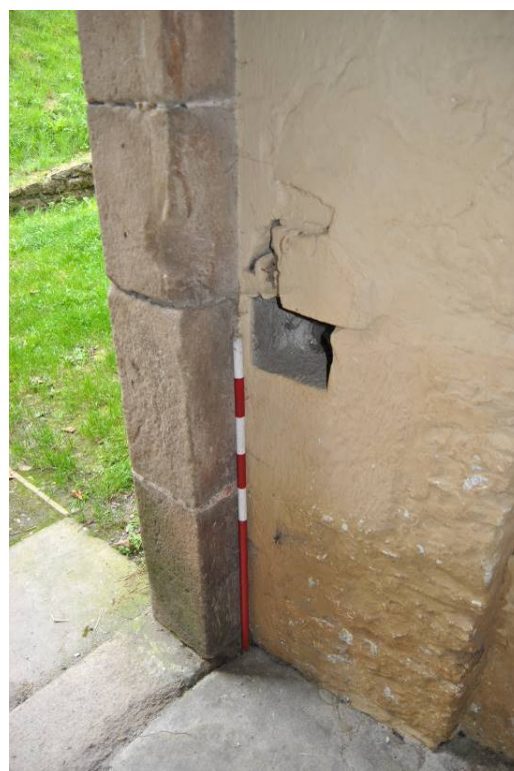
Plate 38: Hole for draw-bar within eastern jamb [d2].
