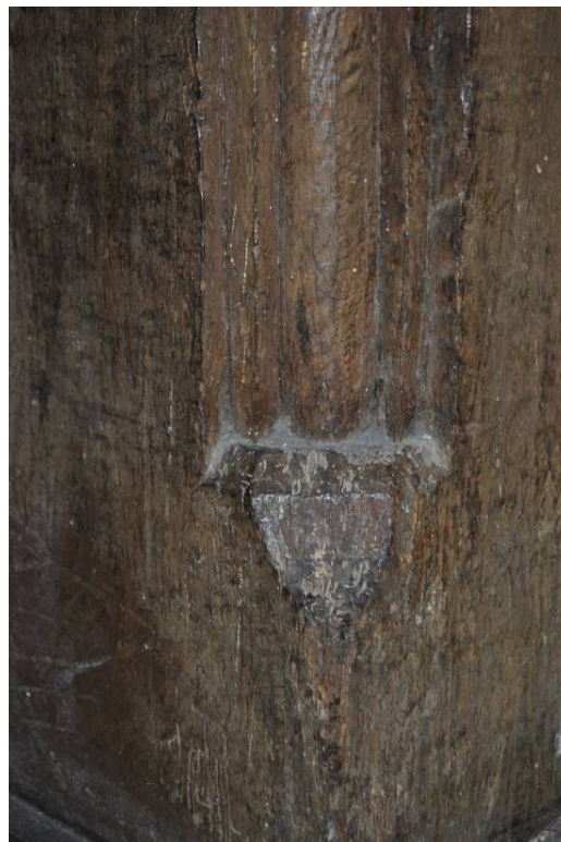
Plate 77: Bold ovolo moulding and run-out stop on corner post of 1F framing [F6].
