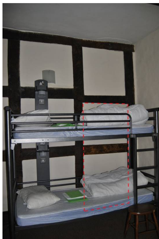
Plate 94: Partition between [F11/12]; former door to right, outlined in red; NB. dropped rail over.
