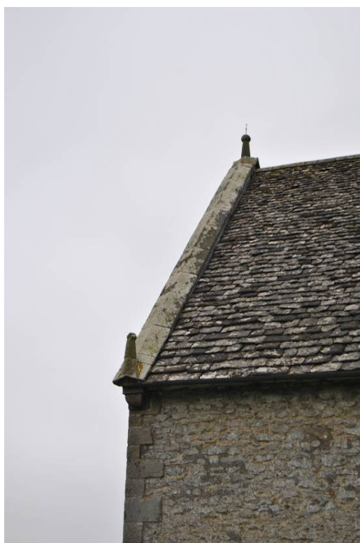
Plate 4: Detail of stone coped gable (service wing).
