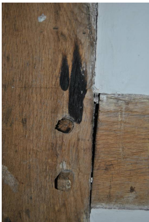
Plate 109: Detail of taper burn.
