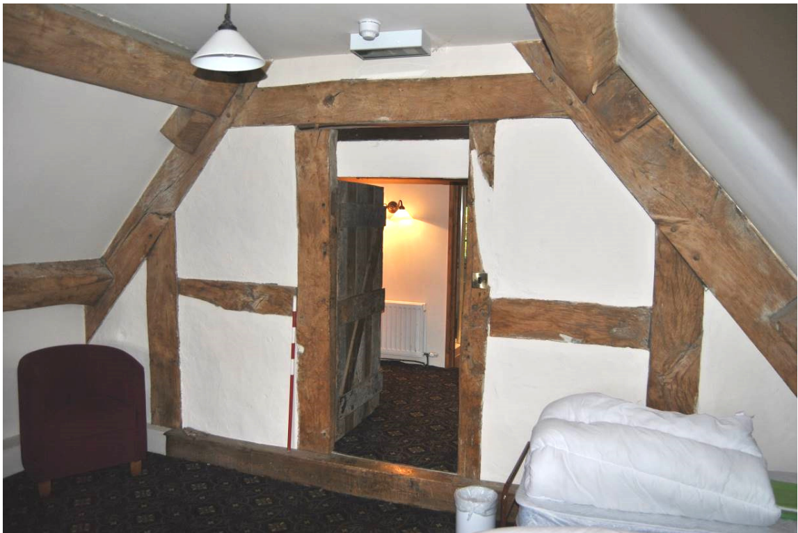
Plate 116: Infilled truss T6 between [S2/4]. NB. double purlin to south, single purlin to north.
