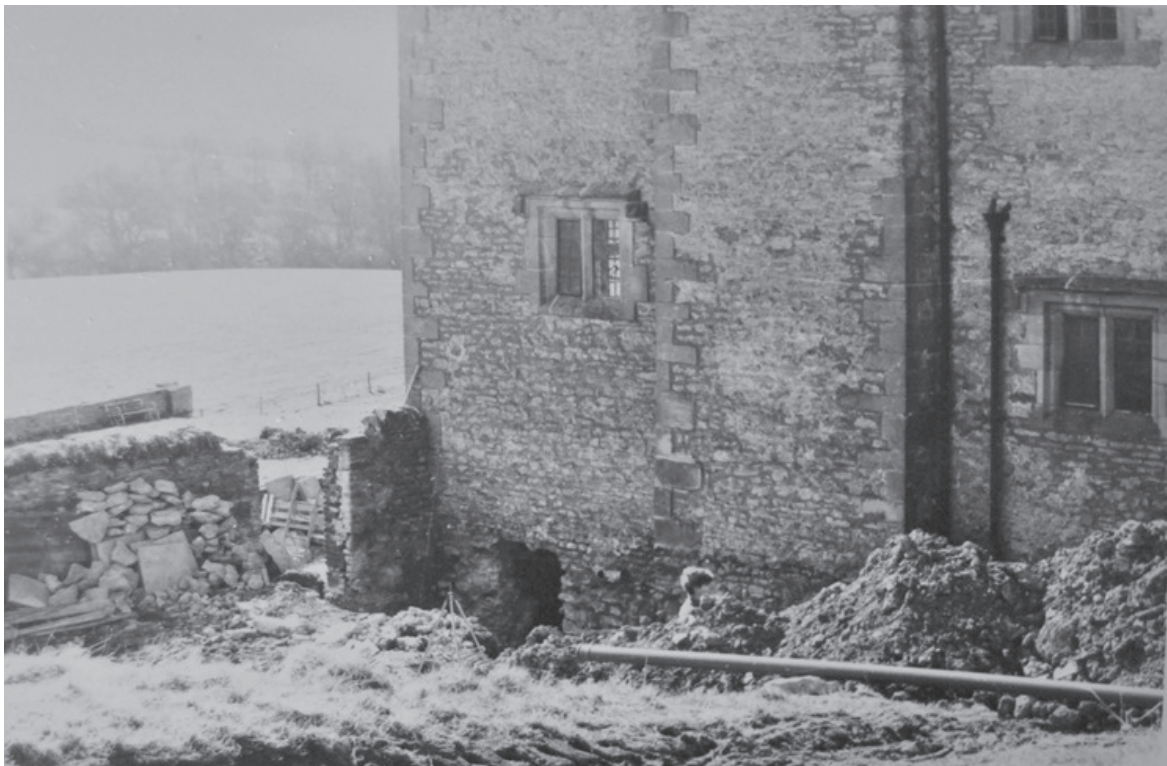
(b) Excavating steps to newly formed door into basement of east wing, 1975.
