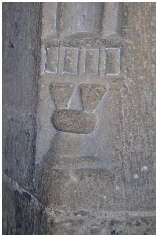
Plate 51: Detail of FP chamfer stop.
