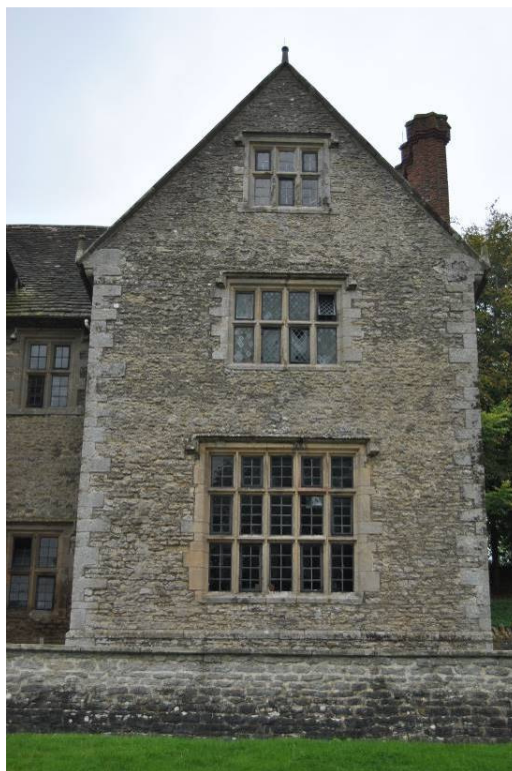
Plate 15: Eastern, parlour wing NB: diamond quarries to 1F window, w23 (see Figure 5b).
