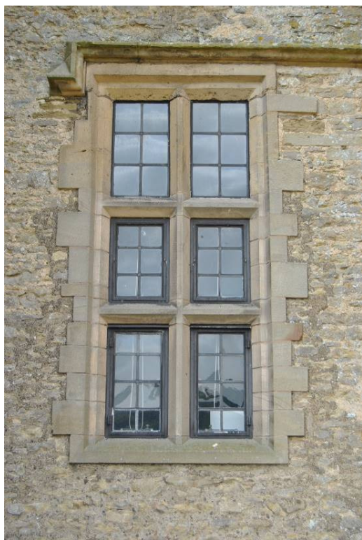
Plate 14: Enlarged window w3 lighting low end of hall, NB: small size of stones used in lower jambs.
