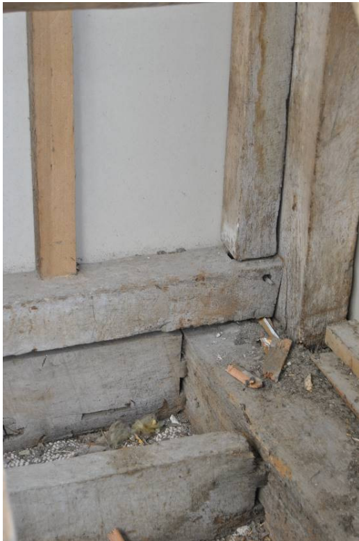
Plate e. Studs tenoned into independent cill set atop floor beam/tie-beam.
