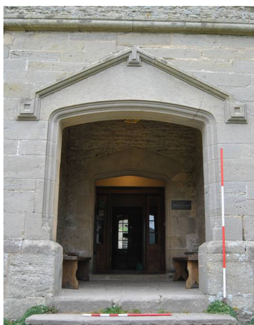
Plate 9: Principal doorway to porch tower with unusual detached pediment.
