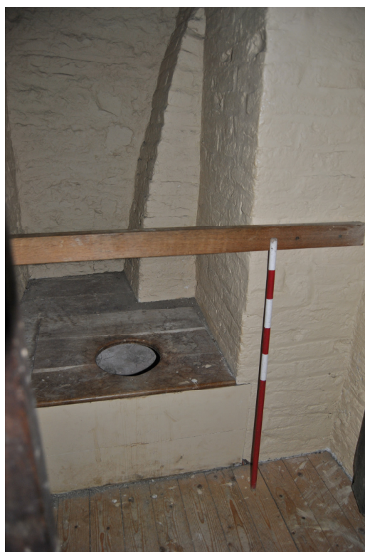
Plate 75: Garderobe [F10] (2F chute and vent to right -see Appendix D).
