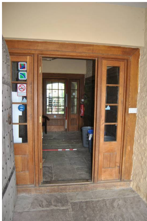
Plate 36: Cross-passage [G2] looking north with inserted fire partitions/doors.
