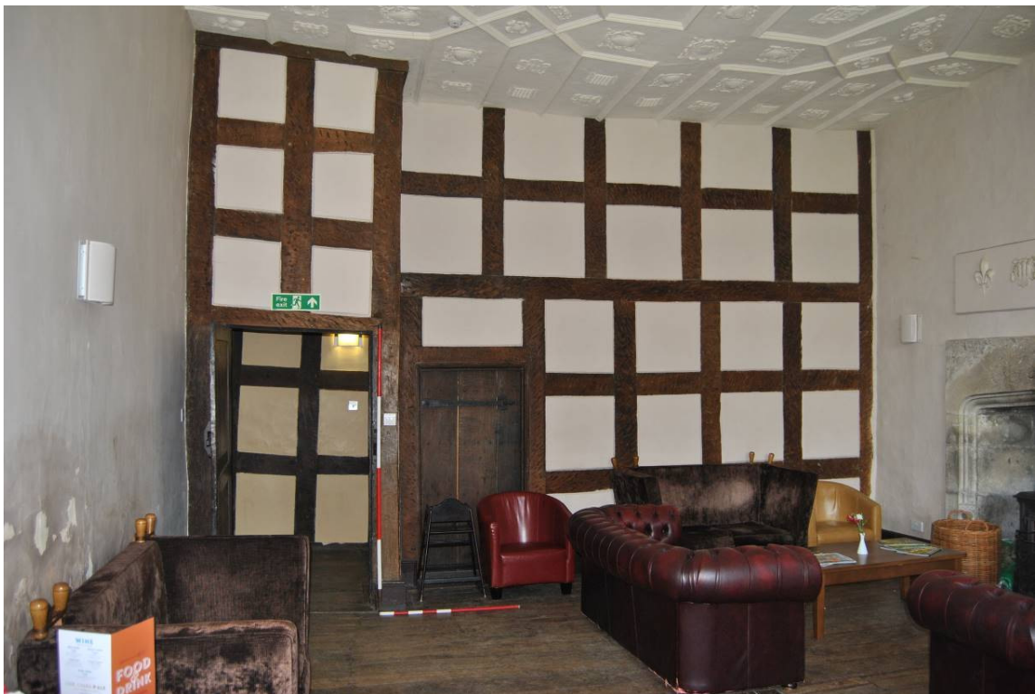
Plate 59: Timber-framed construction of north wall, Parlour [G8]; both door locations appear primary though d13 (left) has been adapted.
