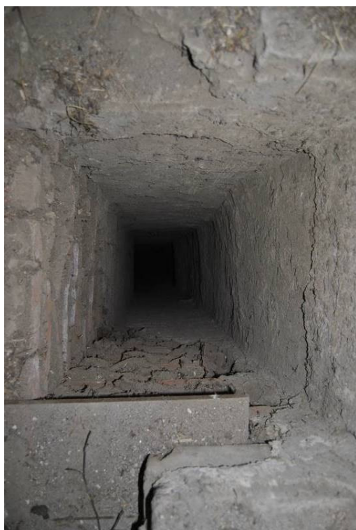
Plate i. 2F garderobe chute (foreground) and probable vent flue (left) with lintel.
