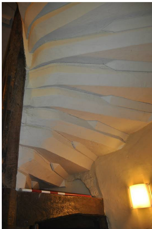
Plate 71: Soffit of solid oak treads, Stair A. NB. lower doorhead morticed into newel.
