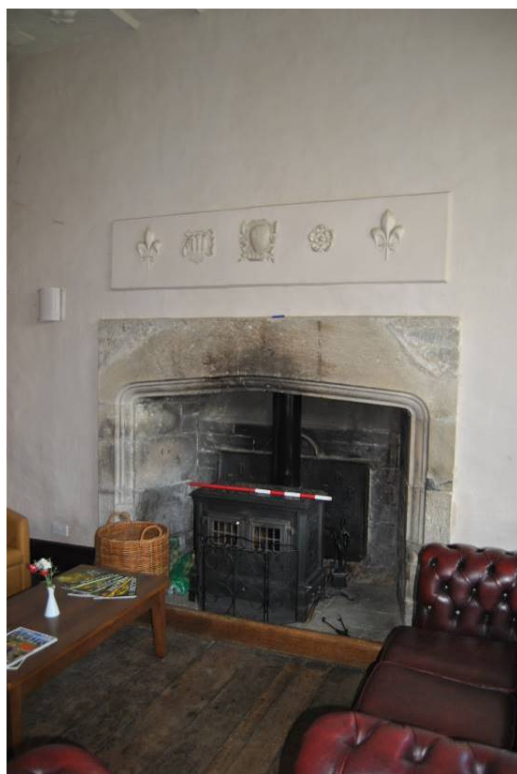
Plate 62: FP in east wall [G8] with iron fire-back.
