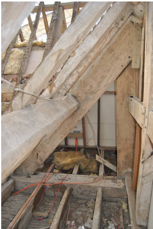
Plate g. Stop-chamfered lower purlin.
