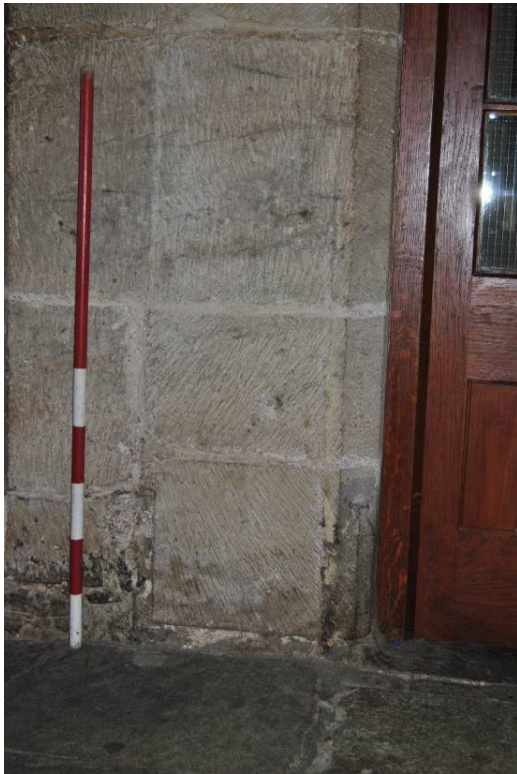
Plate 39: Faint scar of former transverse wall in [G2], removed during 1970s upgrading.
