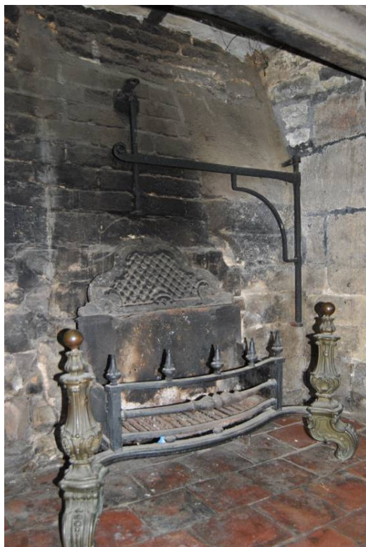
Plate 52: Detail of dog-grate and pot-crane.
