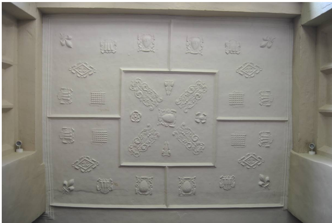
Plate 54: Decorative plaster ceiling over projecting bay window.
