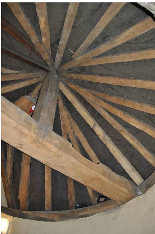
Plate 103: Conical roof structure of Stair A.
