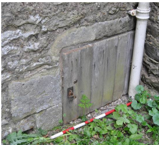
Plate 20: Access hatch at base of garderobe.
