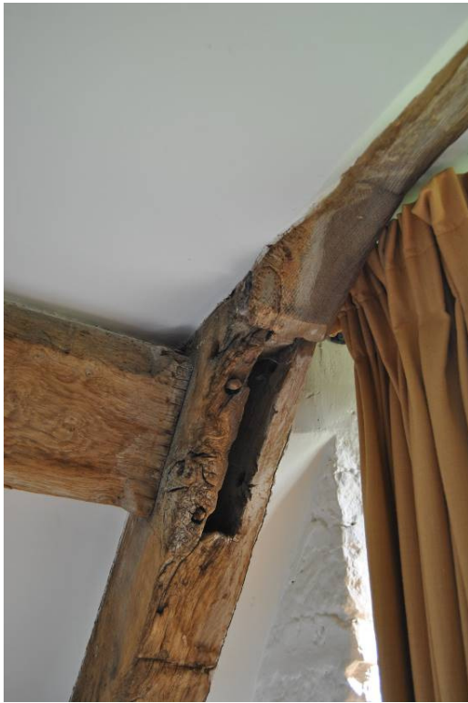
Plate 114: Truss at [S8] gable with raised collar.
