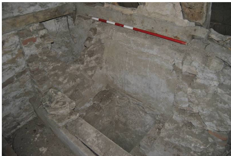
Plate i. 2F garderobe chute (foreground) and probable vent flue (left) with lintel.
