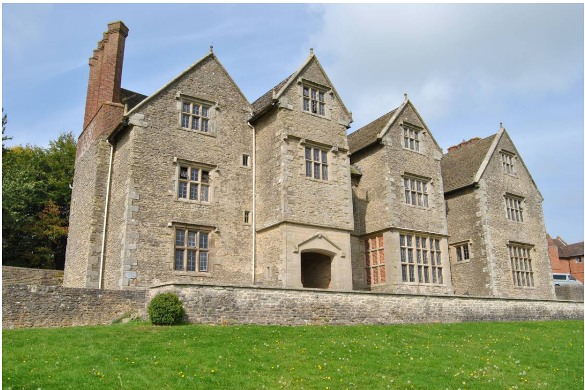
Plate 2: General view of south elevation; service wing recessed to left, projecting parlour wing to right with projecting porch tower and bay window.
