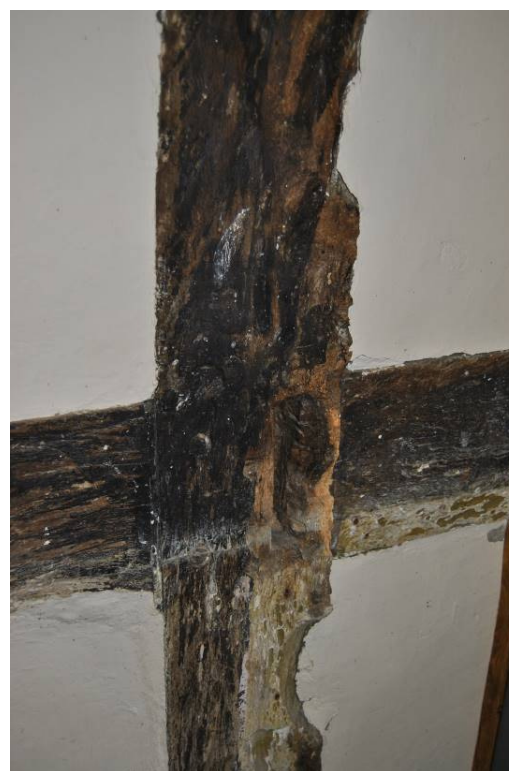
Plate 89: Room [F8]; redundant mortice of former partition.
