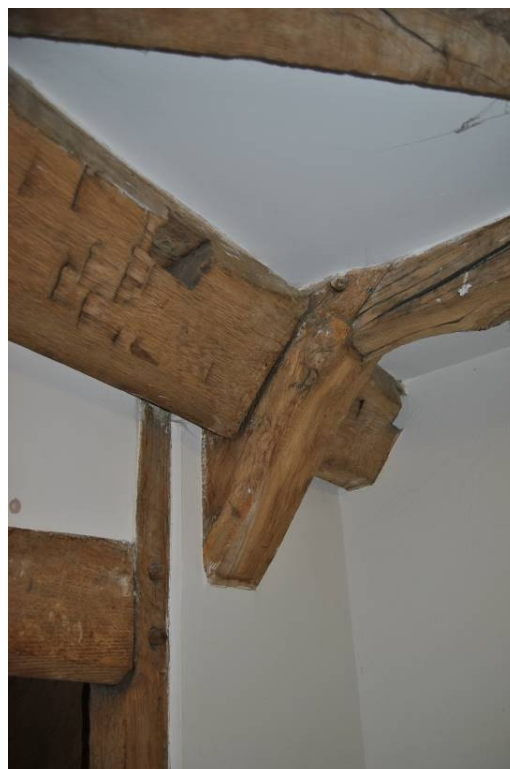
Plate 110: T1, detail of high purlin to south roof slope above door-head of d31.
