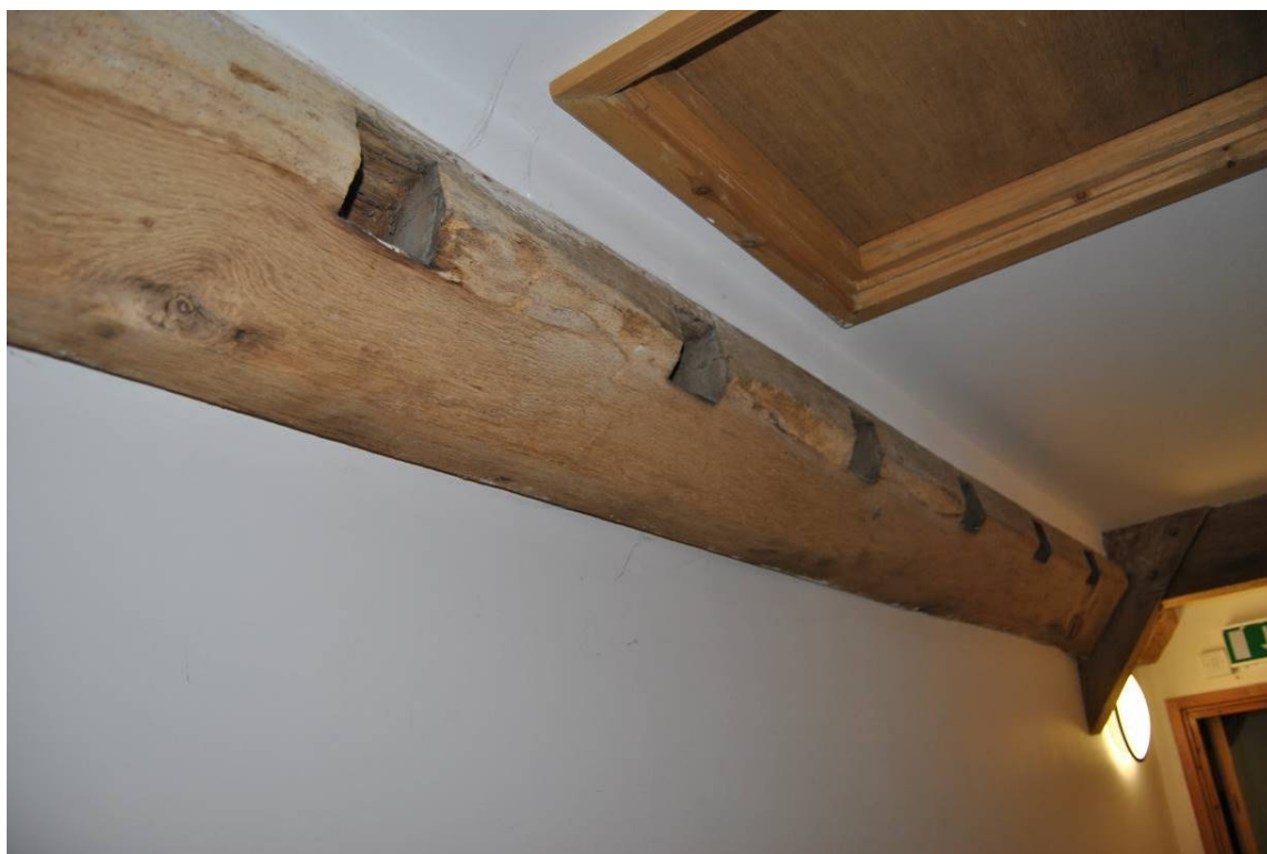
Plate 111: Redundant ceiling joist sockets within south purlin, hall range roof.
