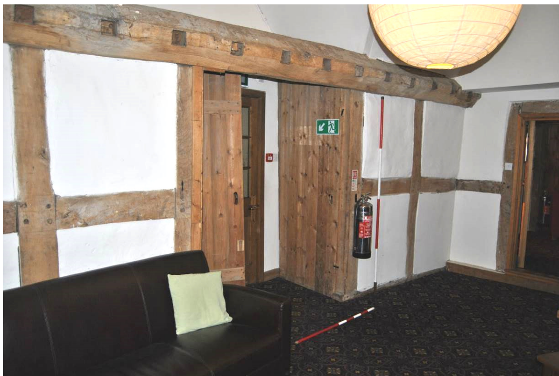
Plate 104: Room [S1] looking north-east, with timber-framed wall and doorway to Stair A; note joist sockets to purlin.
