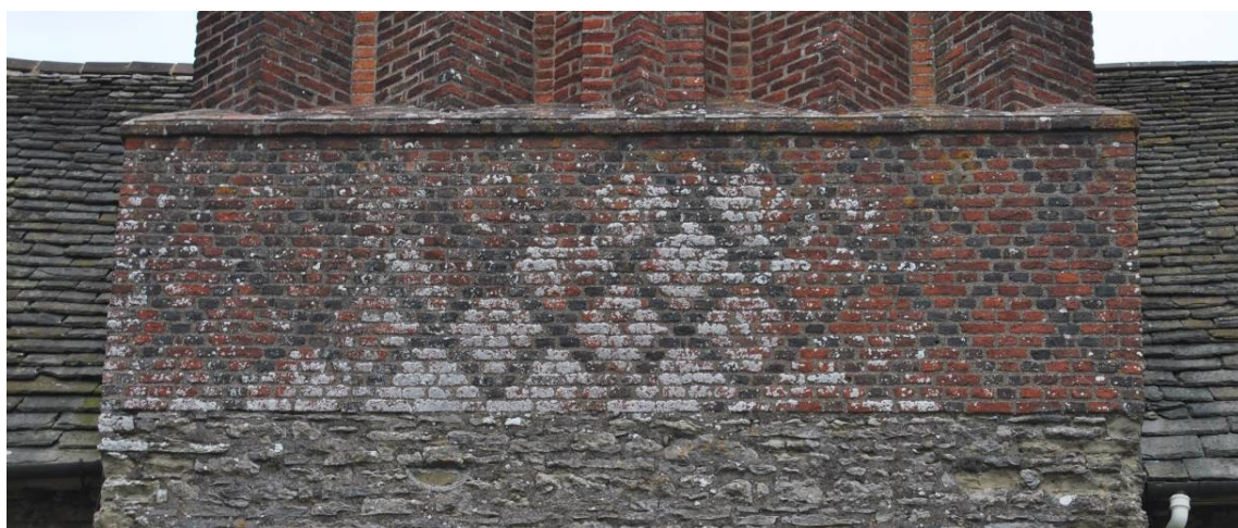
Plate 26: Detail of diaperwork brick to head of western stack.
