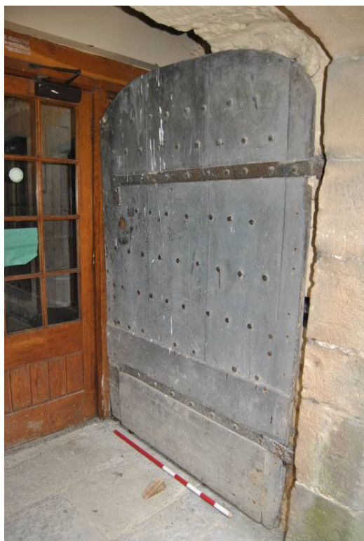
Plate 37: Rear, double-thickness door [d2]; exterior.
