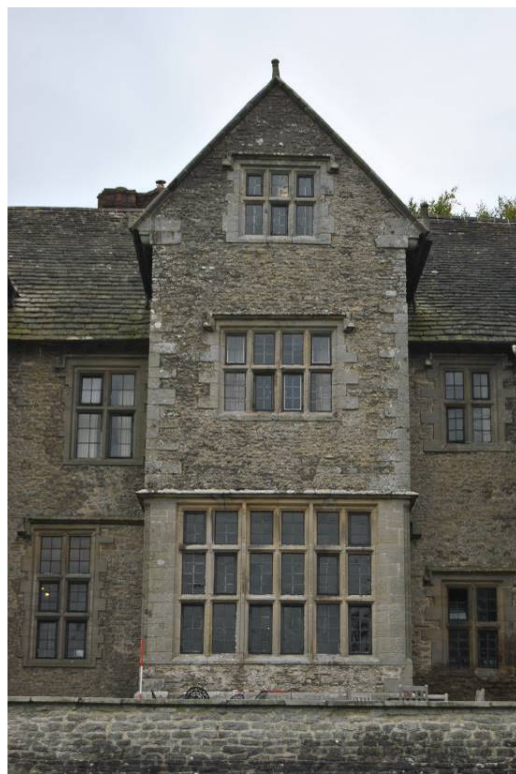
Plate 11: Projecting window bay, high end of hall, NB: continuous hood-mould extending over w3 to west.
