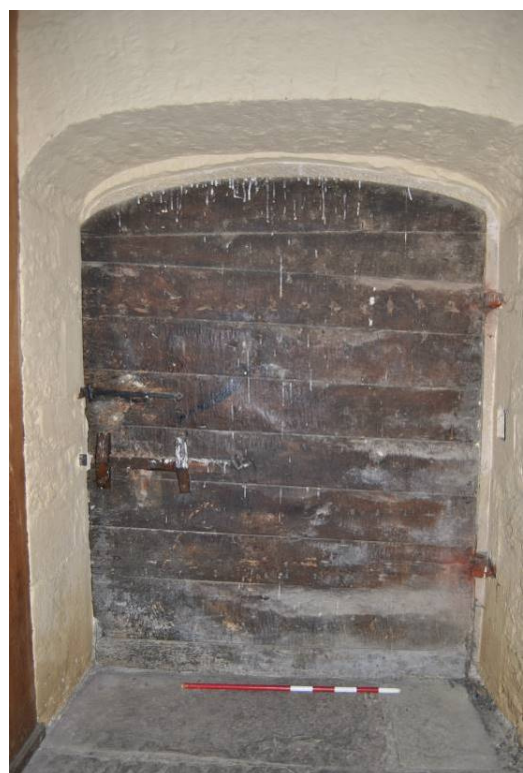
Plate 34: Principal double-thickness door [d1]; interior.
