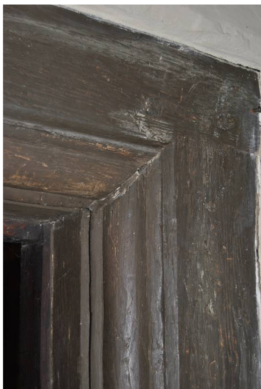
Plate 44: Door d3; detail of ovolo moulding and mitred head.
