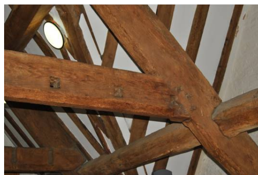
(a) Joist sockets to T10.
