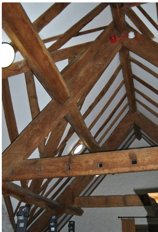
Plate 126: Roof structure over [S10]; double purlin and ridge piece.
