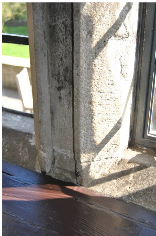
Plate 49: Window w5; variant mullion profile with sunk fillet.
