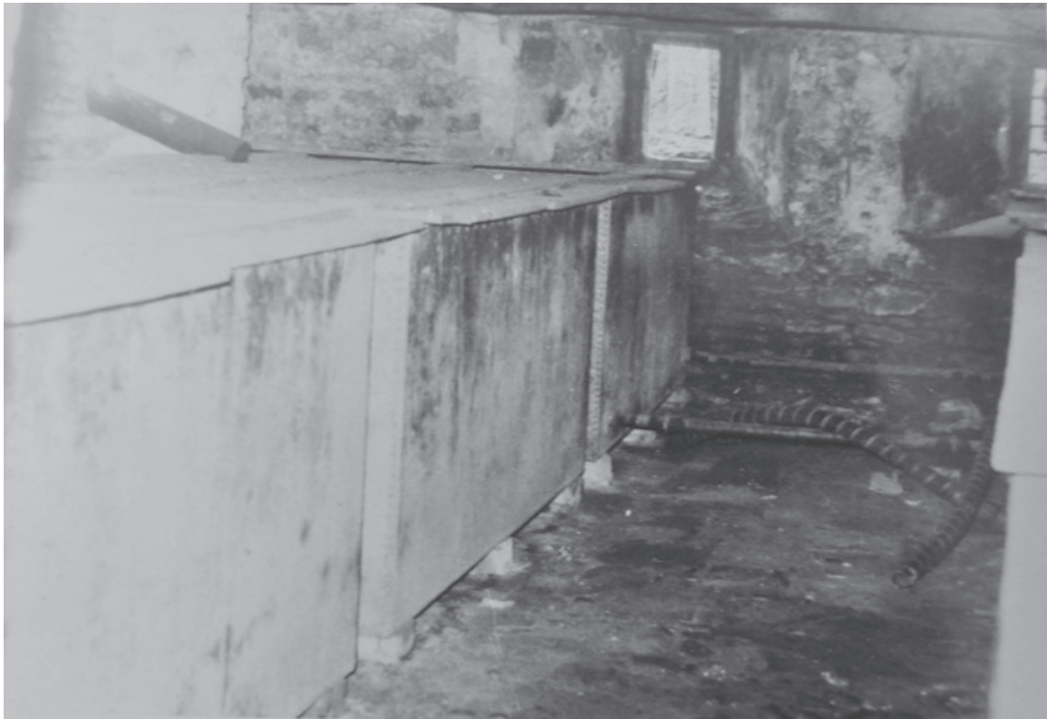
(a) Water tanks formerly located within basement of east wing, pre-1970s improvements NB. inlet pipe feeds collected rainwater from roof gutters.
