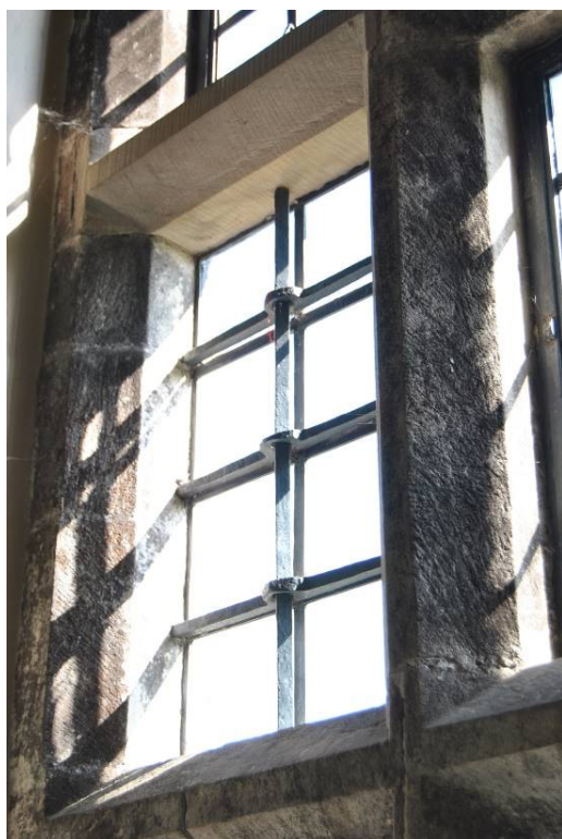
Plate 48: Bay window w5; standard and saddle bars, NB: renewed transom.
