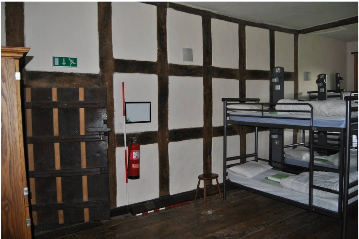
Plate 79: Principal chamber [F1], timber-framed east wall, NB. dropped rail over primary doorway d21.
