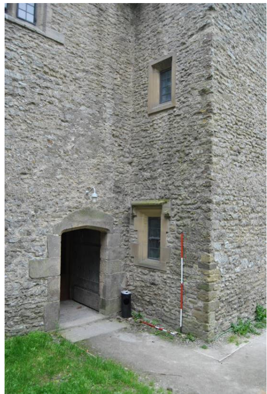
Plate 22: Primary north door to cross passage, NB: inserted windows to service wing (1970s).
