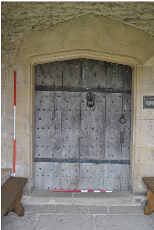
Plate 33: Principal double-thickness door [d1]; exterior.
