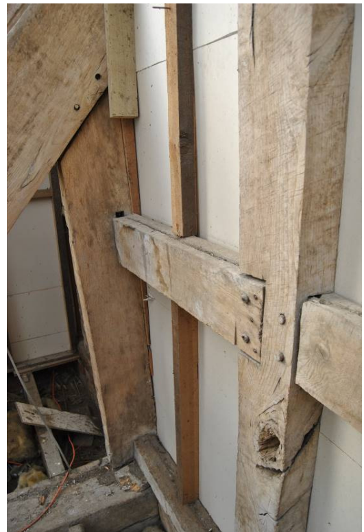
Plate h. Variant mid-rail, tenoned to QS, lapped to stud.
