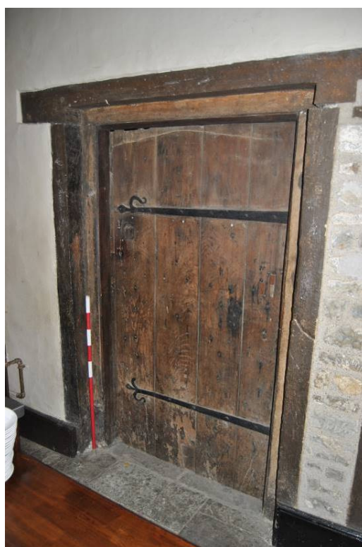
Plate 45: Door d4: unchamfered frame, re-used door.
