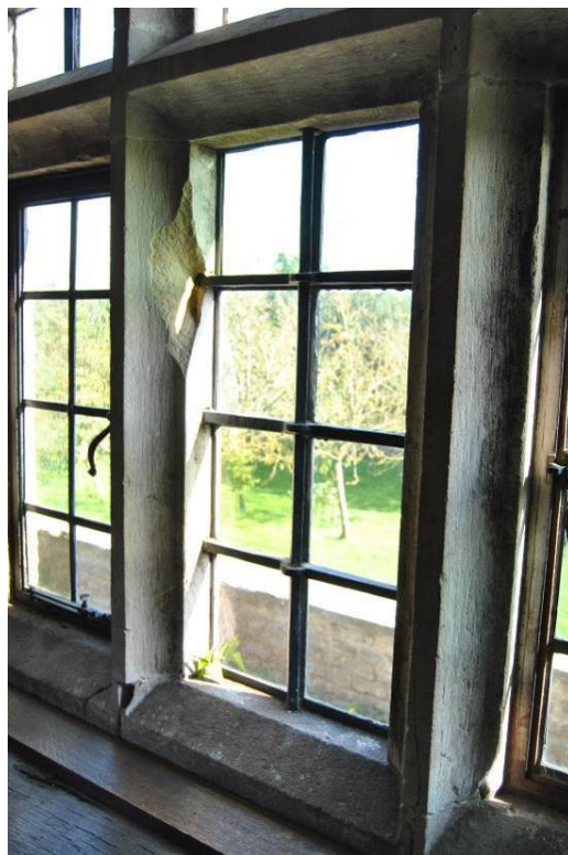
Plate 61: Hollow chamfered mullions, w9.
