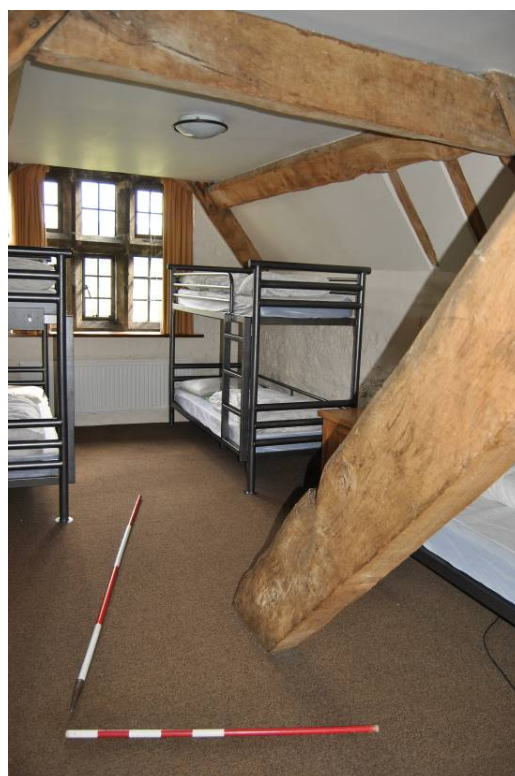
Plate 113: Room [S8] looking south, NB: foot of southern principal (T1) of hall range roof.
