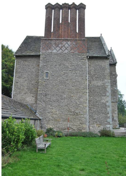
Plate 25: Western elevation, NB. rebuilt upper stacks and enigmatic, single-light window at 1F level.
