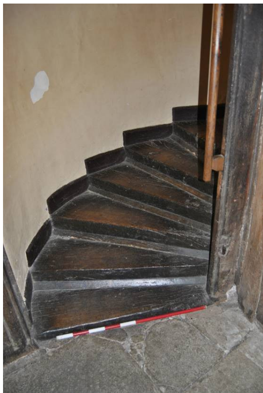
Plate 70: Base of mast-newel stair A.
