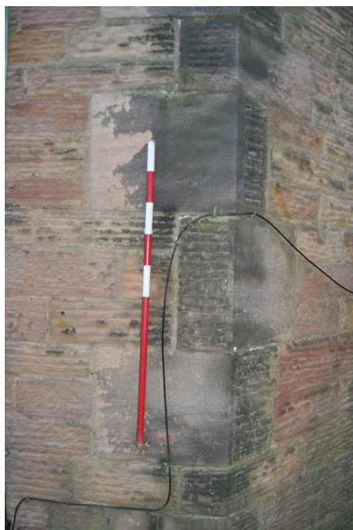
Plate 37: Detail of horizontal tooling, incl. to quoins
