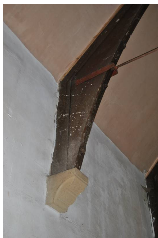
Plate 60: Base of roof truss on stone corbel.
