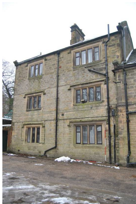
Plate 24: Three storey section of Bay 9, NB. variation in stone colour to upper storey
