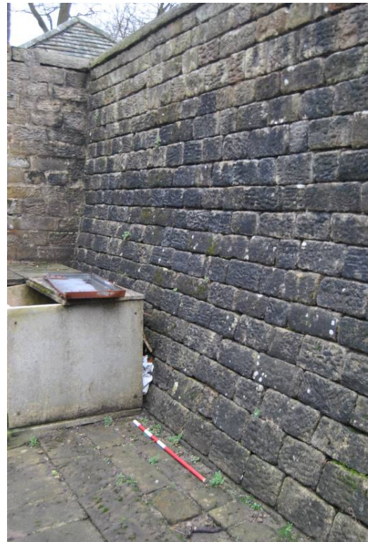
Plate 67: Battered retaining wall of kitchen garden.
