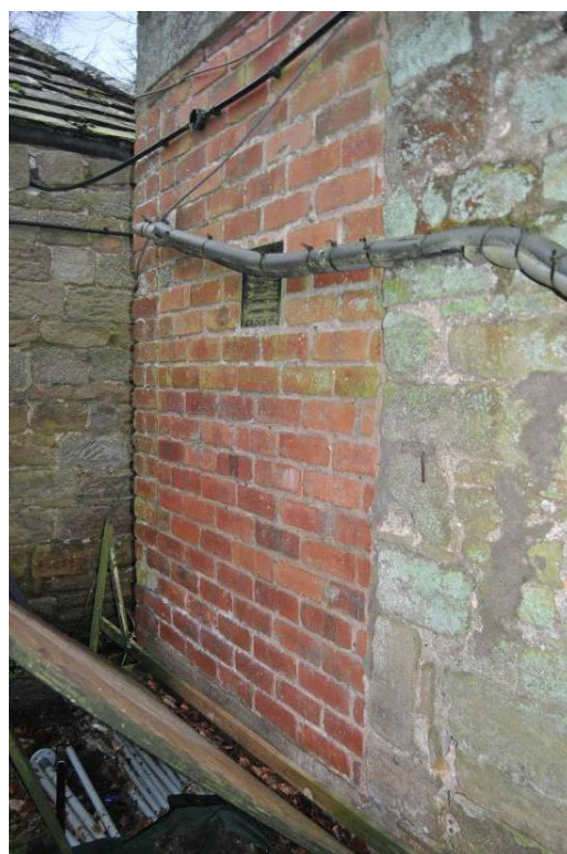
Plate 114: Blocked door at east end of north elevation.
