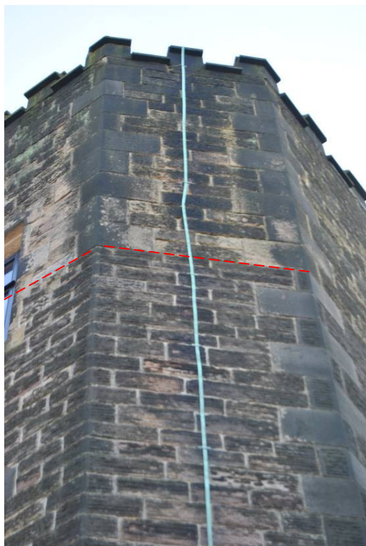
Plate 36: Change in stonework (marked in dashed line) denoting raised upper storey.
