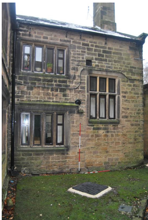
Plate 38: Kitchen range, south elevation NB SJ beneath left hand jamb of mid-height window.
