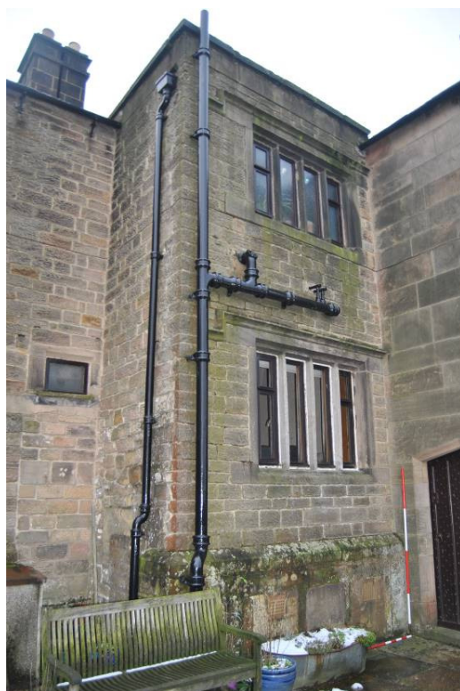
Plate 18: Flat-roofed former stair turret at Bay 6; NB. blocked cellar windows to plinth.
