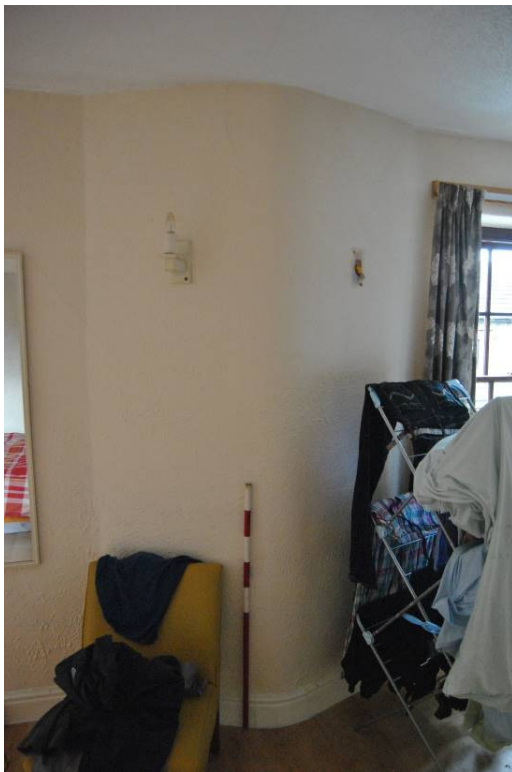
Plate 121: Angled projection to centre of south wall related to former back to back fireplaces (Figure 27).
