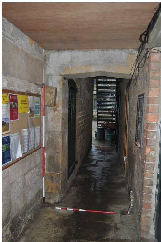
Plate 77: Original door [d25] to passage between stable and coach house, looking south. NB. plinth to base of left hand jamb.
