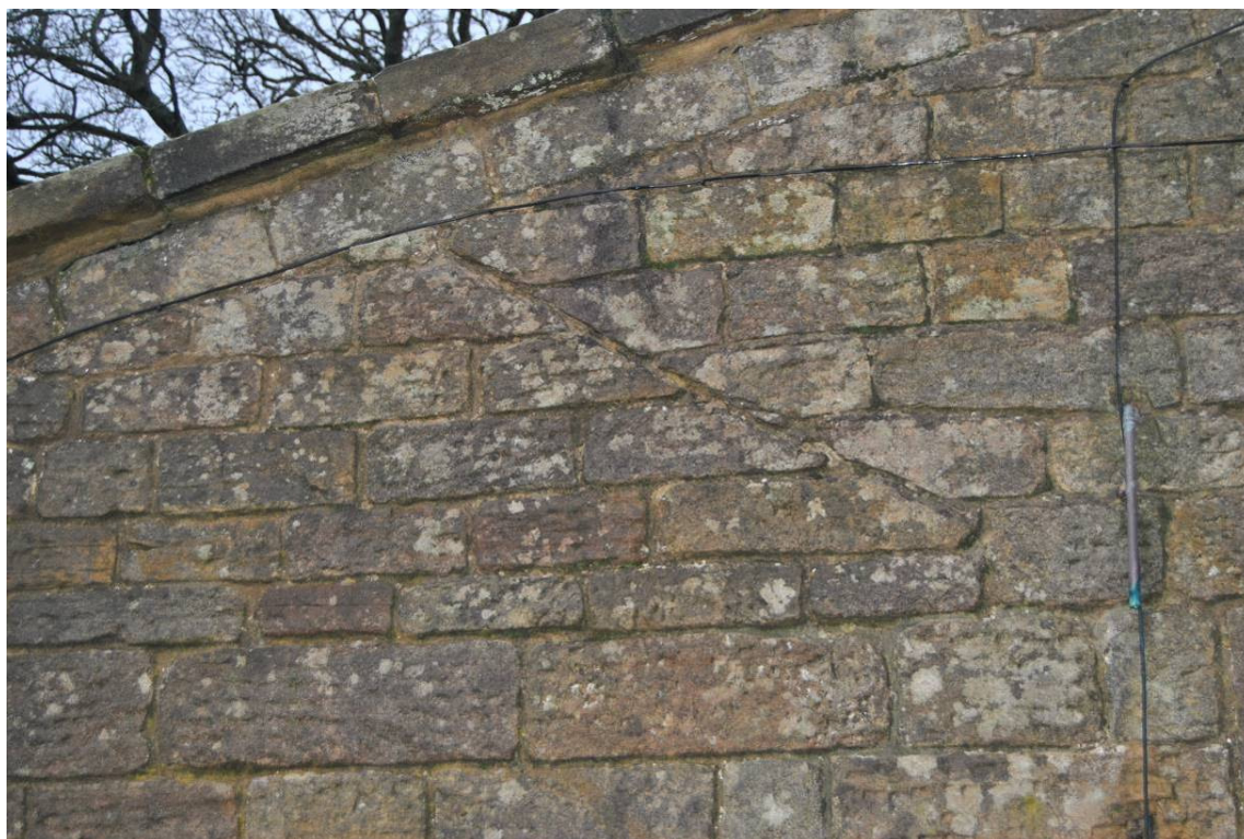
Plate 98: Detail of sloping scar and discontinuous coursing indicating eastern roofslope of former parallel stables range (see Figure 13b).
