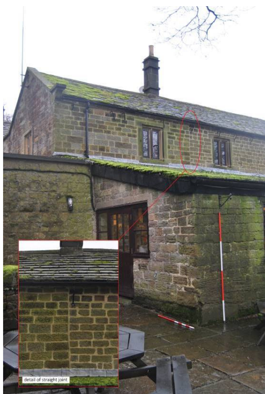
Plate 75: Detail of phase break at N end of stables.
