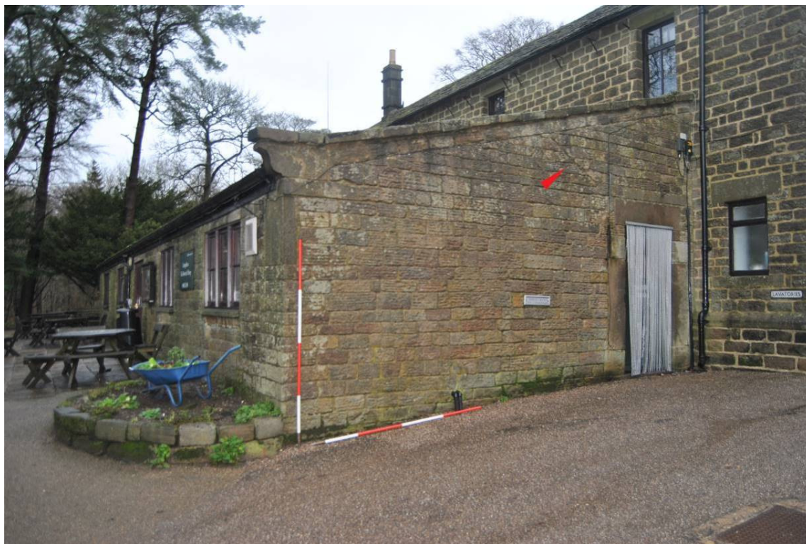
Plate 97: South elevation of café block incorporating fabric from former parallel range; NB: scar of former roofline (marked with red arrow – see detail Plate 98).
