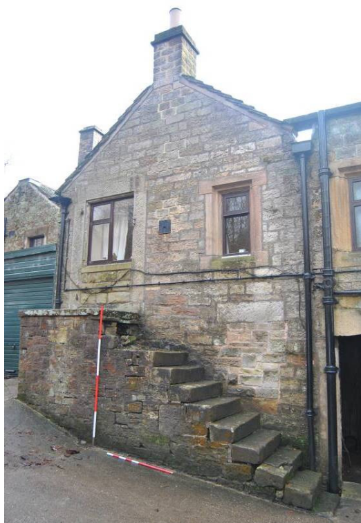
Plate 124: North gable of transverse extension F with tallet-step rising to former 1F doorway, [w18].
