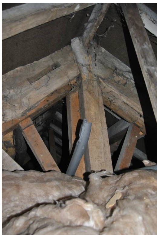
Plate 109: Timber king-post roof over coach house B (visible above [F14]).
