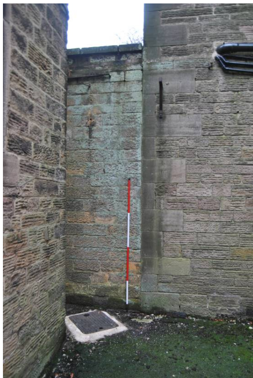
Plate 34: SJ at Bay 3/gun room, NB: horizontal tooling To Bay 3 (right).
