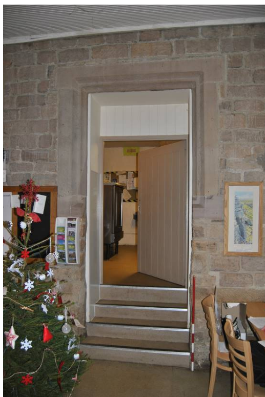
Plate 81: Former window converted to door [d9] (1977).
