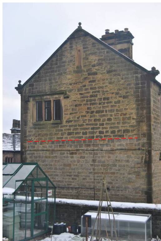
Plate 42: East gable end of Bay 9 with clear change of colouration indicating former eaves line (dashed line).
