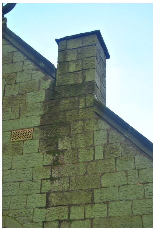
Plate 55: Single-flue stack breaks eastern roof slope.
