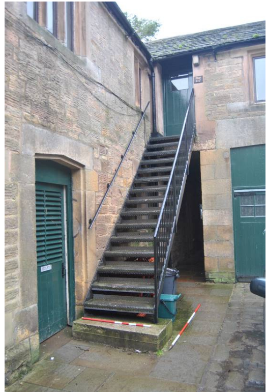
Plate 102 : Steel stair serving first floor apartments via inserted 1F door.
