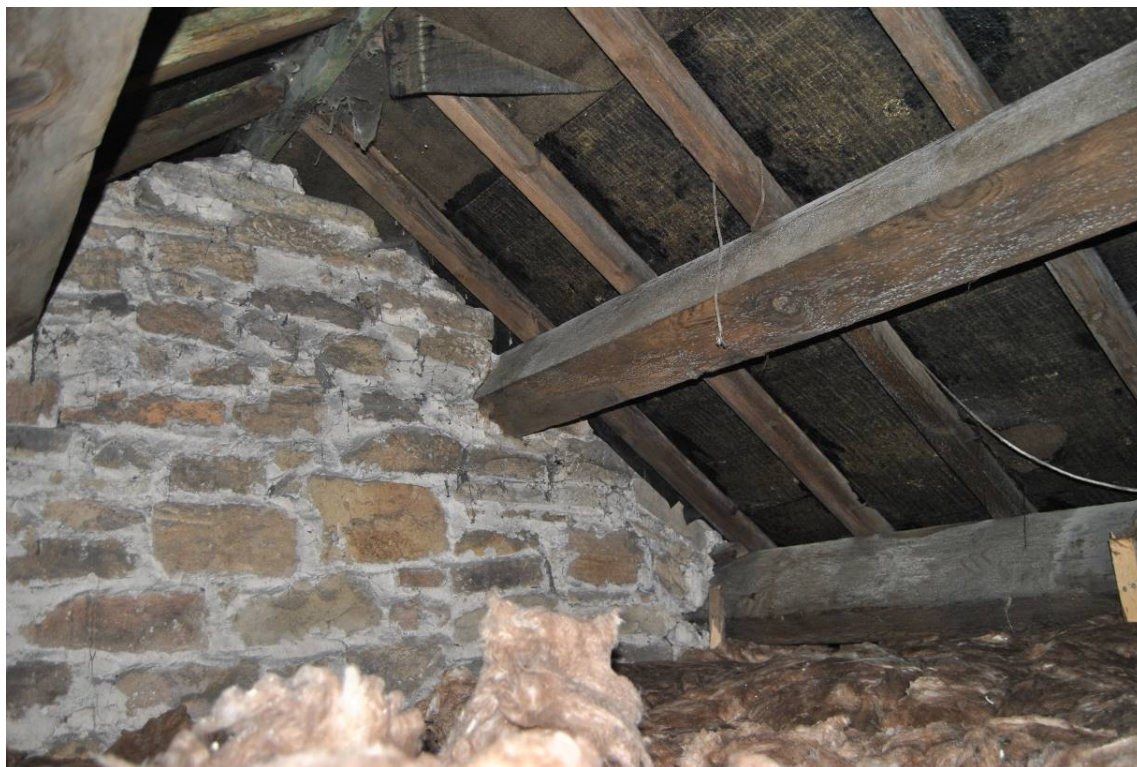
Plate 95: Roof structure over Stables A (visible above [F5]) with two tiers of side purlins supported by stone bay partitions extending to apex.
