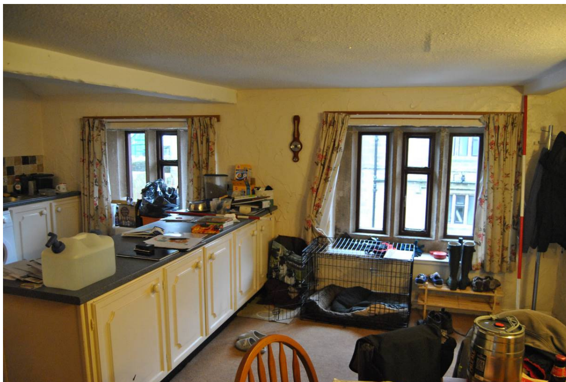
Plate 106: Two-bay kitchen/diner [F12] with ceiling beams marking truss locations.
