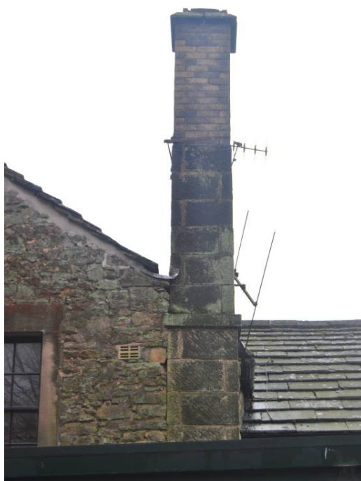
Plate 113: Detail of ashlar stack, raised in brick.
