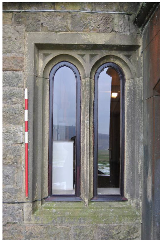
Plate 14: Variant windows at Bay 2-4; two-centred heads, (near semi-circular) and sunk spandrels.
