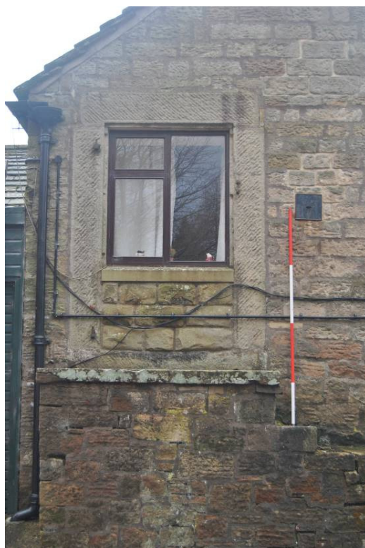
Plate 125: Window [w18], former doorway, NB. diagonal scoring to jambs/lintel.
