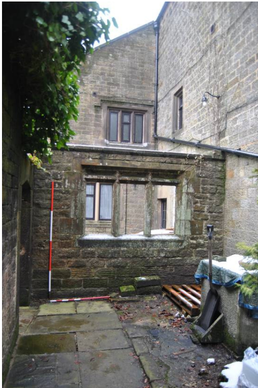
Plate 43: Remnant of extended 'Servants' Hall' incorp re-set window from original north gable end.
