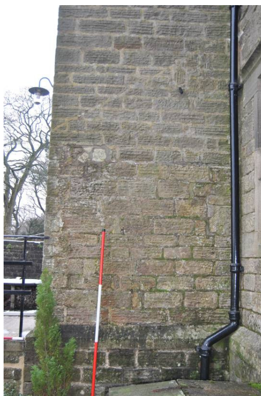
Plate 20: Sloping roof scar to southern return of Bay 8.
