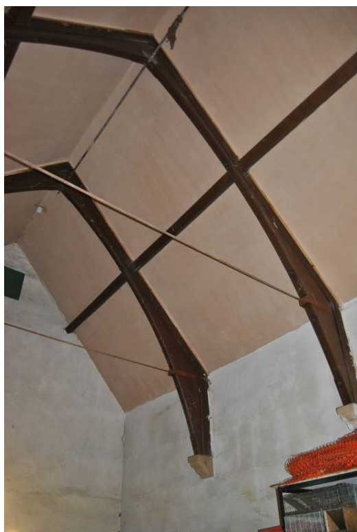
Plate 59: Roof structure with transverse iron ties at eaves level and longitudinal tie to apex.
