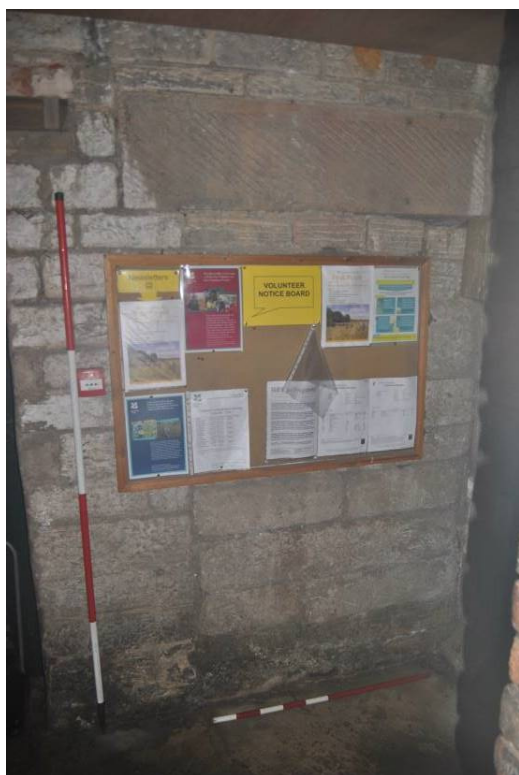
Plate 126: Blocked door to block F within transverse passage, NB. diagonal scoring to lintel.
