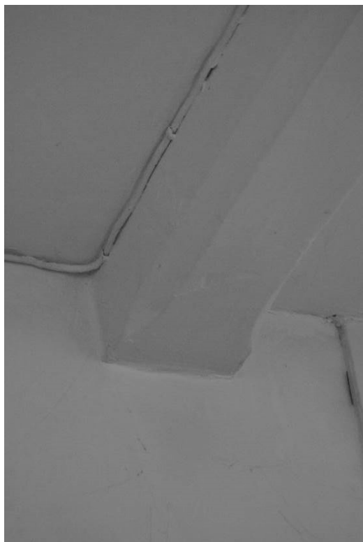
Plate 89: Stop-chamfered ceiling beam.
