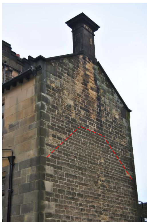
Plate 32: North gable of Bay 3 with evidence for former lower roof line (dashed line).
