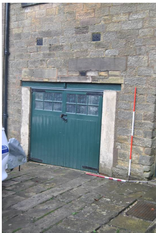
Plate 111: Inserted door [d17] (1968) with stone lintels of former window openings over (see Figure 15c).
