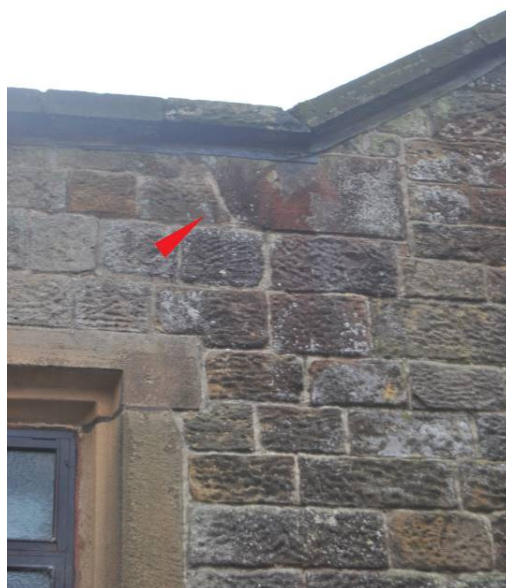
Plate 86: Western kneeler (arrowed) incorporated into later walling.
