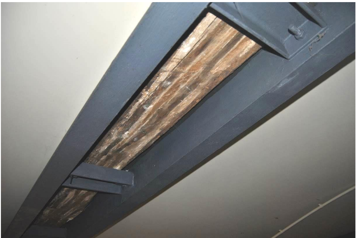
Plate 6: Primary transverse ceiling beam clasped by C-section steels.
