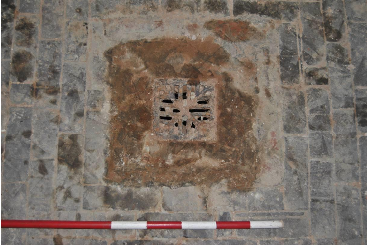
Plate 12: Surviving iron drainage grille at centre of loose-box 2 (note edge-laid brick floor).
