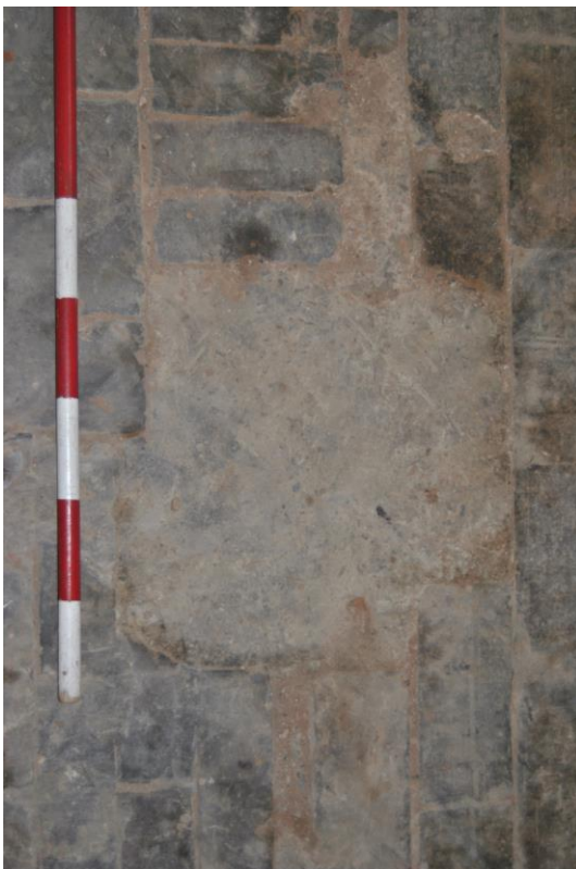
Plate 16: Stone pad to west end of former partition between loose-boxes 1 and 2.
