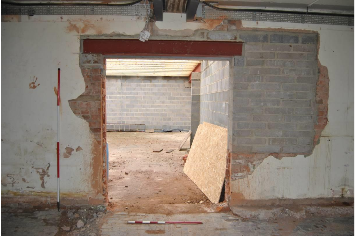
Plate 7: Newly formed opening to east all with blocked secondary window to right; note timber lacing in brickwork to left of new opening.
