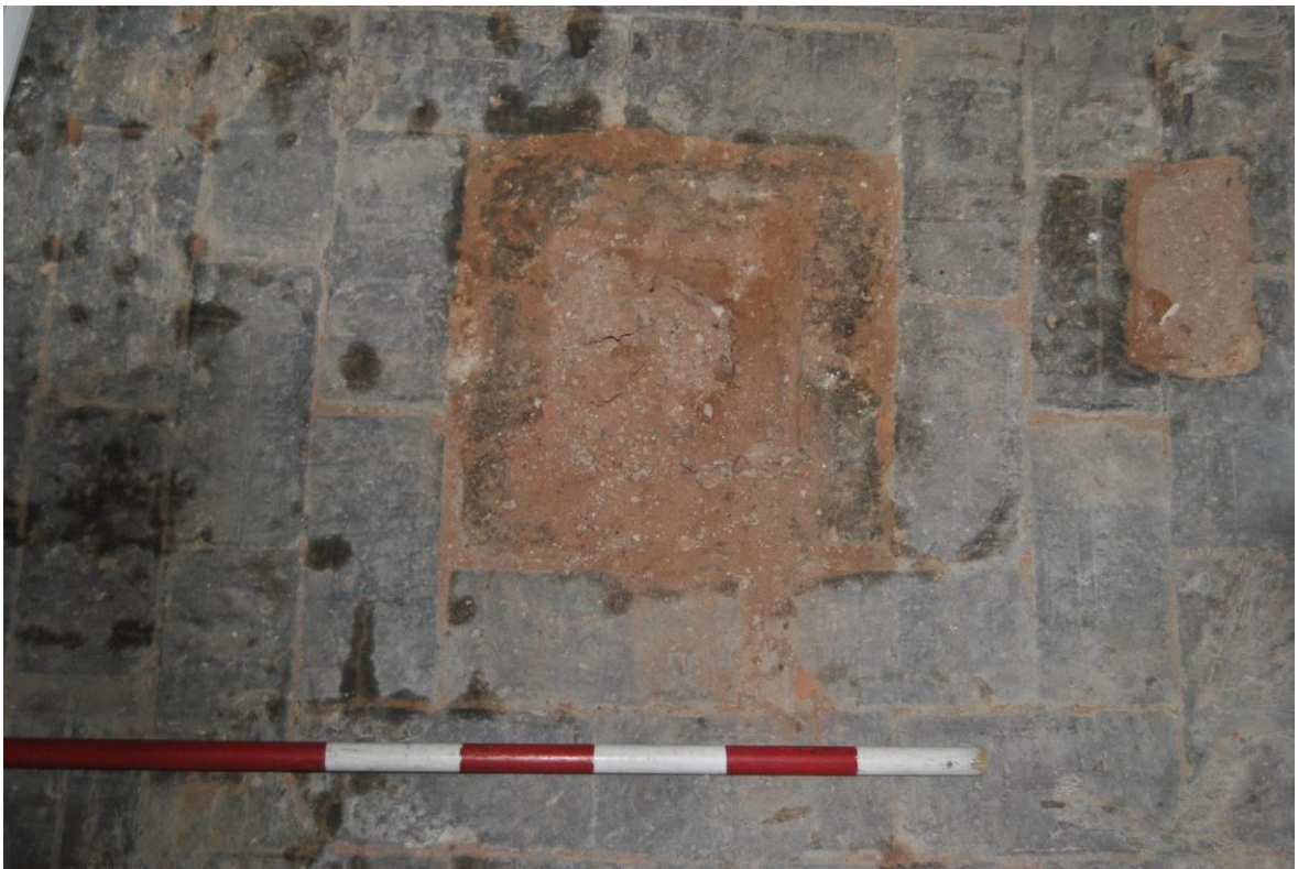
Plate 13: Missing iron drainage grille at centre of loose-box 3 (note face-laid brick floor).
