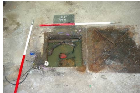
Photo 35. Sump pit in base of cellar floor, looking west.
