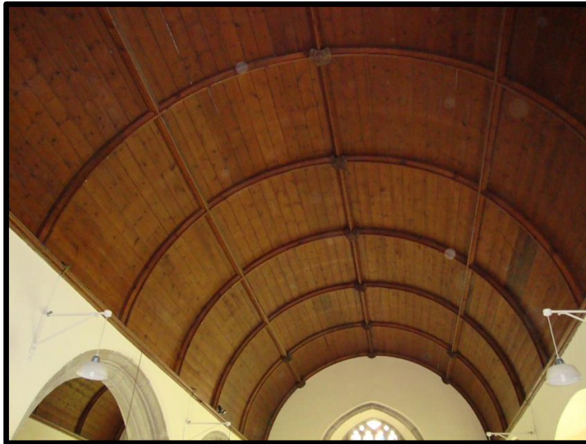
Fig. 2 View of the underside of the nave roof showing modern ribs and boarding, with ?reused bosses ornamenting the ridge rib and forming a celure over the sanctuary
