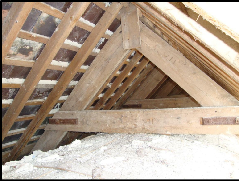
Fig. 4 View of the inside of the aisle roof at Woodland, above ceiling level, showing a 19th-century roof structure of widely-spaced 'A'-frame trusses supporting a boarded ceiling imitating the curved form of a traditional wagon roof.
