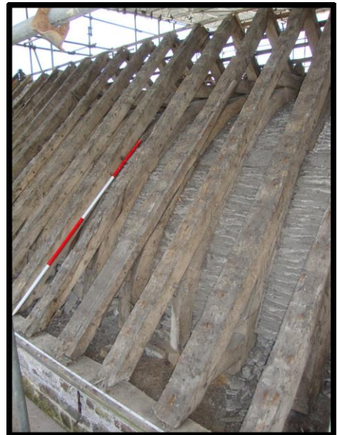
Fig. 6 An authentic C15th wagon roof (at High Bickington), showing the regularly-spaced, closely-set arch-braced trusses forming a curved roof structure above a later ceiling
