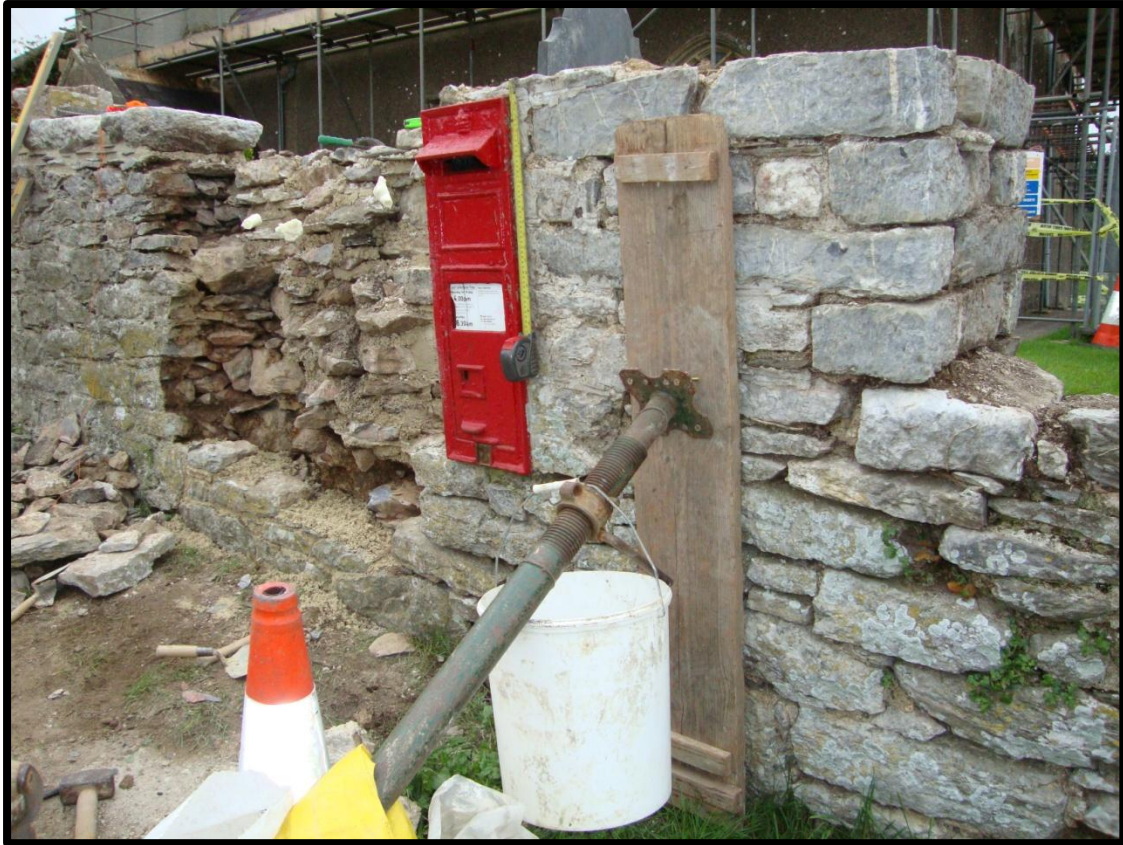
Fig. 7 View of the churchyard wall prior to rebuilding, showing the collapsing section of walling containing the Victorian post box and the Harris memorial. The church, under scaffold, lies in the background ( \frac{1}{2} metre scale).
