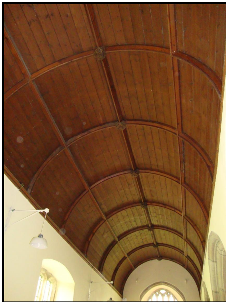
Fig 3. View of the underside of the aisle roof showing ?reused bosses ornamenting the central rib.
