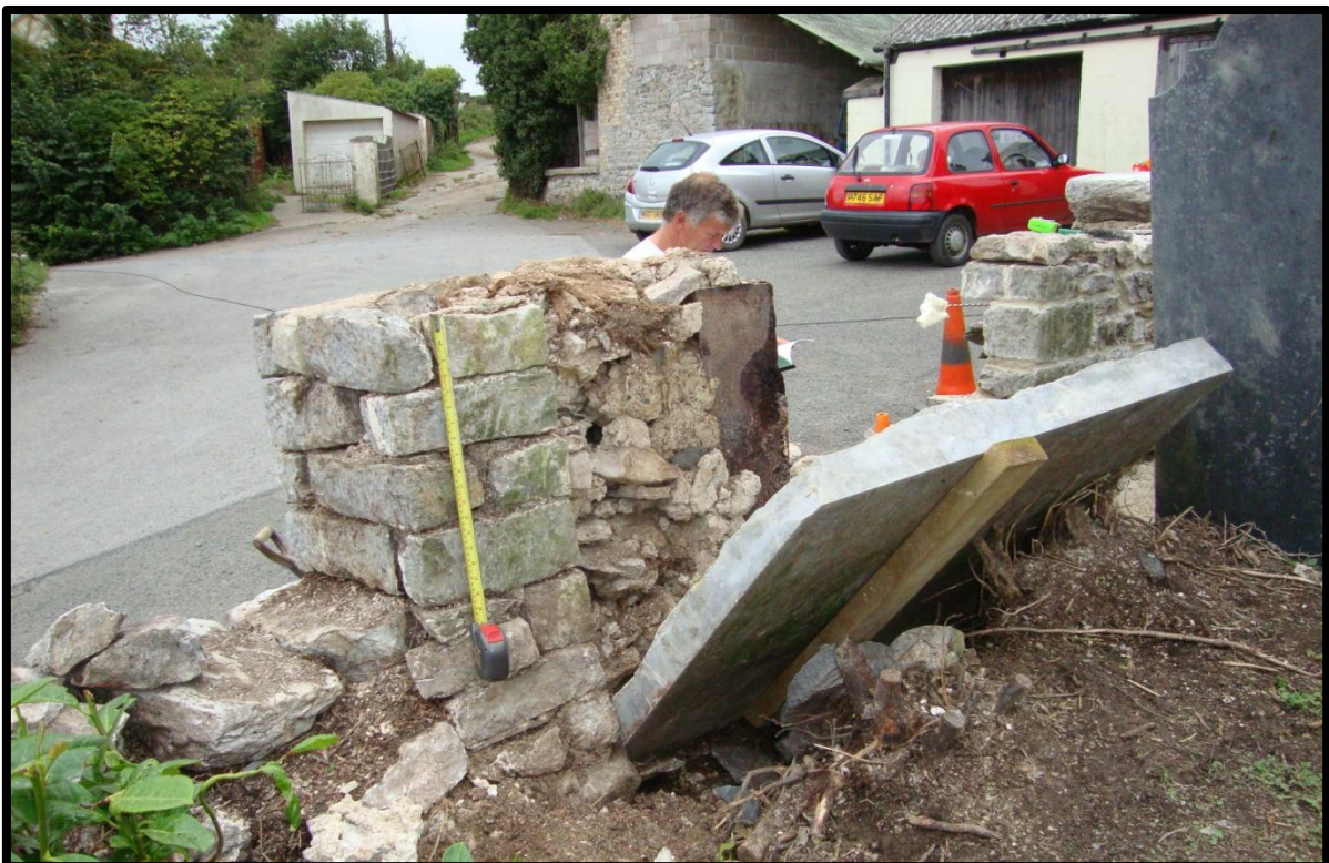
Fig. 8 Detail of the recess in the raised section of walling, designed to accommodate both the Harris memorial and the Victorian post box. The Harris memorial is shown temporarily supported during the works ( \frac{1}{2} metre scale).
