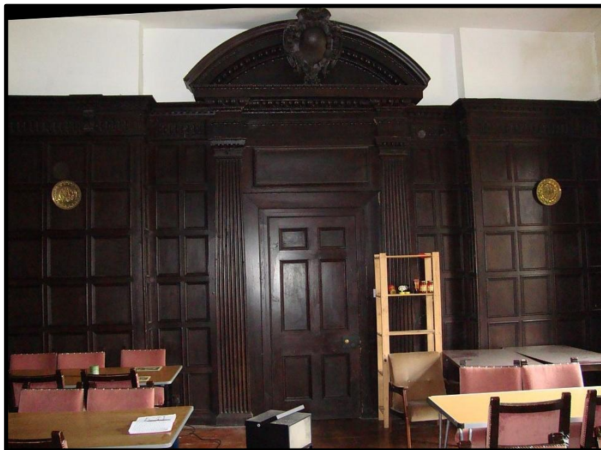
Fig. 10 Detail of the door case linking the staircase with the Hall, looking south, showing the panelling. A corresponding door case in the opposite wall, if in situ , would appear to confirm a north-south processional route from the main entrance in the east wing to the staircase.
