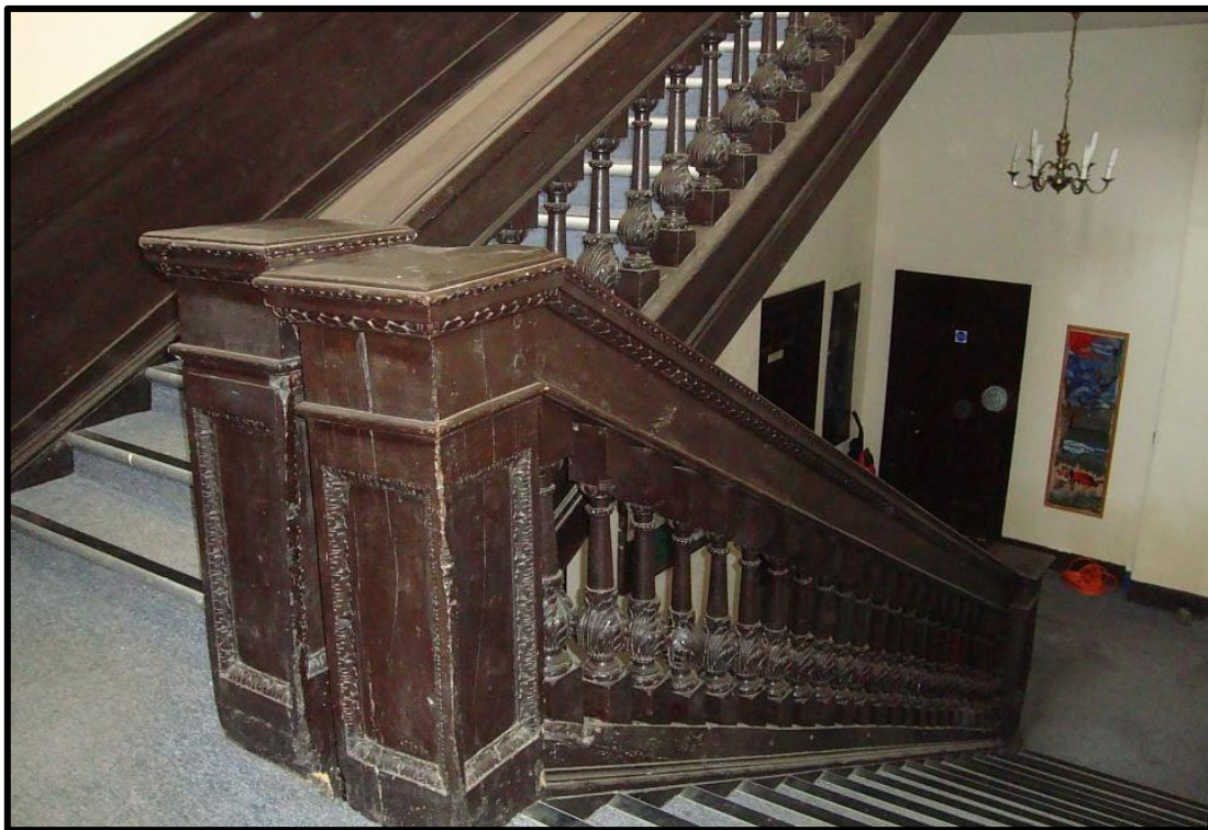
Fig. 8 Detail of the 17th-century staircase showing the high quality architectural detail and the clumsy junction of the two flights.
