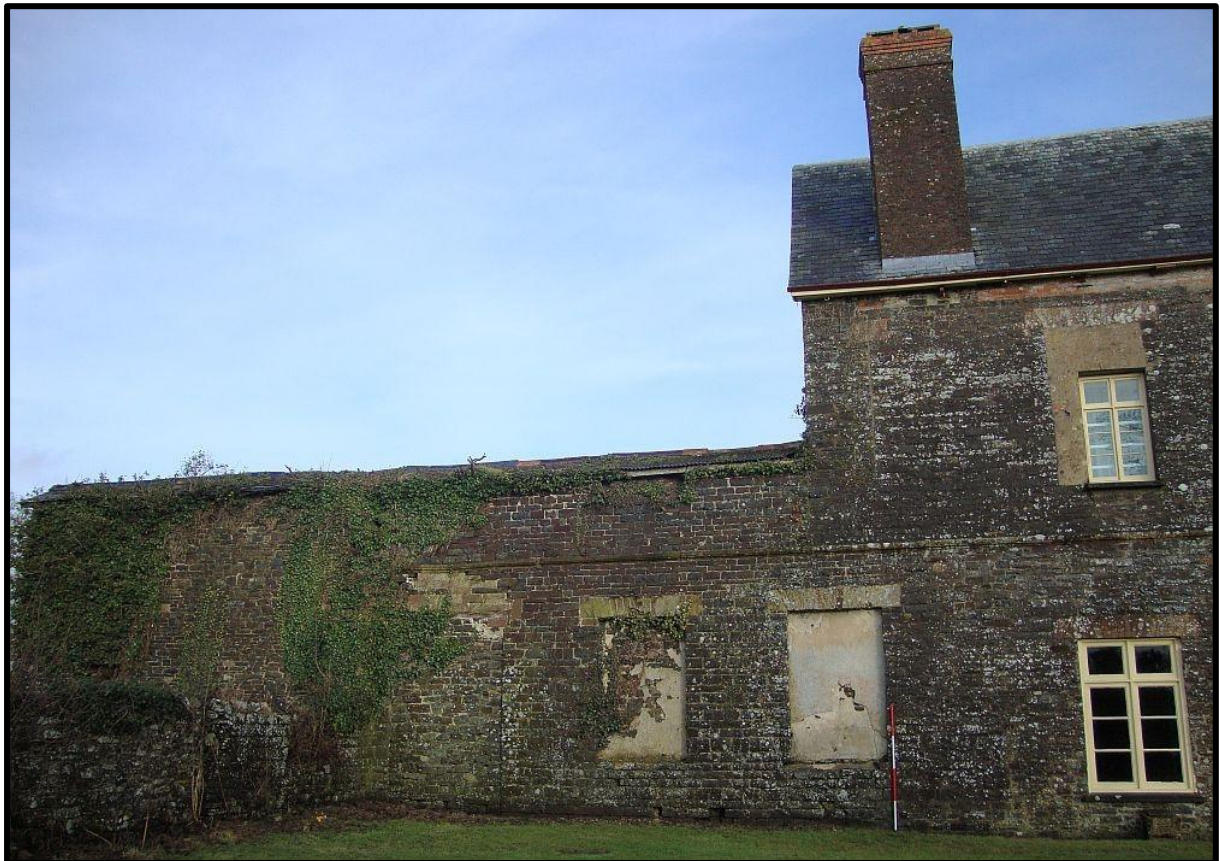
Fig. 5 Part of the west elevation showing the higher level of the windows south of the door to the loggia, perhaps suggestive of a symmetrical central block in the east range forming a corps de logis facing east, with a central doorway to the loggia in its rear elevation.
