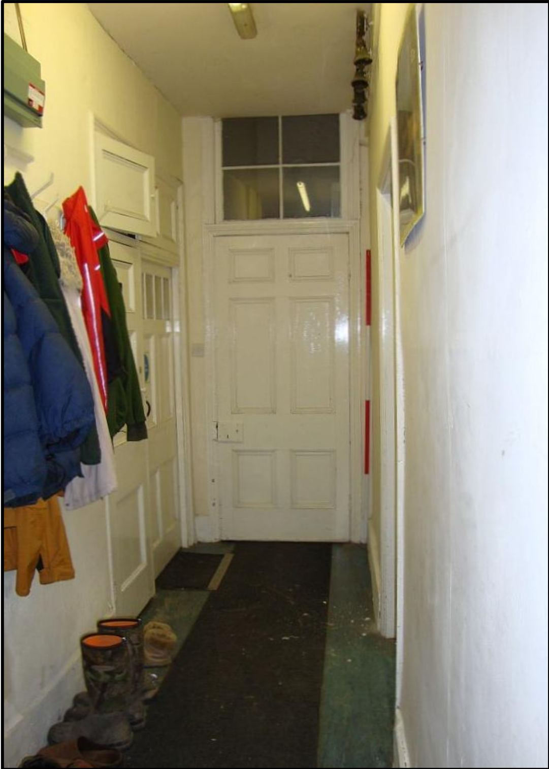
Fig. 13 View of the kitchen passage, looking east, showing the cupboards occupying a partially blocked (window) embrasure to the north (left), the 19th-century kitchen door with over light and the bells for summoning servants (top right).
