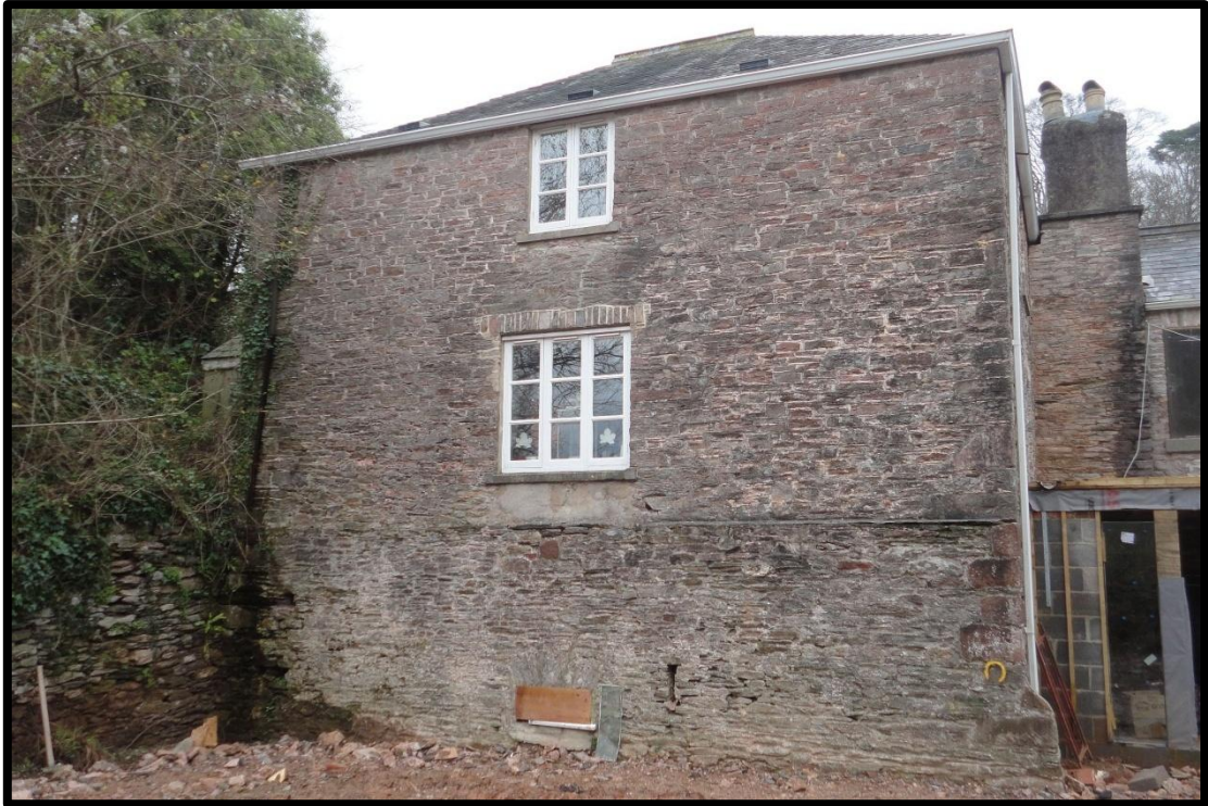
Fig. 4 Elevation of the mill from the site of the wheelpit, showing possible earlier masonry in the lower part of the wall and the raised level of the mill pond (left).
