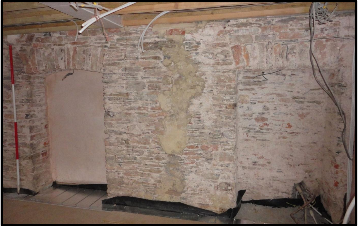
Fig. 10 View of the doorways formerly communicating with the mill, showing the wall scar lying between them, suggestive of a structure abutting the mill and pre-dating the north-western extension.
