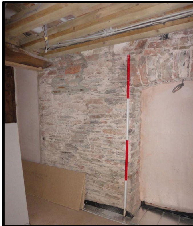
Fig. 11 The shadow of a steep staircase or ladder, rising from the house to the first floor of the extension and with severely restricted head room.
