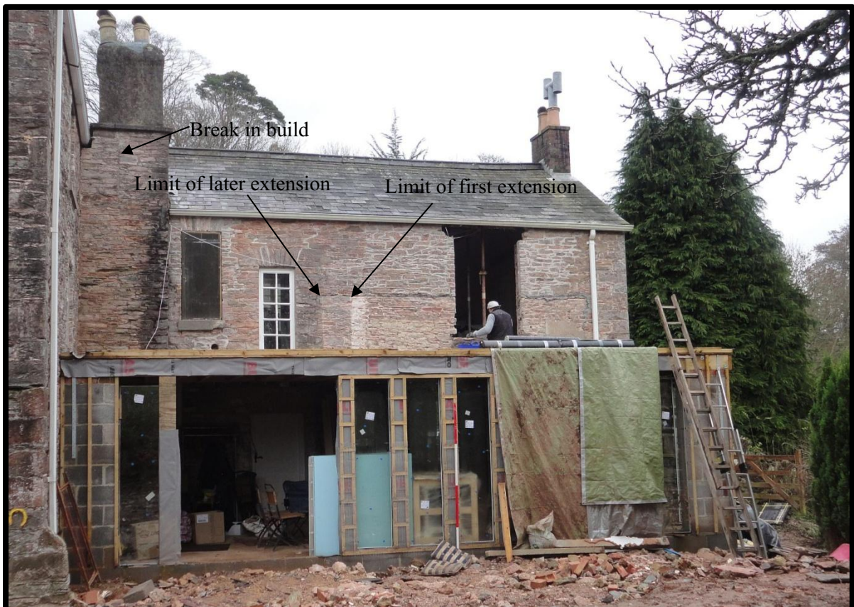
Fig. 7 Elevation of the house from the site of the tail race showing evidence of two phases of rear extension, the rebuilt chimney and the relationship of the lean-to roofs with the first-floor and staircase window openings.
