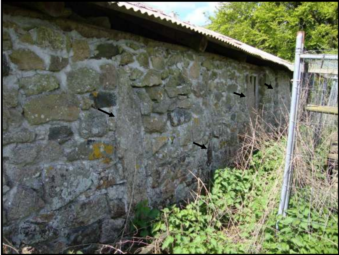
Fig. 16. View of the north-eastern wall of the linhay, showing the positions of some of the granite monoliths (marked by arrows).
