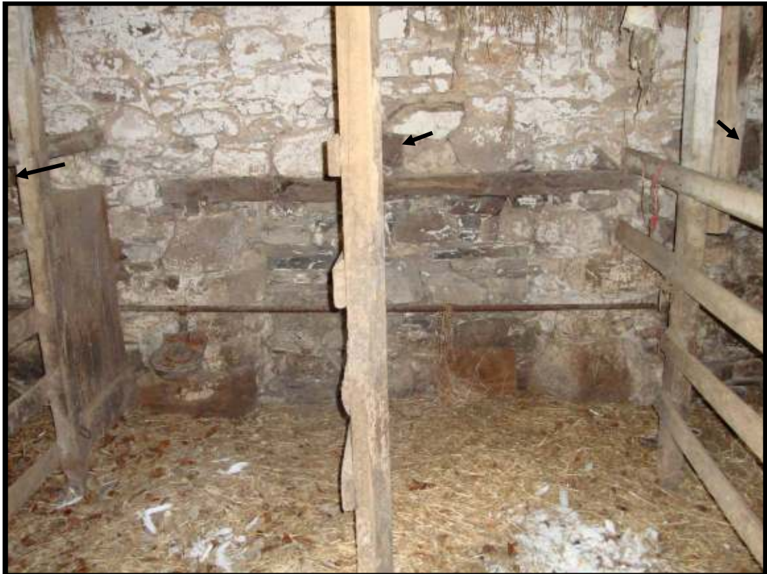
Fig. 14. Detail of the north-east wall of the lean-to showing the blocked, splayed opening at a low level in the end wall of the building and (arrowed) the sawn-off stumps of timbers probably relating to an earlier ceiling, possibly removed when the levels of the farmyard were altered to embank the pond.
