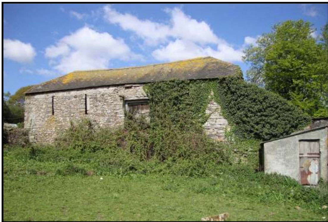
Fig. 6. The south-eastern elevation of the barn, showing the ventilation slits and superimposed doors (partially concealed by ivy) with the remains of a canopy over the first-floor doorway.
