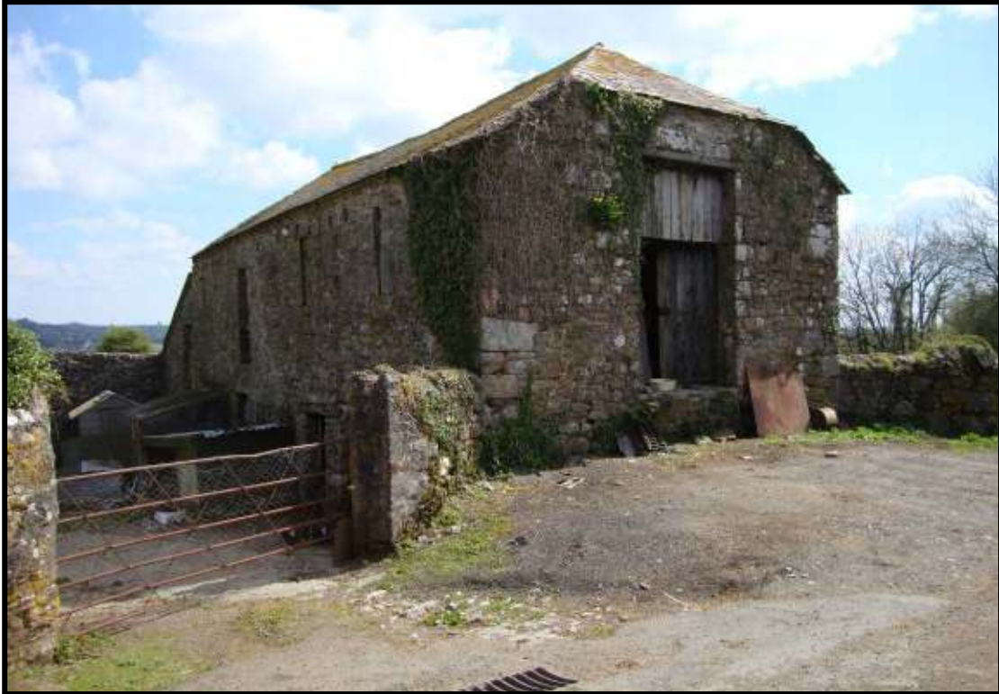
Fig. 5. The south-western elevation of the barn, looking east, showing the changes in level between the road to the south west of the barn and the farmyard on the north west.
