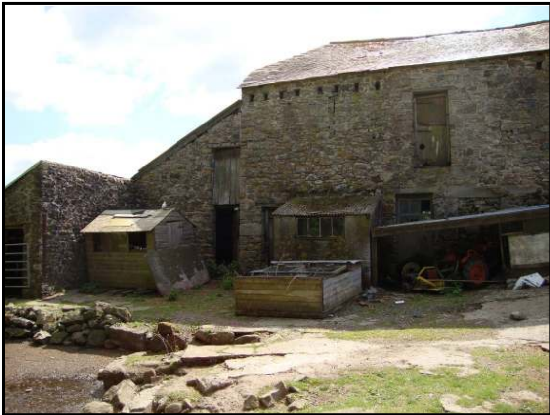
Fig. 12. View of the lower end of the building, showing the clear building break between the end of the barn and the adjacent lean-to structures.
