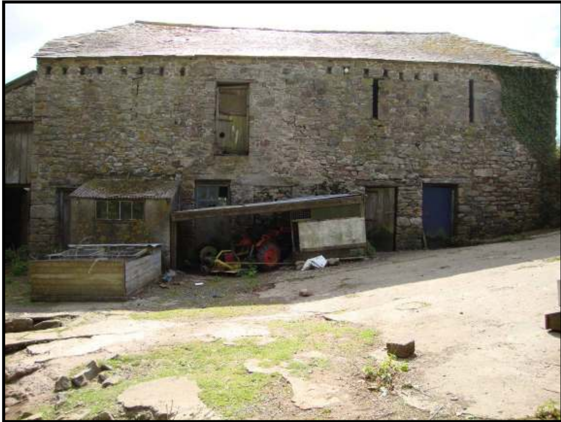
Fig. 8. North-western elevation of the barn, showing the modern accretions hiding the blocked ground-floor doorways and the change in level of the farmyard due to the embanking of the pond.
