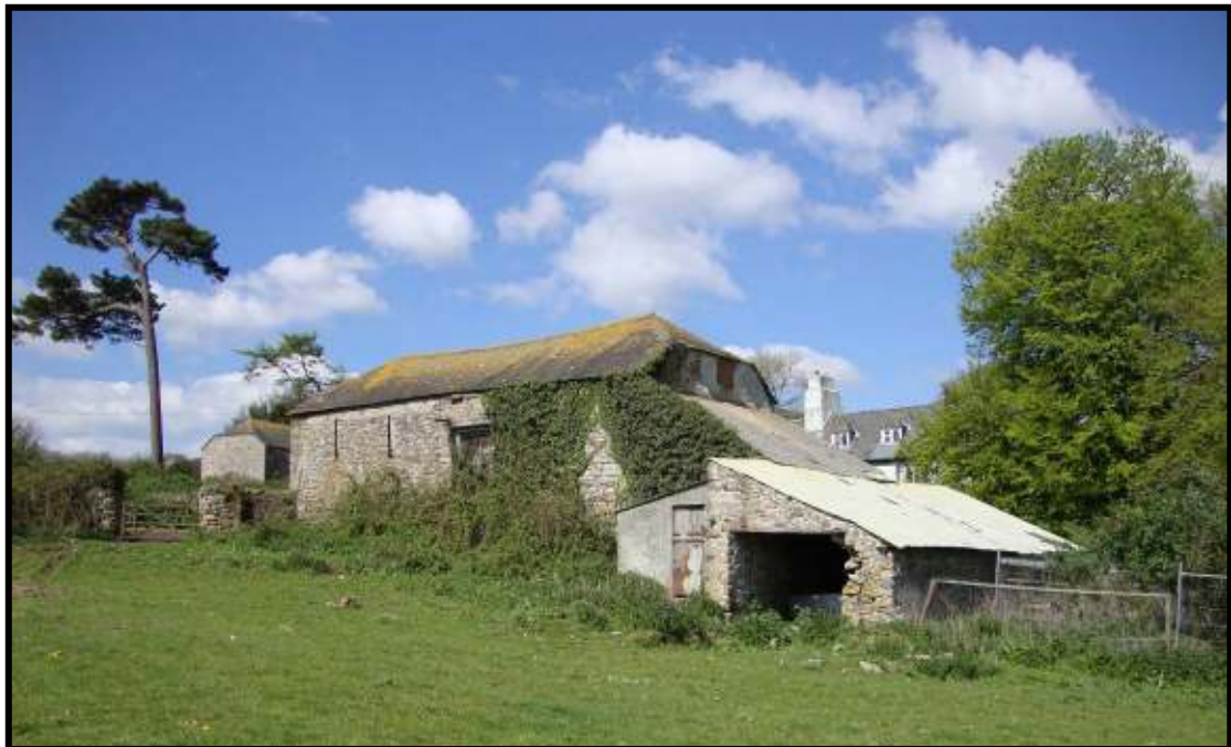
Fig. 7. View of the barn from the east, looking west, showing the lean-to structures against the north-eastern wall and the half-hipped gable of the original structure showing above these.
