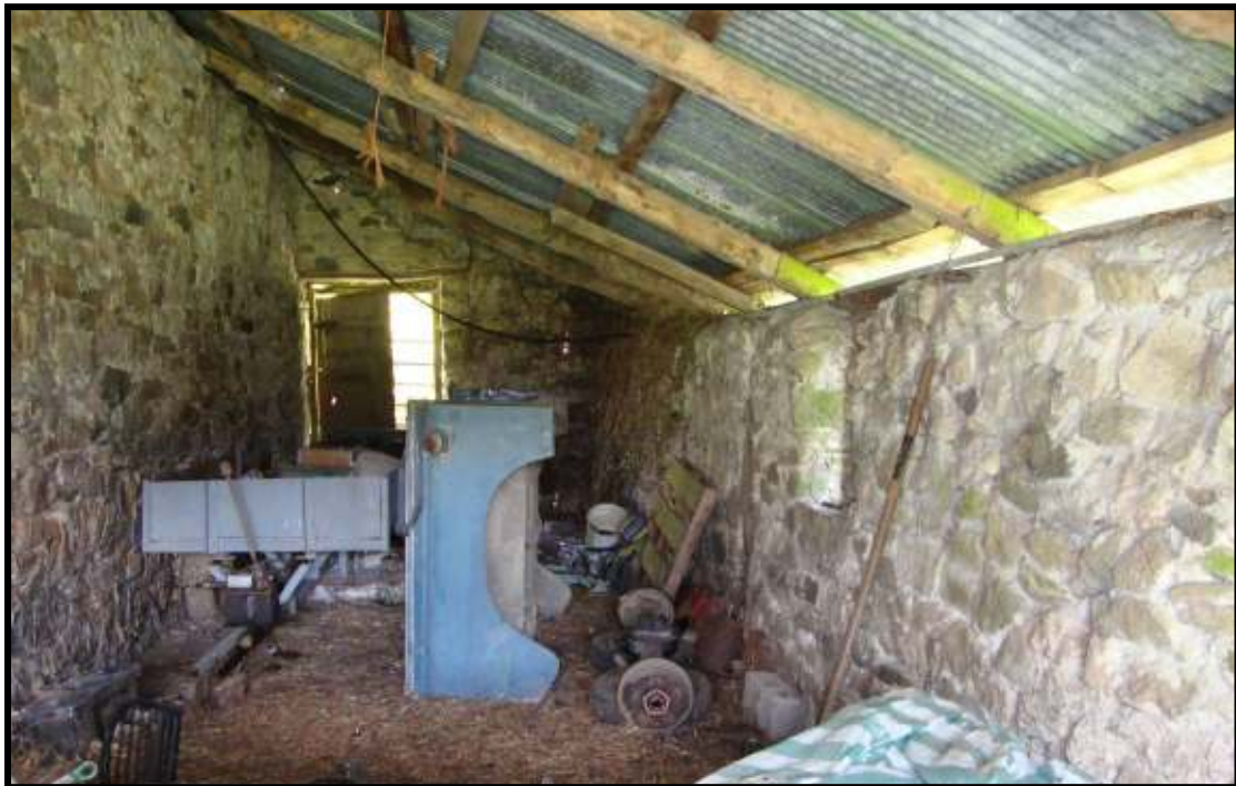
Fig. 17. Interior of the linhay showing the modern roof structure and the wall (right) infilling the gaps between the monoliths.
