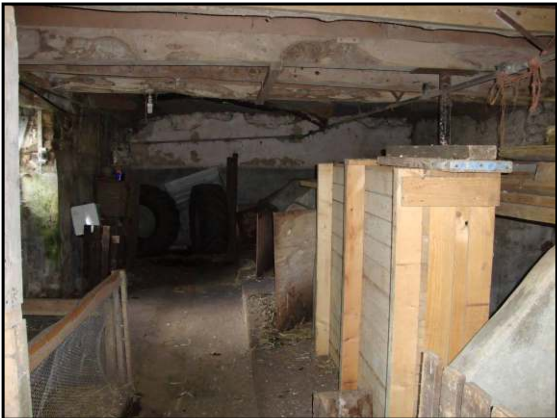
Fig. 10. Interior of the shippon, looking to the north east, showing the concrete stalls and the beams reinforcing the threshing floor above.
