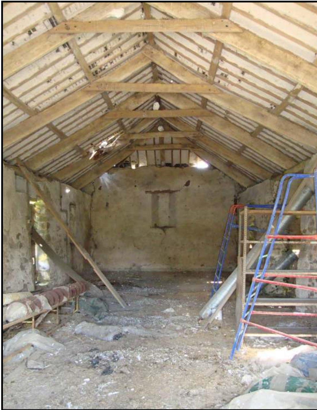
Fig.11. Interior of the first-floor threshing barn showing the opposed doorways in each side, the blocked ventilation slit in the north-eastern gable and the structure of the roof.
