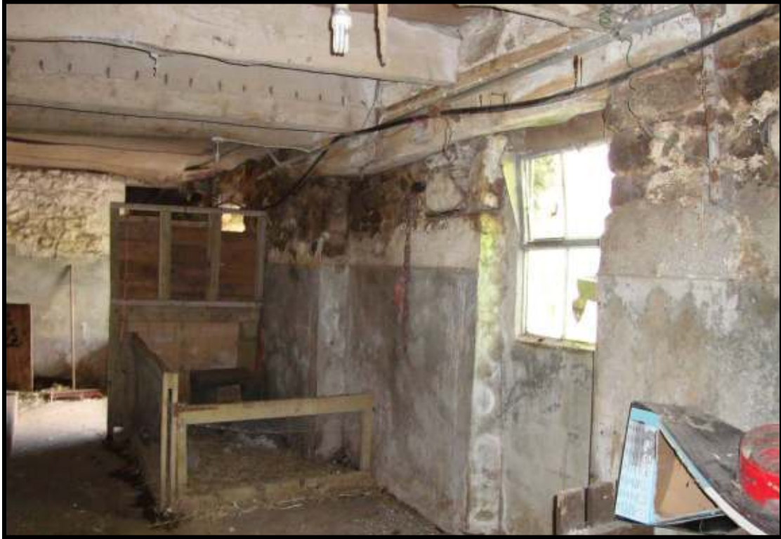
Fig. 9. Interior of the ground floor, looking west, showing the wide blocked doorway in the north-west wall, which is balanced by a similar doorway opposite.
