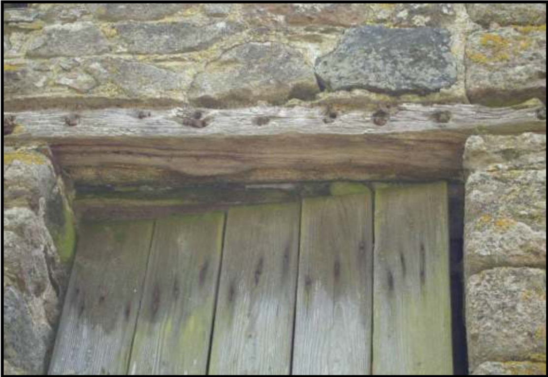
Fig. 13. Detail of the lintel above the lean-to loft doorway showing the series of holes suggesting reuse of the timber from a rod and muntin partition.
