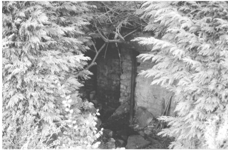
Plate 3: Close-up of entrance to air raid shelter
