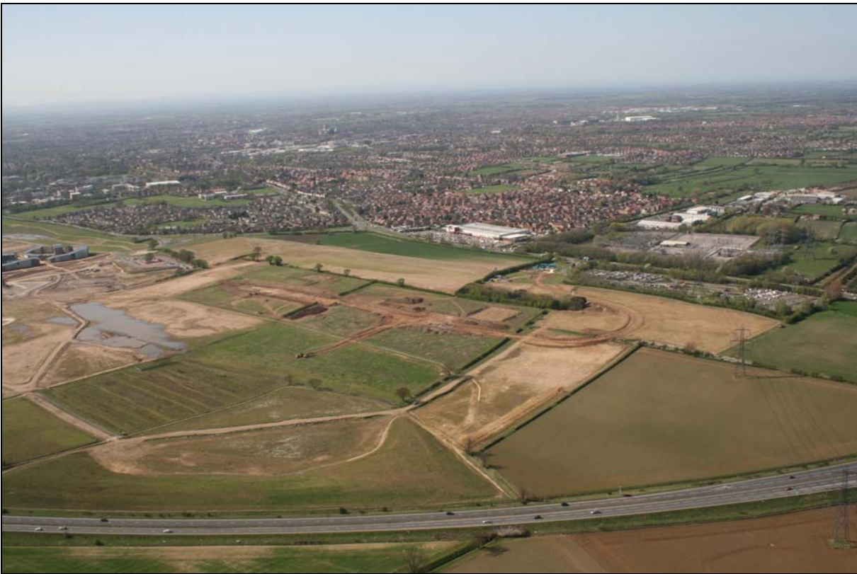
Plate 1. Aerial view of site, looking northwest
