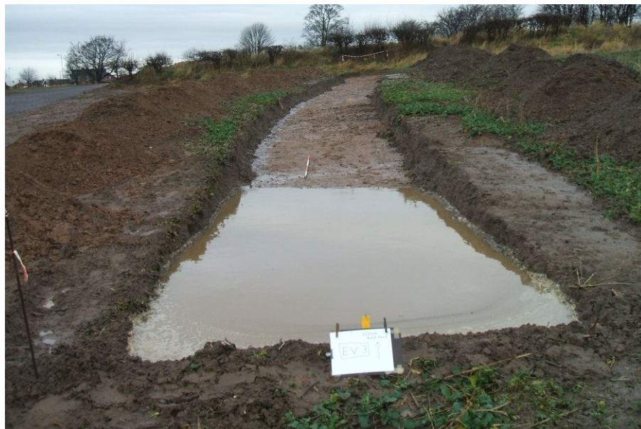
Plate 3 Trench 3, looking N
