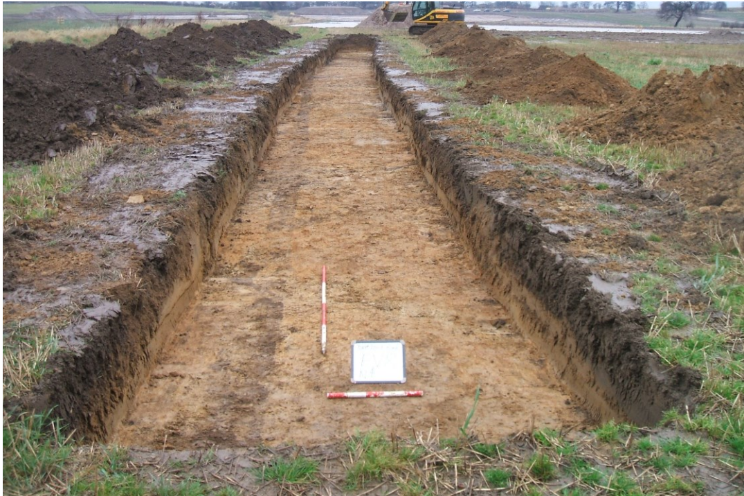
Plate 2 Trench 8, looking N
