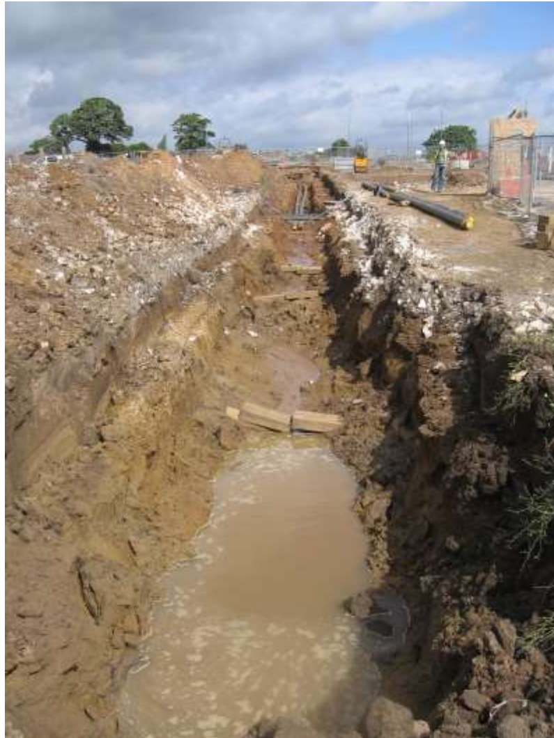
Plate 2 Services trench to the east of Goodricke College on completion, facing south.
