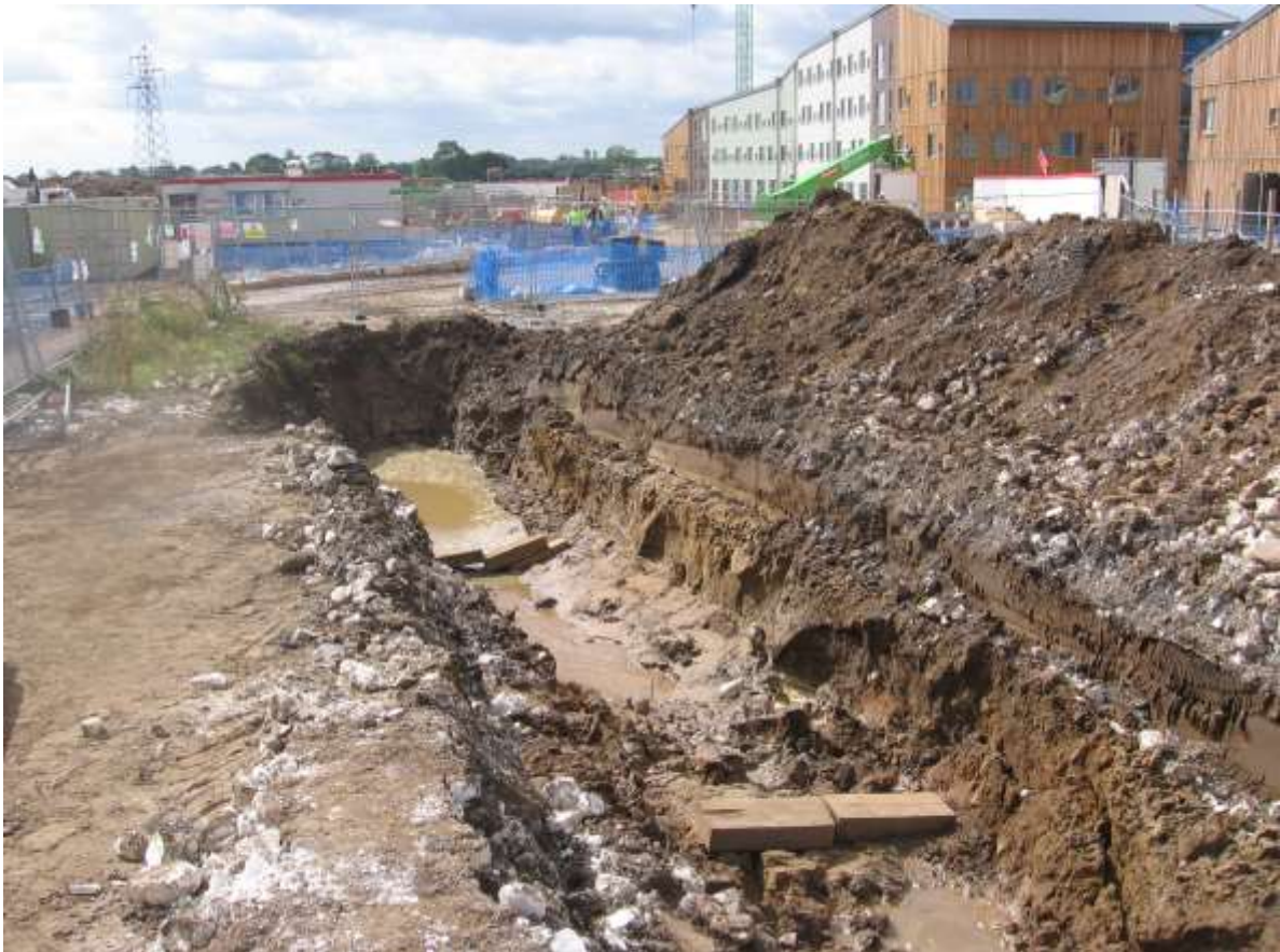
Plate 1 Services trench to the east of Goodricke College, facing south.
