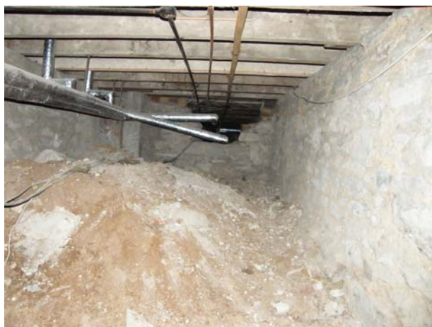
Plate 6: Mound of earth in boiler room
