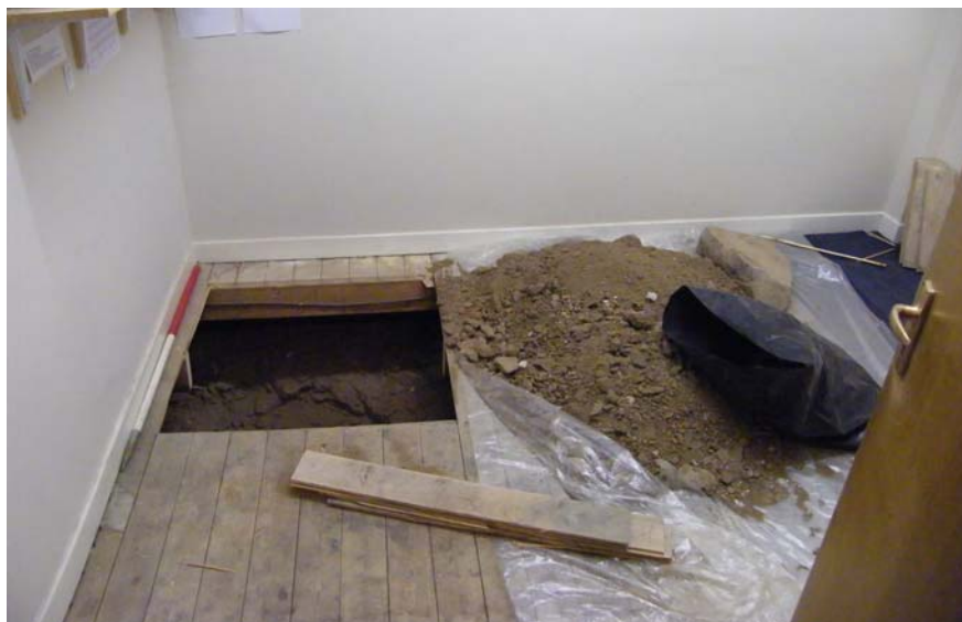
Plate 1: Site as left by contractors
