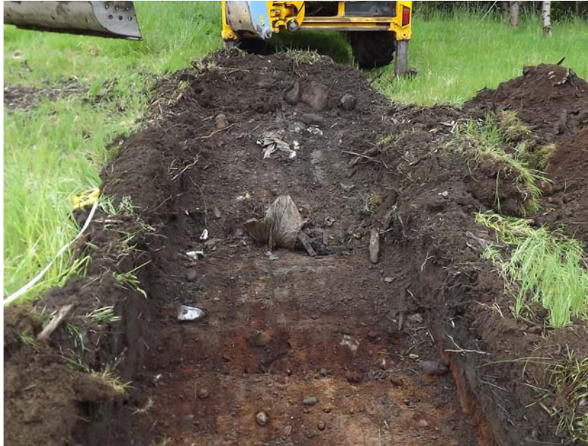
Plate 12 Working shot looking SW. Demolition rubble (1603) sitting directly atop (1602). (Photograph 101)
