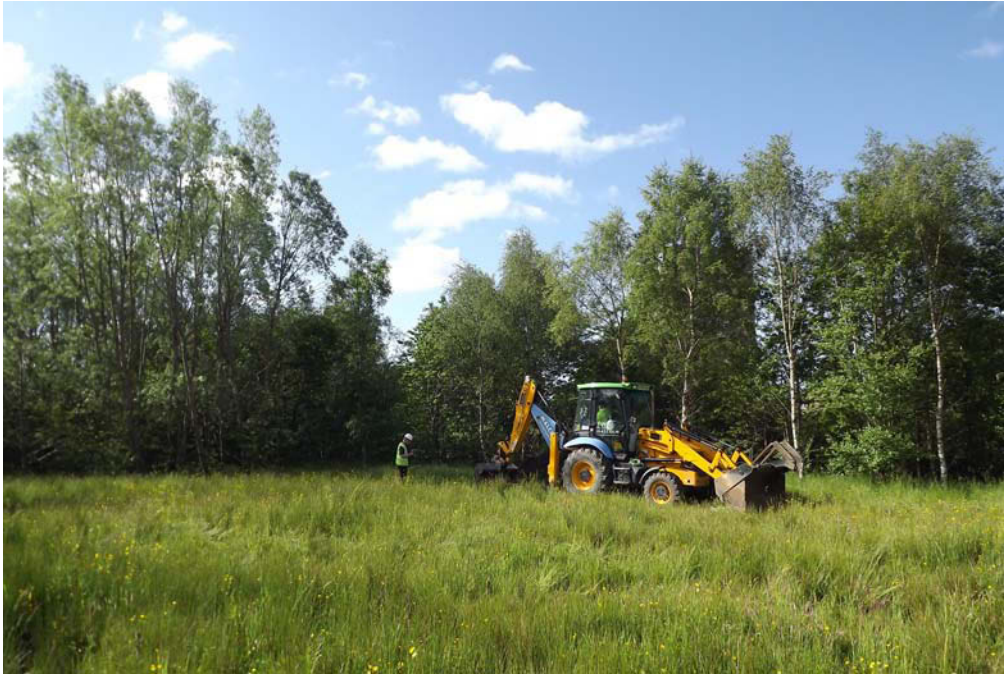
Plate 1 Monitoring the opening of Trench 1 (Photograph 004)
