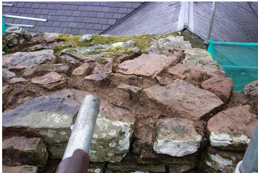
Plate 7: Detail of the concrete mortar of the wall head after weeding
