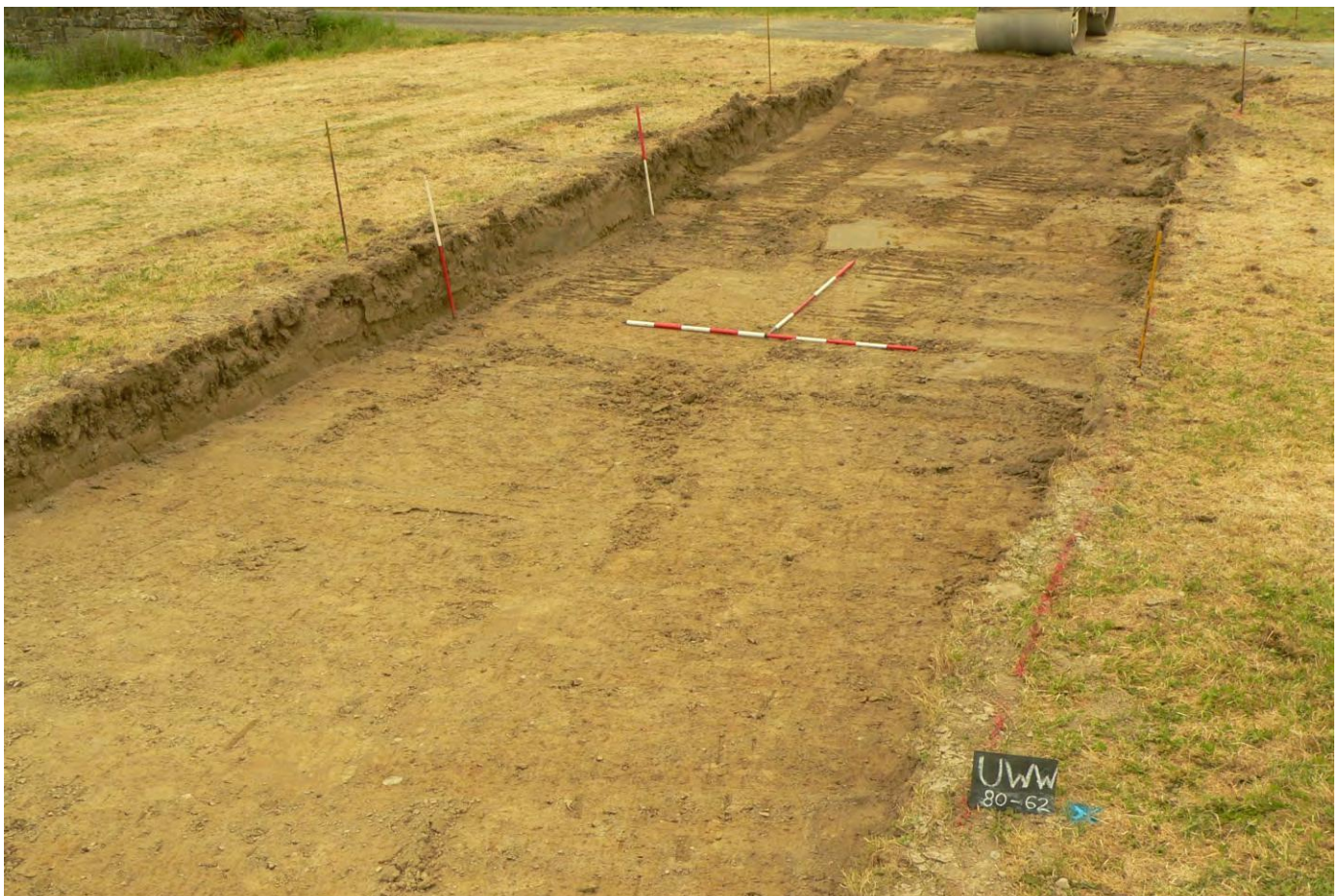
Plate 10 West field - finished formation level from 80 eastwards back to 62 metres west showing largely alluvial topsoil in base of roadline (the roller is sitting on the school driveway)
