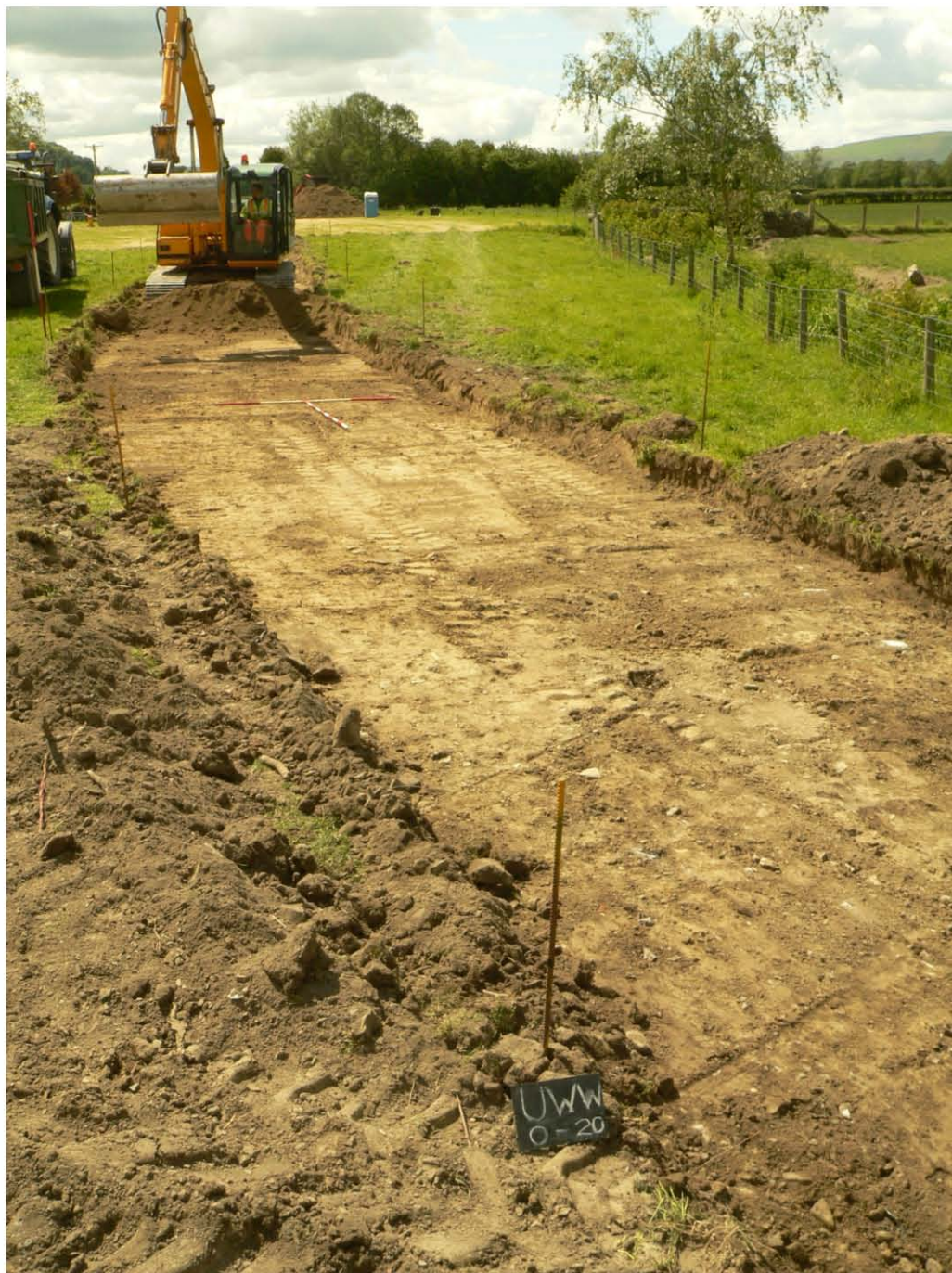
Plate 7 East field, east part - formation level from Zero to 20 metres (west) note the base of machining is still very much in alluvial topsoil
