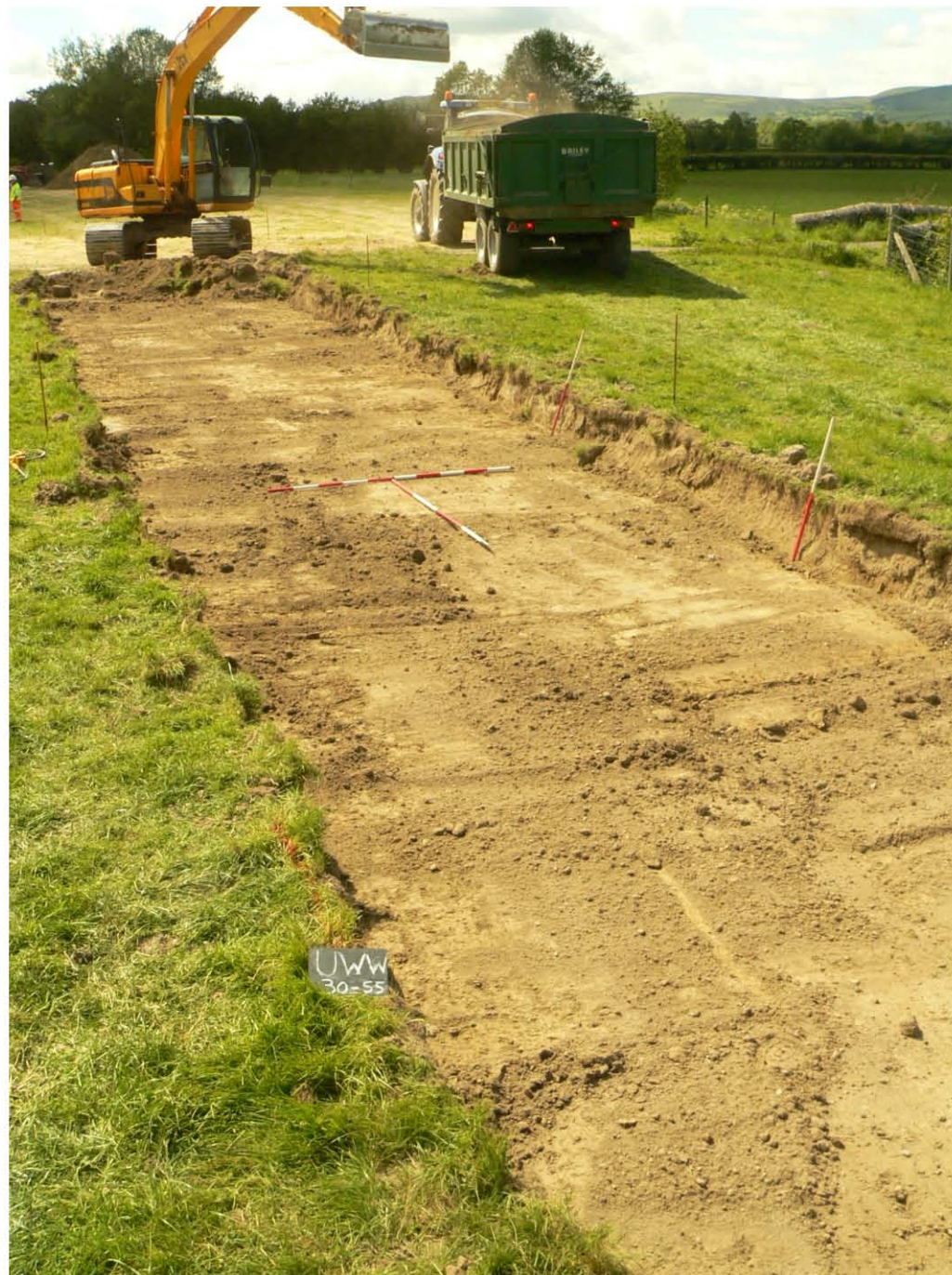
Plate 8 East field, west part - formation level from 30m to 55 metres (west) again, note that the base of machining is still very much in alluvial topsoil
