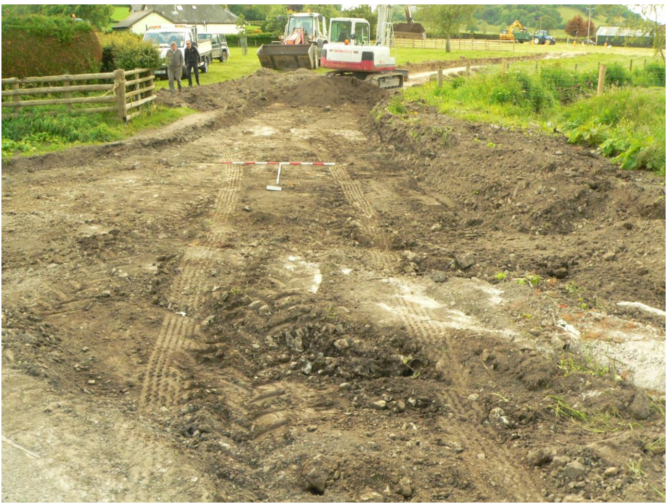
Plate 5 Splay / junction at the far east end of new road showing the intended formation level . The trench shown on Plate 6 is just to the right of the scales
