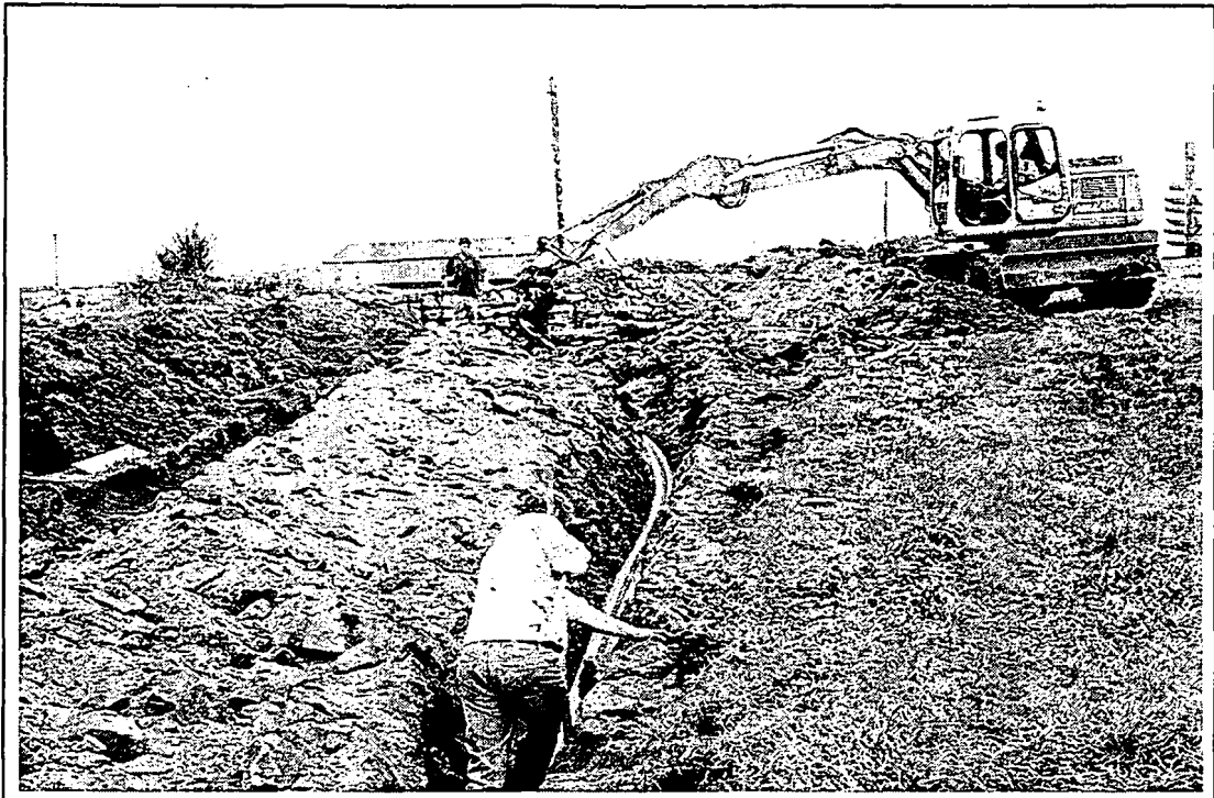
Fig. 20 The laying of the trench in Field 11.
