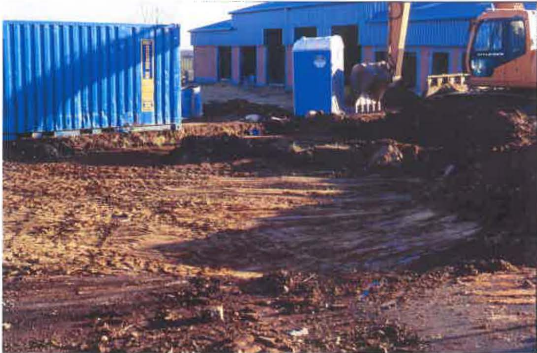
Plate 7: General view looking east from the original car park showing groundworks to northwest of new building.
