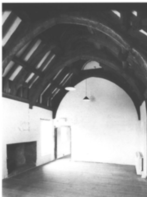
Figure 11.119 (top, right) The great chamber looking east. Note the skirting trunking for electrical services and electrical storage heater (photograph by David Garner, February 1995; EH B950946).
