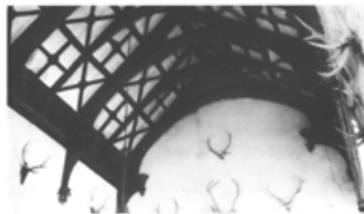
Figure 8.24 Orleigh Court, Buckland Brewer: the hall roof (EH/NMR BB69/615).
