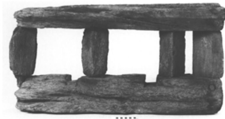
Figure 9.24 The diamond-mullioned window frame from the hall store, catalogue no. 135 (photograph by David Garner; EH B990456).
