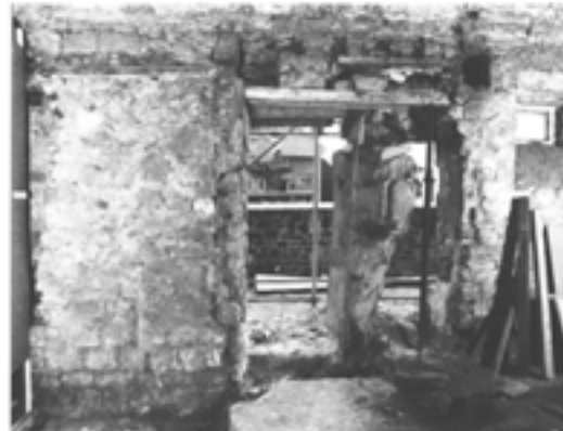
Figure 6.40 The south wall of the service rooms after stripping, but before any masonry repairs in 1985 ( see exterior view of the same, Fig 5.16), with window of phase 7 (for enlarged parlour), blocked in phase 8 and doorway of phase 9 (EH F850039/5).
