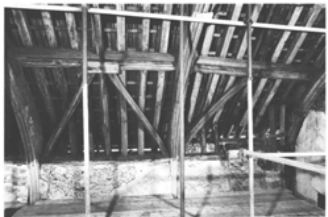
Figure 6.8 (below) Composite interior elevation of the east wall top of the hall prior to the removal of the roof for repair. These are important record photographs, since there is no other record of the cob (and stone patching) of the wall top, apparently butting the roof trusses (a northern half, trusses II–IV and b southern half, trusses IV–VI) (DoE J263/18/78 and J263/17/78).
