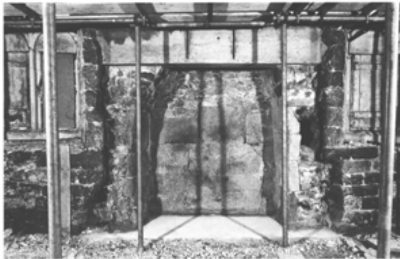
Figure 6.13 The fireplace in 1982 after the construction of the new concrete lintel and hearth (DoE J8/2/82).
