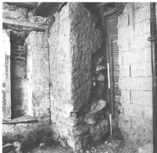
Figure 5.9 Southern end of the surviving west gable wall of the south range, showing original stone footings and cob wall and stone refacing of exterior face (right), looking south-west (photograph by David Garner; EH B940374).
