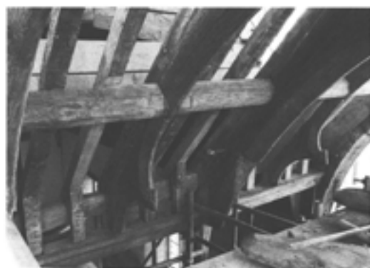
Figure 7.22 (bottom) The great chamber roof during reconstruction of the oversail of the roof of the east range in March 1990, looking south-west. Note the undecorated east face to truss 1 where it abutted the cob gable wall (photograph by Stuart Blaylock; EMAFU 1704/21).
