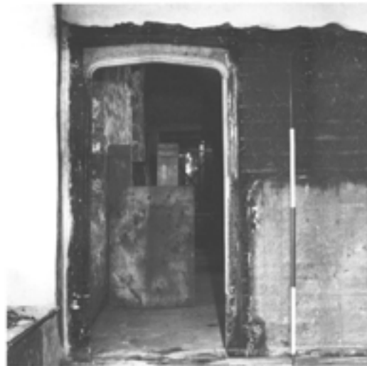
Figure 11.36 (top, left) The new stone arch to the through passage after external re-rendering. This shows limewash carried over wall plaster and stone mouldings to ensure the mouldings 'read' and following evidence of historic arrangements (photograph by David Garner, April 1996; EH B960560).
