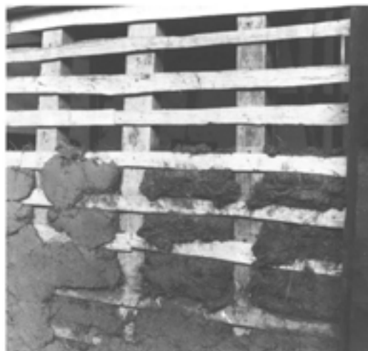
Figure 11.96 (top, left) Cob block 'blocking-up' around the repair area shown in Figs 11.74–75 (photograph by David Garner, May 1994; EH B942058).
