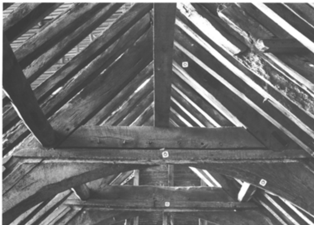
Figure 7.1 The roof of the south range, trusses X and XI (showing protruding pegs) seen from the rear face (photograph by Stuart Blaylock; EMAFU 1924/1).
