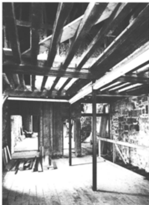
Figure 6.27 (right) As Fig 6.26, northern half looking west, also showing mortices for timber pegs in the side of the post of the screen to the hall (extreme right) (DoE J492/4/79).
