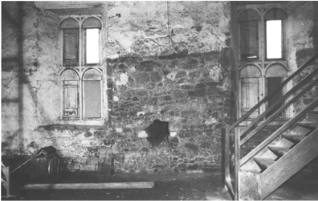
Figure 6.11 East wall of the hall, interior elevation in 1978 before the removal of the masonry blocking the fire- place. Note the moulded block (catalogue no. 112) in infill (white stone to the left of the hole in blocking) (DoE J10/7/78).
