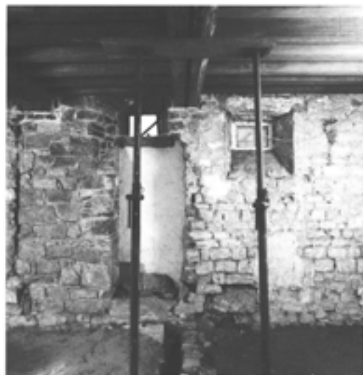
Figure 6.41 A similar view to Fig 6.40 in 1993, after two phases of masonry repairs and excavation of the sleeper wall for the screen (bottom) (photograph by David Garner; EH B933571).
