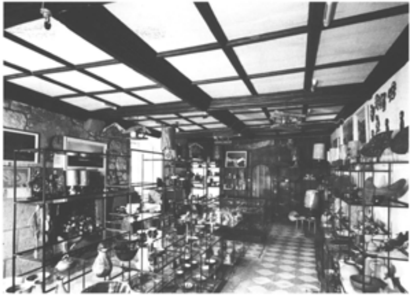
Figure 2.25 (above, left) Detail of the parlour ceiling in the 1950s, looking west, bays 2 (in foreground) to 4. Note the detail of the mouldings of the panels. The later shallower form is otherwise recorded only in a sketch (NMR AA 57/171).
