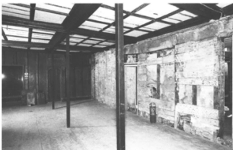
Figure 6.18 (above, left) The ground-floor partition at the south end of the hall after reconstruction but before infilling, 1987 (photograph by Keith Wiscott; EMAFU 1398/23).
