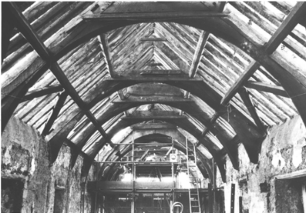
Figure 7.28 General view of the roof of the oriel and inner chambers in May 1988, looking east, with truss IX in the foreground. Note especially the differential treatment of the feet of the trusses: those on the right (lodged on the stone of the south wall) are cut off at the base of the arch braces; those on the left (set in the cob of the north wall) have long posts stretching down to floor level (see elevation Fig 6.25) (photograph by Stuart Blaylock; EMAFU 1449/23a).
