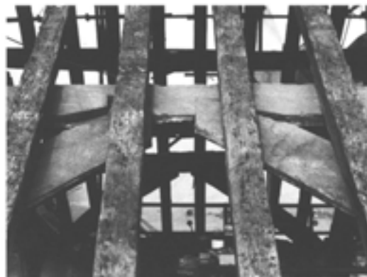
Figure 7.33 As Figure 7.32 from the outside, bay 8, south, showing the gap at the apex of the windbraces, looking north (photograph by Stuart Blaylock; EMAFU 1803/15).
