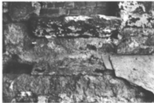
Figure 5.6 Detail of the breccia block reused as a window sill above the porch ( see Fig 5.2 ), August 1991 (photograph by Stuart Blaylock; EMAFU 1843/15).
