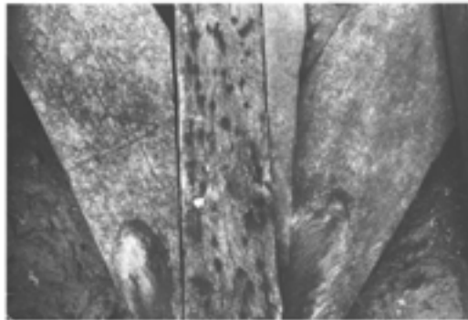
Figure 7.37 The lower ends of windbraces in the oriel chamber, showing assembly marks, truss X, bays 9/10, south side (photograph by Stuart Blaylock; EMAFU 1803/21).
