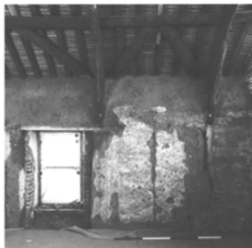
Figure 5.14 South elevation of the oriel chamber, showing position of the oriel (see detail in Fig 6.69), the foot of truss X bearing on the window lintel and the foot of truss XI bearing on cob. The brick facing of phase 8 post-dates the removal of cob west gable (extreme right) (photograph by David Garner; EH B931152).
