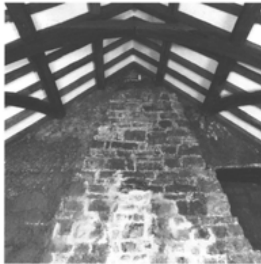
Figure 11.50 The north wall of the kitchen (first-floor chamber) showing the display of repairs: various daubed wall surface repairs and cob/lime wall face rebuilding to the left; cob brick piecing in to the niche on the right; lime-mortar repointing to the stonework (photograph by David Garner, February 1995; EH B950937).
