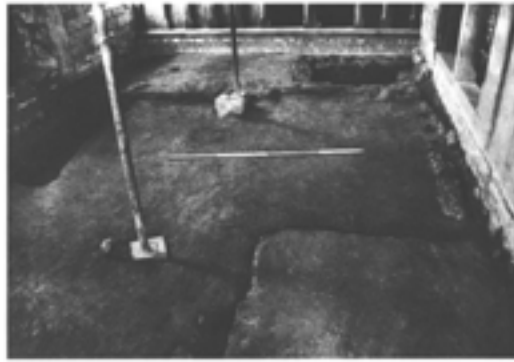
Figure 4.5 The early building beneath the parlour (phase 2) under excavation in 1989, looking west. Note the wall bases and the wardrobe pit at rear right. The vestigial nature of the structures is shown by the height of the wall bases (photograph by Stuart Blaylock; EMAFU 1581/11).
