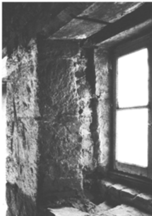
Figure 6.38 Detail of window 256 looking north-west, showing the chase for the frame in the reveal and lintel and the slot for a partition in the inner lintel (photograph by Keith Westcott; EMAFU 1488/28).
