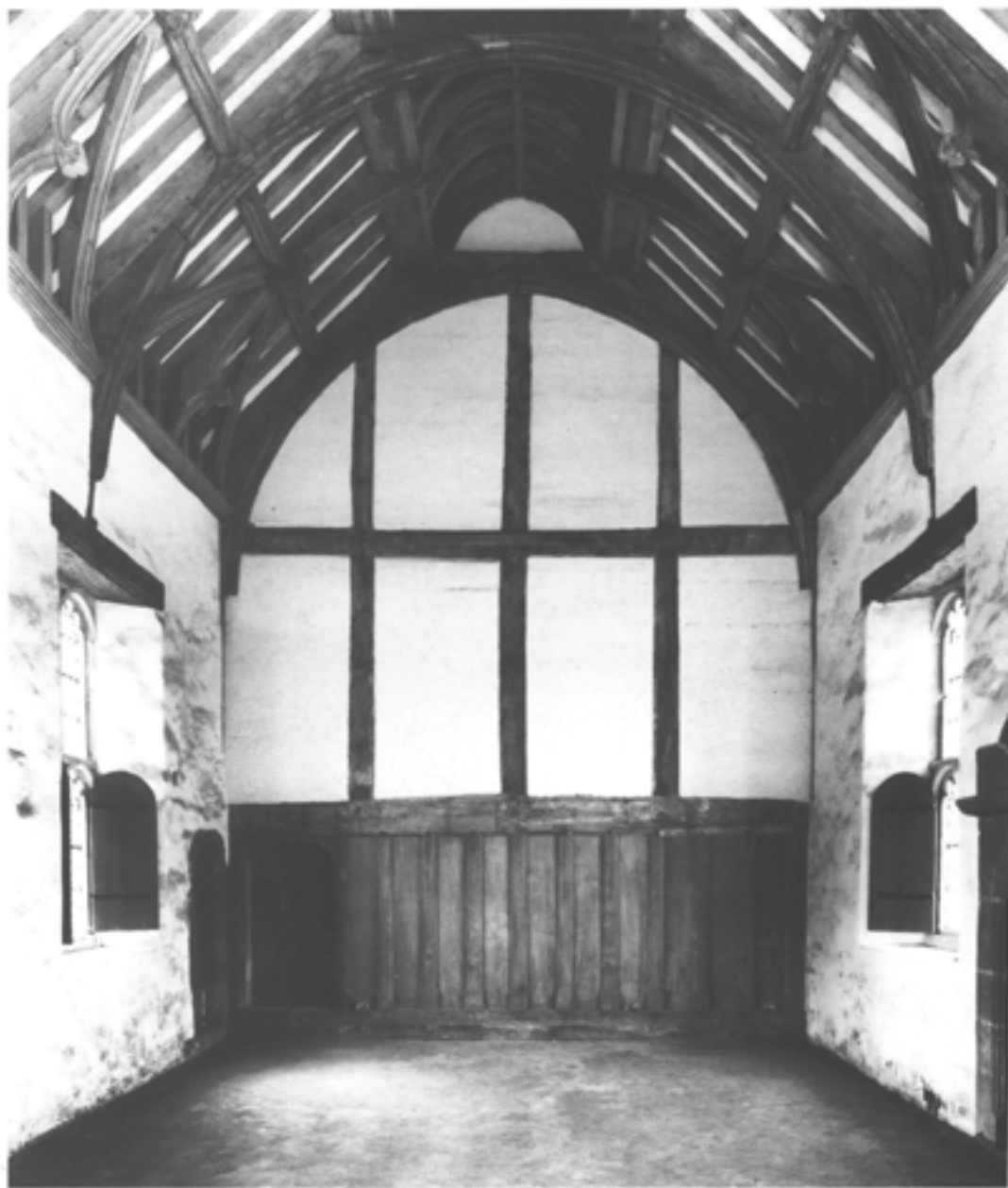
Figure 11.113 The hall, looking north, showing the restored northern partition and the roof (photograph by David Garner, May 1994; EH B942049).
