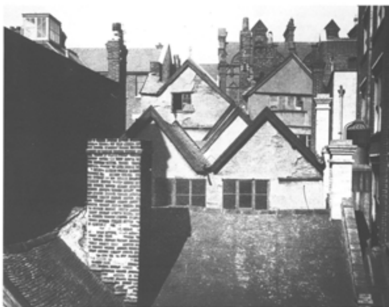
Figure 9.3 Old roofs at the rear of 76–81 Fore Street, Exeter, in 1893 (reproduced courtesy of the Westcountry Studies Library, Exeter).
