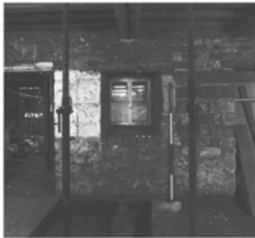
Figure 6.37 North elevation of the service rooms in July 1993 (photograph by David Garner; EH B933570).
