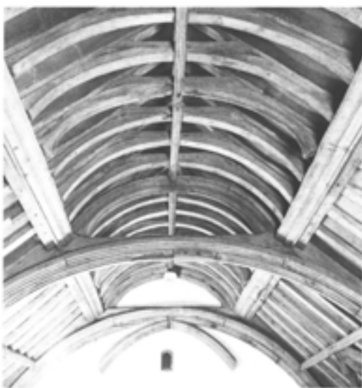
Figure 8.22 Cadhay, the hall roof: detail of the coving, upper purlins and arch braces (photograph taken by David Garner with kind permission of O N W William-Povelett Esq; EH B960126).
