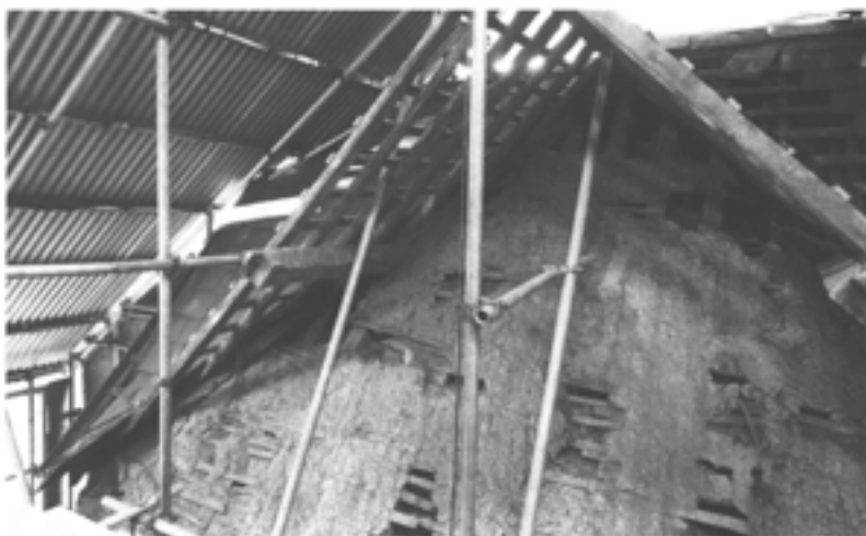
Figure 7.11 (top) The southern end of the hall roof, trusses V and VI, with lath and mud-plaster sealing of south range roof (beyond) (DoE J263/26/78).
