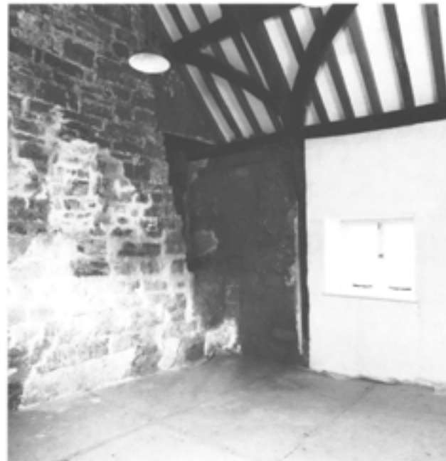
Figure 11.129 (left) The kitchen chamber, looking north-west and showing walling left unplastered, subsequently plastered over (photograph by David Garner, February 1995; EH B950936).
