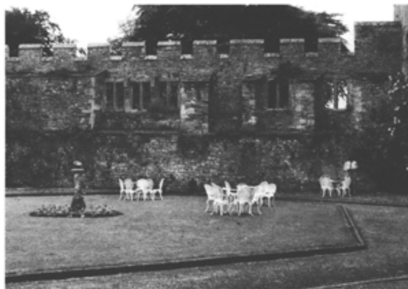
Figure 8.3 Thornbury Castle, Gloucestershire, the stone boundary wall of the gallery around the Privy Garden: (left) west wall, interior (EA 3431/21); (right) detail showing the blocked doorway that gave access to the gallery (via stairs) from the first floor of the adjacent range (EA 3431/34) (photographs by Stuart Blaylock).
