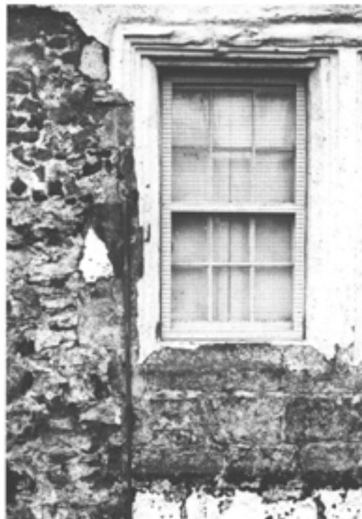
Figure 5.3 (left) The reveal of the east window of the hall store. Note the inner splay and the chase for a timber frame, looking south-west, 1985 (EH C850070).
