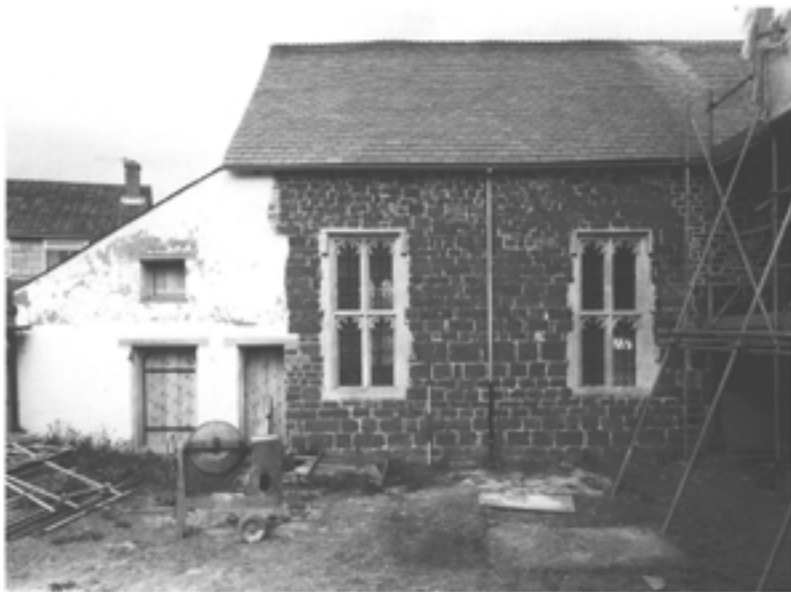
Figure 11.86 (above) The west elevation of the hall; the windows tracery has been fully reinstated and the secondary window removed and blocked (highlighted by the distinctively sized, coursed and pointed masonry at the upper right-hand side). Notice in the roof the 'pig'-course (sudden diminution) near the ridge. This mistake in laying out had to be perpetuated in the Stage 2 roofing of the south range (photograph by David Garner, April 1992; EH A920553).
