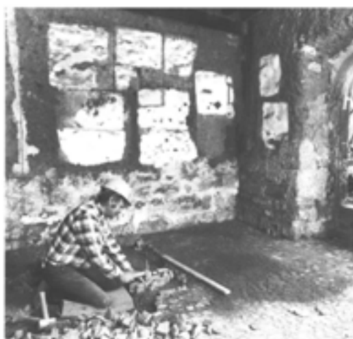
Figure 11.43 (below, left) Laying the floor in the screens passage: cobbles in a cob mix (photograph by David Garner, July 1991; EH B917144).
