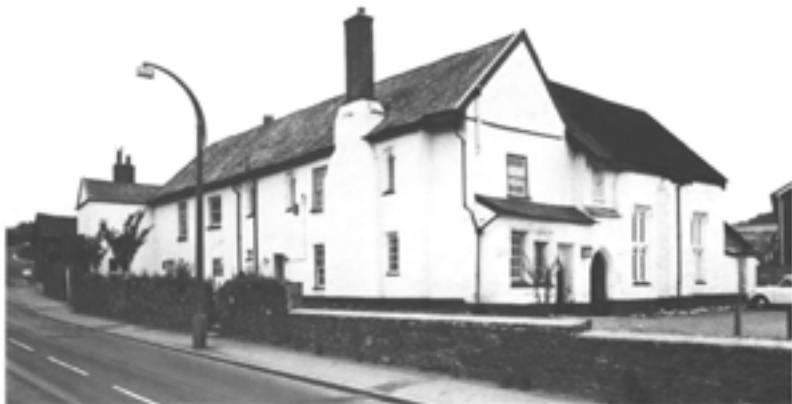
Figure 2.11 The building from the south-east in 1969 (RCHME BB69/5012).
