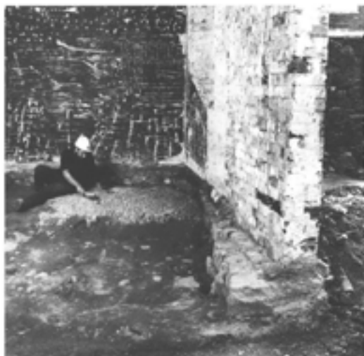
Figure 4.26 Excavation within the annexe in July 1994, looking south. Note the two walls on different alignments (photograph by David Garner; EH B943785).
