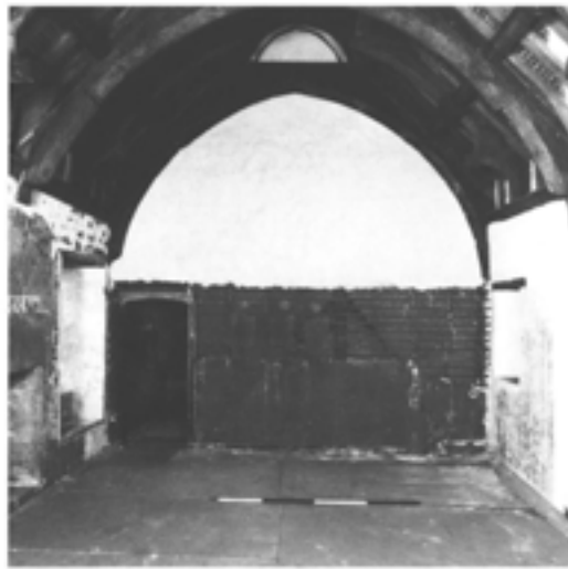
Figure 11.17 (below, left) The framed wall panel ('daub screen') between the great chamber and hall with most oak lathing reinstated in the early stages of being daubed, looking north (photograph by David Garner, October 1990; EH B906970).
