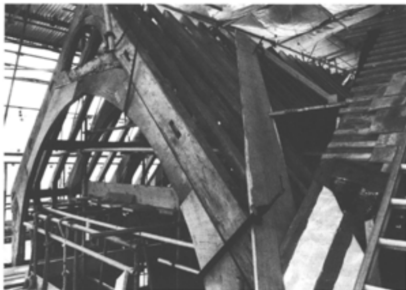
Figure 7.22 (bottom) The great chamber roof during reconstruction of the oversail of the roof of the east range in March 1990, looking south-west. Note the undecorated east face to truss 1 where it abutted the cob gable wall (photograph by Stuart Blaylock; EMAFU 1704/21).
