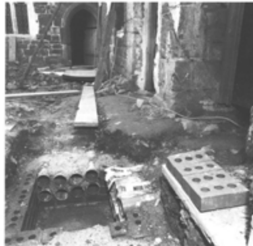
Figure 11.54 The draught under construction below the floor of the pentice passageway (photograph by David Garner, March 1994; EH B940969).
