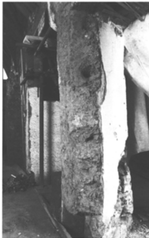
Figure 6.70 The west reveal of door 200 formerly leading to the gallery, showing reverse splay, looking west (photograph by David Garner; EH B940400).
