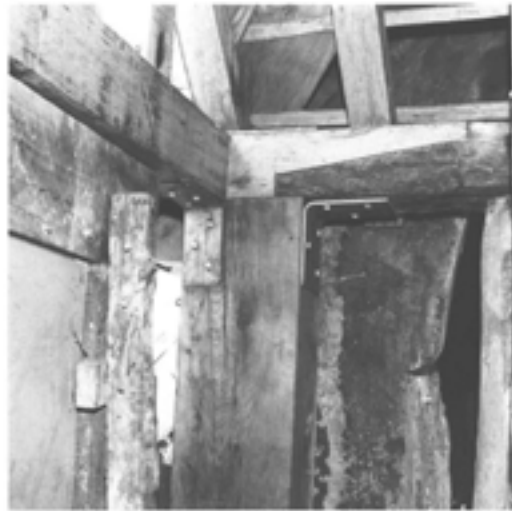
Figure 11.74 (top, left) The jointed-cruck post of west range truss 1, seen from the south. The repair was designed to slide into place from the side and was fixed to the original by three oak pegs; the engineer's recommendation was '1) prop post from cruck down to floor to allow post to shrink upwards and 2) pack to make good any shrinkage' (MS specification by Arthur McCallum, December 1992) (photograph by David Garner, March 1994; EH B940979).
