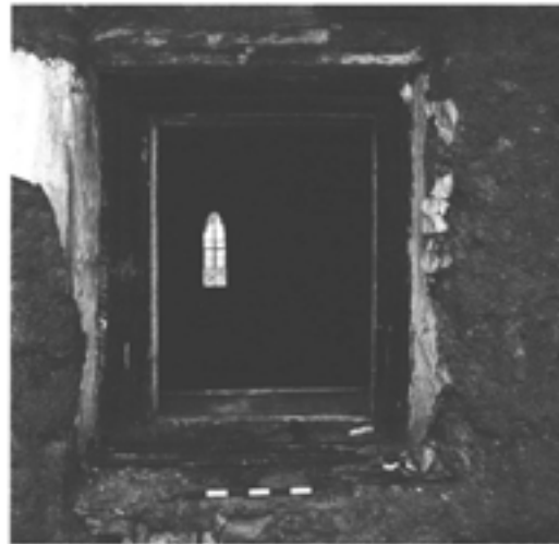
Figure 5.20 Detail of window 137 showing the inserted moulded frame and the original lintel (photograph by David Garner; EH B934812).
