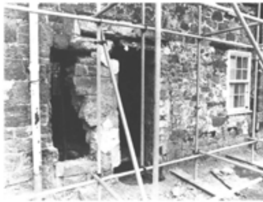
Figure 5.16 The south range, exterior, detail of the south wall of the parlour/service rooms in August 1985, before commencement of rebuilding: pair of windows of phase 7 and blocking of phase 8, doorway of phase 9 (EH F850039/3).
