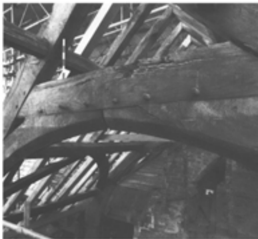
Figure 7.39 General view of the interior of the roof of the west range, with truss II in the foreground, looking south. Note the protruding pegs (photograph by David Garner; EH B930166).
