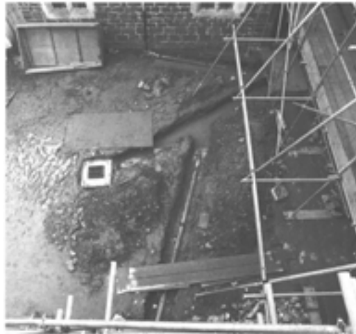
Figure 4.14 Service trenches dug for drains in the central courtyard, December 1993, looking east (photograph by David Garner; EH B936795).
