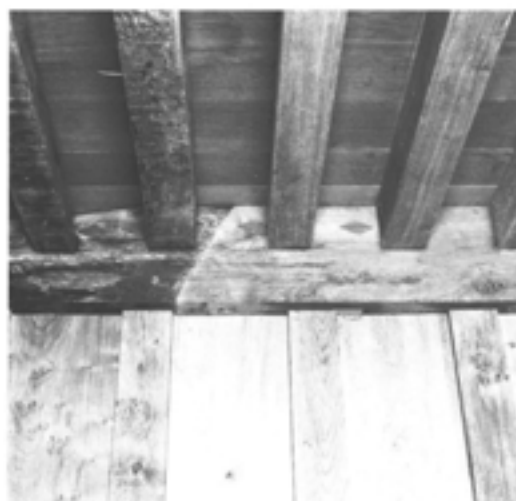
Figure 11.69 The ceiling/first floor structure in the south range service room, with reinstated beam 6 doubling as headbeam to a new partition. Note the original (left) and reinstated (right) floor joists. The diamond-shaped timber pellets conceal the heads of bolts connecting a concealed metal fitch plate to the timber, a standard modern 'traditional' solution. The profile of the new timbers matches that of the originals (photograph by David Garner, April 1994; EH B942043).
