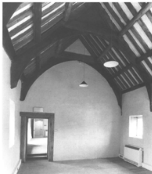
Figure 11.122 (top, left) The inner chamber, looking west to new cob wall (photograph by David Garner, June 1995; EH B953006).
