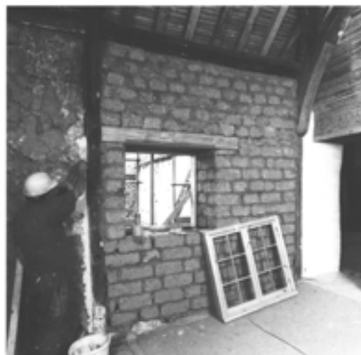
Figure 11.29 Completed cob block reinstatement to the east wall of the kitchen chamber, including the new window. The window had no historic precedent and was introduced to bring extra light into the room (photograph by David Garner, July 1994; EH B943806).
