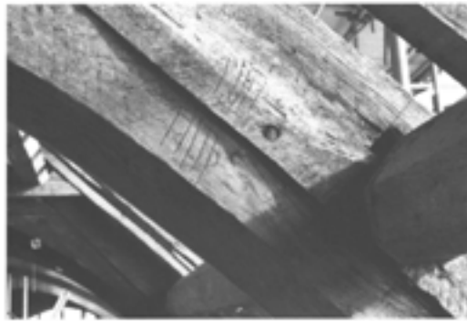
Figure 7.36 Detail of assembly marks on truss IX, south side, principal rafter and arch brace (photograph by Stuart Blaylock; EMAFU 1803/2).
