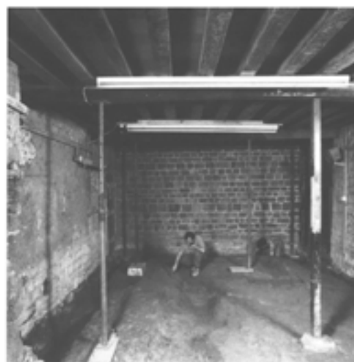
Figure 4.11 Excavation of the west service room of the south range in September 1993, looking east. Note the foundation trench to the left and the rebuilt stone cross wall in the background (photograph by David Garner; EH B934821).
