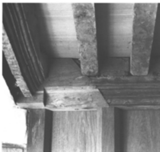
Figure 11.70 The south end of beam 4 reinstated (south-west corner of the parlour). Here the profile of the new work is deliberately left un moulded to confirm the repair by more than just its newness. The lamination of timbers facing the repair suggests that it is in situ shuttering for a mass resin repair (photograph by David Garner, April 1994; EH B942038).
