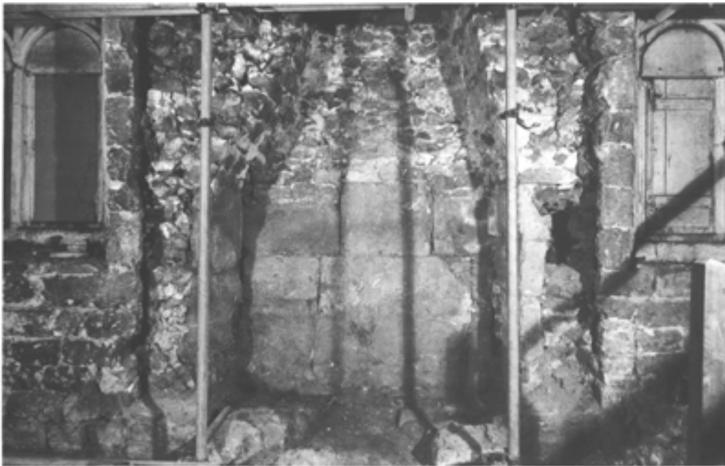
Figure 6.12 Detail of the fireplace in 1981 after the removal of the blocking (DoE J11/5/81).
