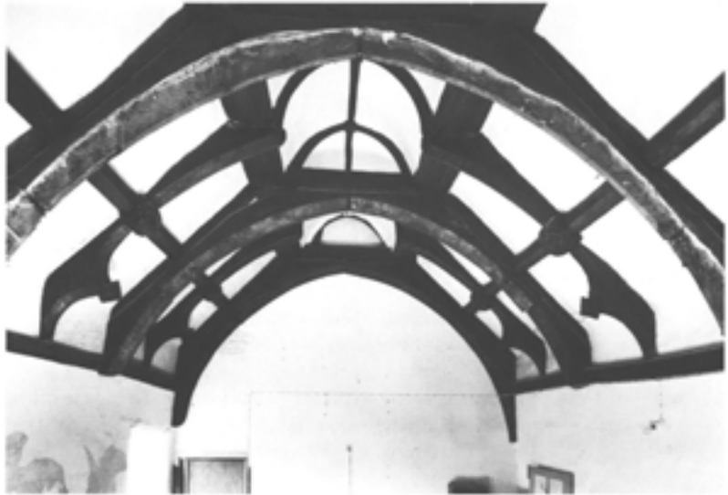
Figure 2.26 (above, right) The parlour in 1969, looking west (RCHME BB69/5034).
