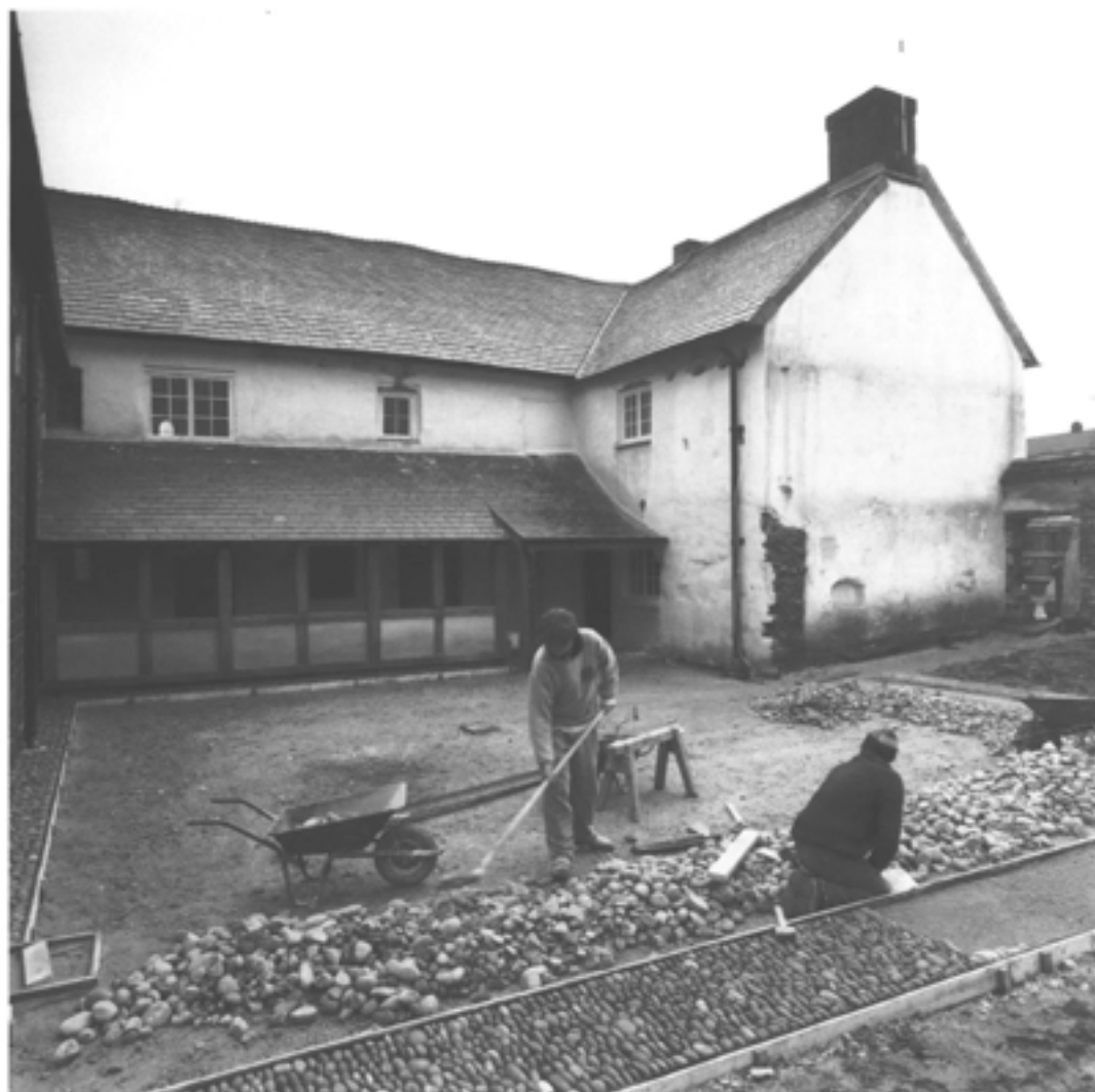
Figure 11.46 View of the courtyard. Note the examples of 'didactic' display in the north gable of the kitchen (the scar of the wall of the west range and the chase of a door frame above) set into the modern render. In the foreground, the laying of stone pitching on the lines of the demolished walls is in progress, again didactic in purpose (photograph by David Garner, February 1995; EH B950948).
