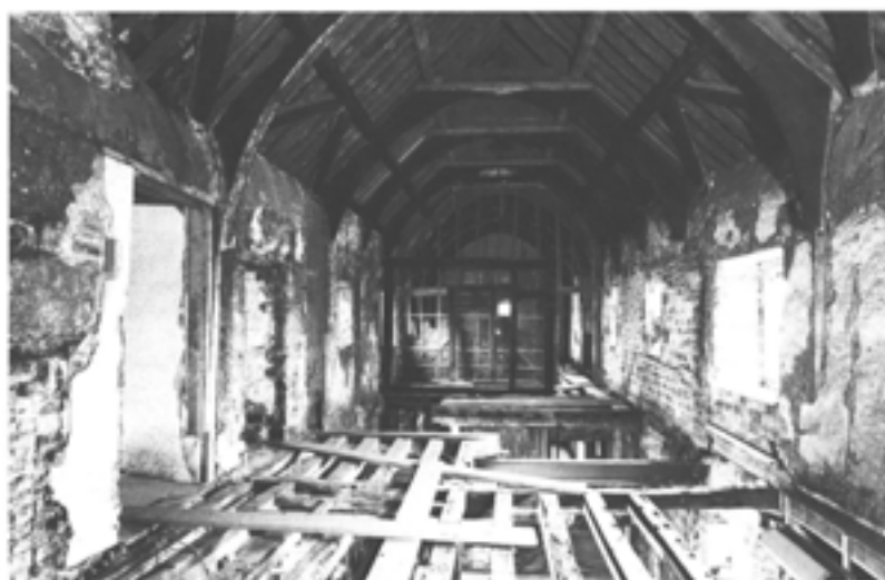
Figure 6.61 (top) The inner chamber looking east after first stripping in July 1978. Note the differential walling materials and 17th-century screen beneath truss VI (DoE 263/13/78).
