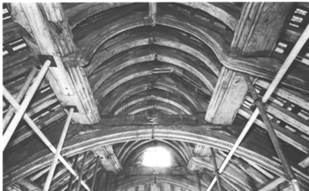
Figure 7.10 The apex of trusses II and III in 1978, showing the coving and the structure where one cove brace is missing (right) (DoE J263/22/78).
