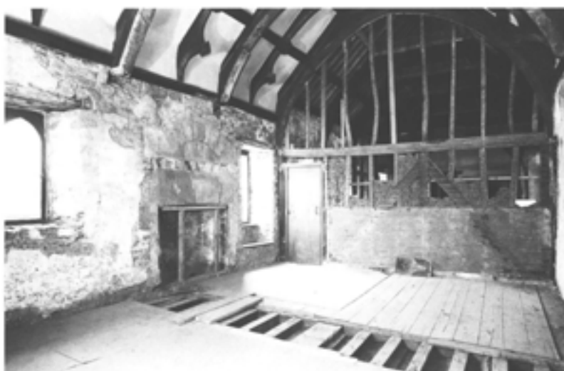
Figure 6.57 (top) The north elevation of the great chamber in July 1978, looking north-west, with later lath and plaster removed, showing the original plaster face and the posts of the roof trusses (DoE J263/14/78).
