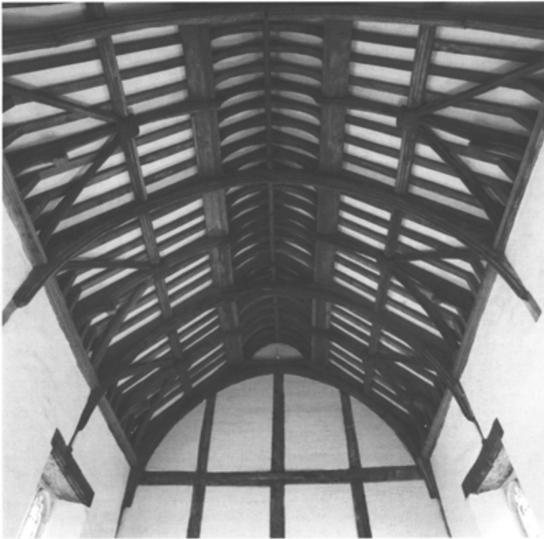
Figure 7.7 The hall roof after repair, May 1995, looking north (photograph by David Garner; EH B953012).
