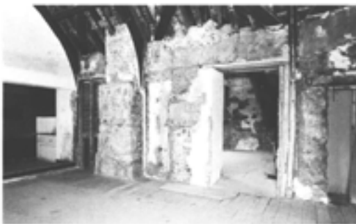
Figure 6.66 The north elevation of the oriel chamber when first stripped, July 1978 (DoE J263/9/78).
