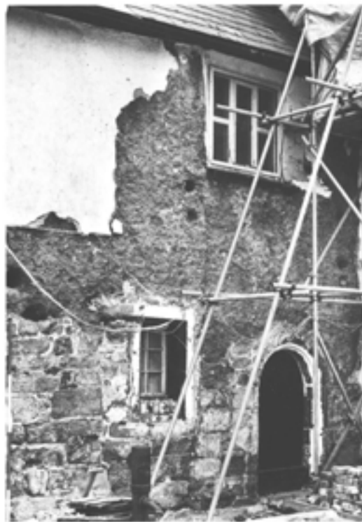
Figure 5.23 The west elevation stripped in August 1988 (photo- graph by Keith Westcott; EMAFU 1497/13).
