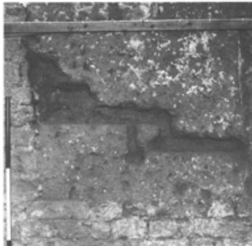
Figure 6.44 Cob of the south elevation showing the secondary chase for a stair ( see Fig 6.22, 342) at the junction of cob and stone walling (photograph by David Garner; EH B940402).
