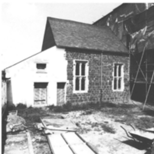
Figure 11.12 The west elevation of the completed hall store; almost all the rendered walling is new (photograph by David Garner, July 1991; EH B917152).
