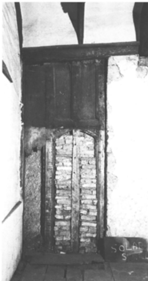
Figure 6.55 Doorway in the south-east corner of the chamber (formerly leading to the south-east range), itself secondary (?phase) and blocked in phase 8 (DoE J263/16/78).
