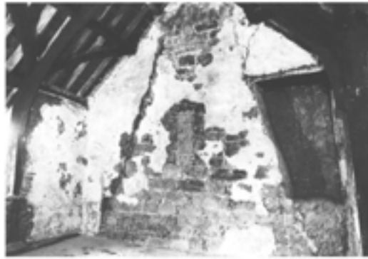
Figure 6.48 The north elevation of the kitchen at first-floor level, showing the masonry chimney flue and cob walling to each side. Note the extent of surviving plaster at this time (July 1978; DoE J263/8/78).
