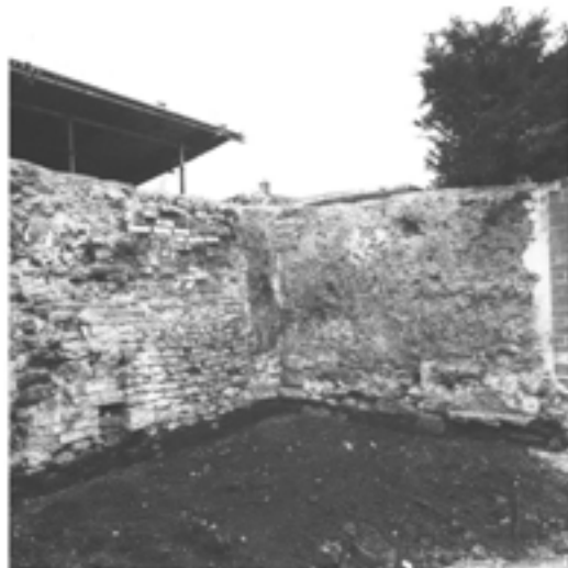
Figure 5.24 The north-west corner of the courtyard in November 1994, originally the interior elevation of the west/north ranges. Note the primary cob and stone footings (photograph by David Garner; EH B945706).
