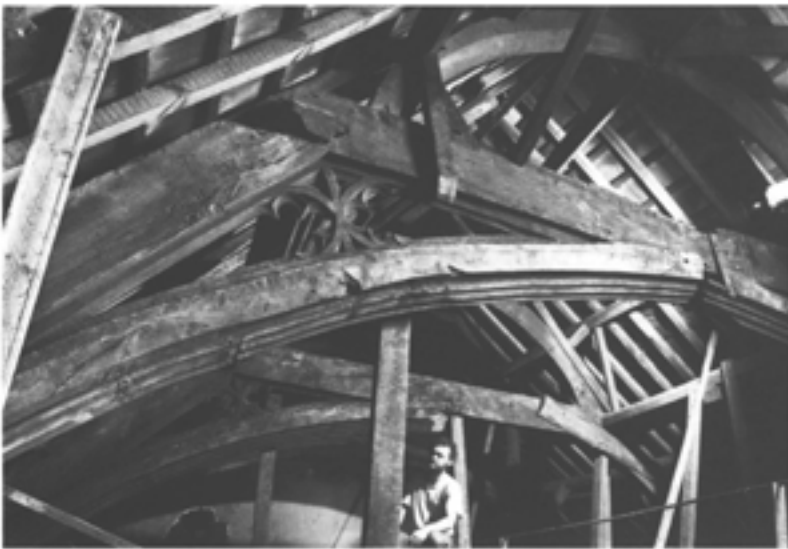
Figure 8.7 Archdeacon of Exeter's House: short principal, collar and arch braces. Note the tracered spandrels and sawn-off upper purlin (photograph by David Garner; EMAFU 3326/12) (source: Exeter Archaeology; © Exeter Archaeology).
