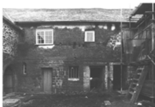
Figure 5.19 The north elevation of the south range in February 1994, showing the wall stripped and partially repaired. Note the sockets for the roof of the pentice (cf elevation Fig 5.17, 346–7; this was the only occasion that the elevation was free of scaffolding, when any of these features were visible) (photograph by David Garner; EH B940403).
