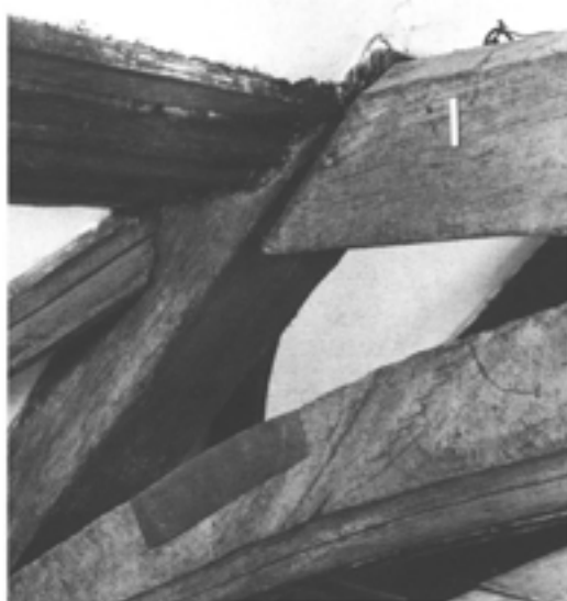
Figure 8.14 Exeter Guildhall: main truss, detail of the collar/arch brace/upper purlin assembly (photograph by David Garner; EA 3620/07) (source: Exeter Archaeology; © Exeter Archaeology).
