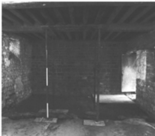
Figure 6.39 The western service room, looking west to the rebuilt cross wall (on original footings) in July 1993. Note the sleeper wall for the screen (photograph by David Garner; EH B933566).
