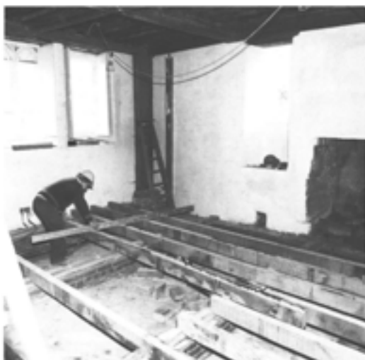
Figure 11.41 (above, left) Section through the cob/lime hall floor, when cut back to accommodate new floor finishes in the screens passage (see Fig 11.43) (photograph by David Garner, June 1991; EH B917139).
