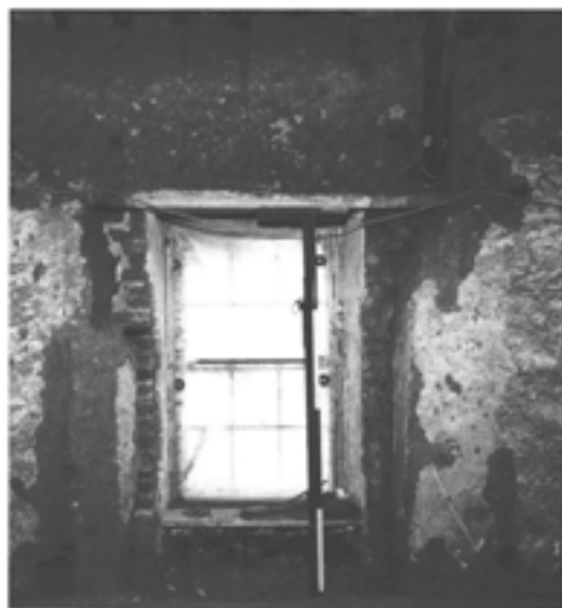
Figure 6.68 Detail of the oriel window. Note the splayed reveals with primary plaster, later brick filling behind and the foot of truss X bearing on the lintel (photograph by David Garner; EH B930204).
