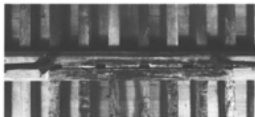
Figure 6.35 Beam 6 seen from below, west at the top (restored to north and south), showing mortises for the posts of the partition and the slot for plank infill (photograph by David Garner; EH B933112).
