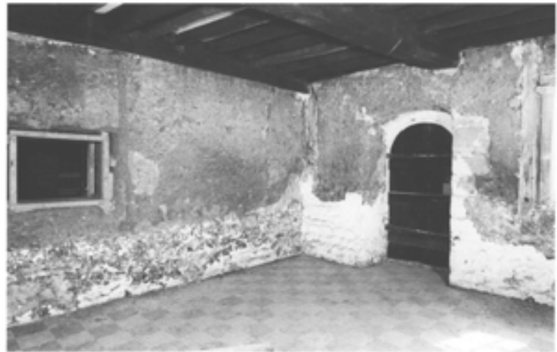
Figure 6.46 The ground floor of the kitchen, looking south-west. Note the relative height of cob/stone footings, the door of phase 5 (cut into cob) and the inserted floor (DoE J263/3/78).
