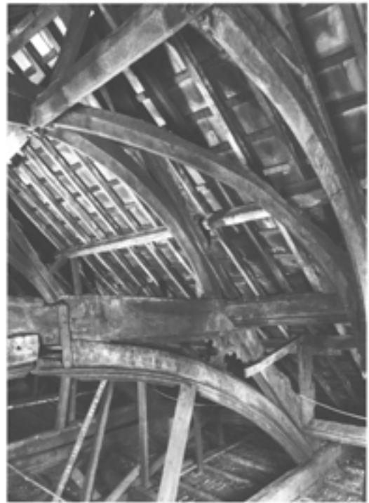
Figure 8.8 Archdeacon of Exeter's House: purlins and 'vaulting' ribs (photograph by David Garner; EMAFU 3326/5) (source: Exeter Archaeology; © Exeter Archaeology).
