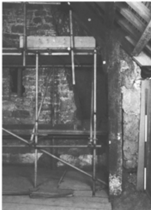
Figure 6.49 The east post of truss II of the roof of the west range, showing the different treatment of this roof. Here the roof trusses were raised first and the cob wall built around them; in section this view shows a narrow gap caused by the shrinkage of the cob (photograph by David Garner; EH B933511).
