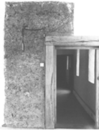
Figure 11.127 (top, left) A 'didactic window' in the south wall of the oriel chamber, showing the foot of truss X bearing on a window lintel and associated cob; now plastered over (photograph by David Garner, October 1996; EH B961847).
