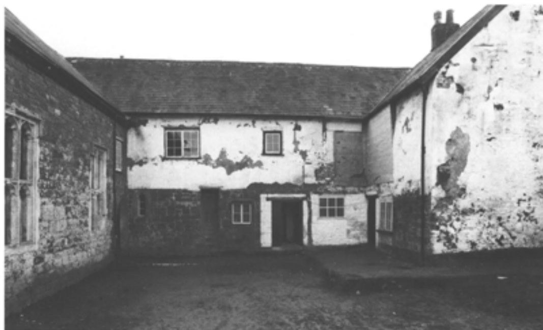
Figure 5.18 The north elevation in 1978, after the backfilling of excavations (DoE J10/3/78).
