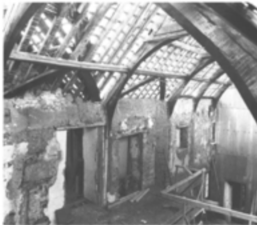
Figure 7.38 Oblique view of the north elevation of the oriel and inner chambers, when the floors were removed in October 1985. Note the scar of the cross wall, right of centre, and traces of ceilings in oriel chamber (EH B850150/6).
