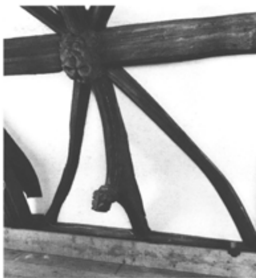
Figure 8.13 Exeter Guildhall: detail of bay 1, looking west, showing the intermediate truss and windbraces (photograph by David Garner; EA 3621/01) (source: Exeter Archaeology; © Exeter Archaeology).
