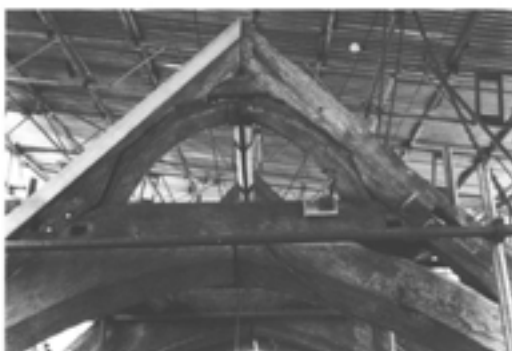
Figure 7.20 Detail of truss IV when the rafters of bay 4 were dismantled in April 1989, looking east. Note especially the mortices for the upper purlin and cove purlin (EH B891266).
