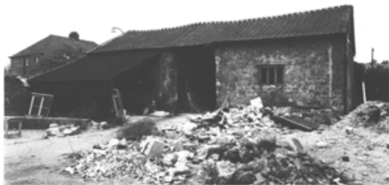
Figure 2.15 The east elevation of the barn in 1969. Note the three-light window (RCHME BB69/5022).
