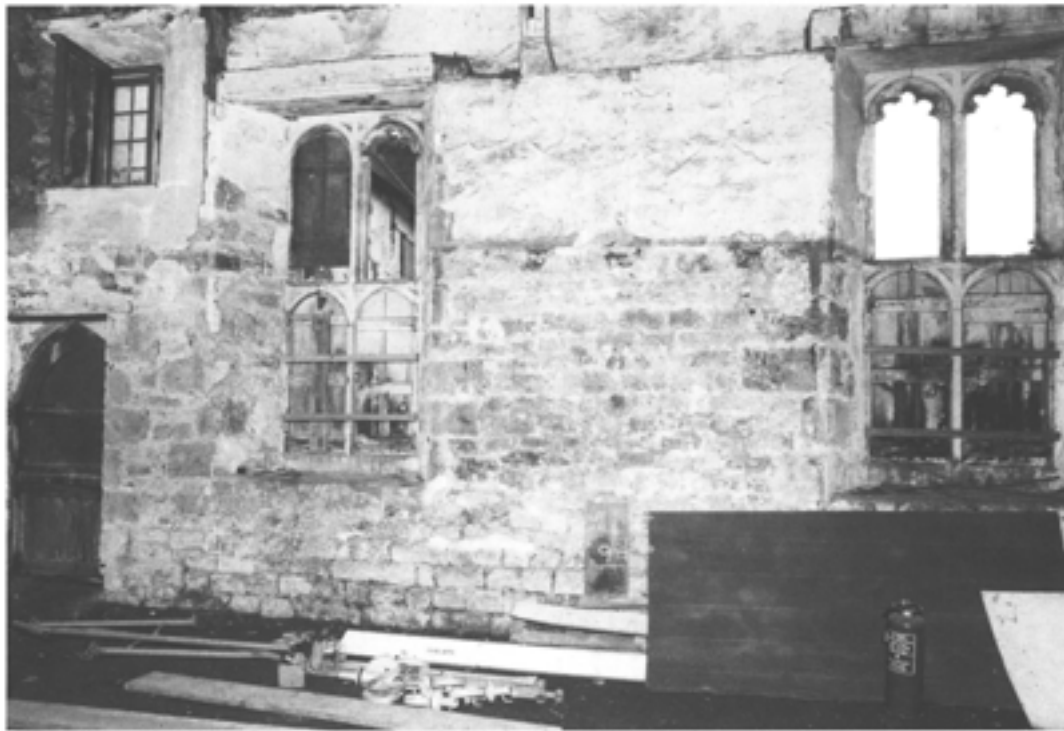
Figure 6.8 (below) Composite interior elevation of the east wall top of the hall prior to the removal of the roof for repair. These are important record photographs, since there is no other record of the cob (and stone patching) of the wall top, apparently butting the roof trusses (a northern half, trusses II–IV and b southern half, trusses IV–VI) (DoE J263/18/78 and J263/17/78).
