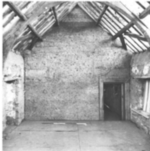
Figure 11.15 (top, left) The east elevation of the reconstructed stone cross wall in the south range in 1993 before plastering (photograph by David Garner, July 1993; EH B933548).
