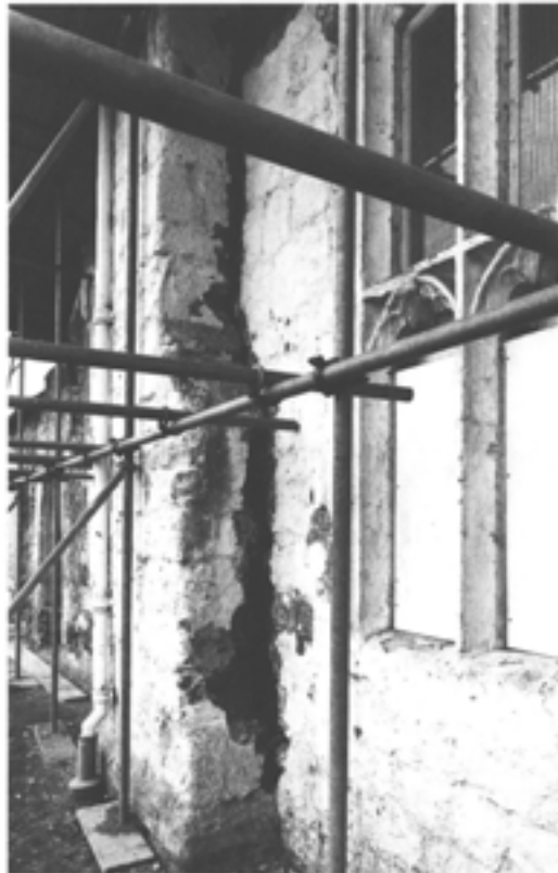
Figure 5.7 Detail of the hall chimney stack, showing the straight joint with the hall fabric, January 1981 (DoE J11/2/81).
