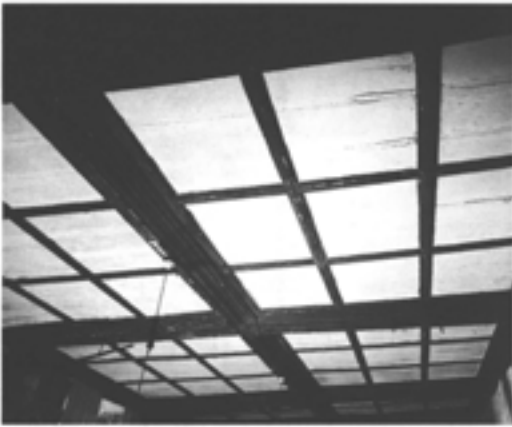
Figure 2.25 (above, left) Detail of the parlour ceiling in the 1950s, looking west, bays 2 (in foreground) to 4. Note the detail of the mouldings of the panels. The later shallower form is otherwise recorded only in a sketch (NMR AA 57/171).
