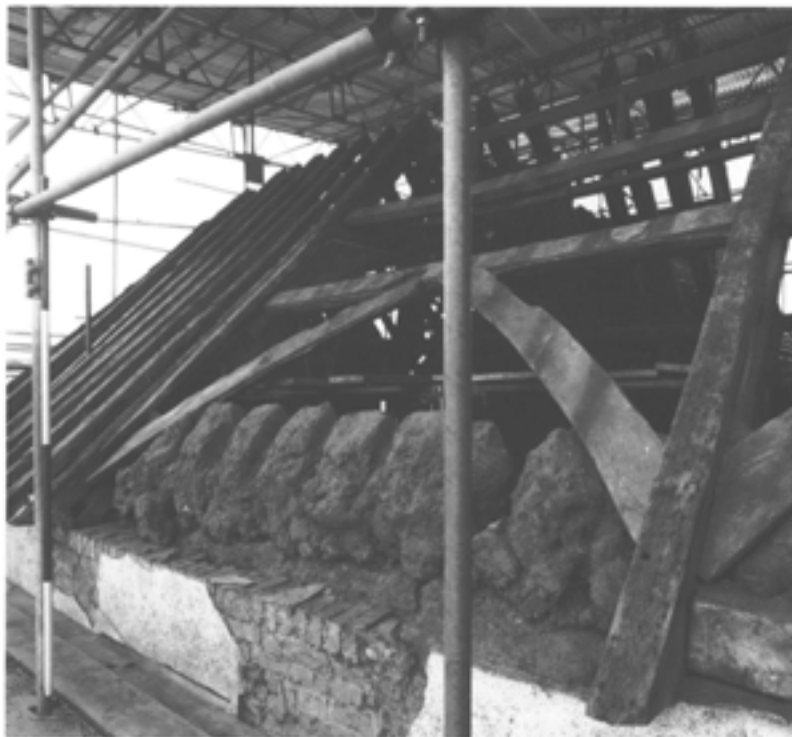
Figure 7.4 The roof of the south range, bay 9 (south), with common rafters and eaves purlin removed in June 1992. Note the cob beam filling on the wall top with impressions of the common rafters and brick fabric on the site of the oriel window (phase 8) (photograph by David Garner; EH B923942).
