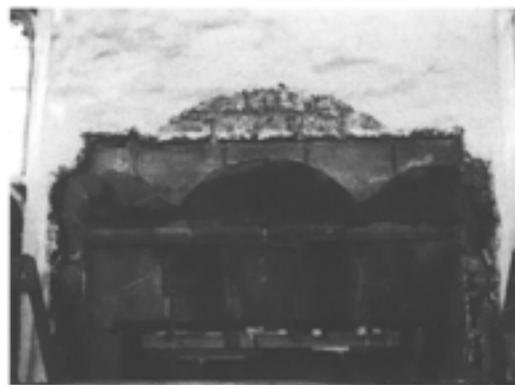
Figure 6.14 The fireplace lintel and relieving arch during recon- struction in 1989. The central voussoir and the second block of the cornice from the left are originals (photograph by Stuart Blaylock; EMAFU 1571/6).
