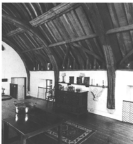
Figure 8.21 Cadhay, the hall roof: bay elevations, looking south- east (photograph taken by David Garner with kind permission of O N W William-Povelett Esq; EH B960124).
