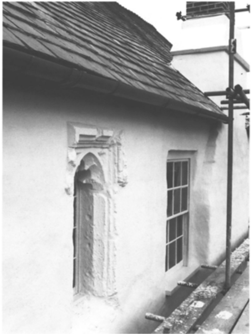
Figure 11.104 (top, left) Dubbing out of exterior stonework, south range (photograph by David Garner, April 1993; EH B931136).
