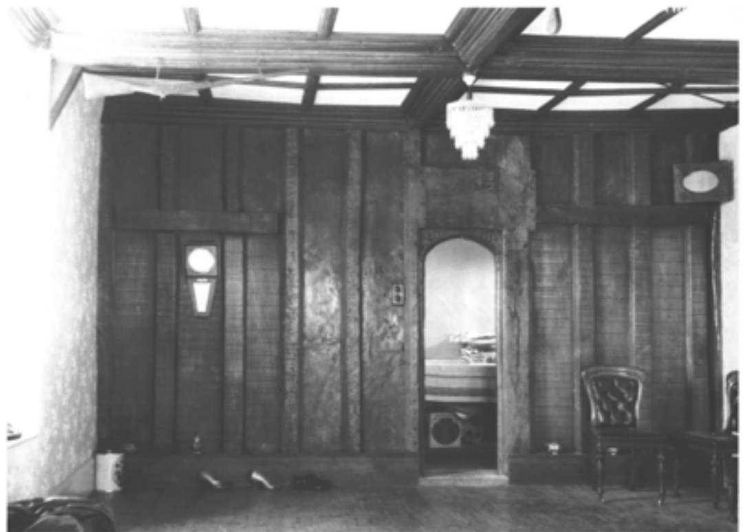
Figure 2.24 The interior of the parlour in the 1950s. Note the screen in position beneath beam 5. The head of the curved post/brace that was inserted to support the south end of beam 4 on the removal of the screen from its original site is visible on the left (photograph by A W Everett; NMR AA 69/1757).
