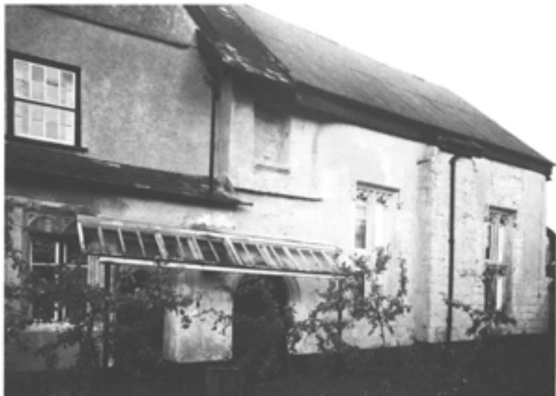
Figure 2.8 The east elevation in the 1950s. Note the corrugated roof of the hall and extent of cob walling, detectable by smooth texture beneath render (NMR AA 57/144).
