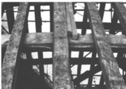
Figure 7.19 Double-pegging of face-halved tenons, truss IX, south side (photograph by Stuart Blaylock; EMAFU 1803/18).
