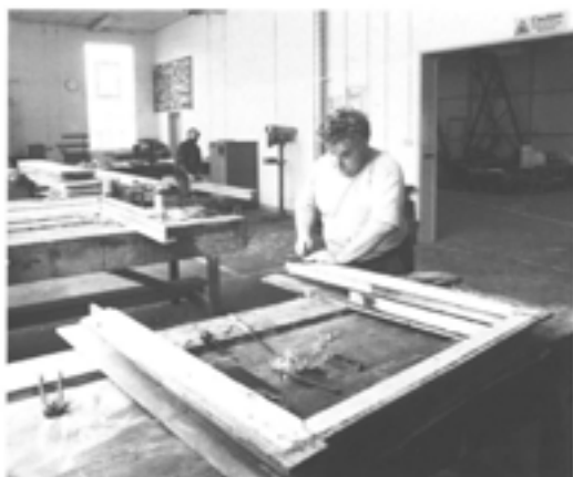
Figure 11.85 (below, right) Repairing the sill of a 19th-century box-sash window on the bench. Sills and the lower sections of boxes are the commonest points at which repair is needed (photograph by David Garner, October 1993; EH B935811).
