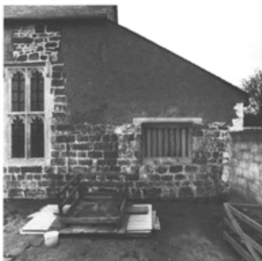
Figure 11.11 The east elevation of the completed hall store; much of the cob walling above the window lintel is new (photograph by David Garner, April 1993; EH B931122).
