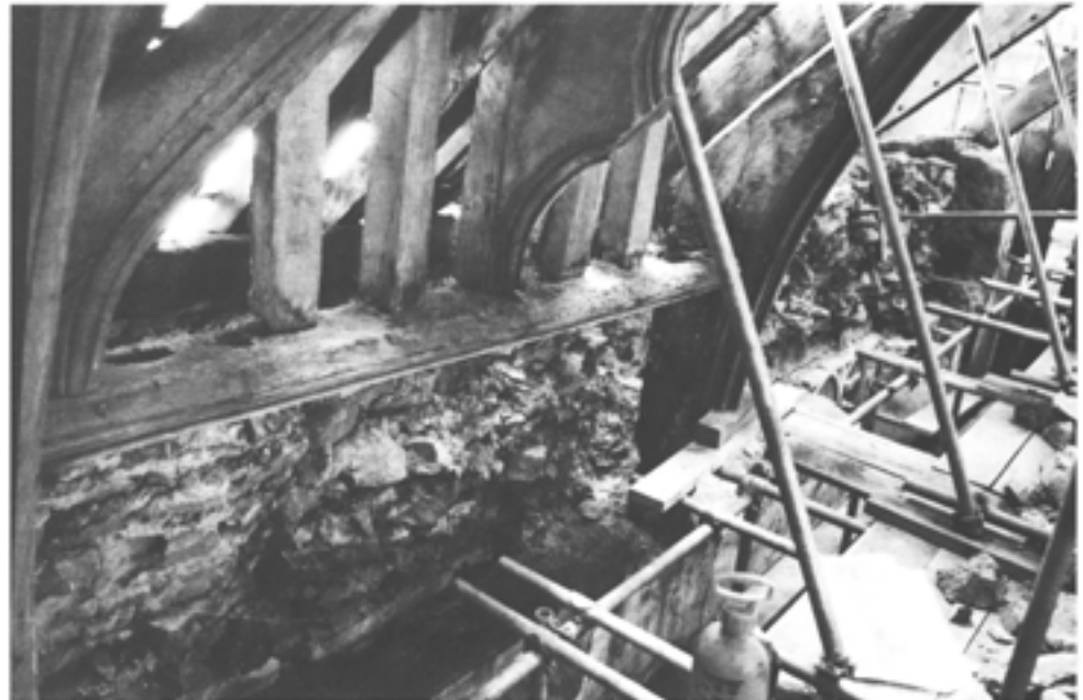
Figure 7.9 (below right) The top of the west wall of the hall, looking north. Truss IV is in the centre, truss III dismantled to the rear. Note the rubble fill of phase 8 in the outer half of the wall top, with cob wall top in the background (DoE unnumbered print).
