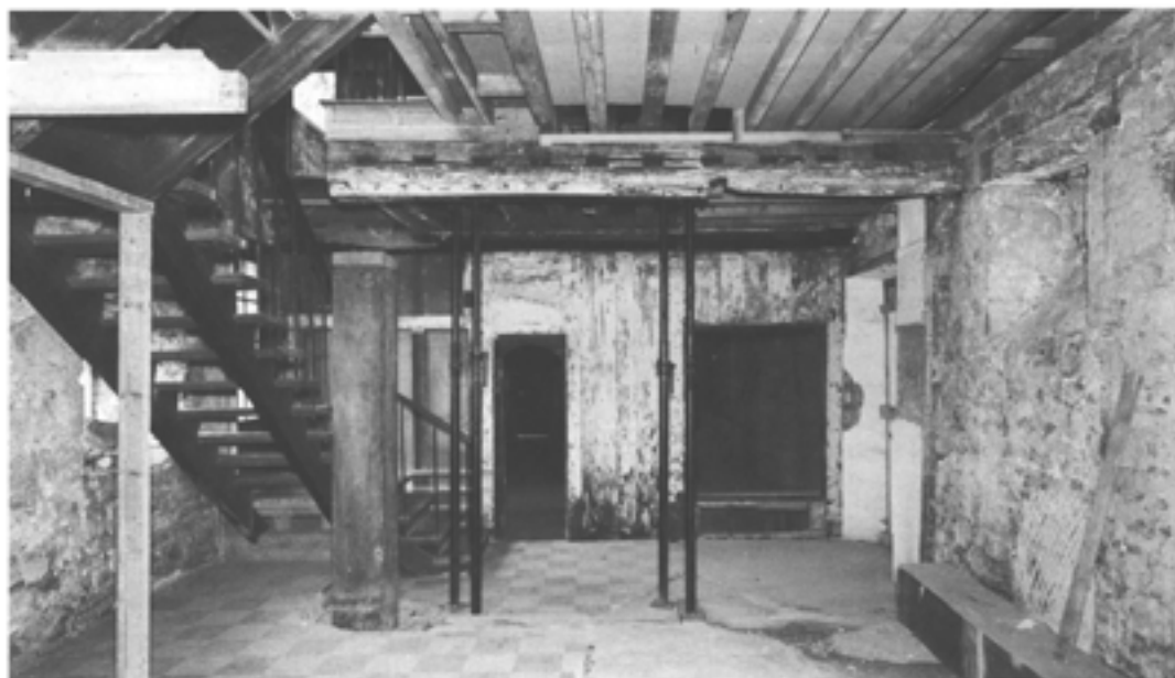
Figure 6.36 Interior of the south range, showing the service rooms after initial stripping, looking east in July 1978. Note beam 6 in the fore- ground, cut away to the north (DoE J263/6/78).
