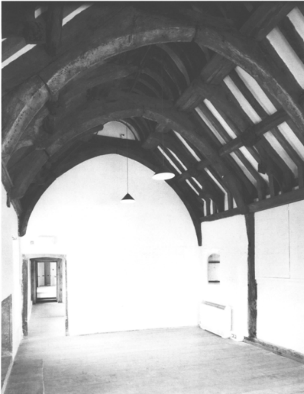
Figure 7.14 General view of the great chamber roof after repair, looking west, May 1995 (photograph by David Garner; EH A950713).
