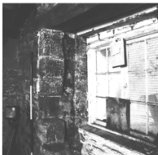
Figure 5.29 Detail of window reveal 360, looking north-east and showing the slot for the window frame (photo- graph by David Garner; EH B942026).
