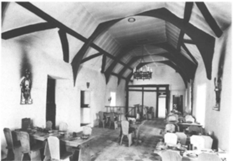
Figure 2.28 The first floor of the south range in 1969, looking east. Note the cross wall has been removed. (RCHME BB69/5038).
