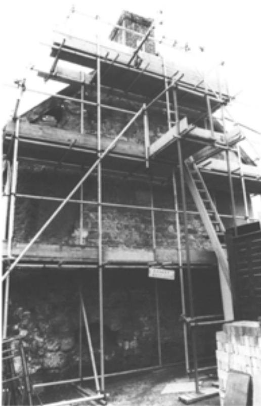
Figure 5.26 The north elevation of the west range stripped and undergoing repairs in 1981 (DoE unnumbered print; EH B960397).
