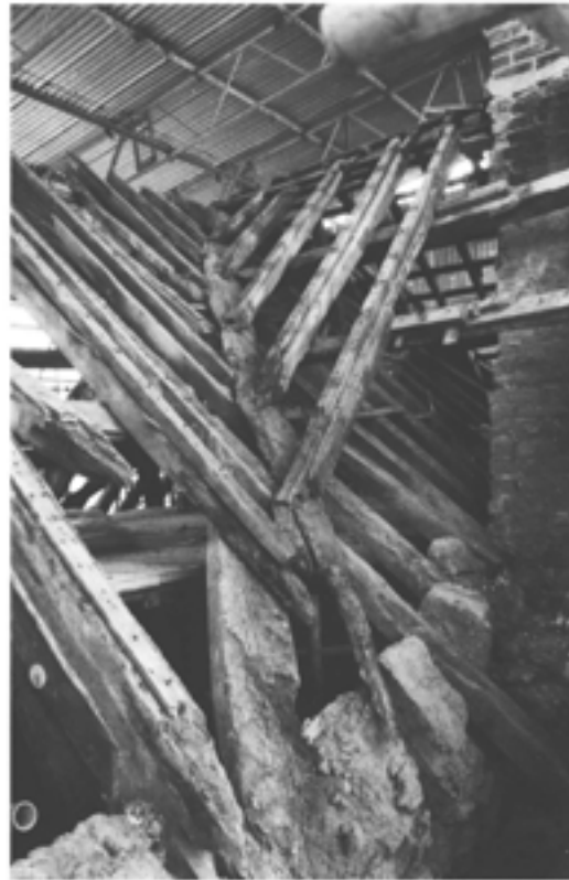
Figure 7.45 Junction of the roofs of the south and west ranges, showing the original lay board and jack rafters, east side, looking south-west (EMAFU 1987/04).
