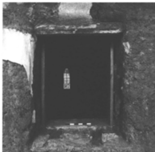
Figure 5.21 As Figure 5.20, with the frame removed, August 1993 (photograph by David Garner; EH B934815).
