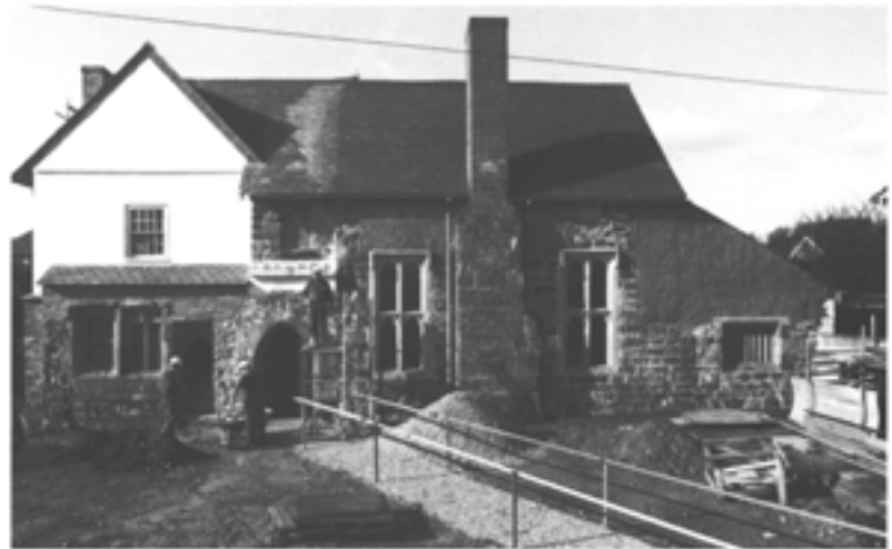
Figure 5.2 (below) General view of the east elevation when stripped for re-rendering in May 1993 (the earliest available general shot) and thus after repairs in masonry and cob (photograph by David Garner; EH B930369).
