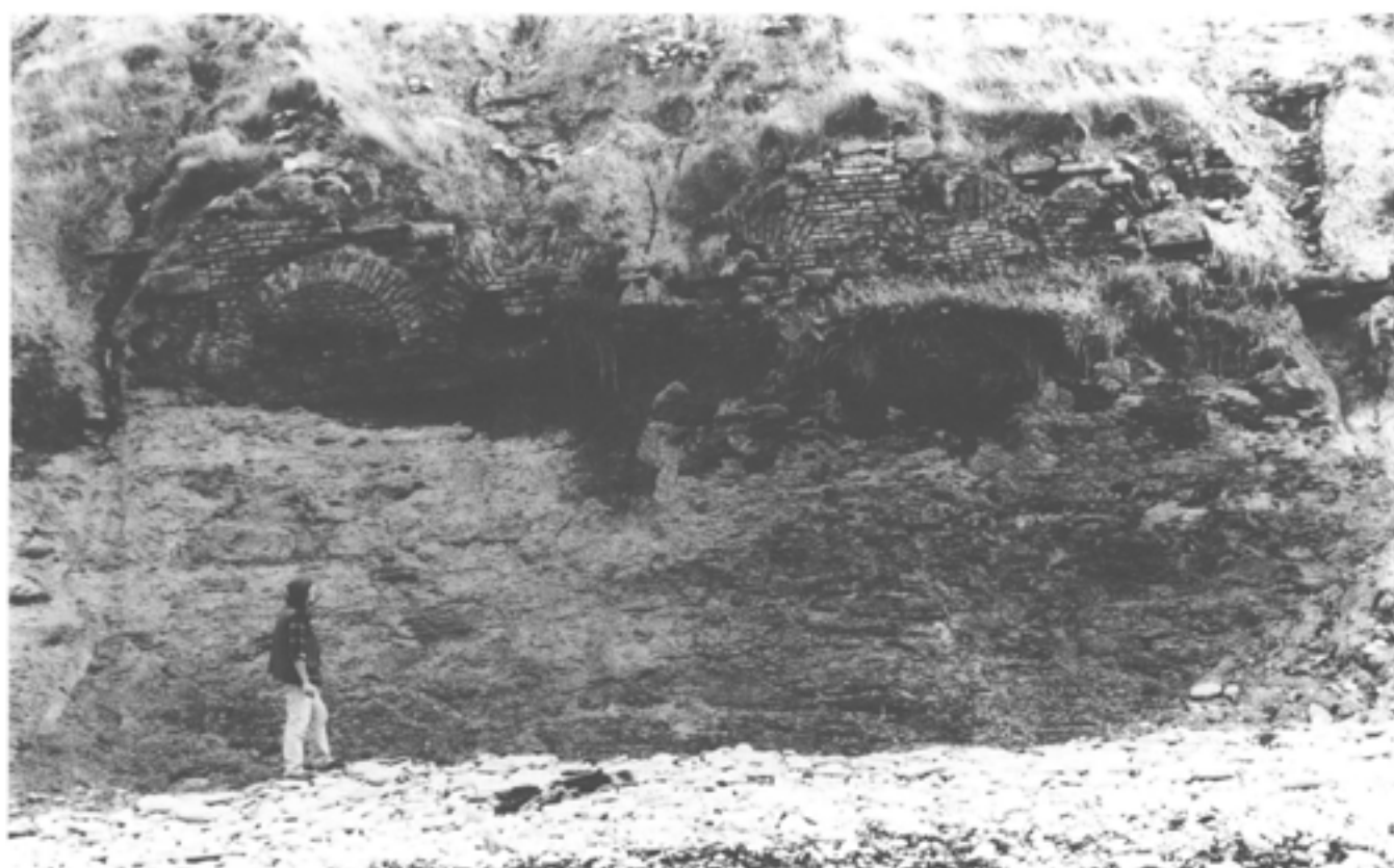
Fig 39 The alum industry at Hummersea Banks, Yorkshire; remains of brick-fronted furnaces suspected to be a range of boiling pans belonging to the alum house (The National Trust)
