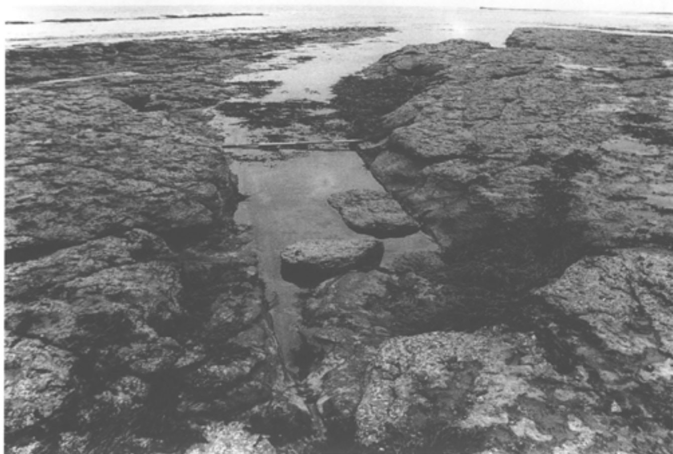
Fig 87 Ravenscar alum works, Yorkshire: rutway (1.2m gauge) used for guiding carts to the mid-nineteenth-century dock below the alum house (The National Trust)
