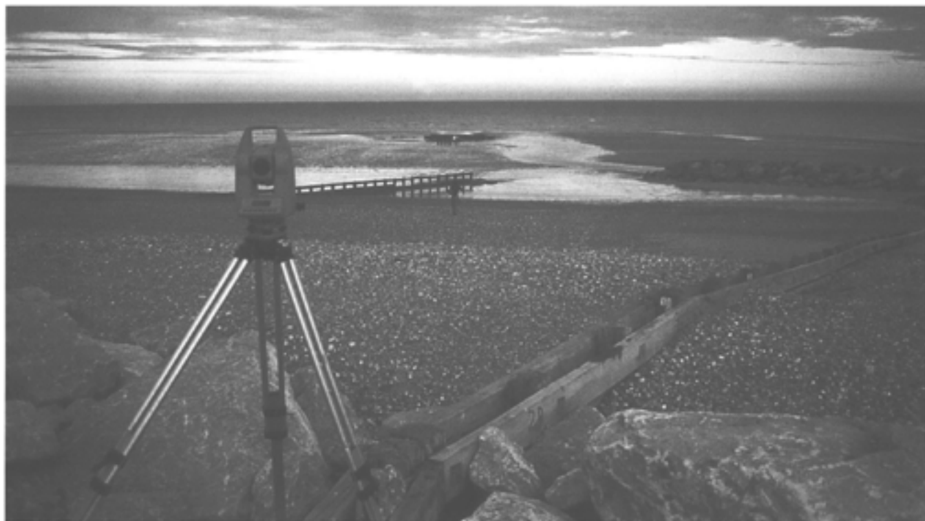
Fig 121 Hastings, East Sussex: engineering solutions to coastal erosion; to supplement earlier wooden groynes, more recent constructions include a boulder barrier at the top of the beach (foreground) and a low-shore barrier (middle right); the coffer dam surrounding the Amsterdam can also be seen (centre) (Photo Jonathan Adams)
