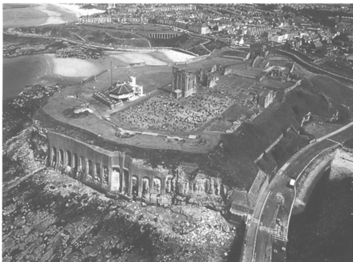
Fig 119 Tynemouth Priory, Tyne and Wear: coastal erosion has necessitated the construction of massive defences to protect the monument
