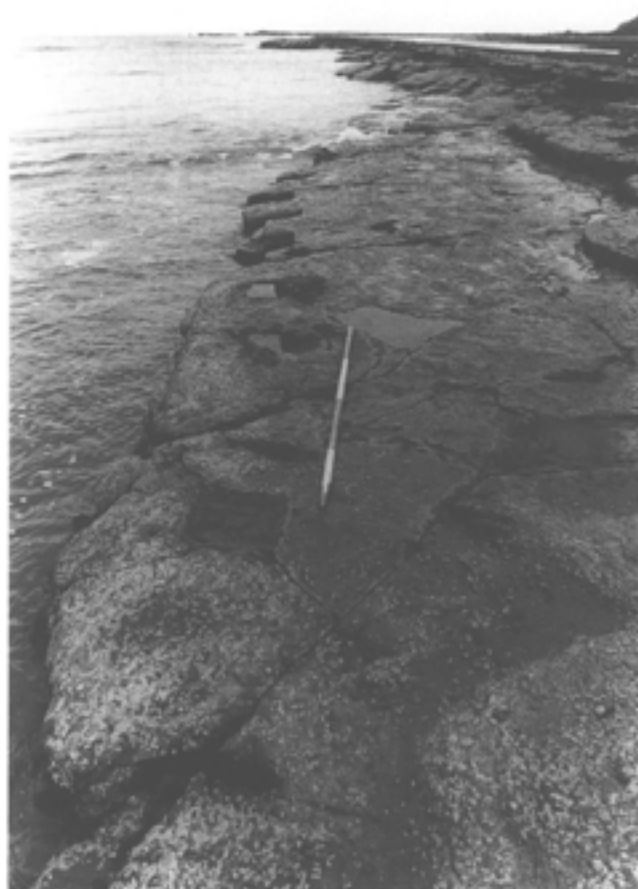
Fig 78 Ravenscar, Yorkshire: presumed sockets (0.45 x 0.45m) for mooring posts of the seventeenth-century dock (The National Trust)
