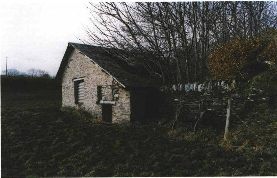
Figure 5.43 The T-bob house at Newland quarry housed the mechanism that hauled the tubs full of limestone out of the deep quarry pit, just behind the stone wall. The winch in the fore- ground was used for this purpose before the T-bob machinery was installed. (AA00/0362)
