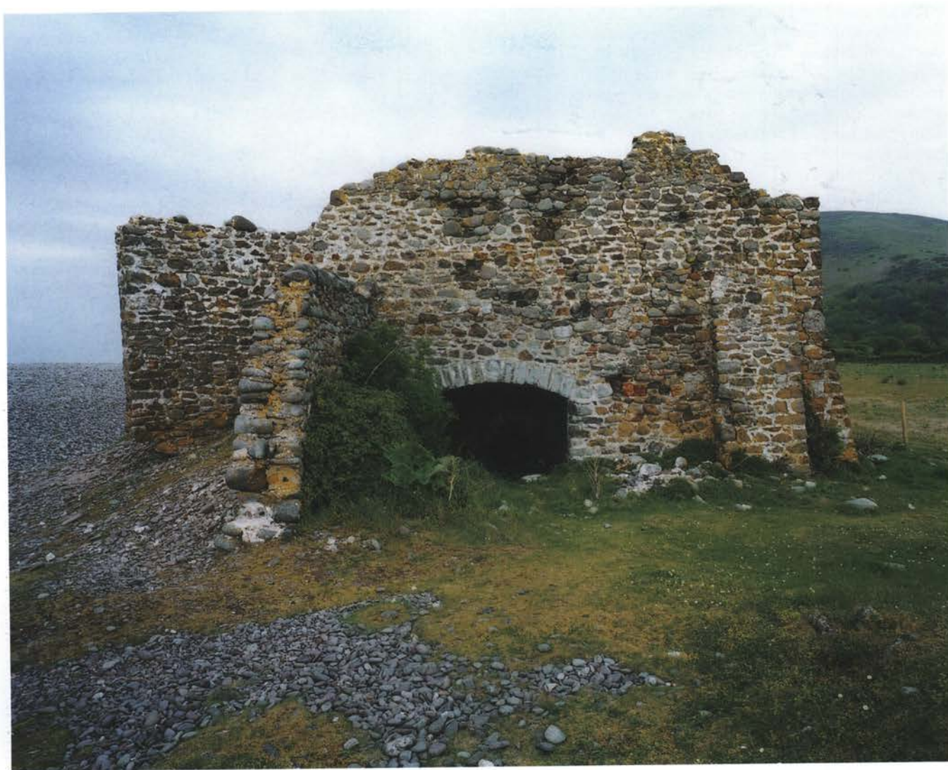
Figure 5.37 The limekiln on Bossington beach received loads of culm and limestone from south Wales. Large cobbles from the foreshore were used in its construction. (AA96/3745) (© Crown copyright.NMR)
