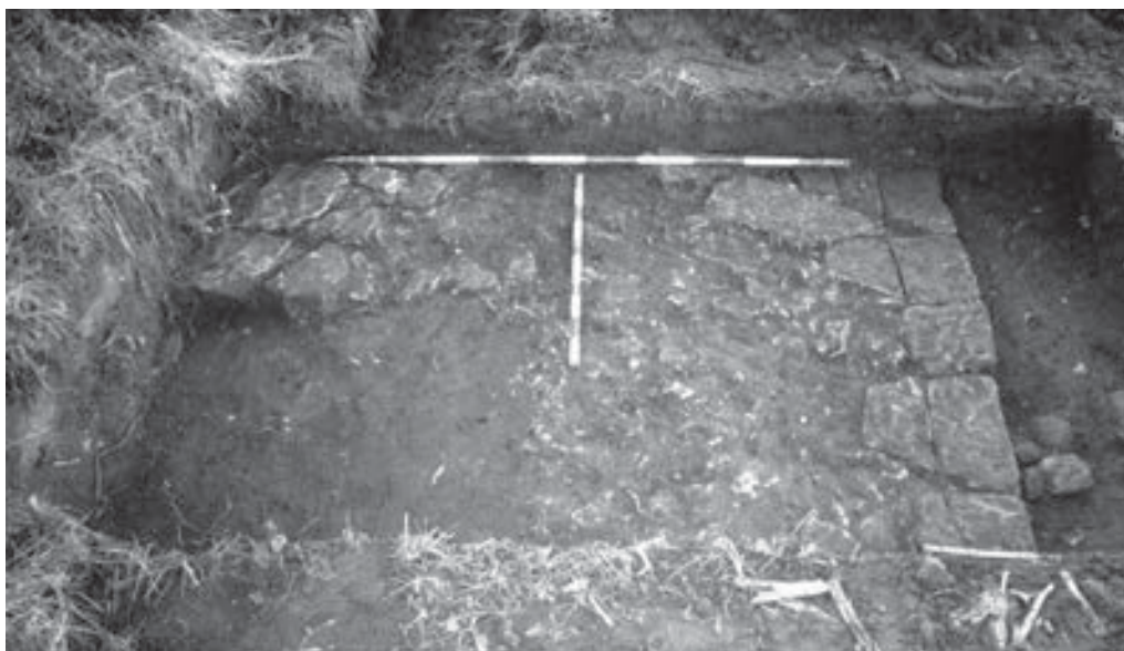
Fig 276 Milecastle 63: flagstone foundation course of Hadrian's Wall in trench. Note the linear crack marking the offset of the north wall face with the flag foundation course.
