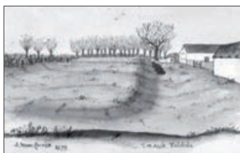
19 S.W. Angle: Vindobala. 1879 (Fig 27) The outline of Rudchester ( Vindobala ) fort Ditch is clearly indicated, including a pool of standing water. Adjacent to the south edge of the Ditch are some of the buildings of Rudchester Farm. A line of trees is shown at the east end of the site and a hedgerow, including several trees, is depicted in an east–west direction, bisecting the southern half of the fort.
