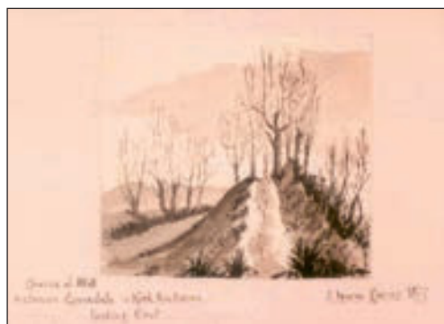
146 Course of Wall between Grinsdale & Kirk Andrews, looking East. 1877 (Fig 153) The depiction is of Long Bank between Ladylands Lane and Kirkandrews. The earth-covered mound of the Wall has a hedgerow growing on top as well as a group of mature trees. A footpath is on the berm with the ground sloping away to the north Ditch.
