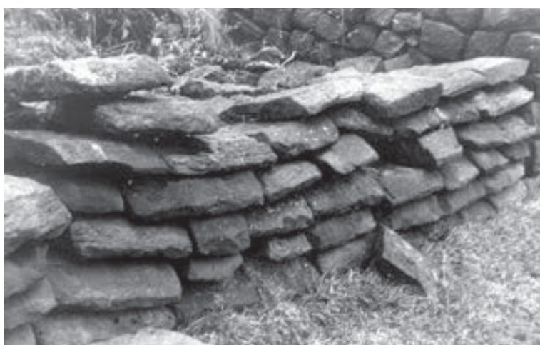
Fig 180 Consolidation on the north face of the Wall at Thorny Doors, where the original Wall face was 10ft (3.05m) high.
