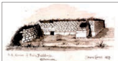
78 N.E. Corner of Public Buildings, Cilurnum. 1877 (Fig 86) The drawing is of the north-east corner of the Commanding Officer's House showing the moulded plinth, the buttress and the curve of the apse end of the bathhouse. The east wall has an outlet at plinth course level. The walls survive up to eight courses above the plinth.
