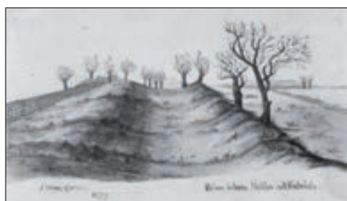
18 Vallum between Heddon and Vindobala. 1879 (Fig 26) The view, looking east, shows the slope of the Vallum Ditch and its two mounds. A stone boundary wall north of the Vallum, probably containing re-used Roman stone, is situated on the south side of the Military road. The depiction is in Wall-mile 12, probably close to T12b.
