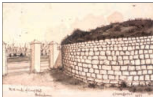
139 N.W. angle of Camp Wall. Amboglanna . 1877 (Fig 146) The angle tower wall was exposed in 1831 by the proprietor Thomas Crawhall (Hodgson 1840, 207). The drawing shows the turf-topped north-west angle of the fort wall standing ten courses above two foundation courses. A two-part gate is erected on the line of the Wall. The three large gate pillars are each topped with a chamfered capstone. The pedestrian entrance, on the east side, has a six-bar gate and the carriage entrance a five-bar gate. A line of bushes grows on the north side of the road outside the fort. Bruce (1863, 177) depicts the gateway with a section of Wall joining on to the angle of the fort but comments that this portion of the Wall had recently been removed to allow for a new entrance to the house.
