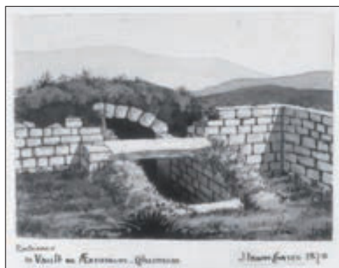
51 Entrance to Vault in Æeararium ~ Cilurnum. 1879 (Fig 59)
