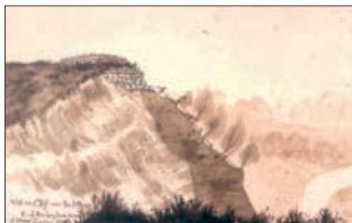
132 Wall on Cliff over the Irthing E. of Amboglanna. 1879 (Fig 139) This shows the section of Wall east of Mc49 (Harrow's Scar) overlooking the steep west bank of the Irthing river. At least nine courses of facing stones are visible above two courses of foundations, the rest of the Wall having been taken away by land slips. The bare slope above the curve of the river has a wooden fence and a line of five trees. An 1848 watercolour by H B Richardson (Bidwell 1989, pl 6) shows the Wall perched on top of the river escarpment and evidence of the river undermining the Wall.
