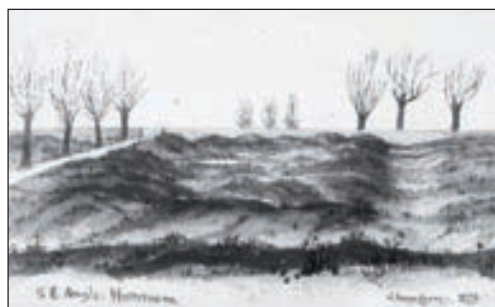
26 S.E. Angle: Hunnum. 1879 (Fig 34) The Ditch and mound of the east wall of Halton Chesters fort are discernable, as well as the tree-lined road through the middle of the fort leading from the Newcastle–Carlisle turnpike to Halton. This road presumably lies above the original Roman road within the fort. A stone(?) wall crosses the fort on the south side of the Newcastle–Carlisle turnpike road. Numerous humps and bumps in the south-east quadrant of the fort indicate the extent of buried buildings within the fort.
