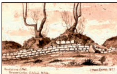
131 Foundations of Wall. Vicarage Garden. Gilsland. N. Side. 1877 (Fig 138) Up to five courses of Wall face are visible, the top of the Wall being covered in turf with two trees growing from the mound. Three cuttings have been made across the width of the Wall and in front are four small piles of Wall core. This section of Wall had been exposed not long prior to this by the vicar of Gilsland, Rev A Wright (Ferguson 1877-8, 24).
