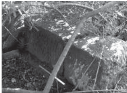
Fig 245 Milecastle 10: photograph of the north-west pier of the north gate in its present state (photograph by P Hill).
