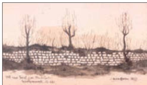
71 Wall near Turret (near Black Carts) recently uncovered – S. side. 1877 (Fig 79)
