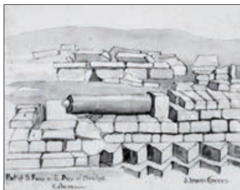
35 Part of S. Face of E. Pier of Bridge. Cilurnum . no date (Fig 43)
