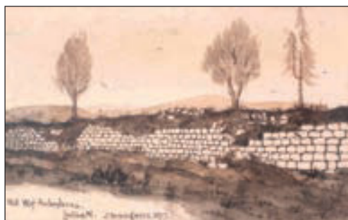
140 Wall W. of Amboglanna. Looking N. 1877 (Fig 147) The south face of the Wall west of Birdoswald stands at least seven courses high, the earth capping containing core work. Sections of the Wall face show evidence of either collapse or robbing of the stone work. Three mature trees are shown on the north side of the Wall. In the distance to the north-west is the outline of the only remaining wall of Triermain Castle, which had been built with re-used Roman Wall stone.
