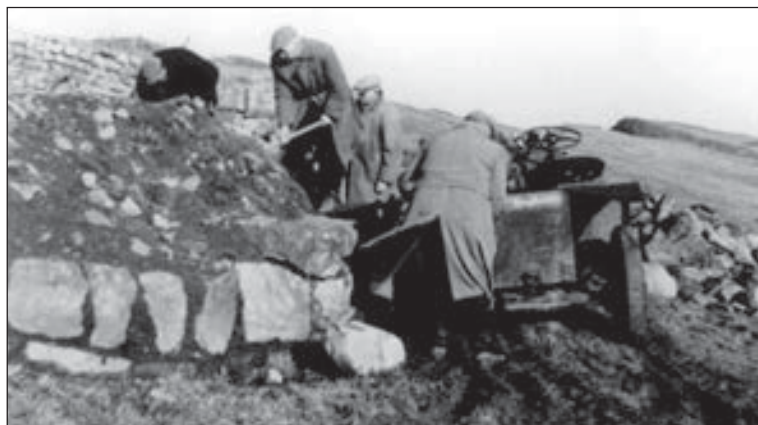
Fig 178 Consolidation team at work at Mc42, Cawfields.
