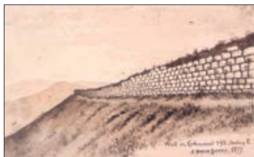
121 Wall on Cockmount Hill. (looking E.). 1877 (Fig 129)
