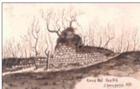
141 Core of Wall. Hare Hill . 1879 (Fig 148) This depiction, possibly of the north face, shows the original core work laid horizontally and a large amount of scrub and small bushes cover the surviving Wall. The north face of the Wall, including a centurial stone found to the west of T53a (RIB 1958) was re-built in the 19th century by Mr Marshall, the Earl of Carlisle's architect (Bruce 1933, 182).
