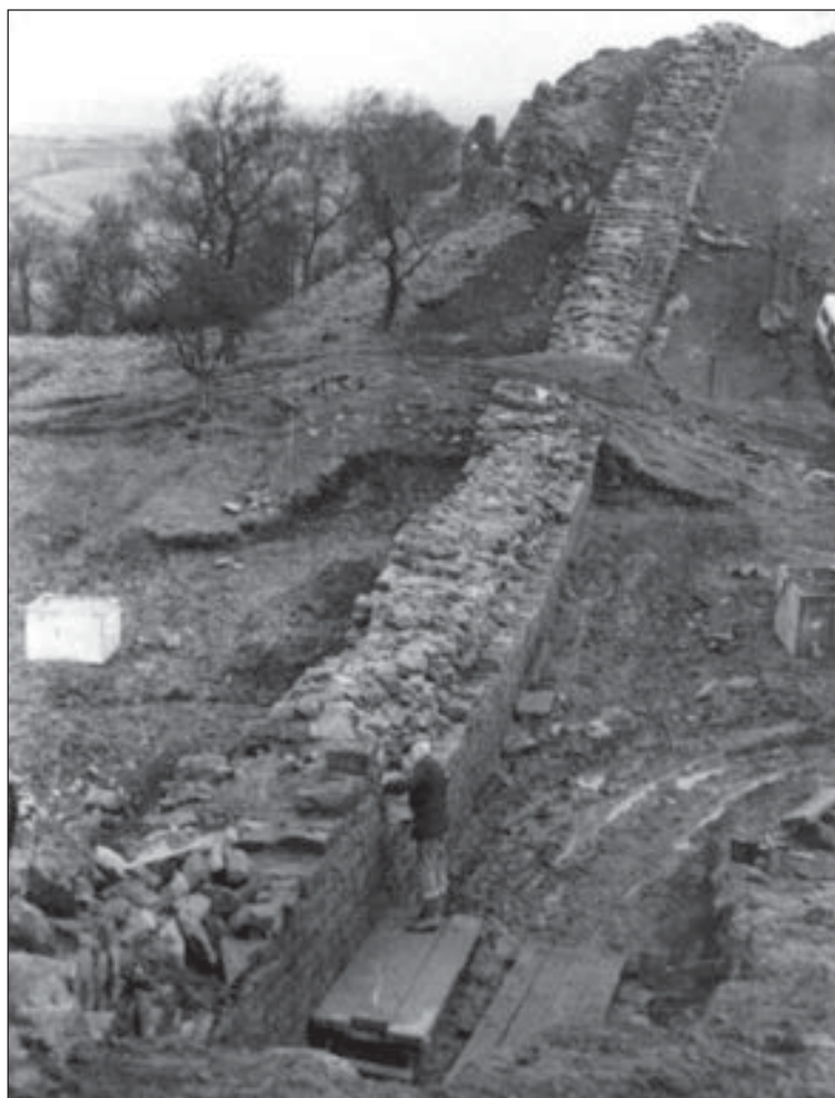
Fig 179 Consolidation on the south face of the Wall at Walltown.
