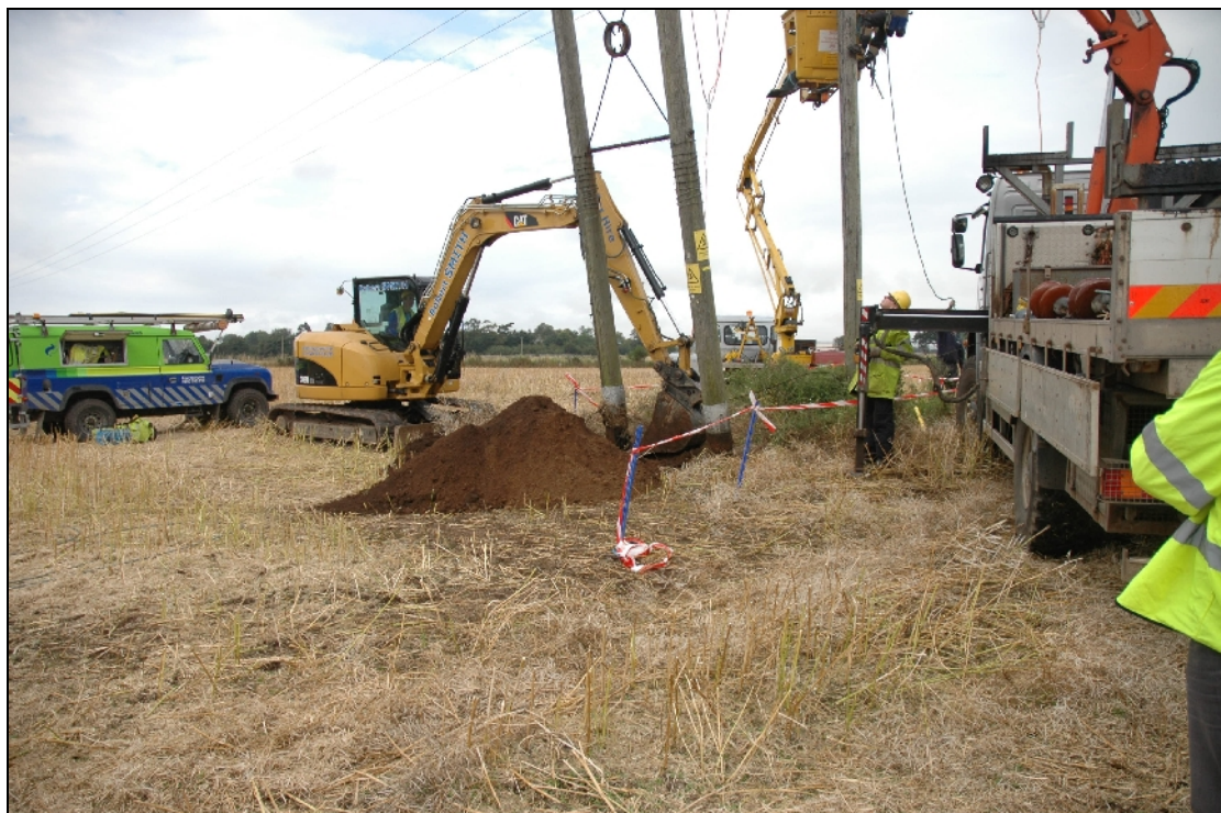
Illus. 5: Double poles during removal, looking NW.
