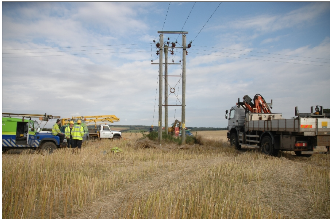
Illus. 2: General view of area prior to removal of double poles, looking N.
