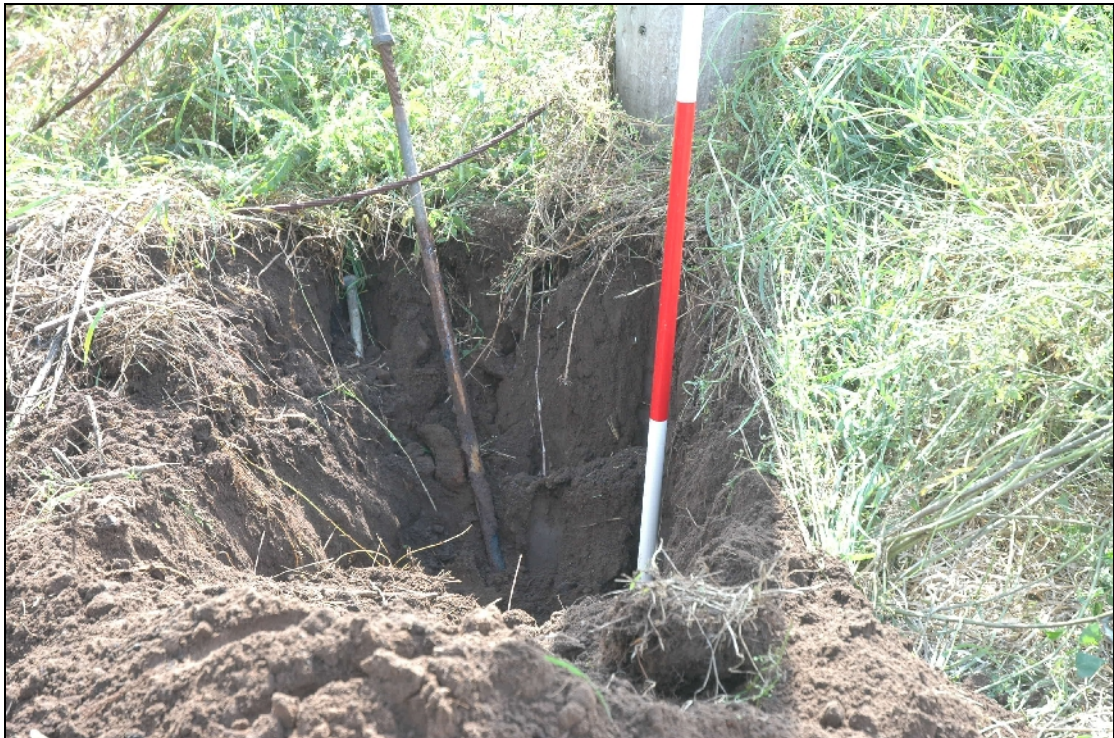
Illus. 7: Machine cut for removal old stay wires, looking SE.
