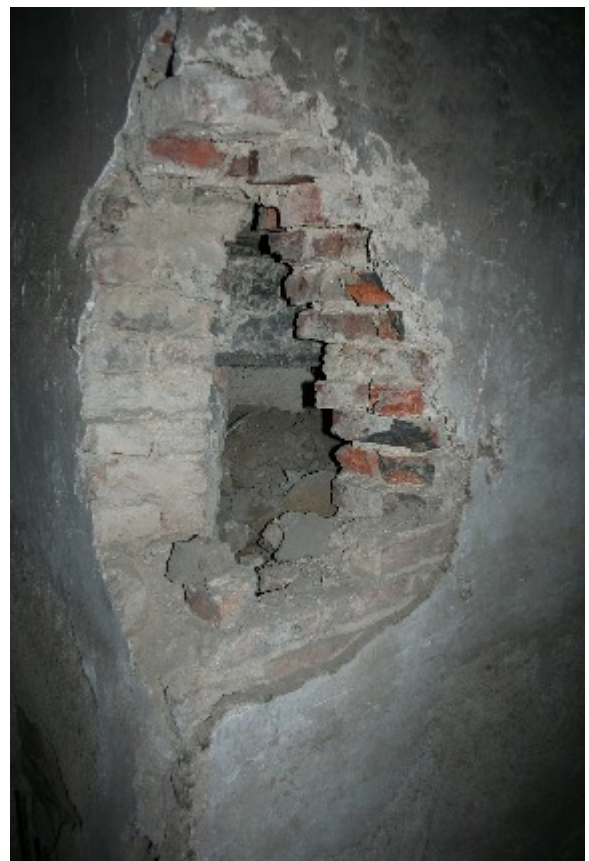
Plate 38. The blocked up fireplace (frame HHR13177)
