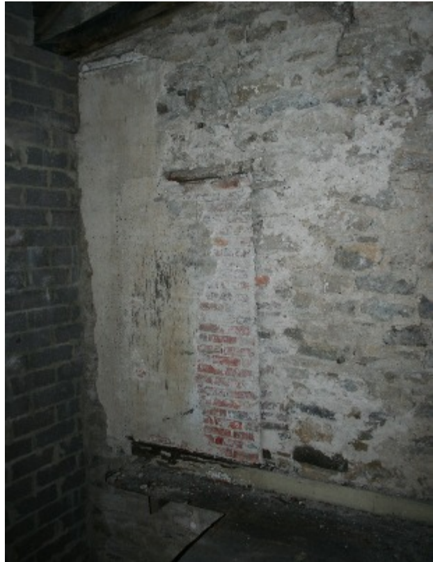
Plate 88. Blocked doorway in Area 32 leading through to Area 33 (frame HHR13393)
