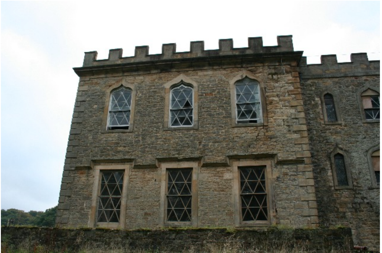
Plate 98 (above). The northern elevation, eastern wing (frame HHR13418)
