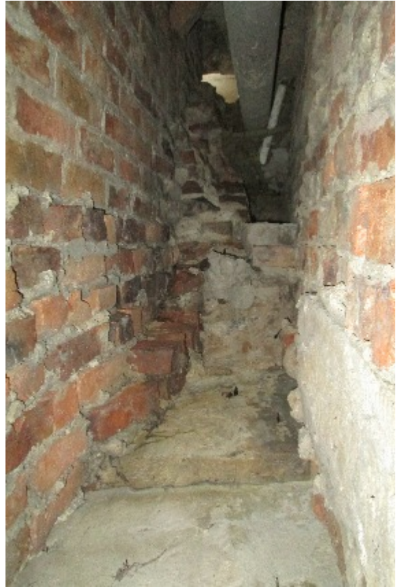
Plate 62. Internal ducting (frame HHR13277)
