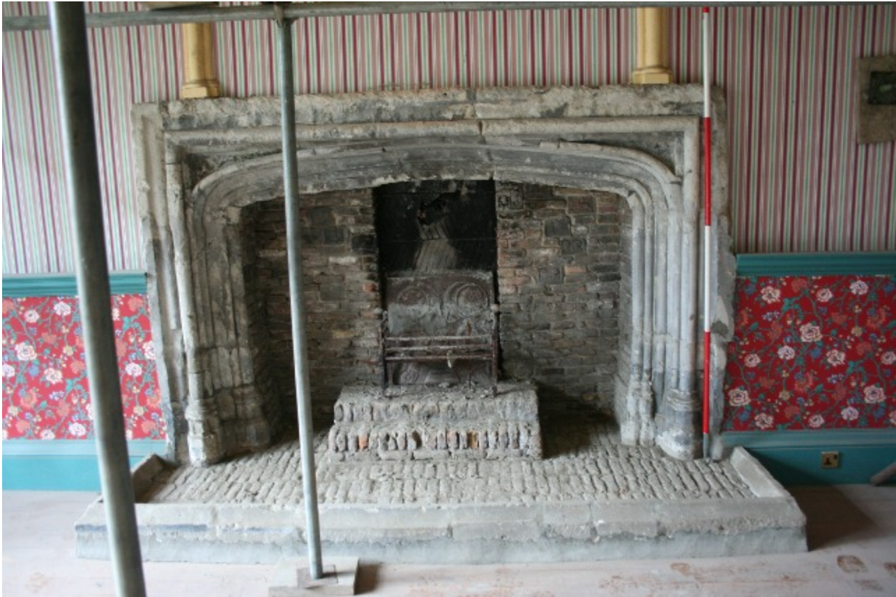
Plate 24. The Crosby Hall 15 th century fireplace (frame HHR13089)
