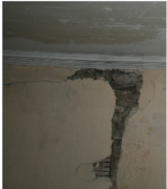
Plate 56. West wall of Area 38, showing blocked up external window (frame HHR13259)
