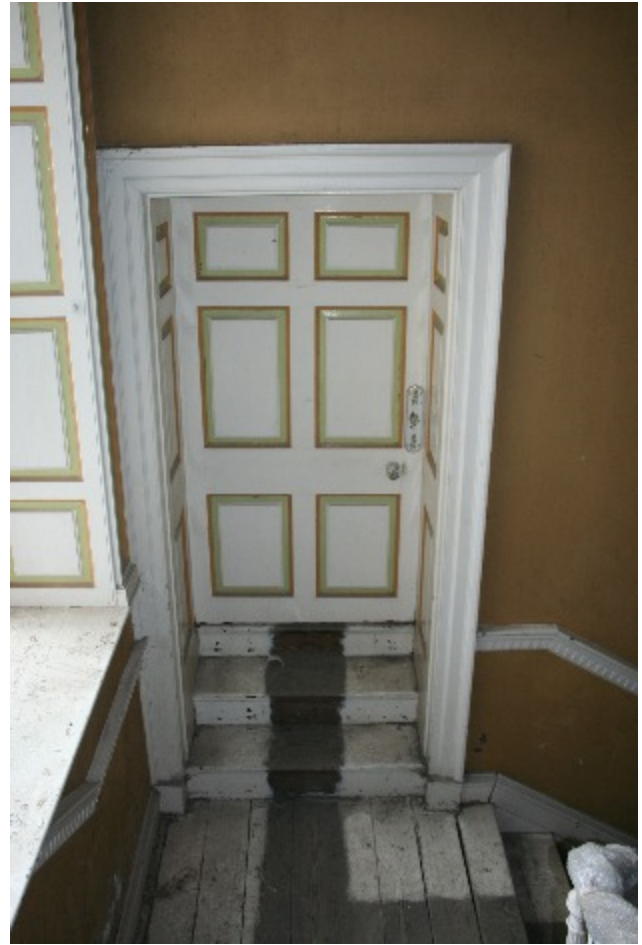
Plate 47. Door to Area 15, off the mezzanine level landing in Area 1 (frame HHR13228)
