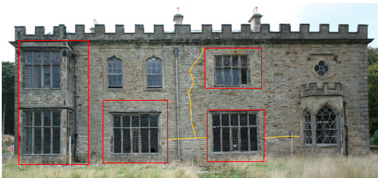
Plate 90. The eastern elevation with location of inserts from Beaudesert (red) and areas of different structural phasing (yellow) (frame HHR13405)
