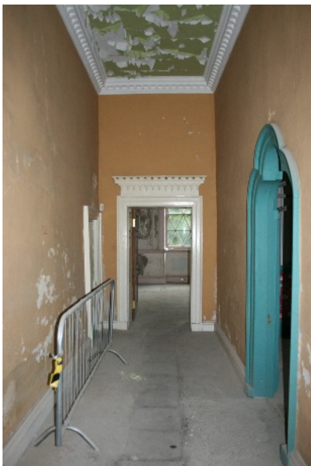
Plate 17. The corridor looking north into the Drawing Room (frame HHR13063)
