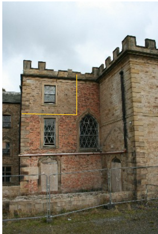
Plate 110. Later brick block, southern elevation, with phases in yellow (frame HHR13440)
