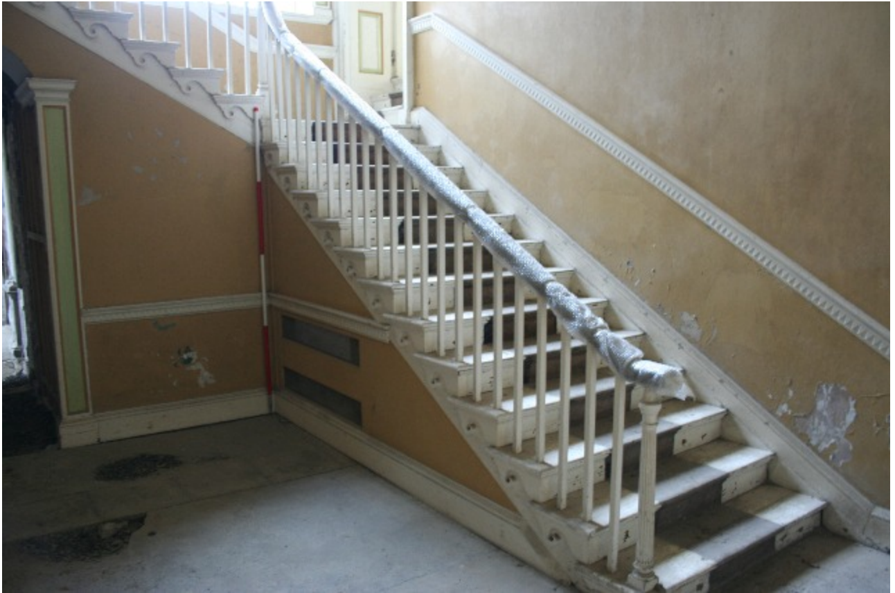
Plate 13. The stairwell, looking southwest (frame HHR13035)
