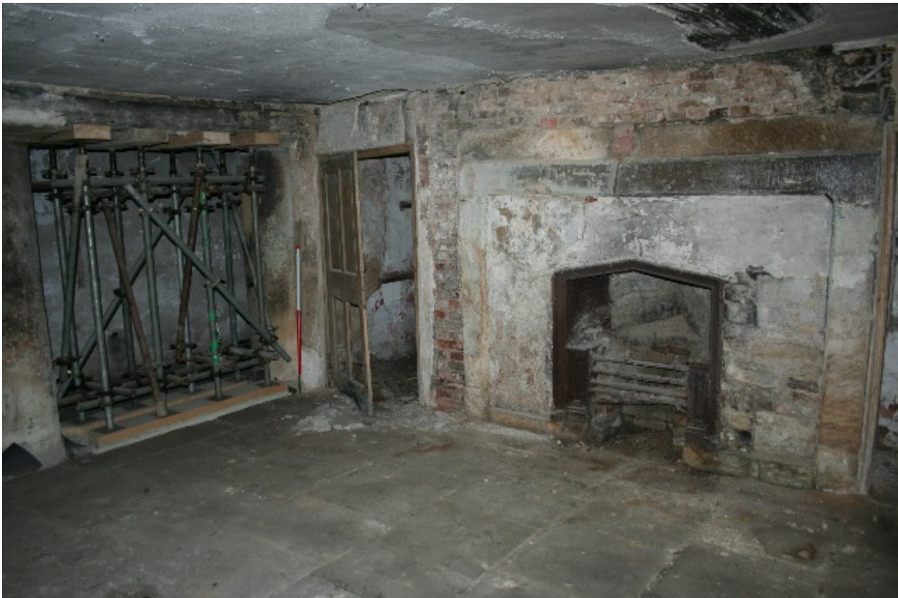
Plate 43. Area 48, looking toward the fireplace (frame HHR13192)
