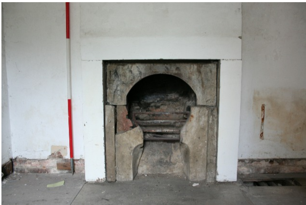
Plate 16. The fireplace in Area 20 (frame HHR13045)
