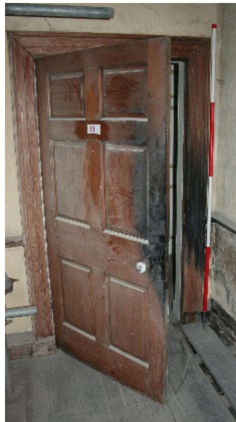
Plate 70. Fire damaged door, Area 10 (frame HHR13322)
