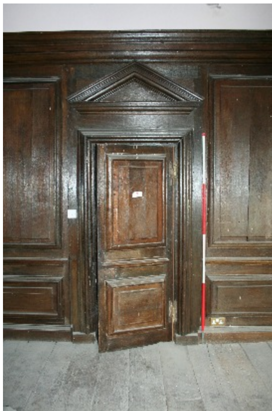
Plate 73 (above). Jacobean door leading to stairhall Area 6 (HHR13347)
