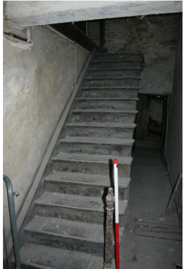
Plate 50. The stairs to the first floor (frame HHR13233)
