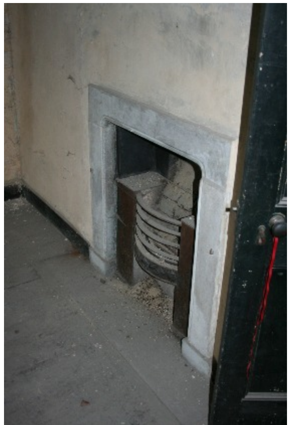
Plate 54. Hob-grate in north wall of Area 38 (frame HHR13255)
