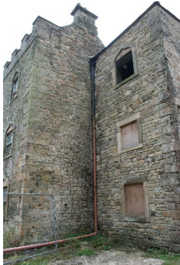
Plate 102. The rebuilt wall and western elevation of the original house (frame HHR13421)
