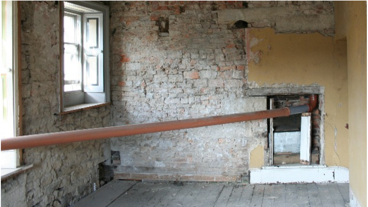
Plate 60. Area 2-5, north wall with mixed construction materials and duct (frame HHR13266)
