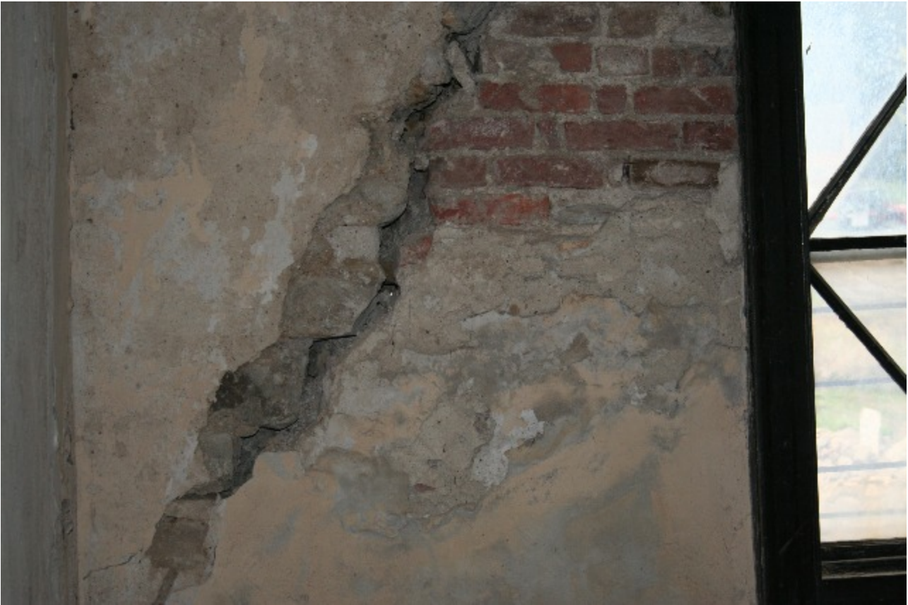
Plate 55. Area 38, crack in south external wall (frame HHR13254)
