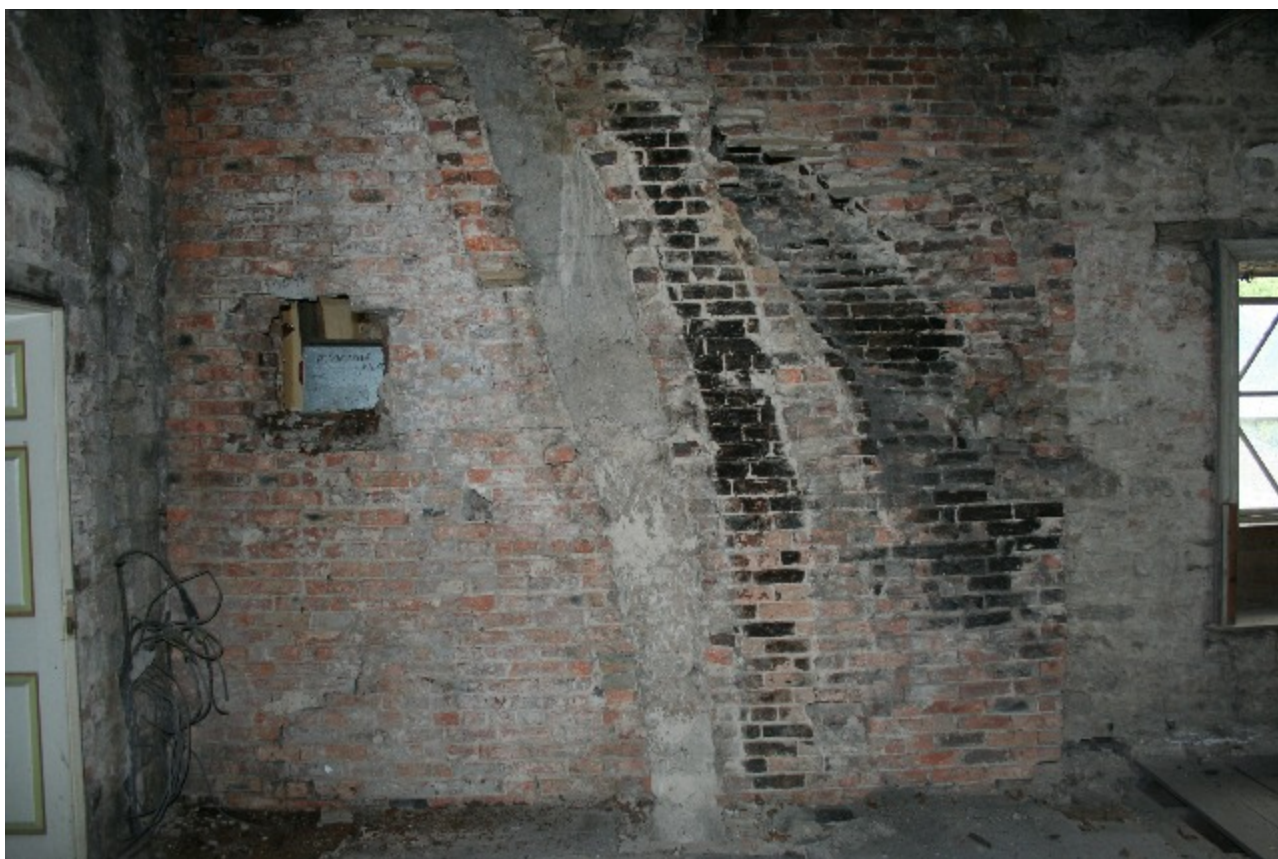
Plate 81. Brick structure in southeast corner of Area 12, view void to duct and flue staining (frame HHR13365)
