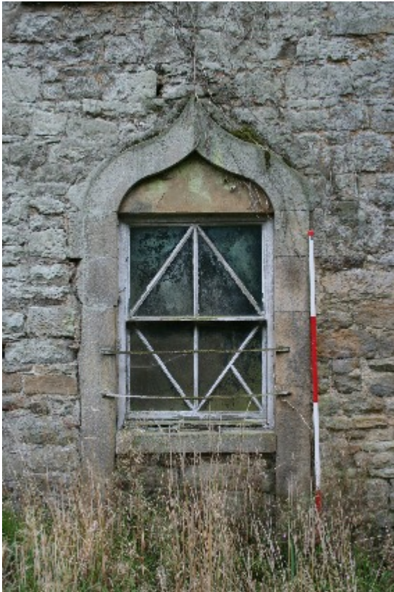
Plate 101. The original door, Door 46 (frame HHR13423)
