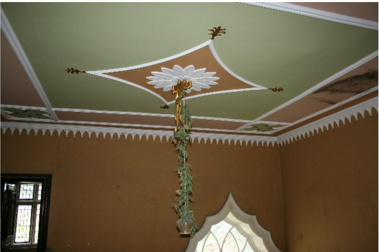
Plate 64. The Rococo Gothic ceiling and cornice (frame HHR13287)
