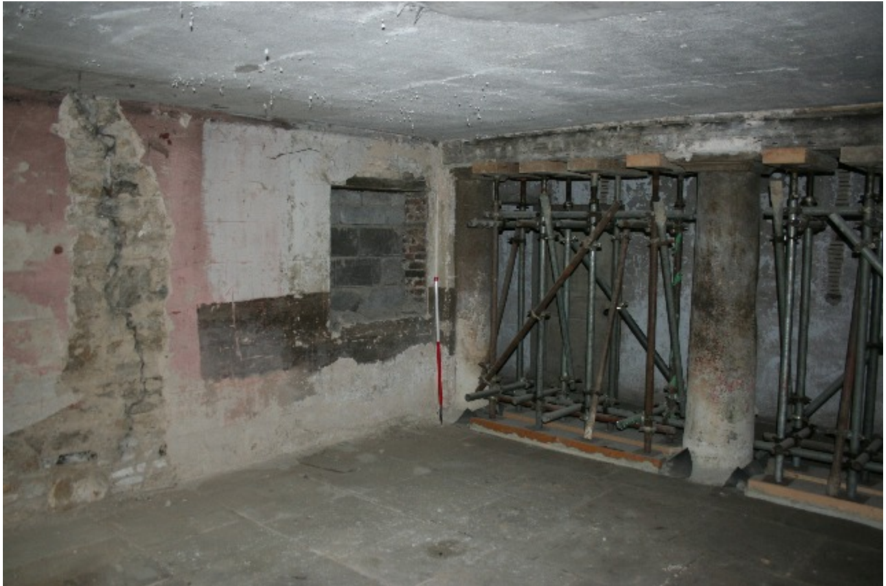
Plate 41. Area 48, looking toward the column and blocked window (frame HHR13191)
