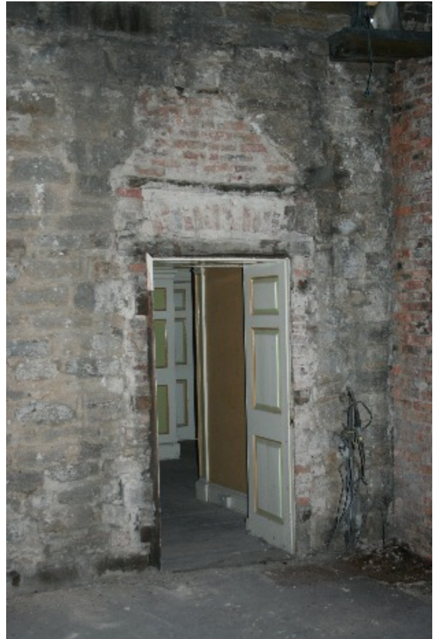
Plate 83. Doorway to Area 7, showing bricked up ogee-arched window (frame HHR13367)
