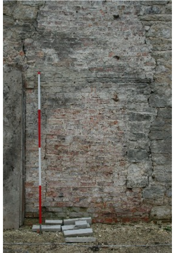
Plate 105. The blocked door (frame HHR13428)
