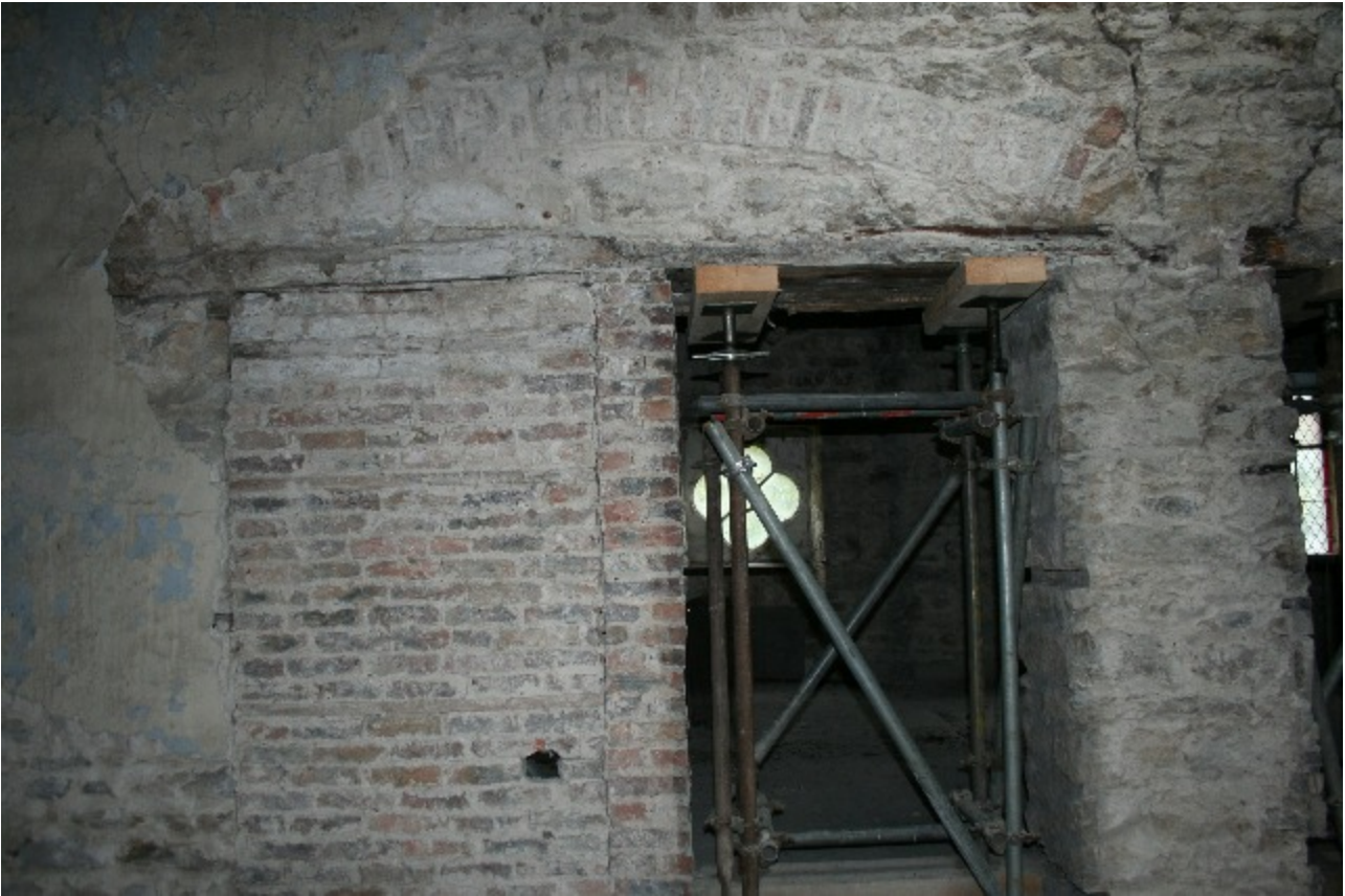
Plate 85. Blocked archway leading through to Area 33 (frame HHR13376)
