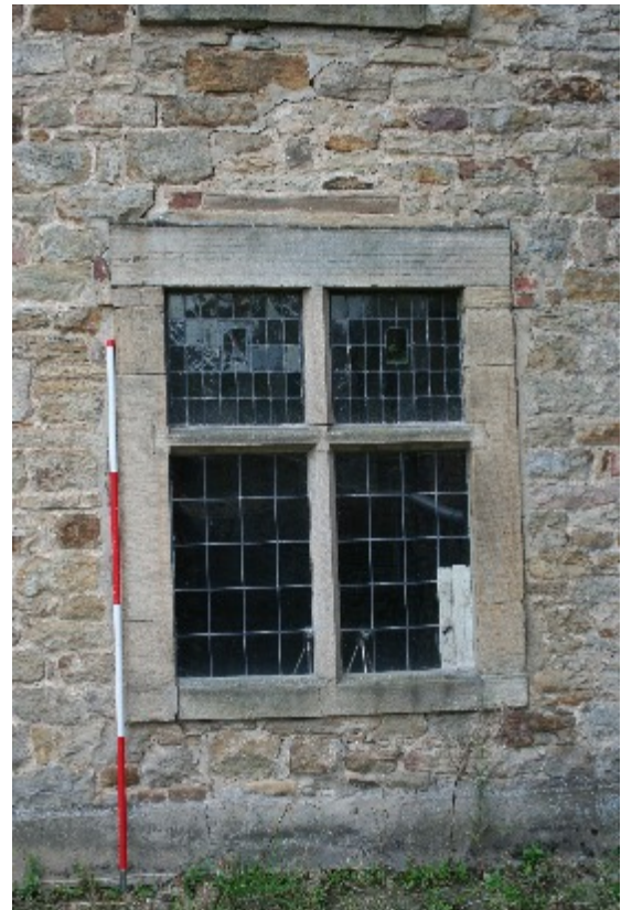
Plate 108. Detail of Window 39, showing blocked ogee-arch (frame HHR13433)
