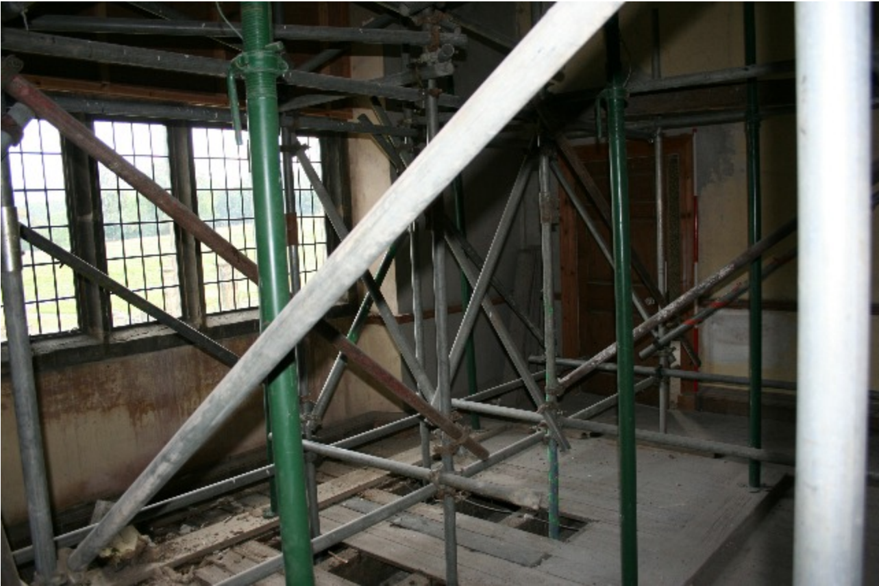
Plate 69. The ceiling in Area 10 is held up by emergency scaffolding (frame HHR13320)
