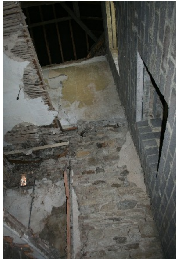
Plate 40. The damaged floors (frame HHR13187)
