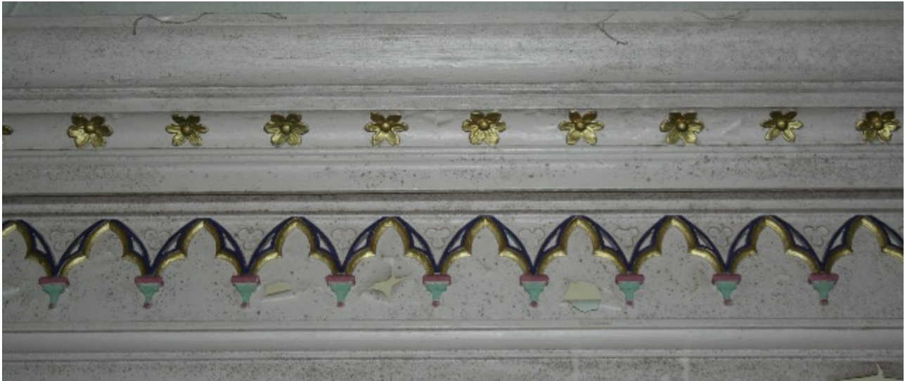
Plate 21. Detail of cornicing (frame HHR13085)
