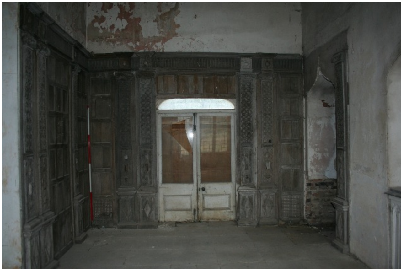
Plate 12. Room 16, looking west (frame HHR13022)
