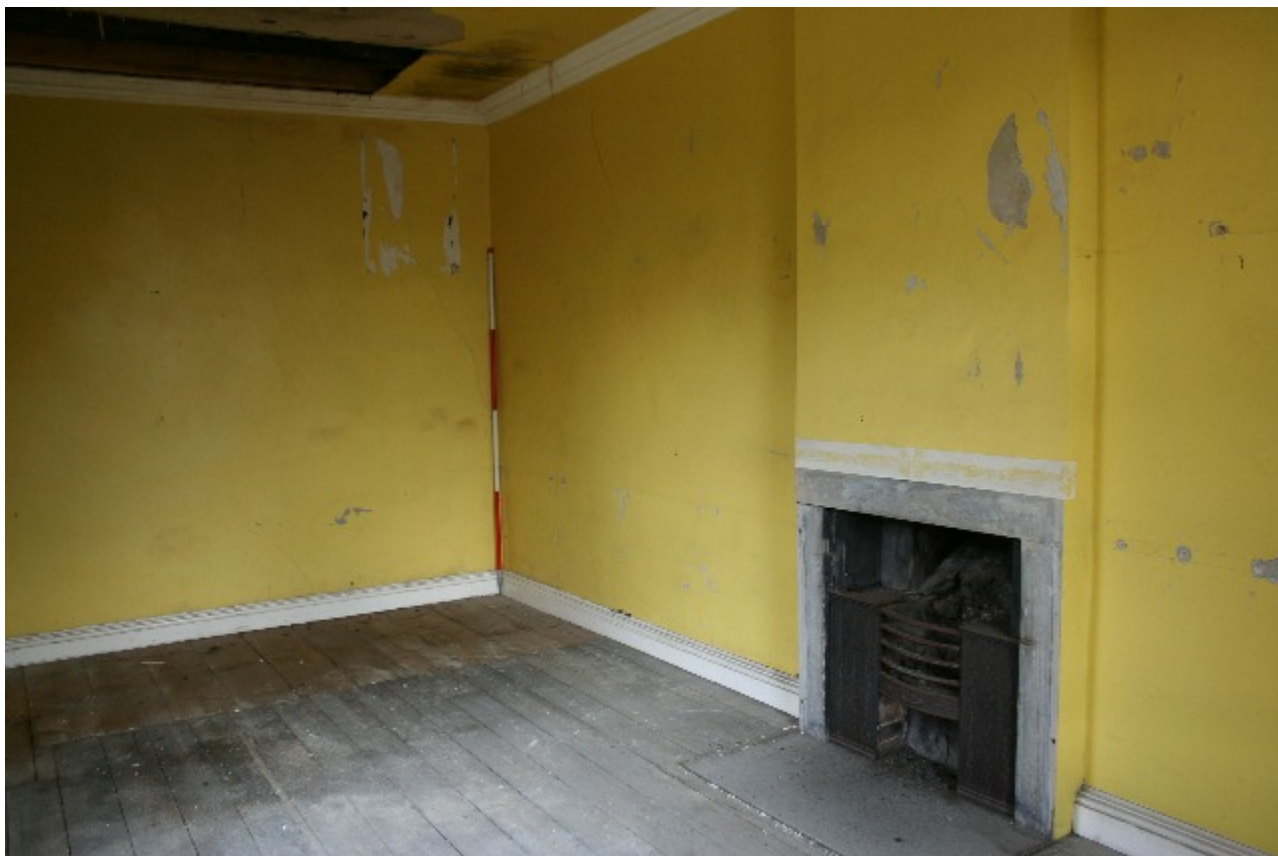
Plate 48. Area 15, looking northeast (HHR13217)
