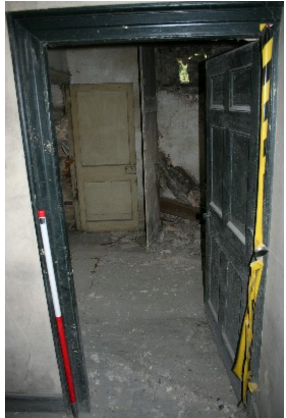
Plate 57. Doorway through to Area 39 (frame HHR13260)
