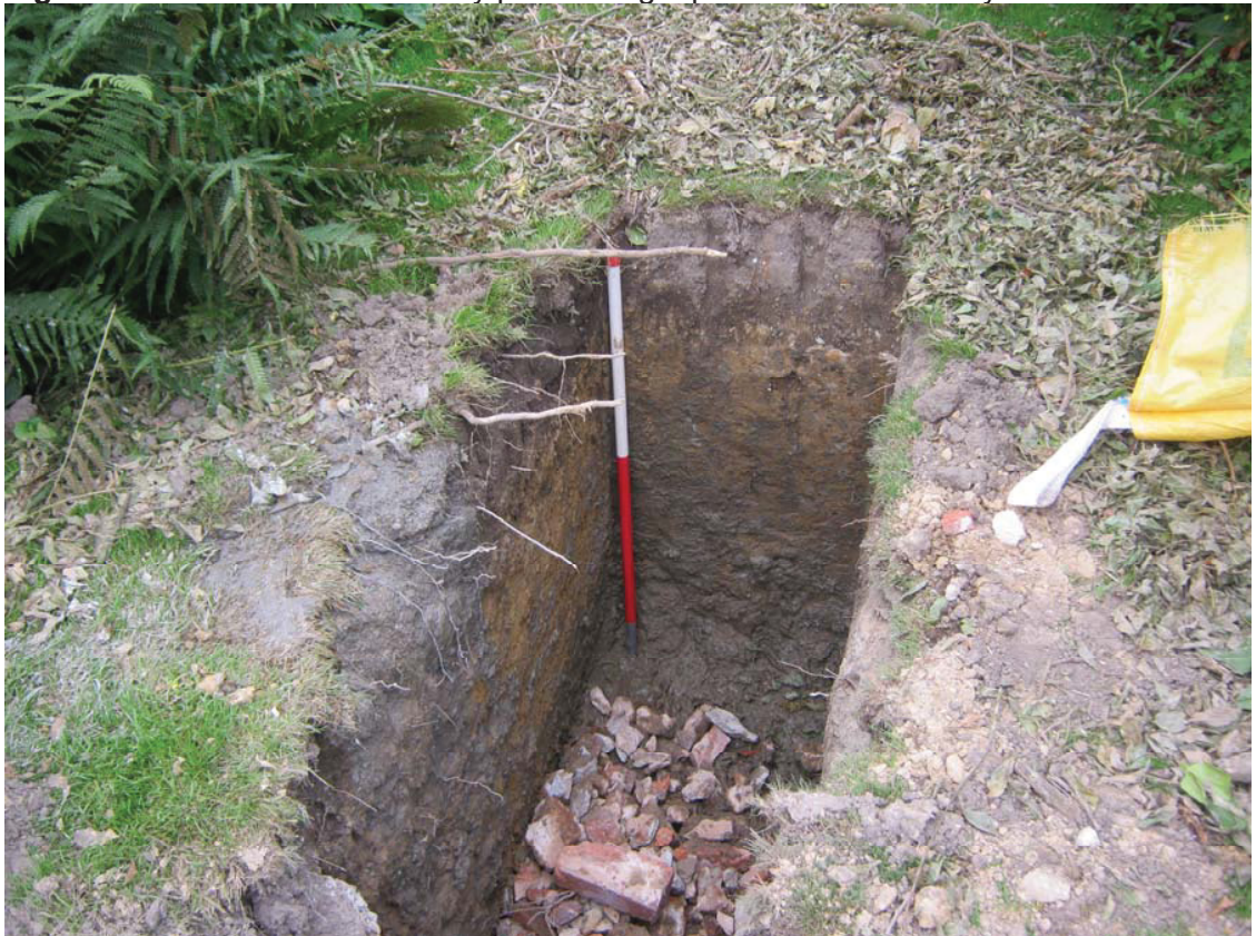
Figure 2: Excavation of soakaway pit showing topsoil over natural clay
