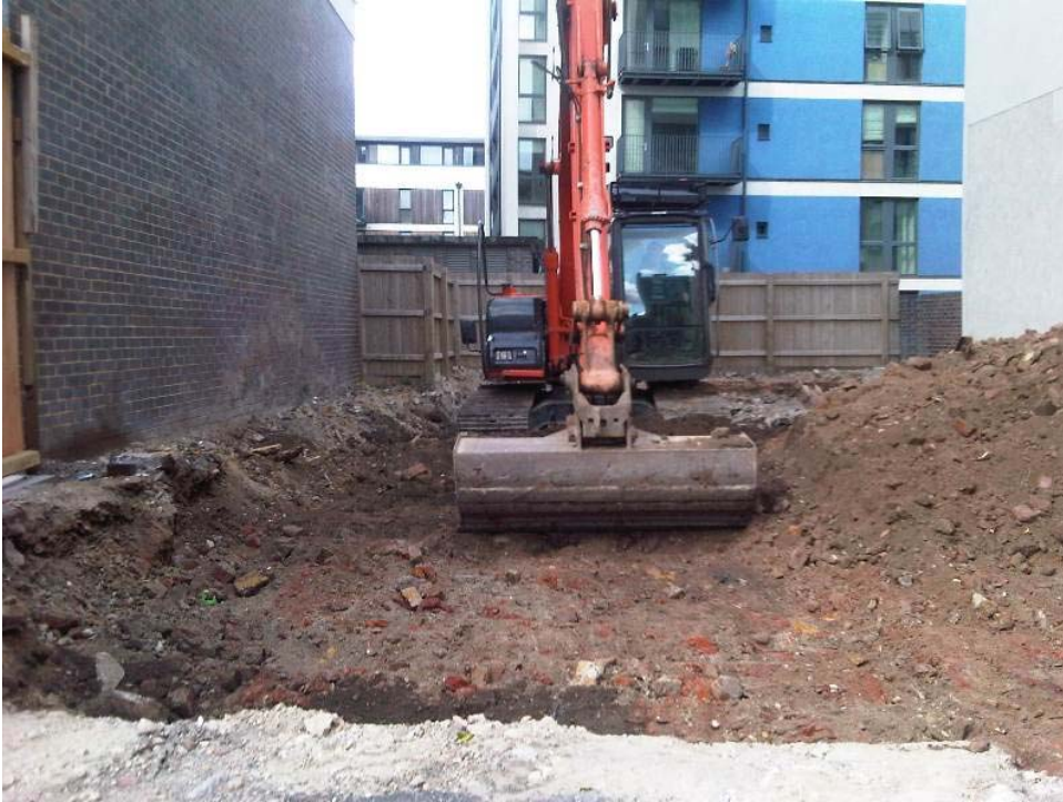
Plate 3: General shot of 0.60m ground reduction taking place
