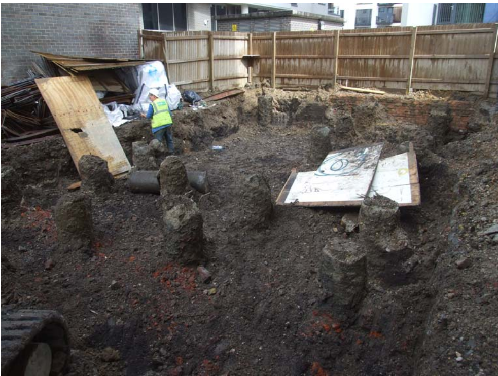
Plate 4: concrete piling after insertion
