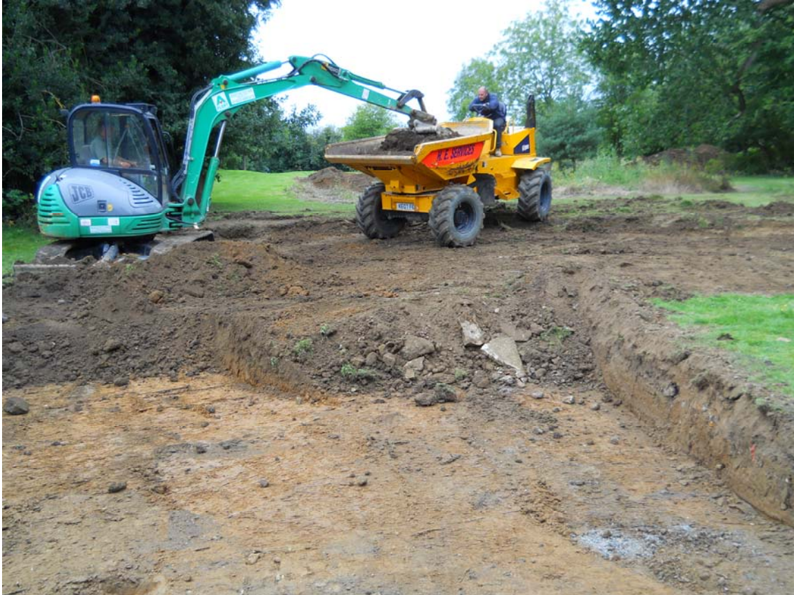
Plate 1: Excavation in Progress to surface of archaeology or natural clay
