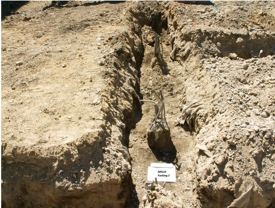
Photo 3: General shot of beam slots with pile cap showing
