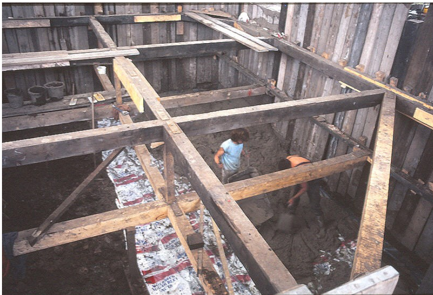
Illus. 2. Shoring in situ showing cramped working conditions
