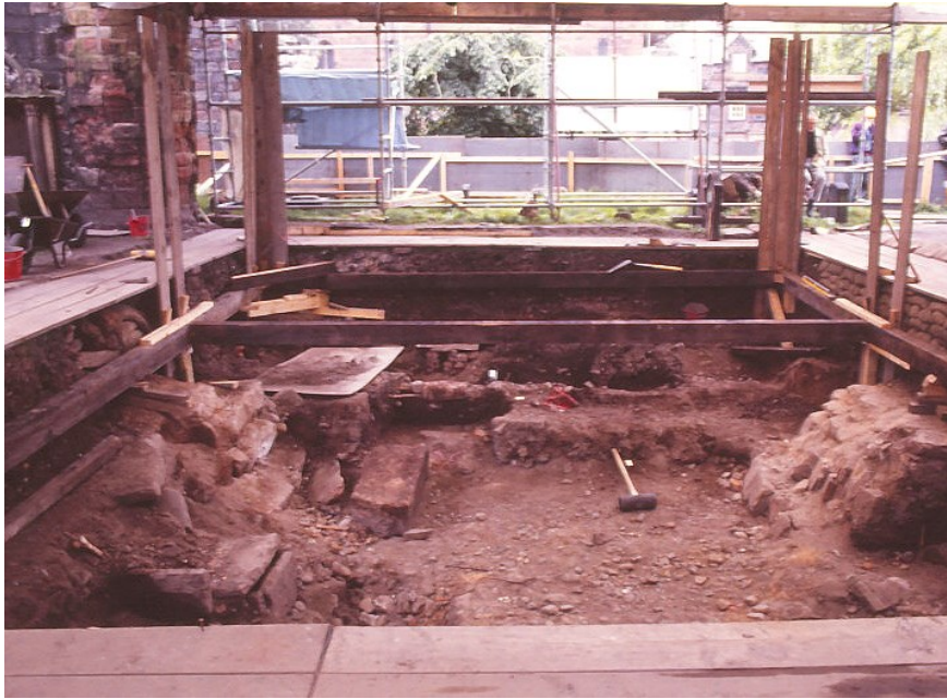
Illus. 1. Shoring being inserted.
