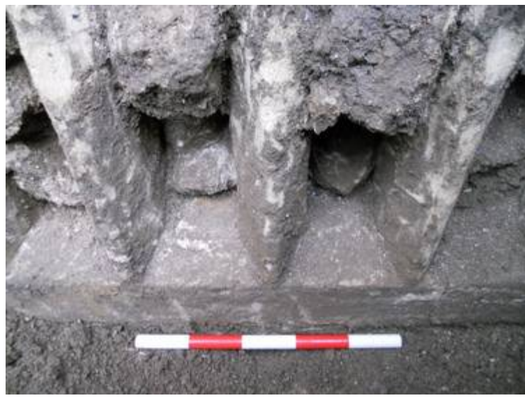
Fig. 24 Detail of the sill and mullions of the window.
