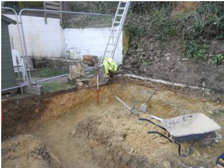
Fig. 27 Footing trenches for the new cabin, looking NW.
