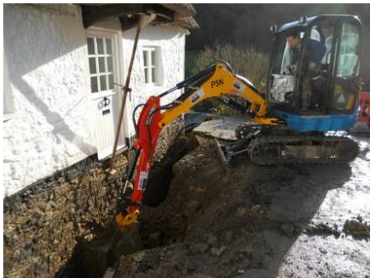
Fig. 19 Work in progress, excavating the French drain, looking SE.
