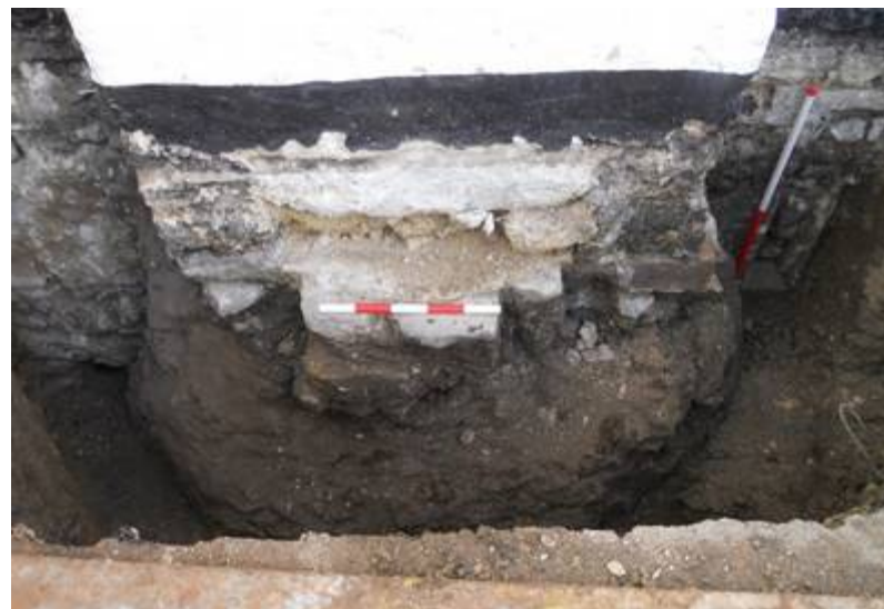
Fig. 20 The threshold of the former porch, showing footings, flagstones and masonry reveals, looking E.
