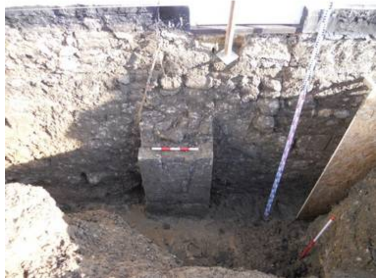
Fig. 26 Buttress fully exposed, with corbel/straight joint to S, looking E.
