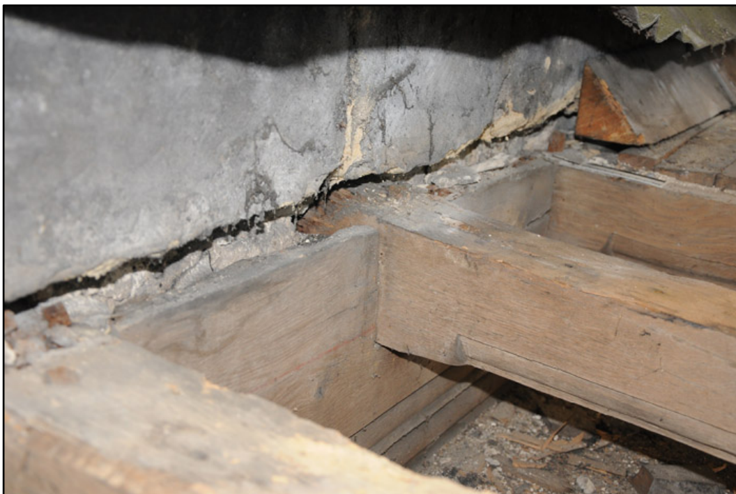
Appendix I.16: Detail of clerestory wall-plate; note how the ends of the rafters are recessed into the masonry.
