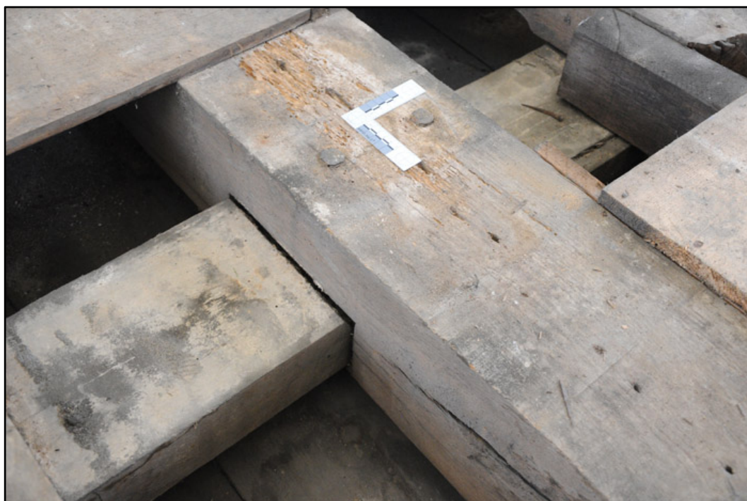
Appendix I.13: Detail of upper face of principal rafter 4; note central ribs are tenoned and securing with pegs (10cm scale).
