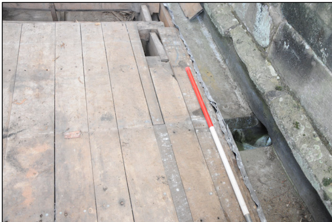
Appendix I.7: General view of upper face of roofing boards after lead sheeting removed (1m scale).
