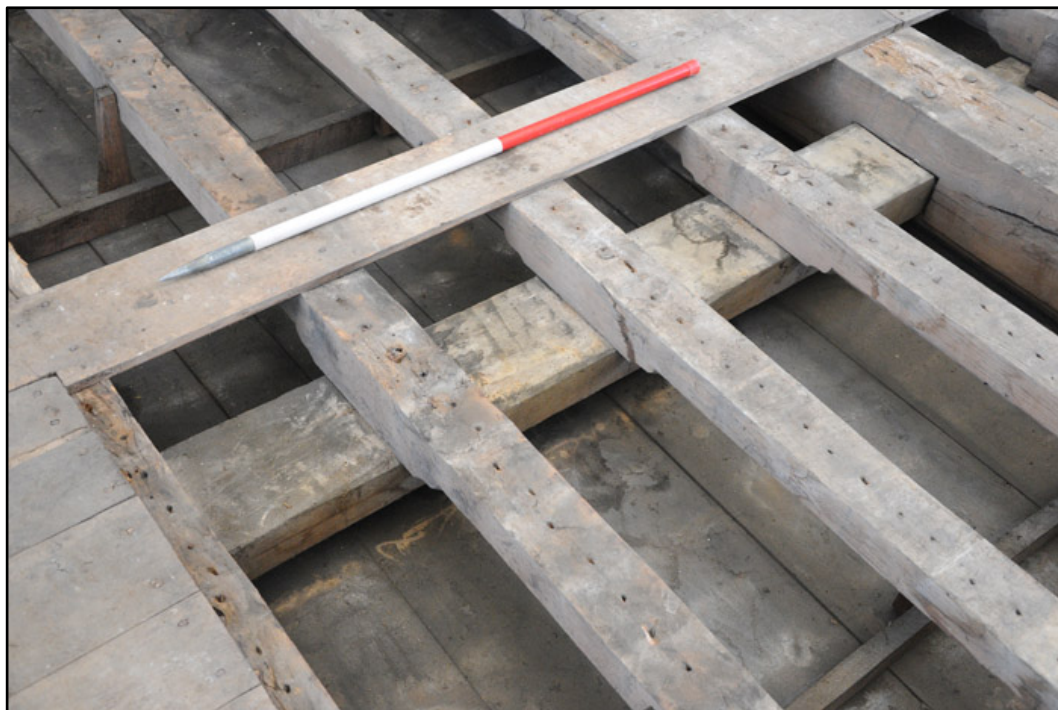
Appendix I.12: Detail of upper face of rafters that over sail the central rib; note each is secured with a peg (1m scale).
