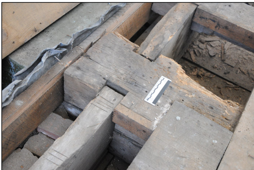
Appendix I.8: North wall-plates that are tenoned on either side of principal rafter 4; note assembly marks (10cm scale).
