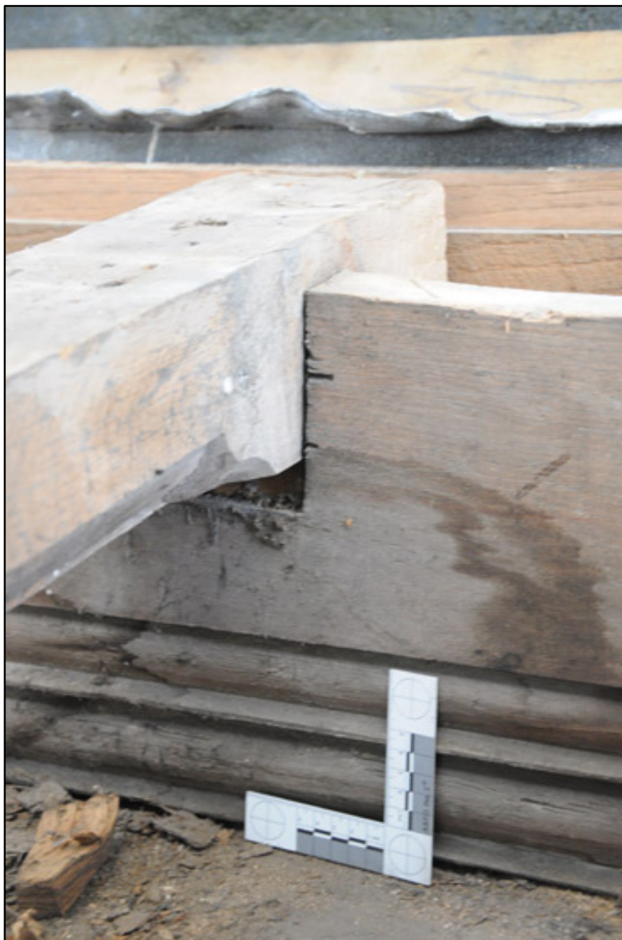
Appendix I.9: Detail of moulding on inner face of north wall-plate (10cm scale).
