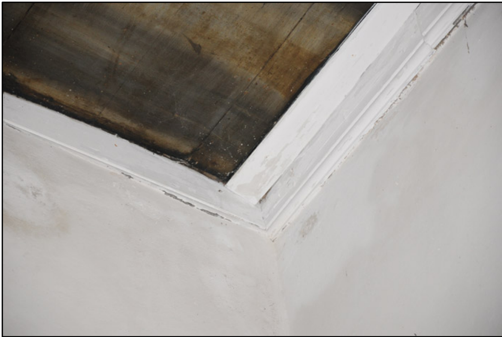
Appendix I.3: Detail of northeast corner of ceiling along north aisle; note timbers used to form a cornice below boards.
