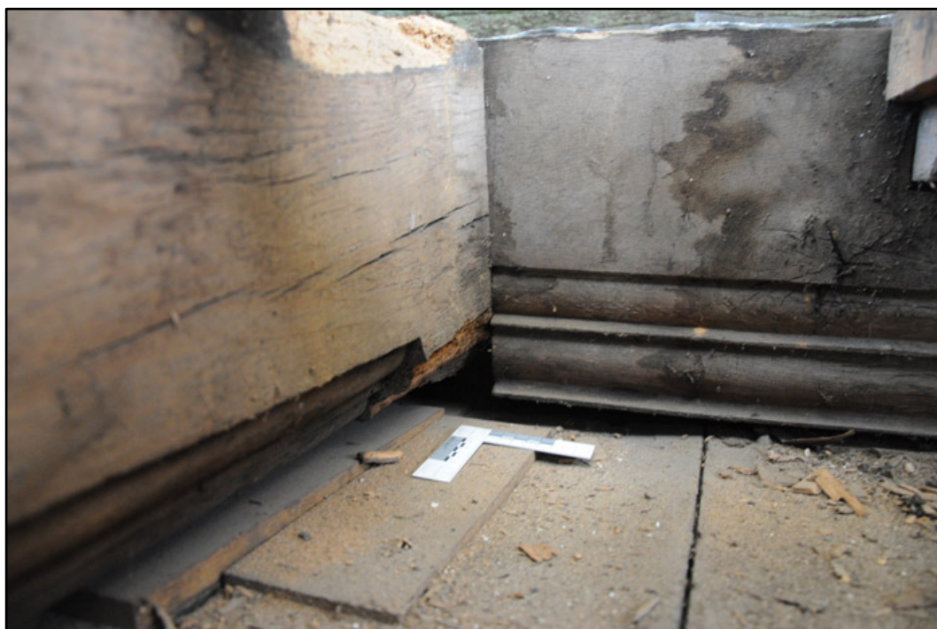
Appendix I.15: Detail of joint between principal beam 4 and north wall-plate (10cm scale).
