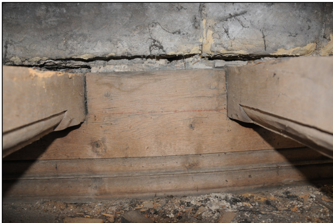
Appendix I.18: Detail of clerestory wall-plate above North Aisle; note original setting-out red pencil line.
