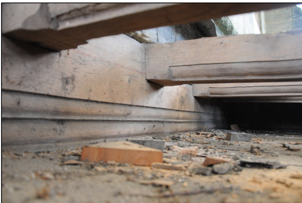
Appendix I.17: Detail of clerestory wall-plate; note crisp and unpainted mouldings on underside of the rafters.
