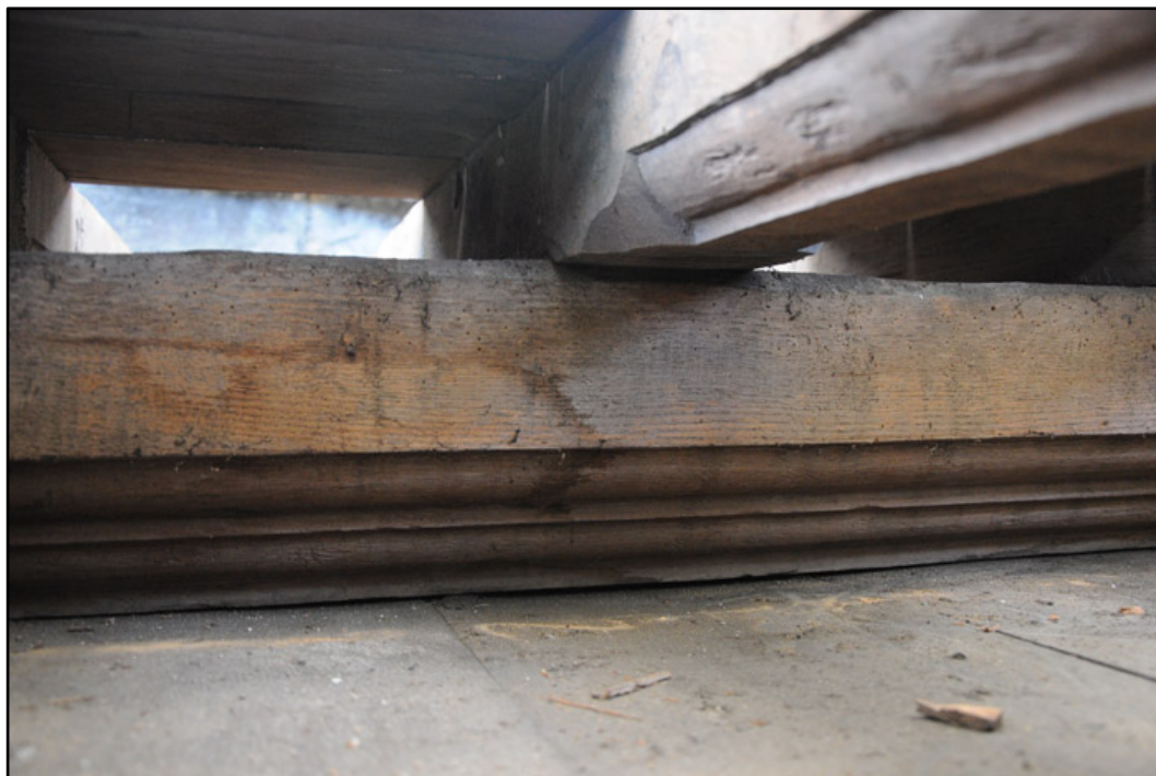
Appendix I.14: Detail of central moulded rib with over sailing rafters.
