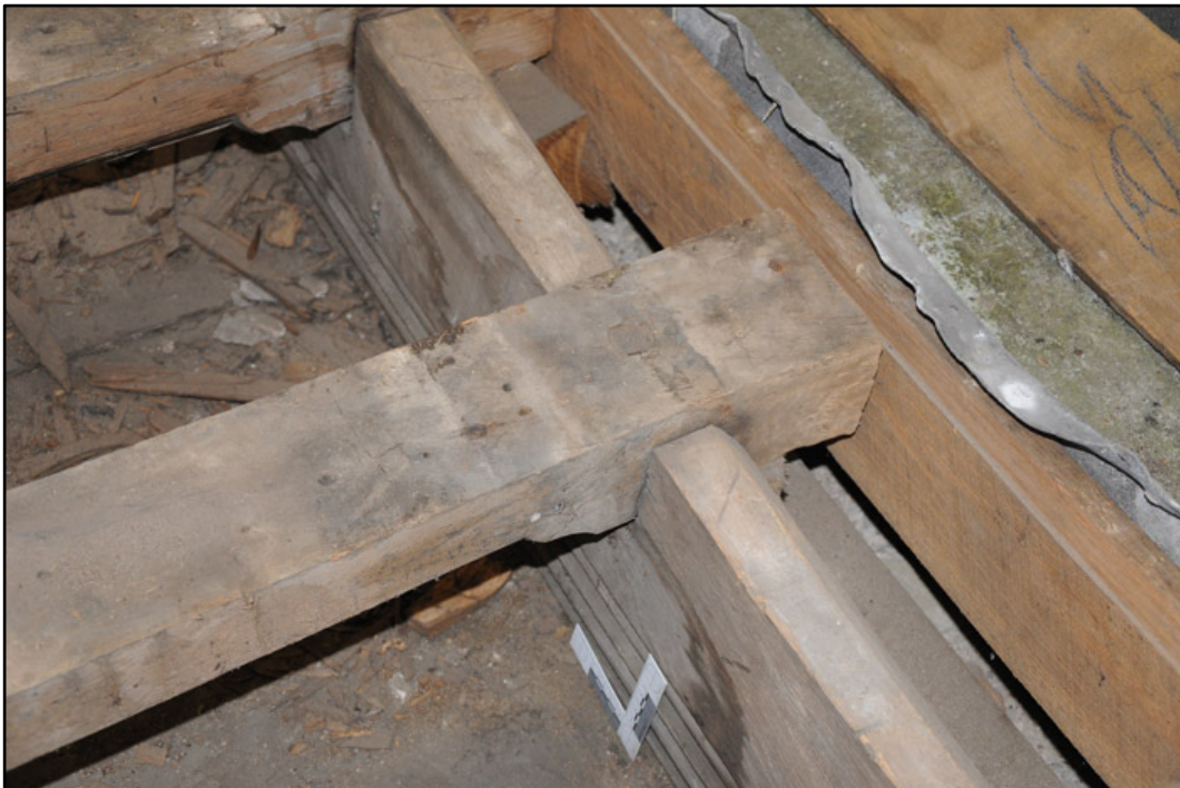
Appendix I.11: Detail of rafter secured with a peg in north wall-plate; note assembly mark 'X' (10cm scale).
