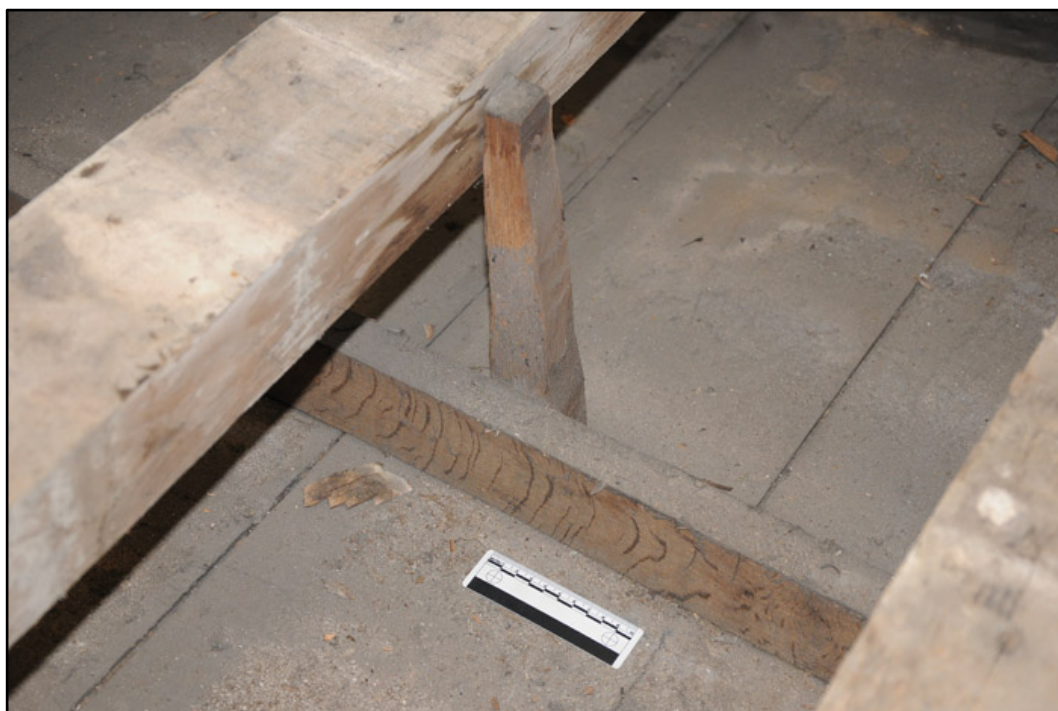
Appendix I.19: Detail of secondary struts used to hang boards for painted ceiling below (10cm scale).
