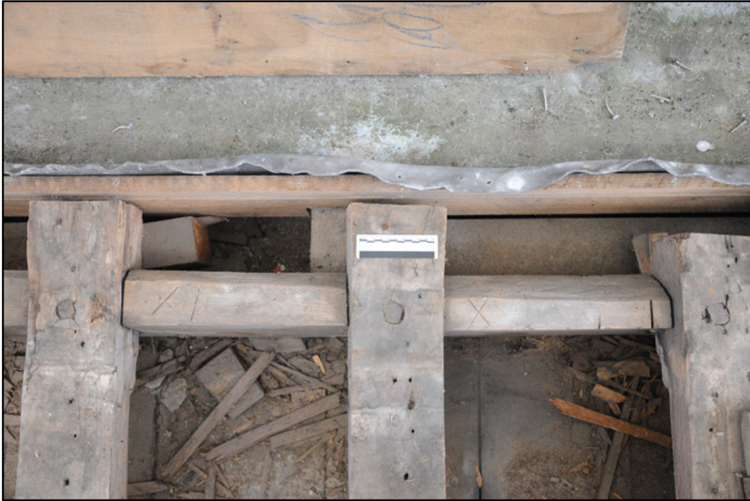
Appendix I.10: Detail of assembly marks on upper face of rafters secured into north wall-plate (10cm scale).
