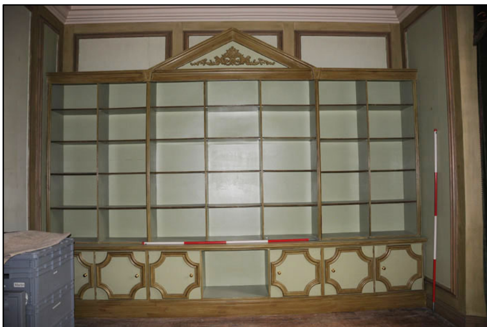
Inserted bookcase against south wall of room FG.I (2m scale)
