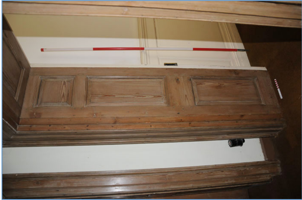
Detail of north doorway leading to east corridor FG.2 (1m scale)
