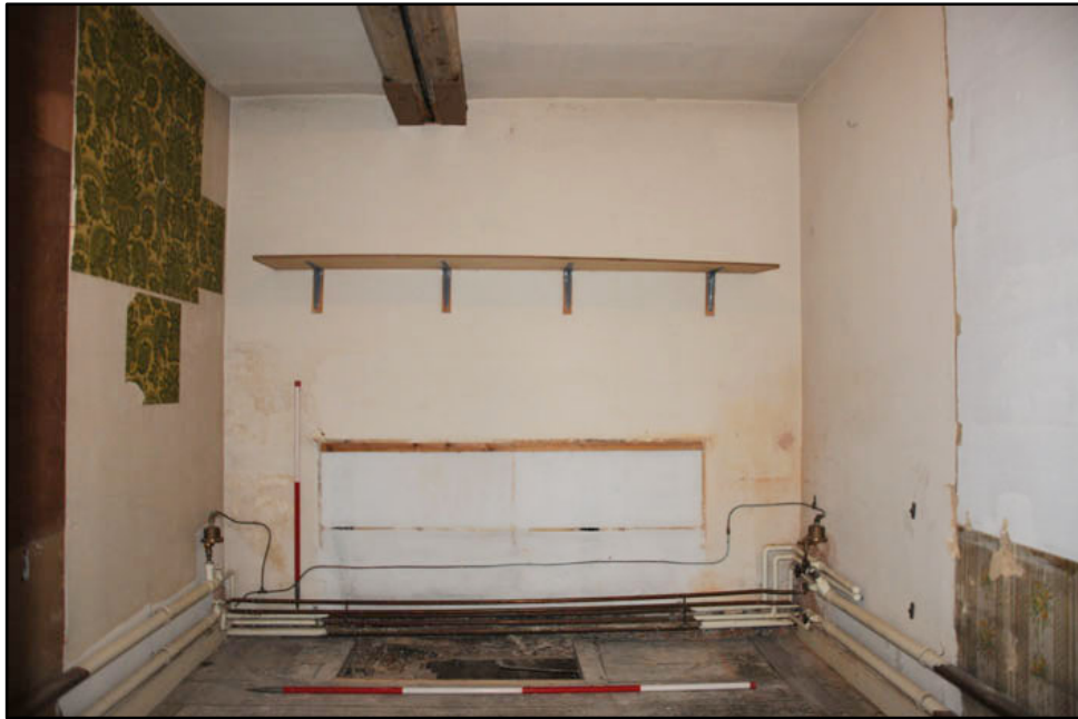
Room SG.4 looking east; note trimmer beams in floor for former hearthstone and scar in rear wall from blocked fireplace (1m/2m scale)
