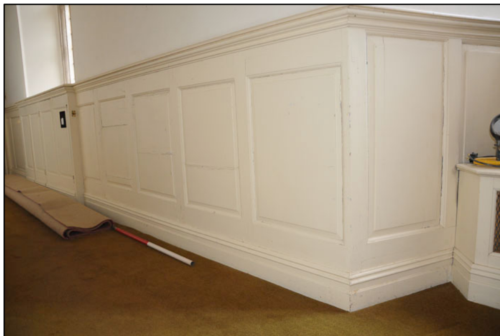
Detail of paneling along east wall of east corridor FG.2 ; site of former fireplace (1m scale)
