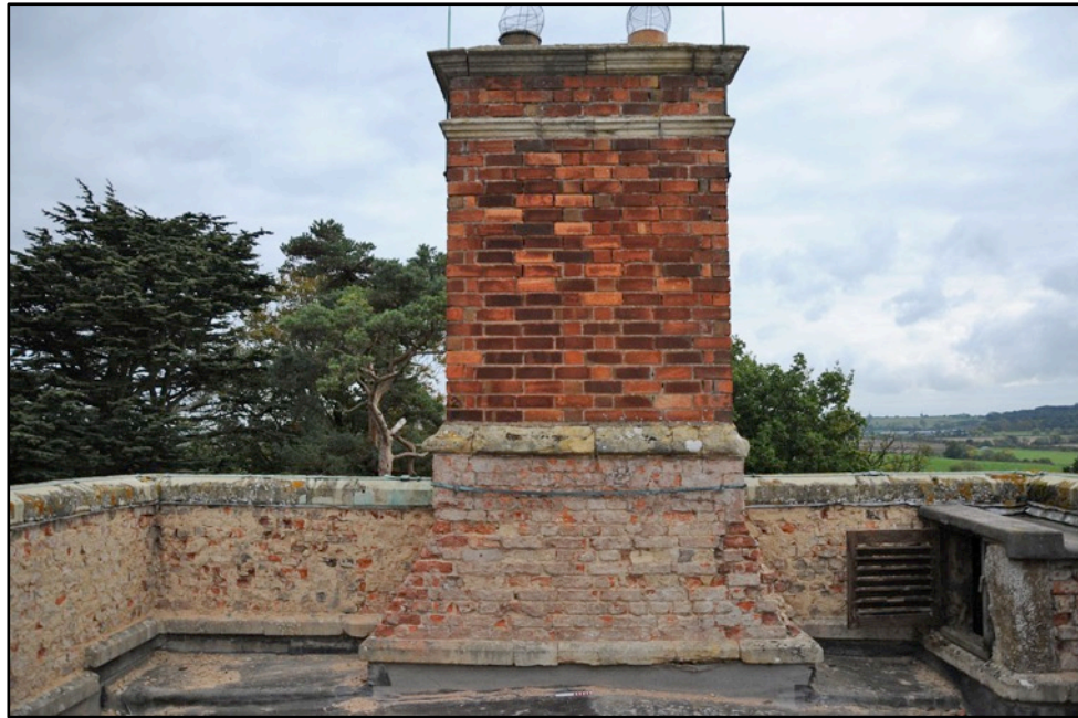
General view of chimney stack against the east parapet of the north wing (20cm scale)
