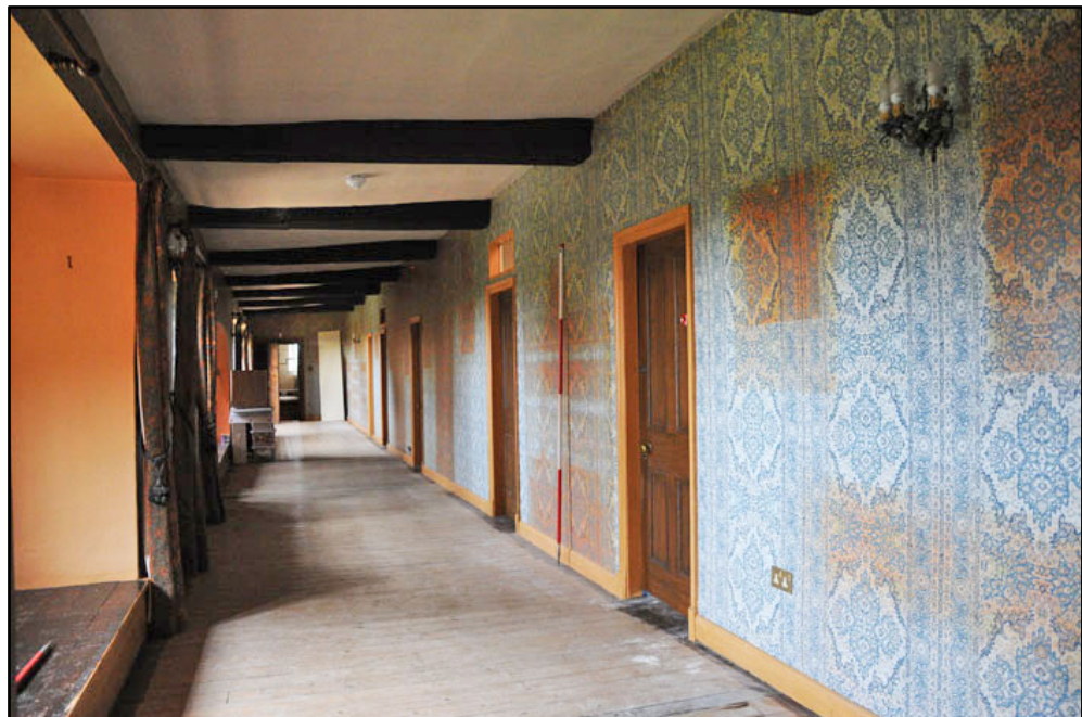
View along attic corridor SG.1 , looking north (2m scale)
