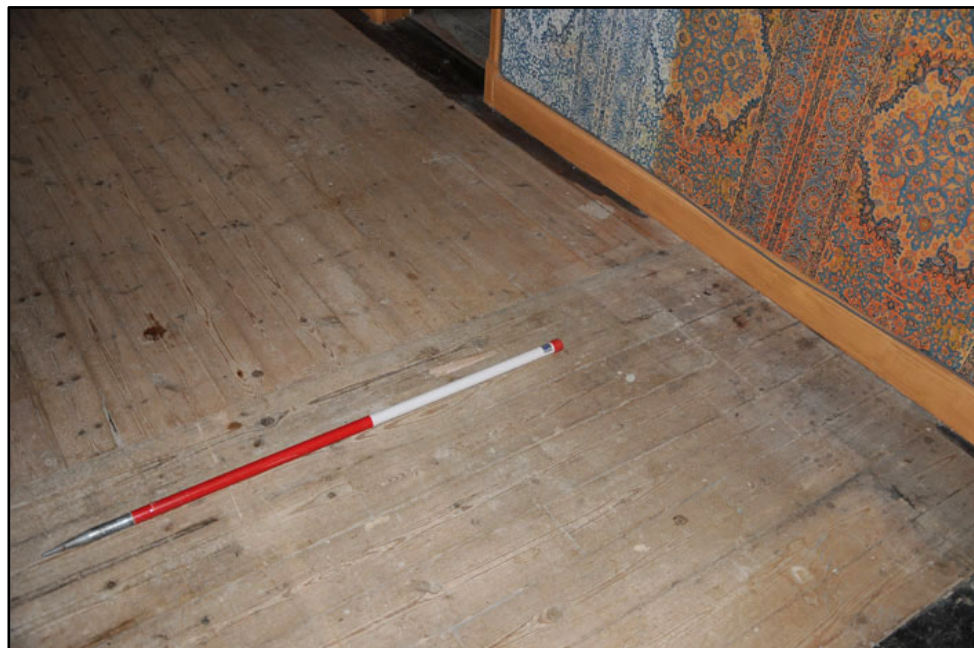
Detail of change in floorboards in SG.1 ; note location of former partition (1m scale)
