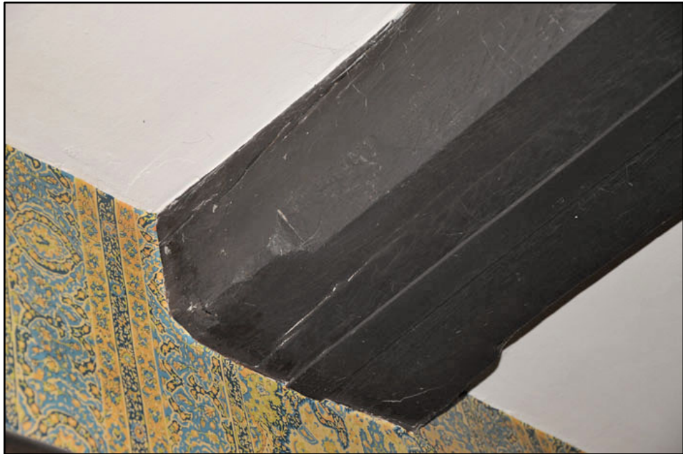
Detail of lambs-tongue stop and chamfer at end of ceiling beam in SG.I
