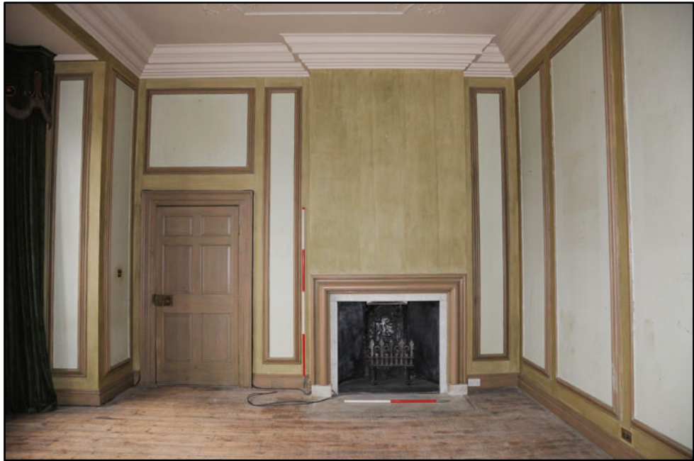
General view of north wall of room FG.I ; note inserted fireplace (1m/2m scale)
