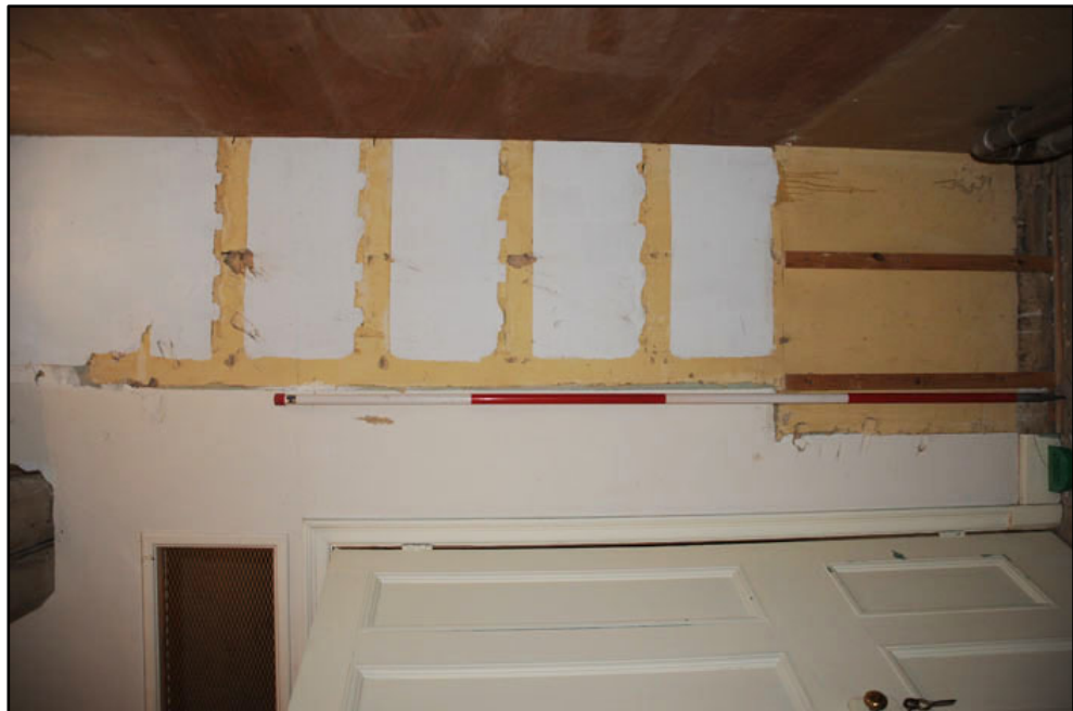
Detail of scar from former laundry shelves in SG.4 ; note lath and plaster construction (2m scale)
