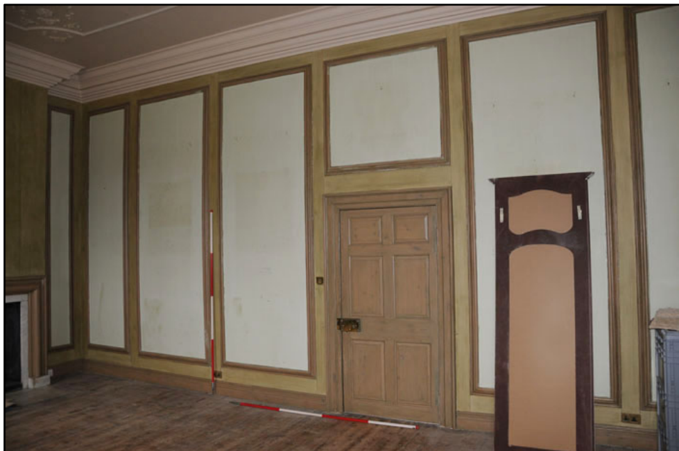
General view of east wall of room FG.I (2m scale)
