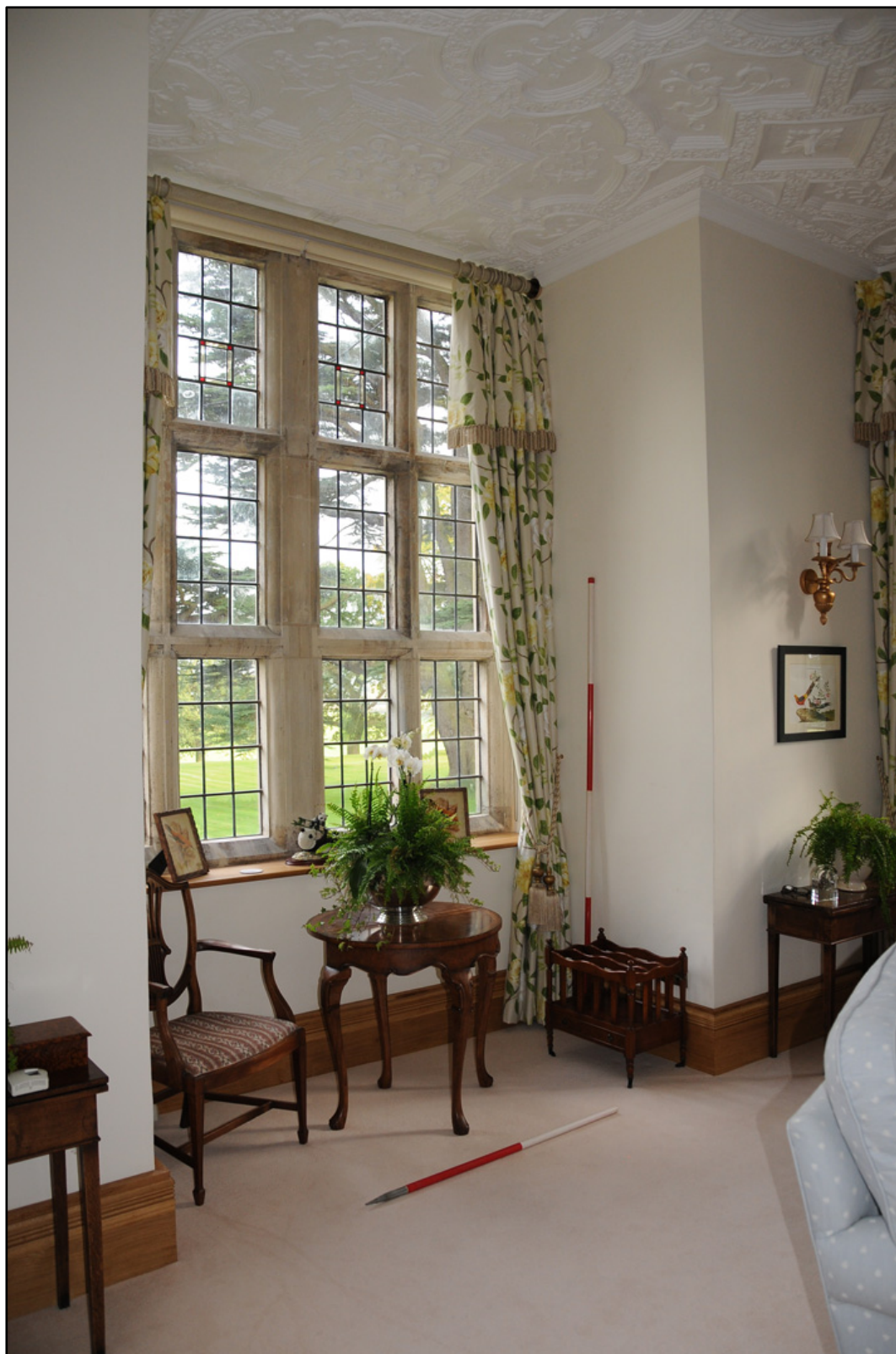
General view of altered window in east wall of room GM (1m/2m scale)
