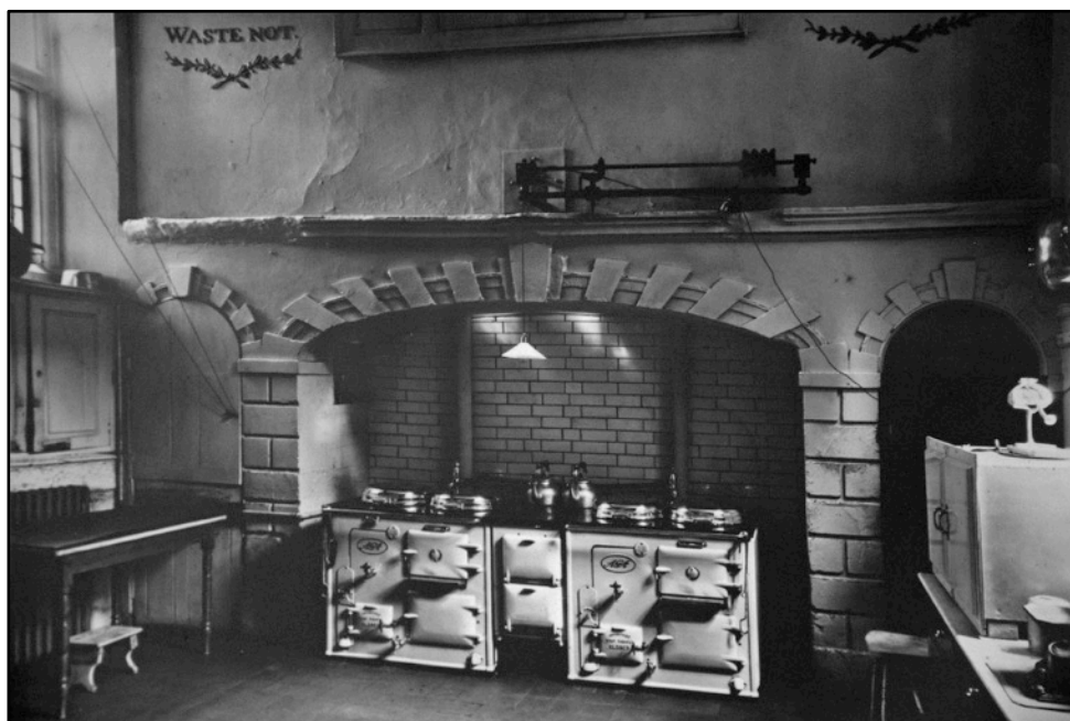
The kitchen in c.2 nd quarter of 20 th C; note lower floor level
