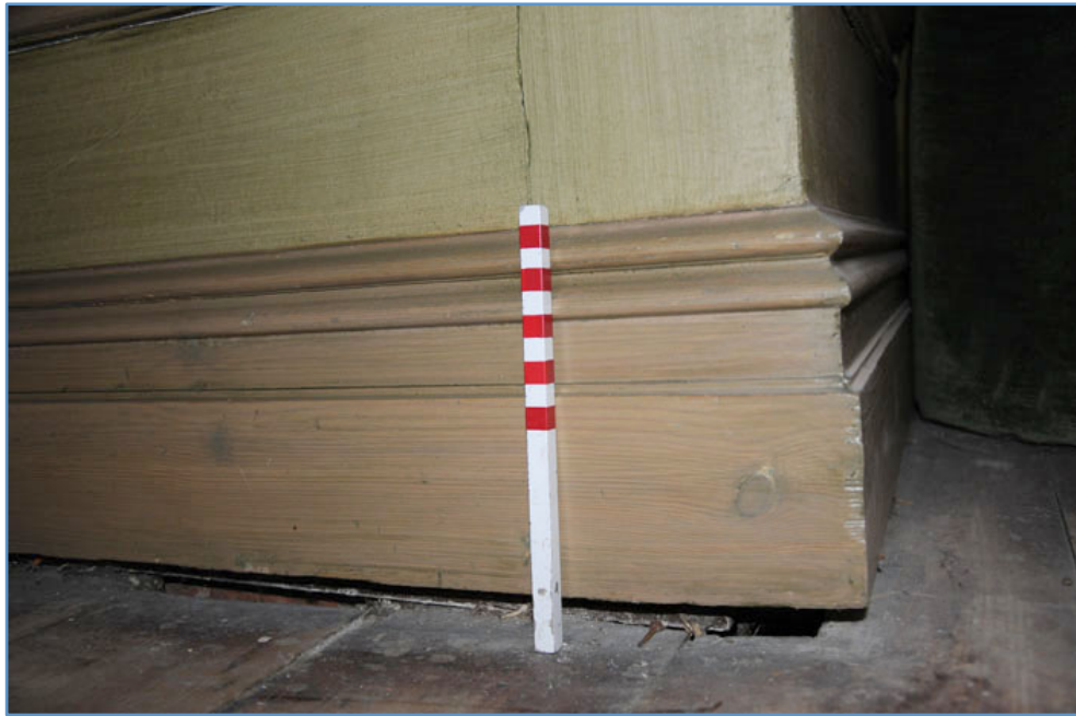
Detail of skirting in room FG.1 ; note floorboards and joists do not match (20cm scale)
