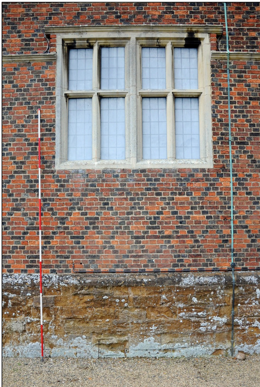
Detail of external ground floor elevation of east elevation of north wing (4m scale)
