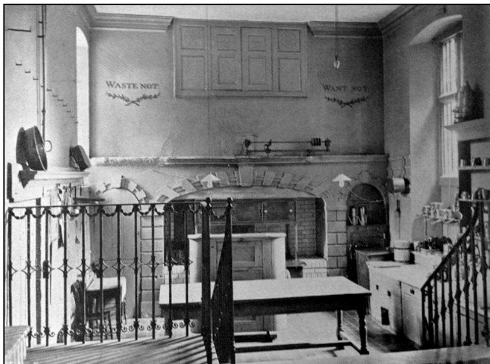
The kitchen in c.1911; note lower floor level and step leading up to the servants hall to the left
