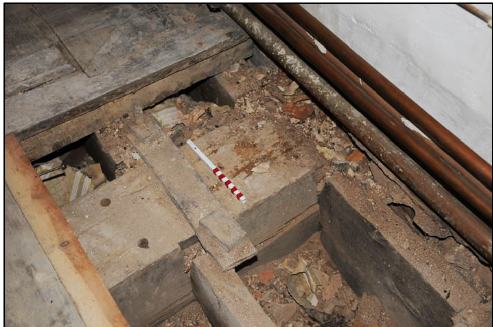
Detail of exposed floor beam in east wall of SG.4 ; note metal strap from historic repair (20cm scale)
