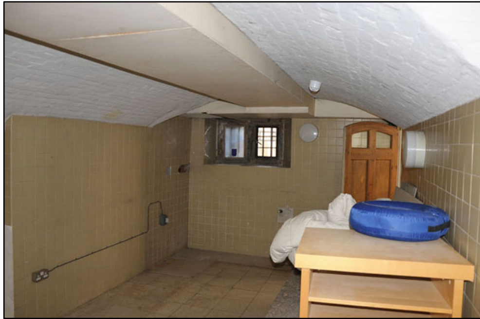
General view of cellar BE previously used as a game larder, looking north
