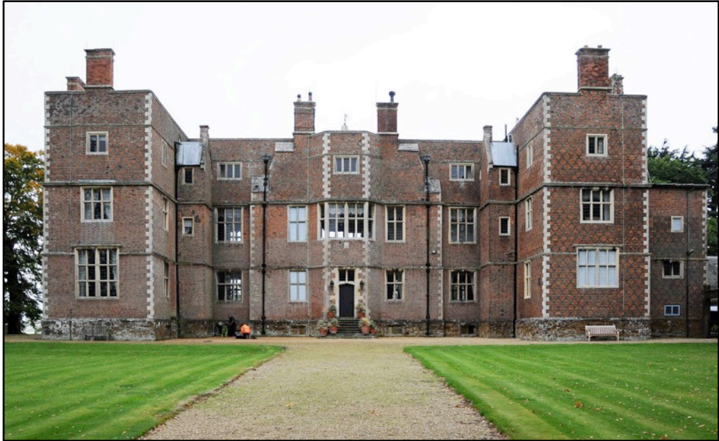
General view of east elevation of Quenby Hall; note ground floor windows on projecting wings
