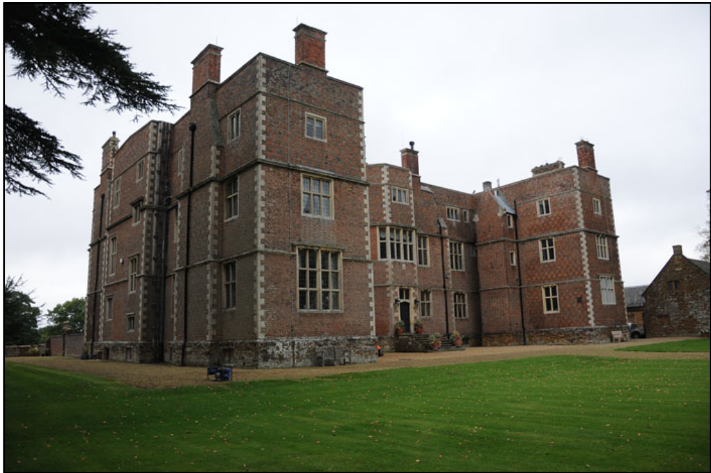
General view of east elevation of Quenby Hall, looking northwest
