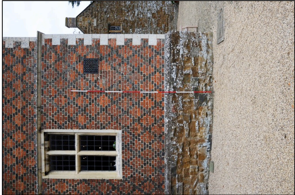
Southeast section of kitchen elevation of north wing; note inserted cast-iron vent (4m scale)
