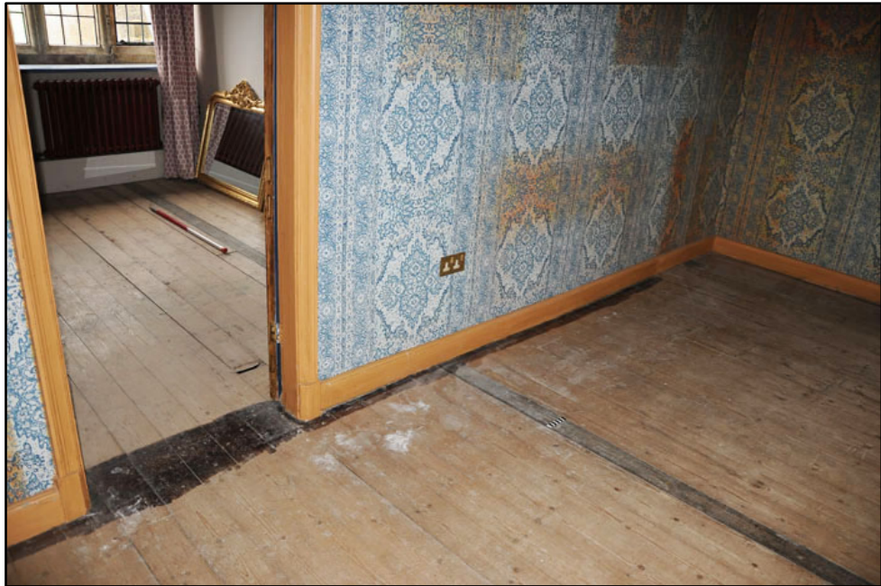
Detail of the floorboards that continue beneath the partition between SG.1 and SG.7 ; note inserted cast iron floor beam (1m scale)
