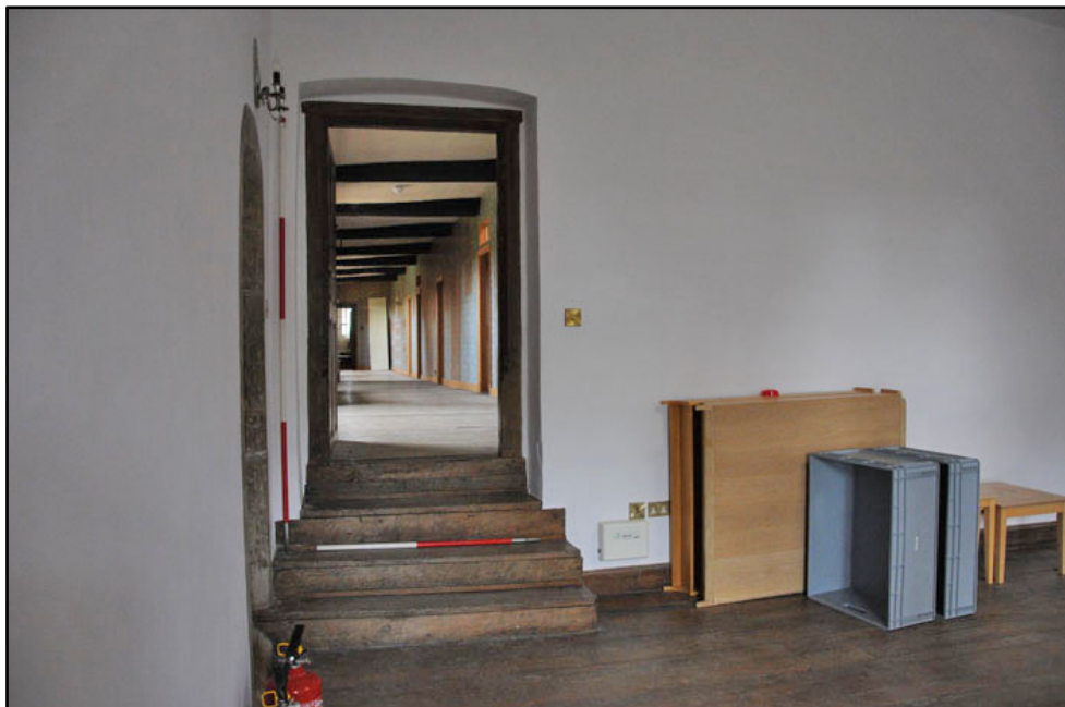
View of doorway at south end of attic corridor SG.1 , looking north (1m/2m scale)
