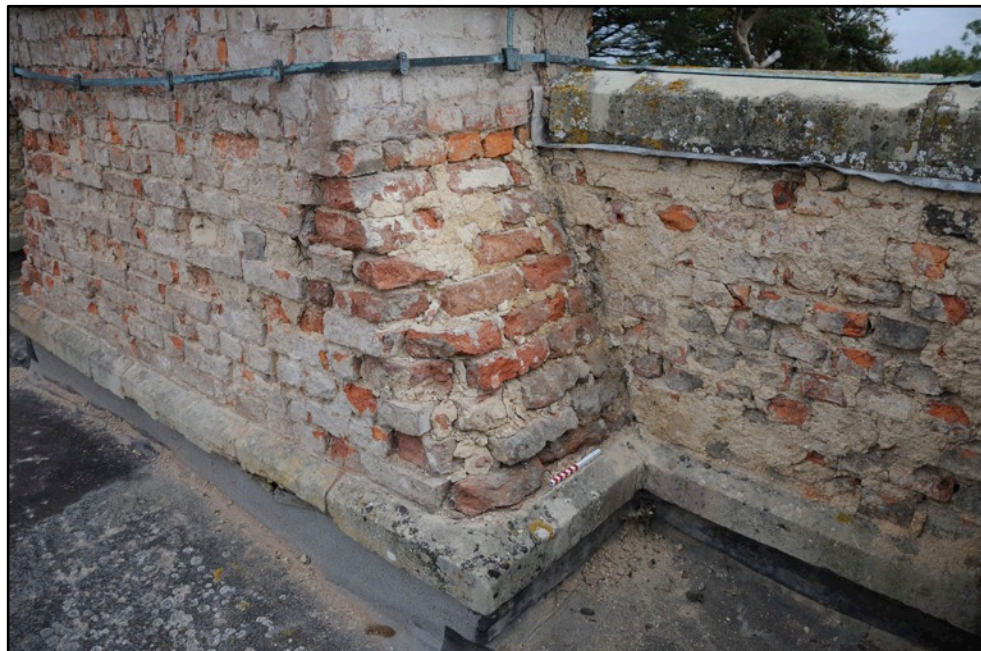
Detail of exposed brickwork against east parapet of the north wing; note continuous plinth (20cm scale)
