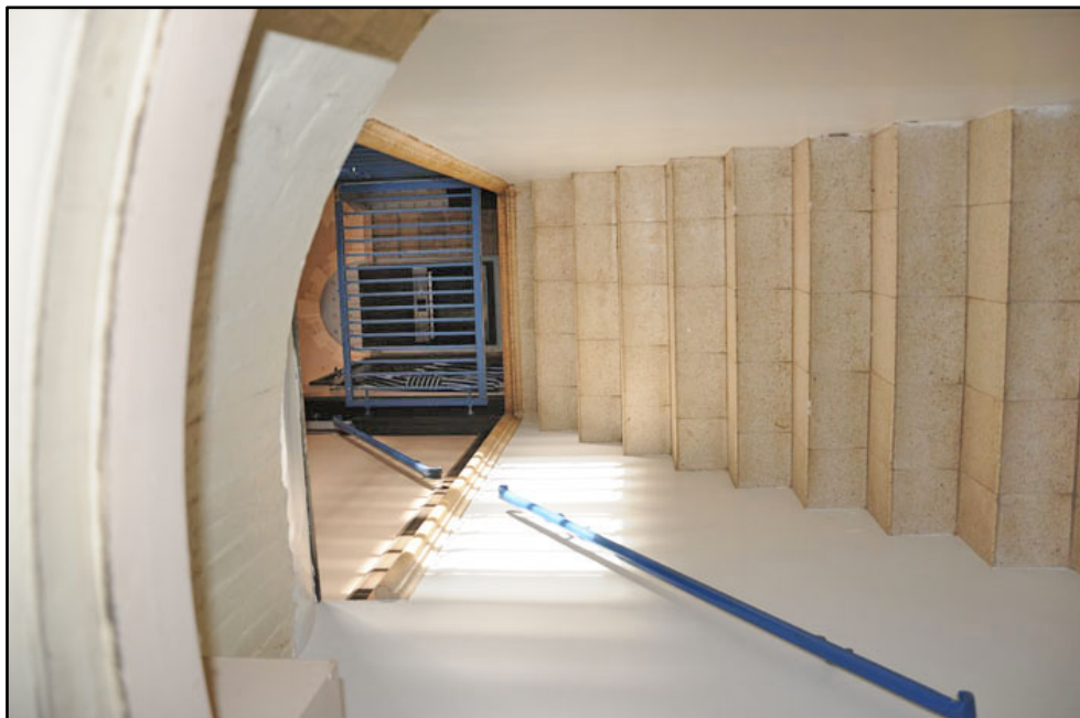
General view looking up towards kitchen from cellar BE ; site of blocked doorway to the left
