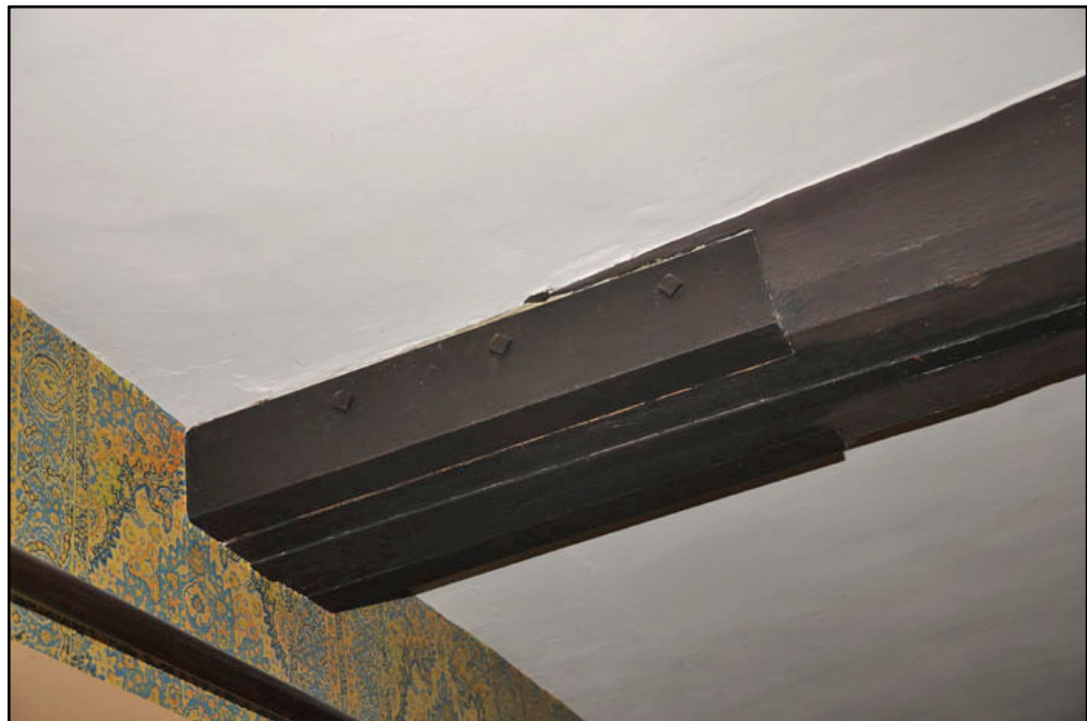
Detail of metal repair at end of ceiling beam in SG.I
