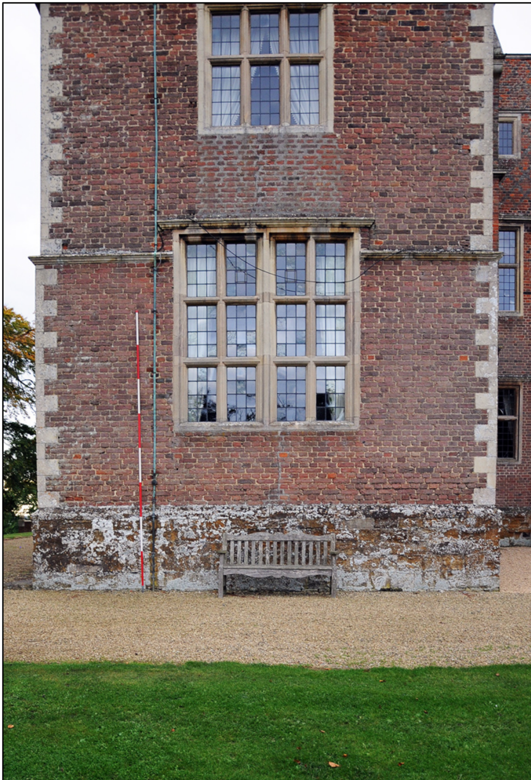
Detail of external ground floor elevation of east elevation of south wing (4m scale)
