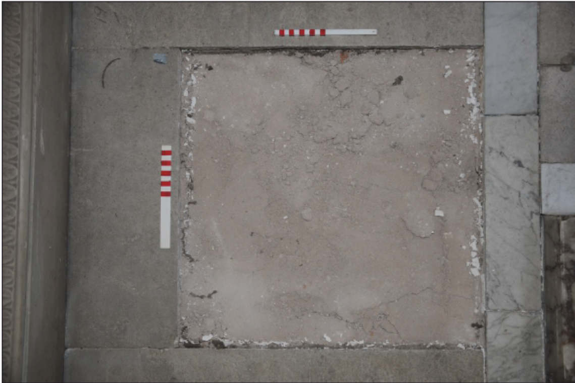
Appendix 2.3: General view of pale pink sand/mortar subfloor in OBI (20cm scale). Photo No.9.
