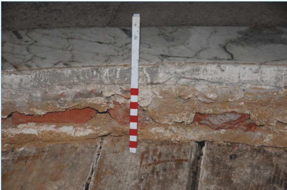
Appendix 2.24: Detail of brick and mortar foundation below outer arc of marble paving in OB6 (20cm scale). Photo No.75.
