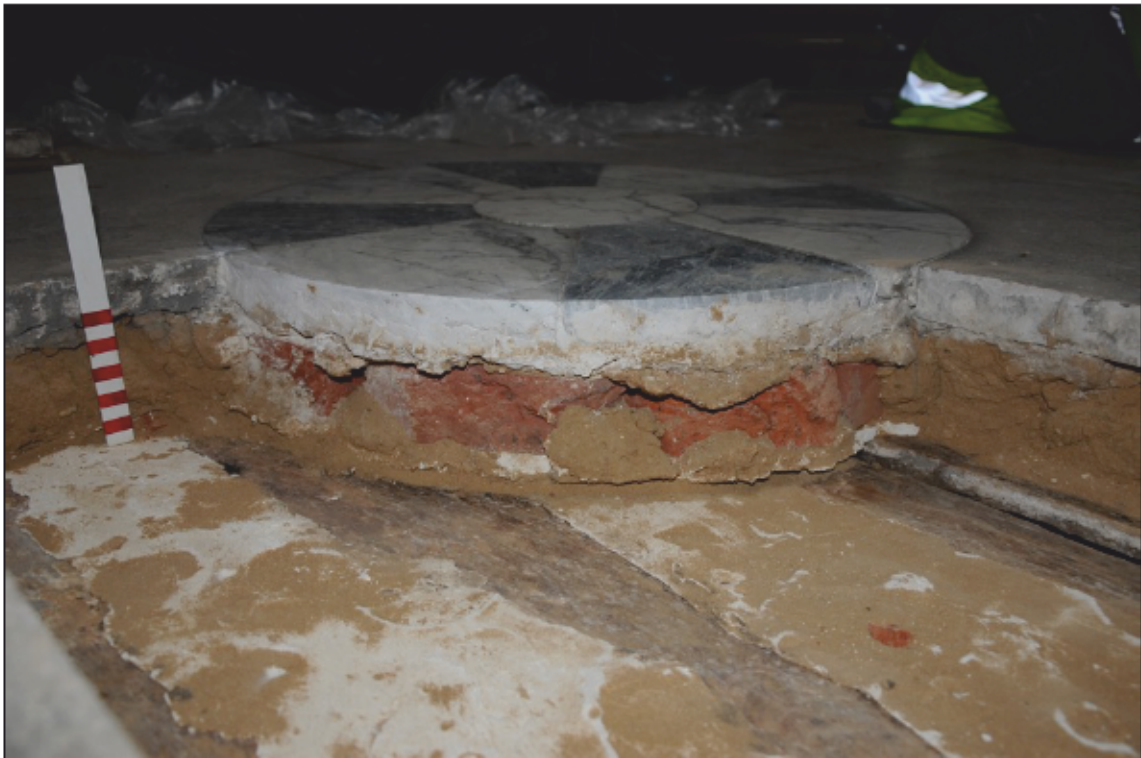
Appendix 2.13: Detail of roundel in OB3, looking west; note mortar torching covering joints (20cm scale). Photo No.35.
