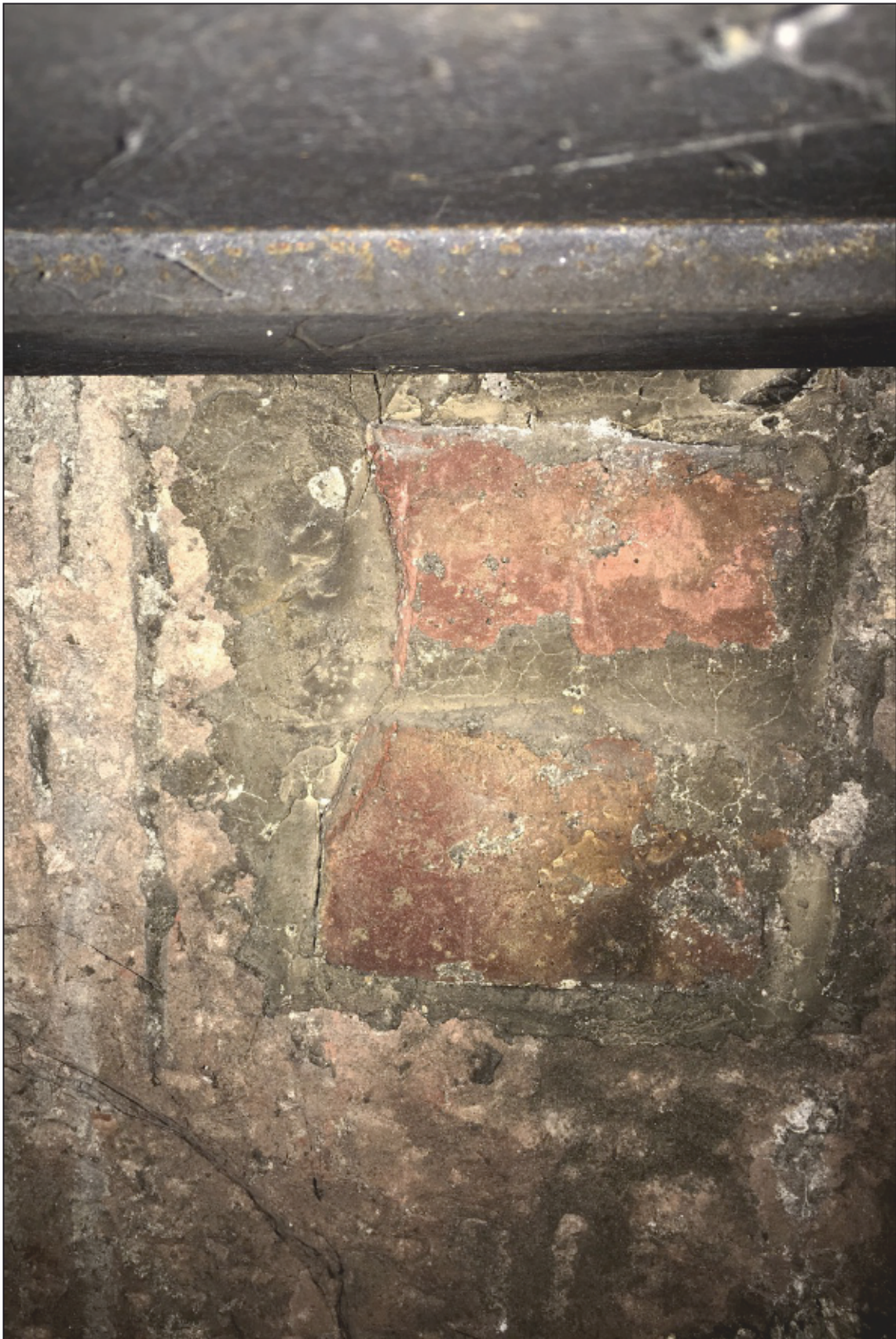
Appendix 2.7: Detail of brick blocking following removal of floor beam below floor in OB2, looking north. Photo No.20.
