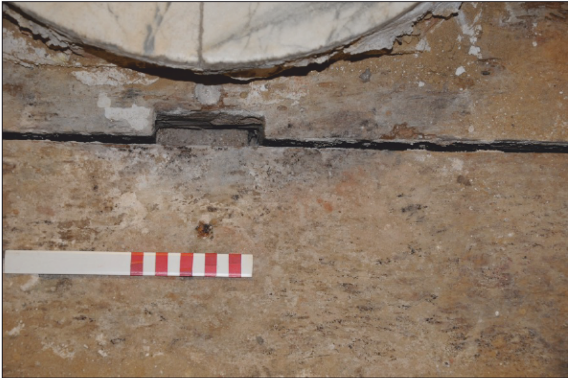
Appendix 2.23: Detail of exposed mortice and tenon in OB6, looking south (20cm scale). Photo No.80.
