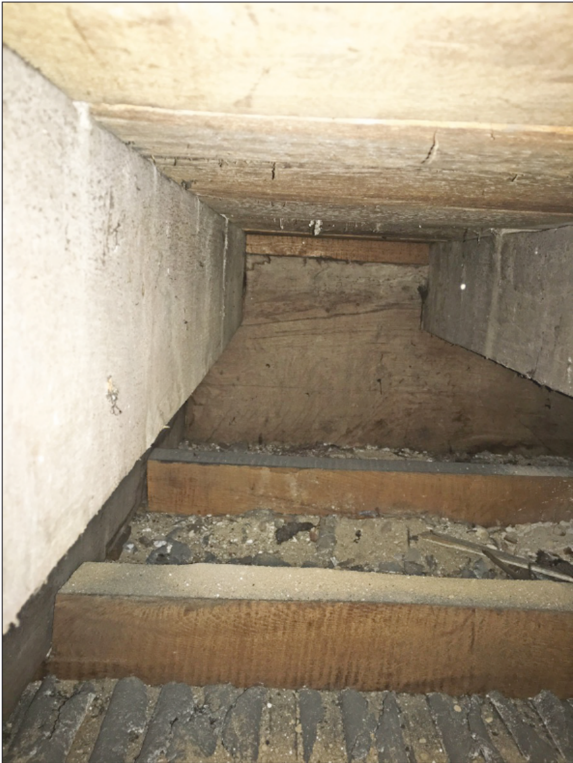
Appendix 2.31: General view of floor void in OB7, looking north; note ceilings joists extend under lower floor joist. Photo No.96.
