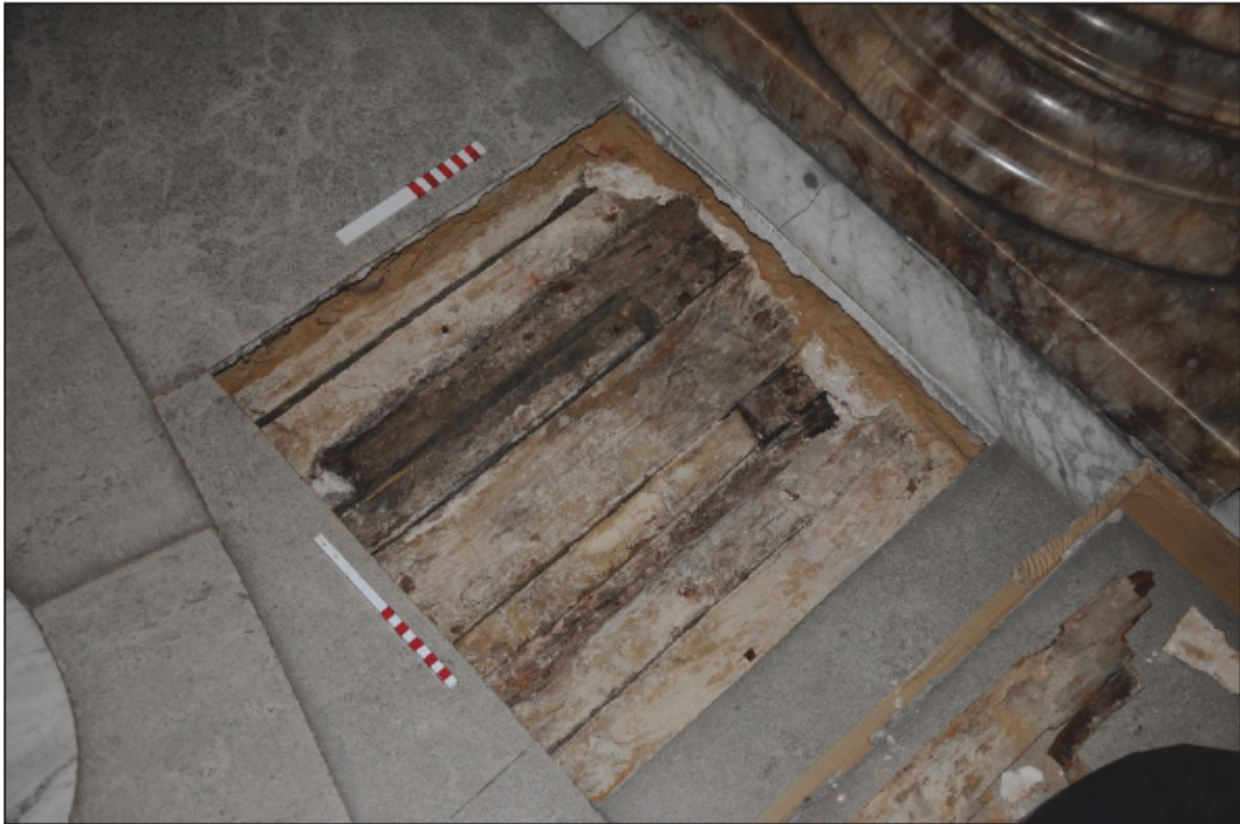
Appendix 2.15: General view of OB4, looking northeast; note inserted secondary planks (20cm scale). Photo No.49.
