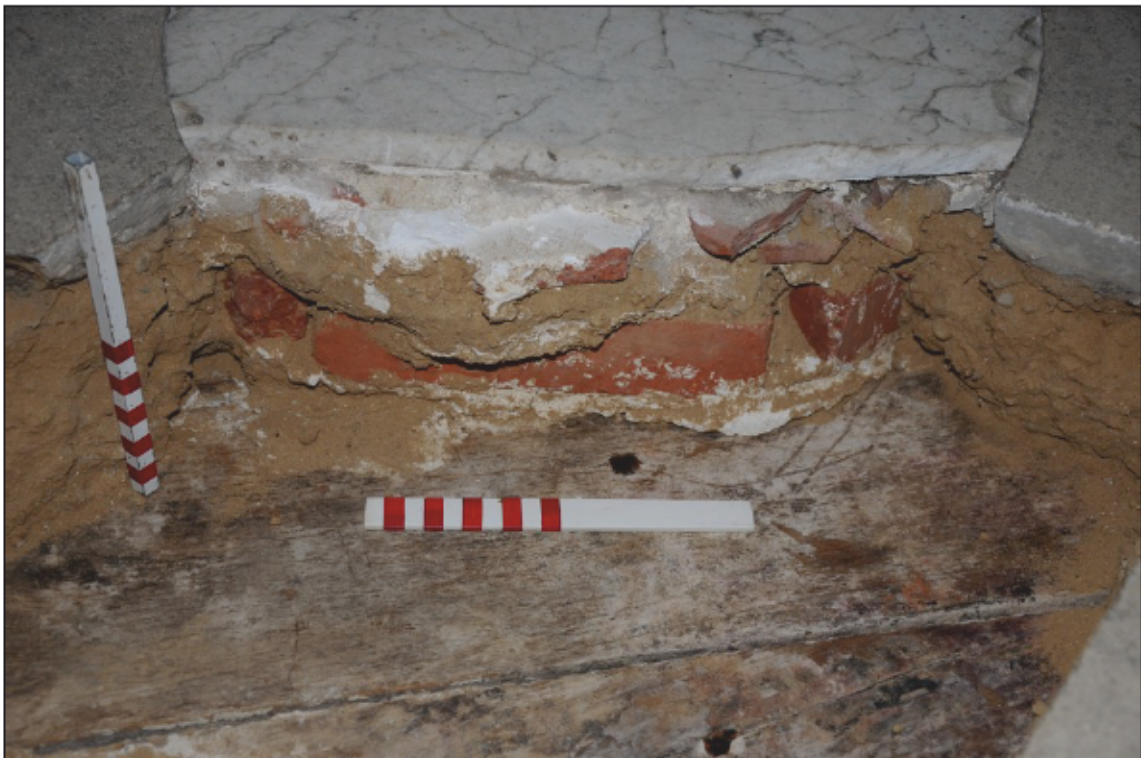
Appendix 2.18: Detail of brick and mortar foundation below marble petal in OB5, looking south (20cm scale). Photo No.60.
