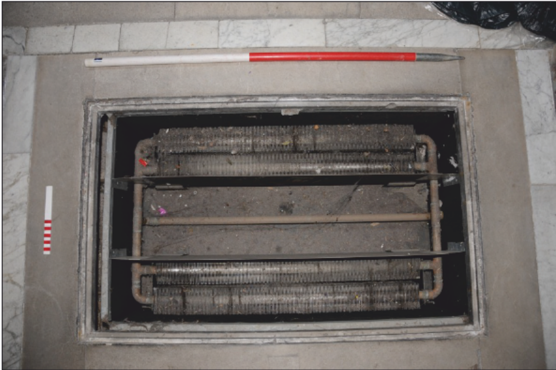
Appendix 2.5: General view of inserted floor heater in OB2 from above (20cm scale). Photo No.17.
