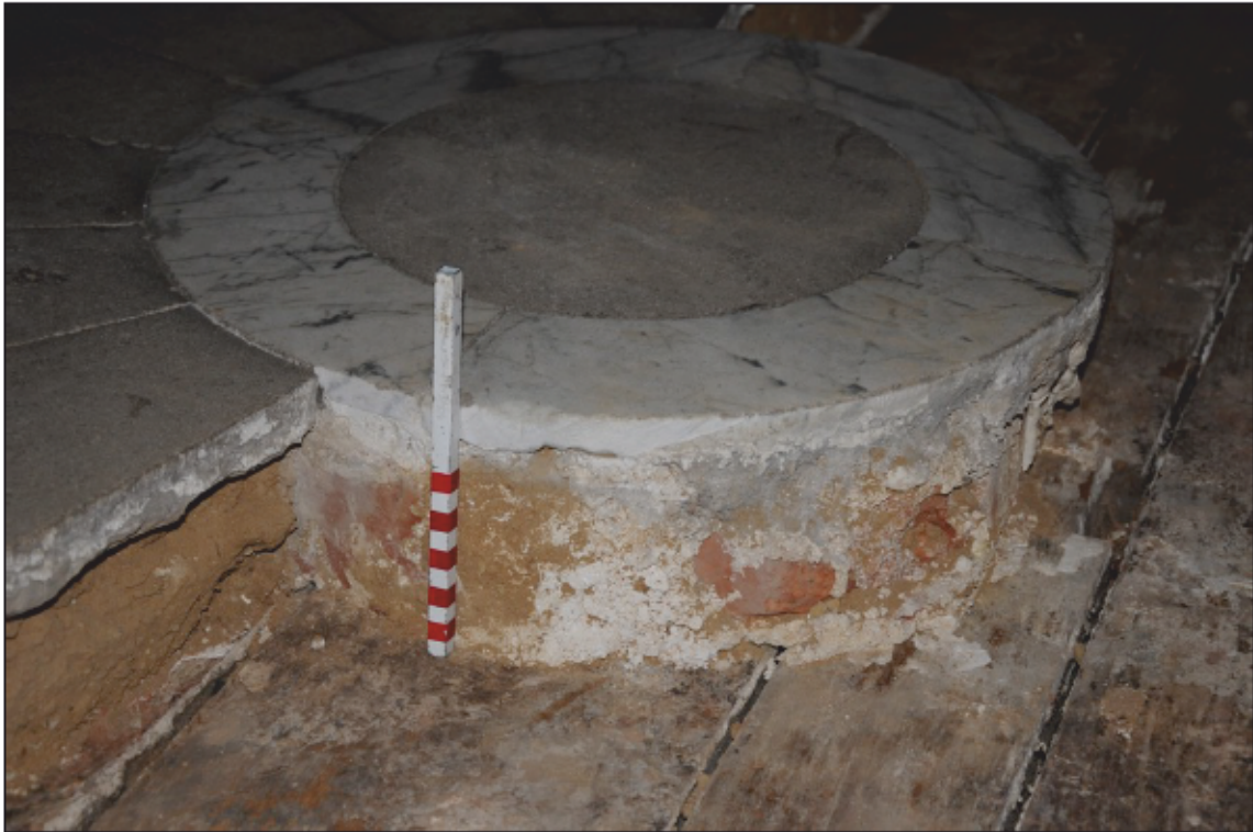
Appendix 2.25: Detail of mortar and brick foundation below roundel in OB6, looking southwest (20cm scale). Photo No.74.
