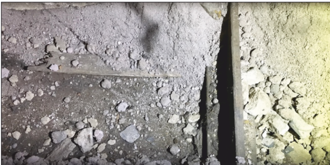
Appendix 2.6: Detail of inserted small RSJ's below floor in OB2 to support floor heater, looking north. Photo No.23.
