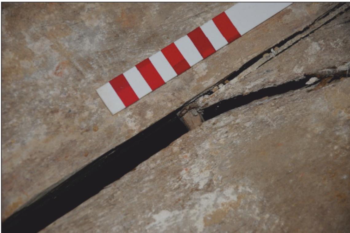
Appendix 2.30: Detail of dowel in OB7, looking south (1cm scale divisions). Photo No.91.
