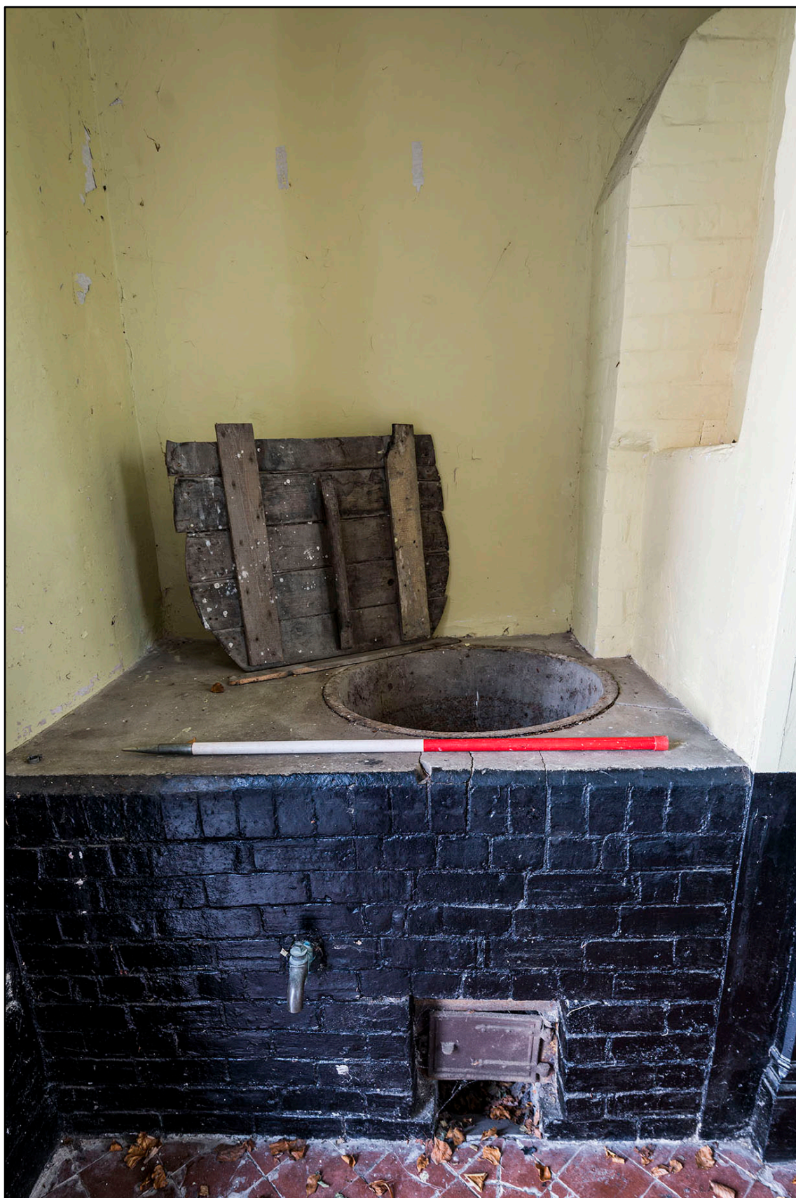
Appendix 2.43: Detail of (east) cast-iron laundry boiler and lid in room 2G4 (Clock House) (1m scale).Photo No.76
