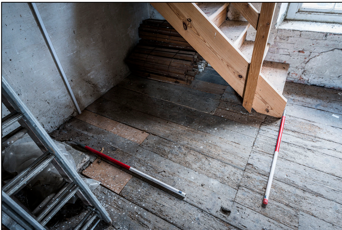
Appendix 2.55: Detail of planking denoting site of earlier staircase in room 2F5 (Clock House) (1m scale). Photo No.91
