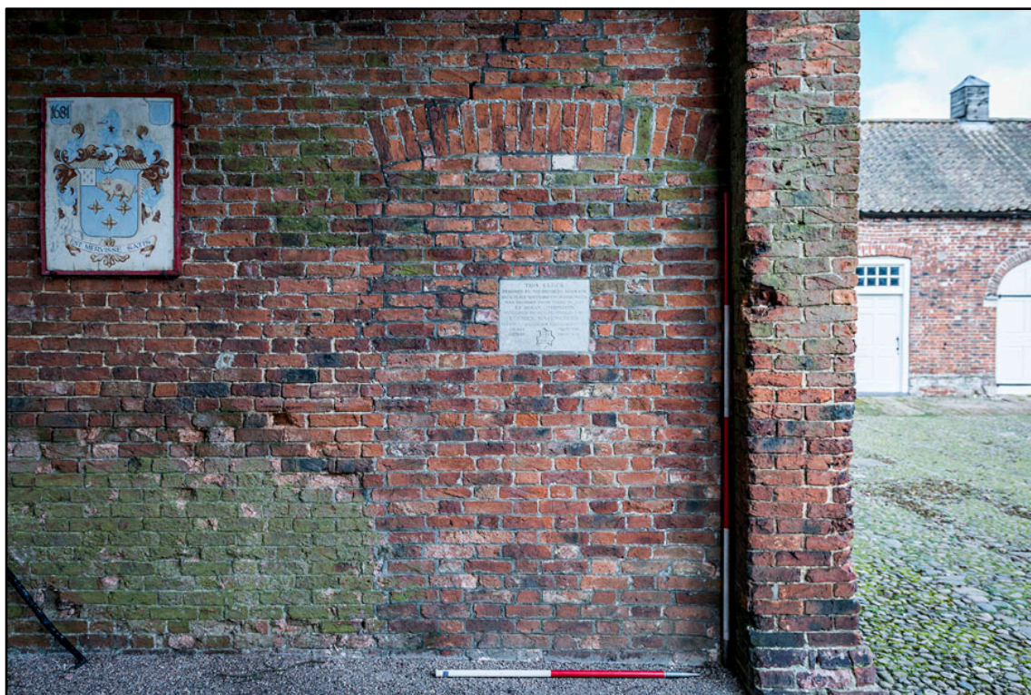
Appendix 2.25: Detail of blocked doorway in north wall of Clock House entrance passage 2G3 (1m/2m scale). Photo No.38
