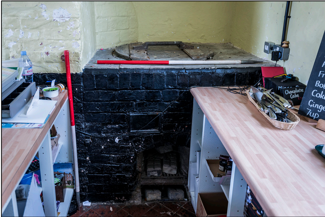
Appendix 2.41: Detail of (west) cast-iron laundry boiler and lid in room 2G4 (Clock House) (1m scale). Photo No.78
