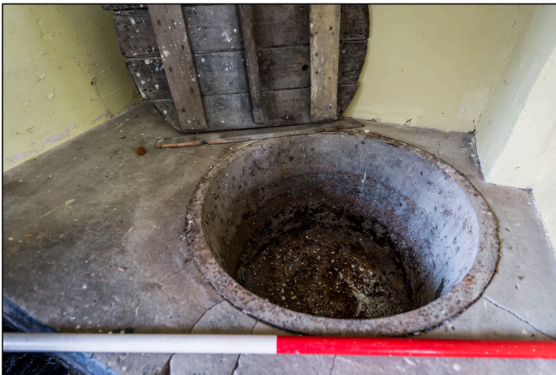
Appendix 2.44: Internal detail of (east) cast-iron laundry boiler in room 2G4 (Clock House) (1m scale). Photo No.77
