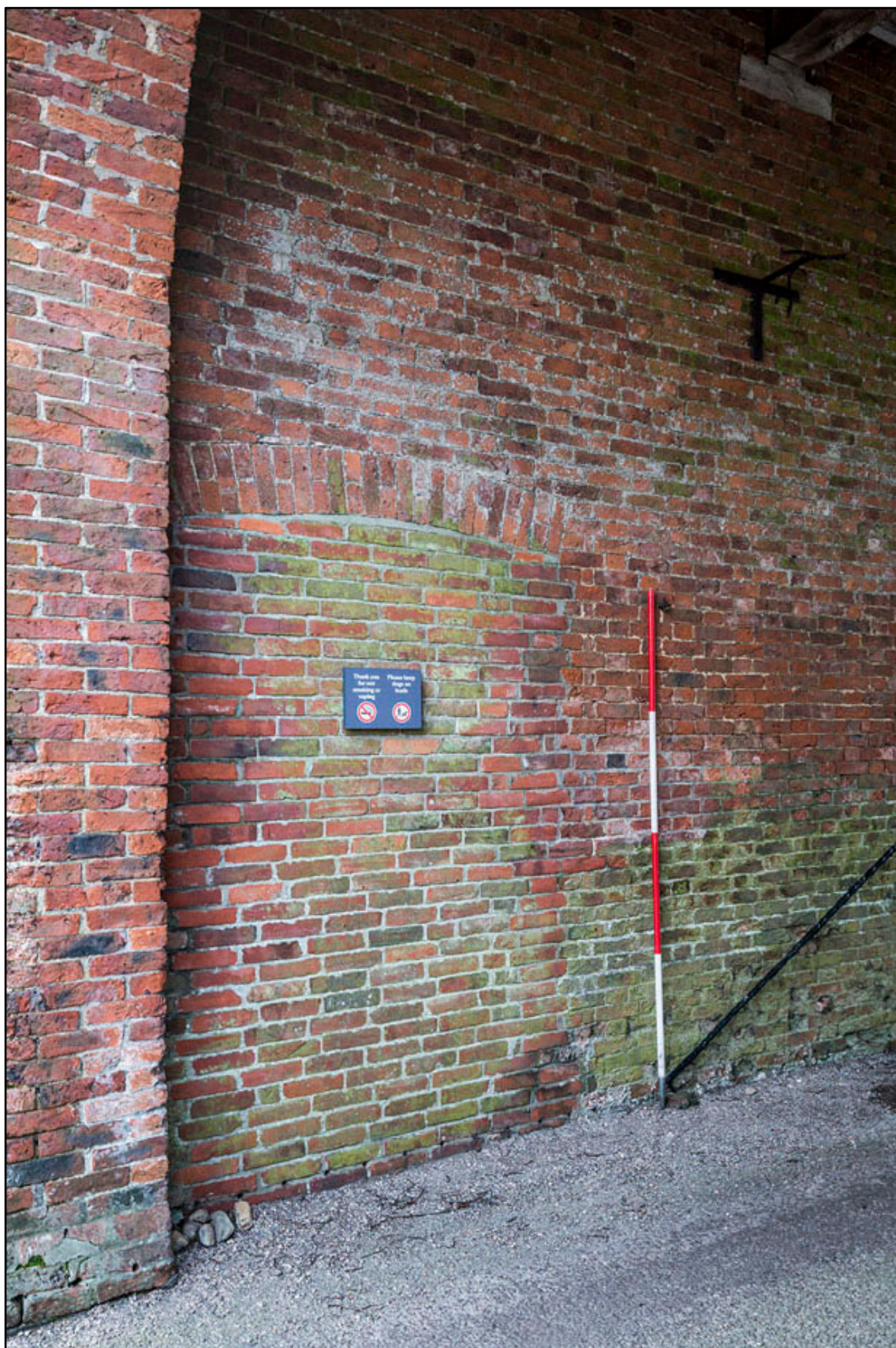
Appendix 2.23: Detail of blocked doorway in south wall of Clock House entrance passage 2G3 (2m scale). Photo No.36
