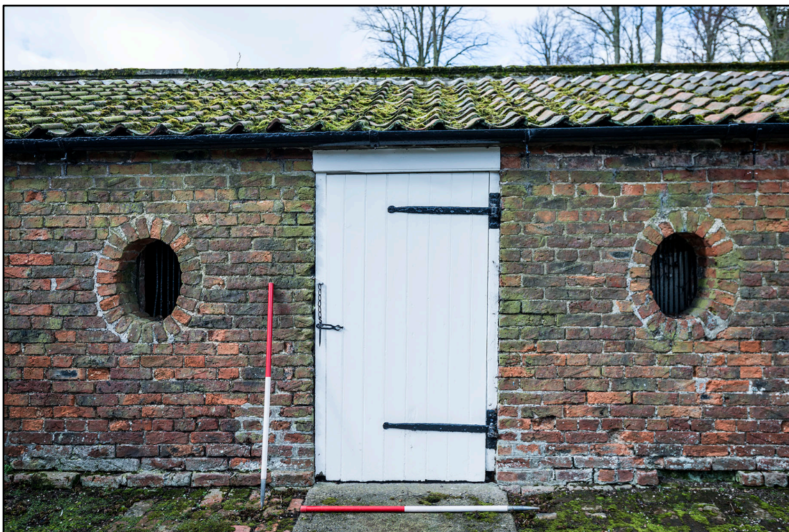
Appendix 2.9: Detail of vertical baton door into room IG4 (Outbuildings), looking west (1m scale). Photo No.21
