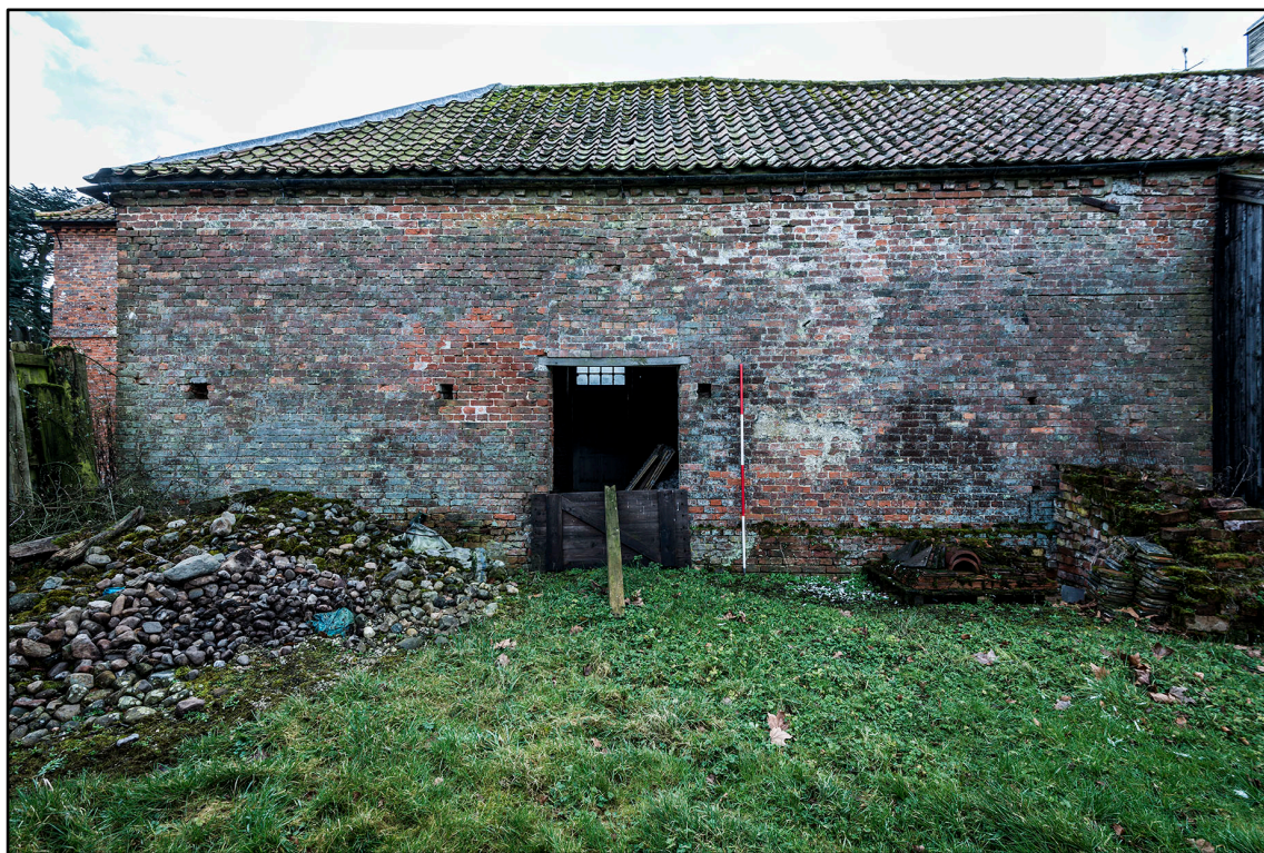
Appendix 2.67: Detail of doorway in northeast wall of Coach House; note blocked upper floor access (2m scale). Photo No.42
