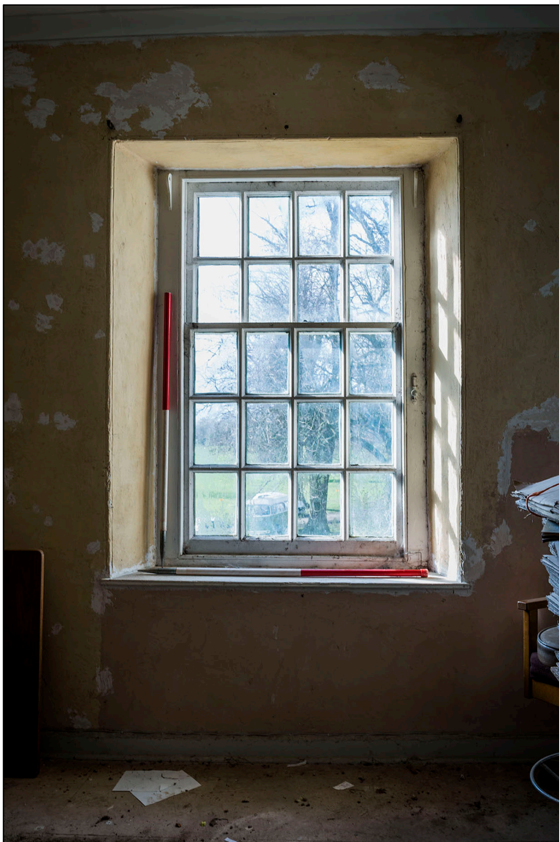
Appendix 2.36: Detail of sash window in room 2F4 (Clock House); note brackets for blinds (1m scale). Photo No.71
