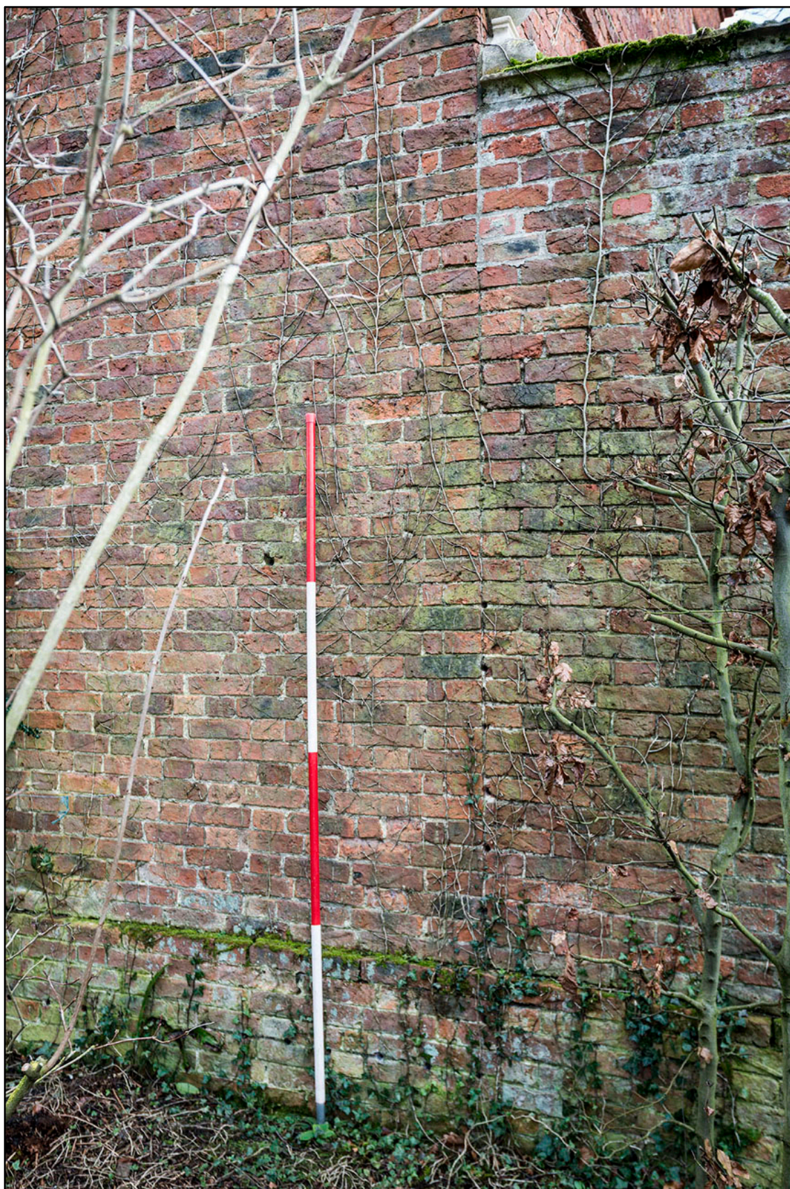
Appendix 2.21: Detail of vertical joint between garden wall and SW corner of Clock House (2m scale). Photo No.23
