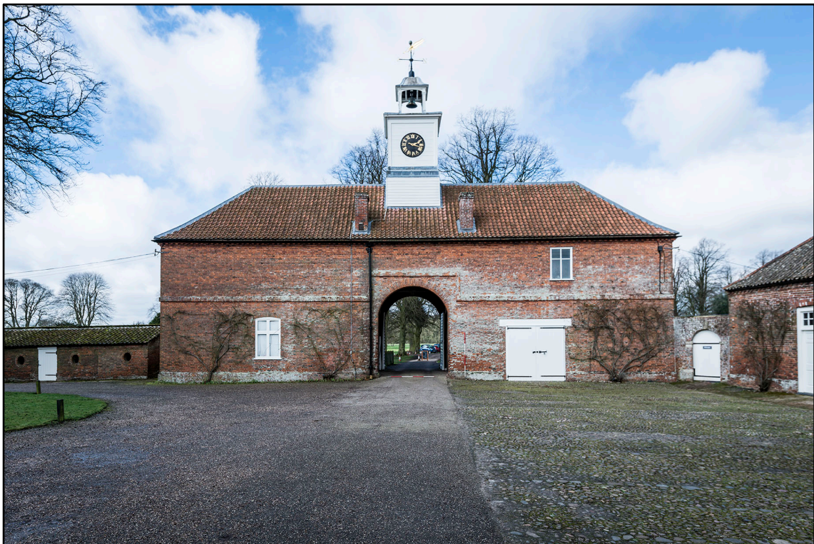
Appendix 2.17: General view of east elevation to Clock House (2m scale); note inserted double doors. Photo No.14
