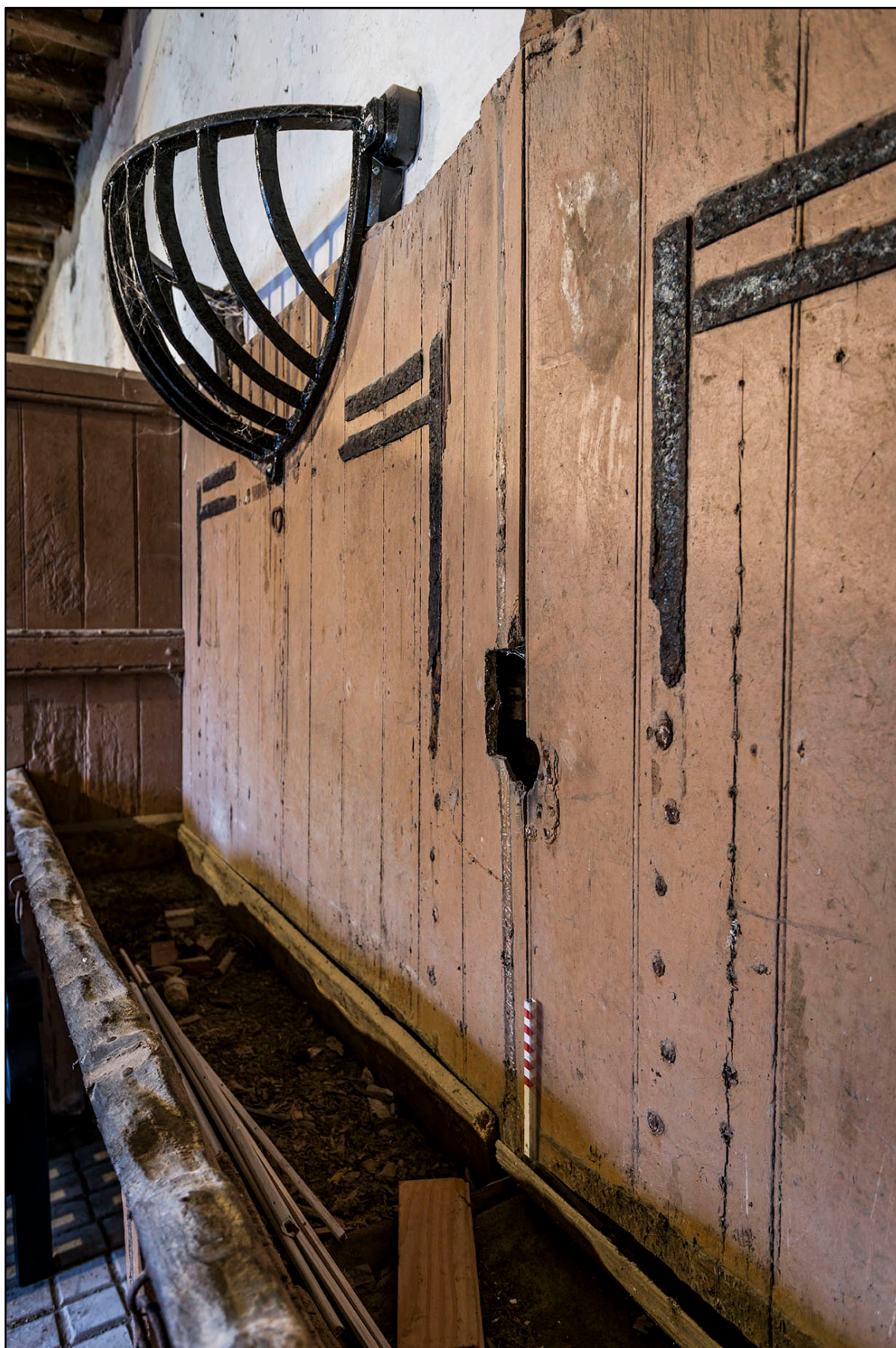
Appendix 2.101: Detail of cast-iron manger and iron strap-work in end stall in room 4G2 (Stables) (20cm scale). Photo No.110
