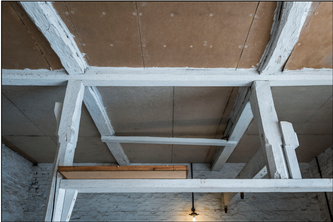
Appendix 2.81: Detail of ceiling and timber posts in room 3G3 (Coach House); note truncated timber post. Photo No.101
