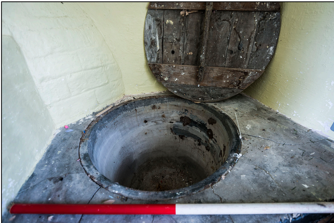
Appendix 2.42: Internal detail of (west) cast-iron laundry boiler in room 2G4 (Clock House) (1m scale). Photo No.79
