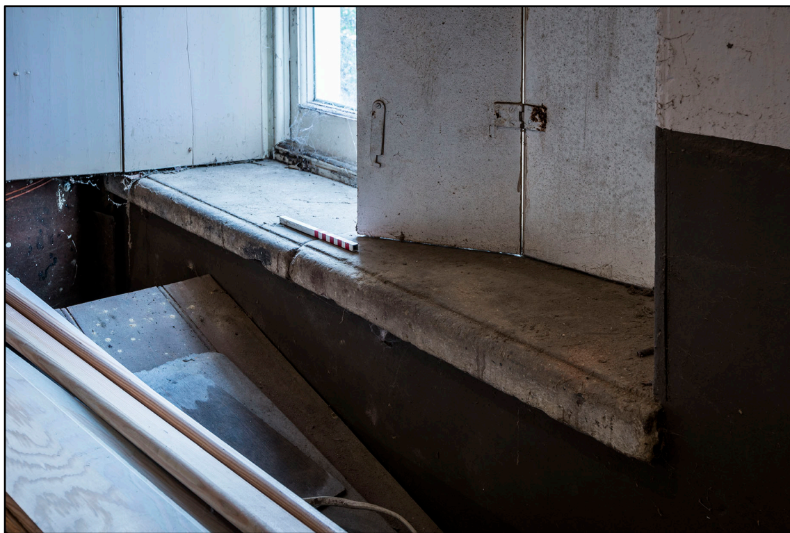
Appendix 2.30: Detail of stone window sills in room 2G2 (Clock House) (20cm scale). Photo No.66
