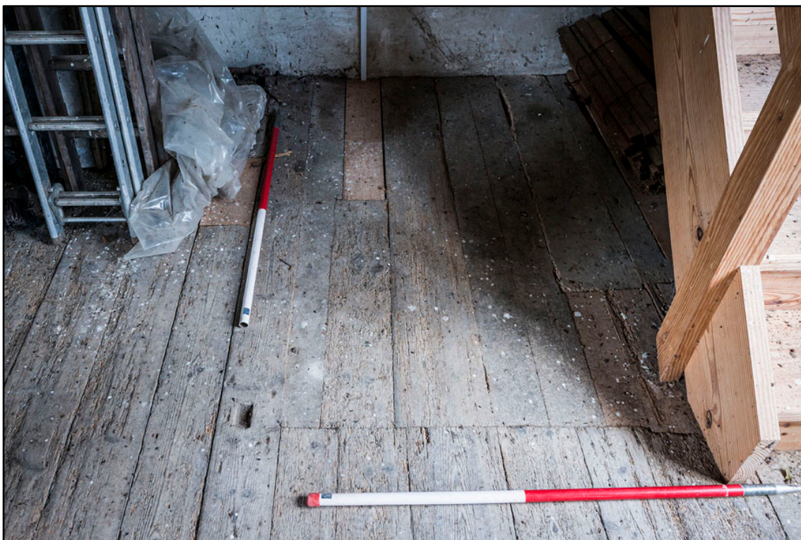
Appendix 2.54: Detail of planking denoting site of earlier staircase in room 2F5 (Clock House) (1m scale). Photo No.90
