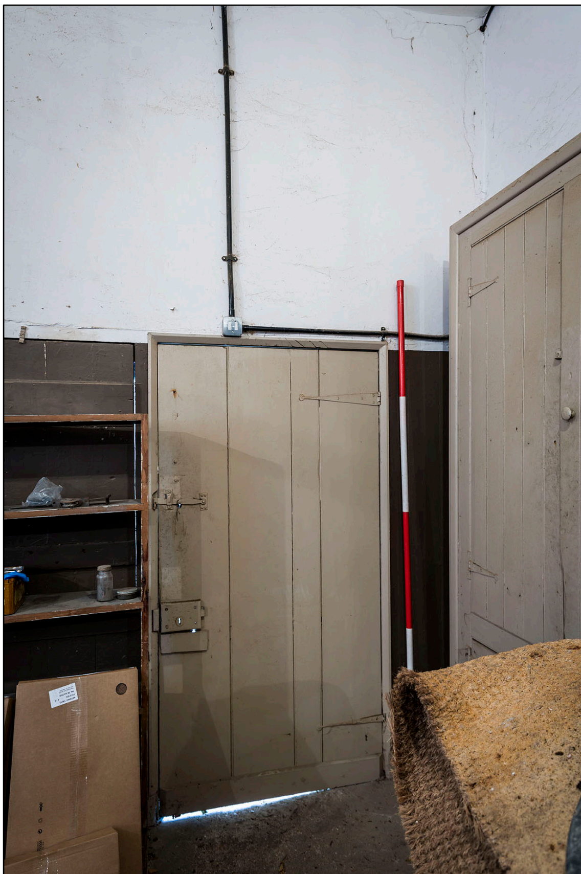
Appendix 2.31: Detail of baton door with strap hinges in south wall of room 2G2 (Clock House) (2m scale). Photo No.64
