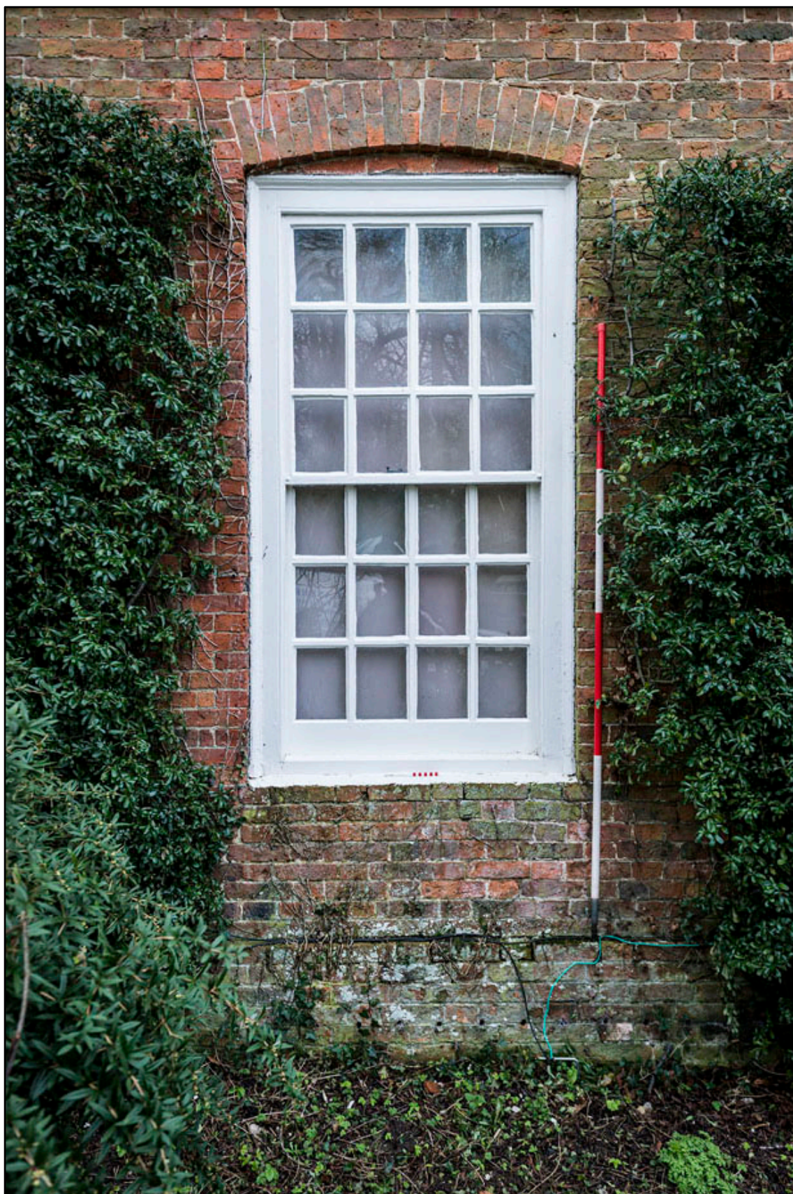
Appendix 2.22: Detail of external sash window on west elevation of Clock House (20cm/2m scale). Photo No.25
