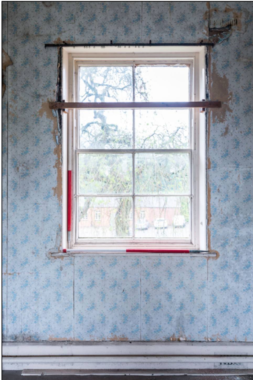
Appendix 2.76: Detail of hung-sash window in room F11 , looking west (1m scale). Photo No.91
