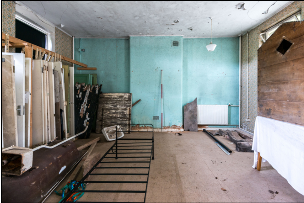
Appendix 2.54: General view of room G18 , looking north; note blocked fireplace and inserted radiator (2m scale). Photo No.67
