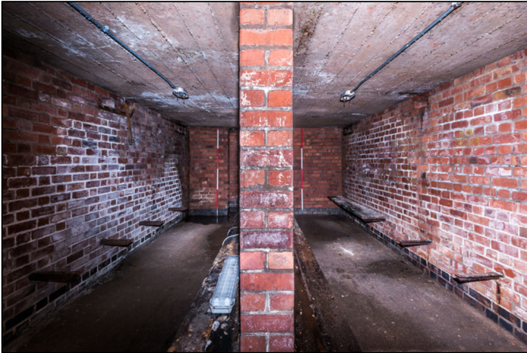
Appendix 2.101: General view of interior of air-raid shelter; note spine wall to separate male/female areas and iron bench supports still in-situ (2m scale). Photo No.117
