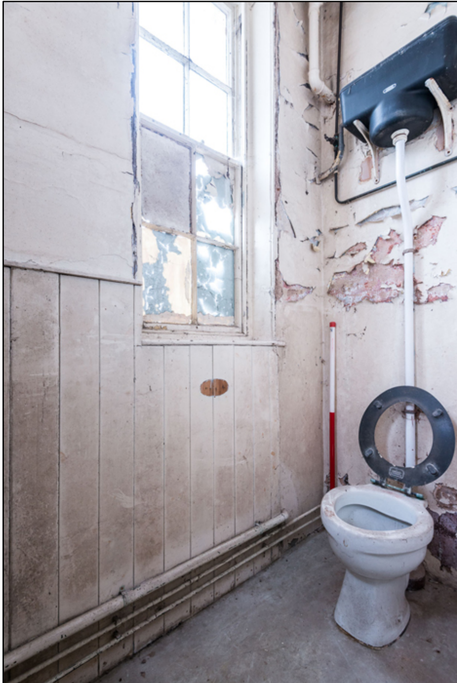
Appendix 2.30: Detail of timber match boarding in toilet G13 (1m scale). Photo No.36
