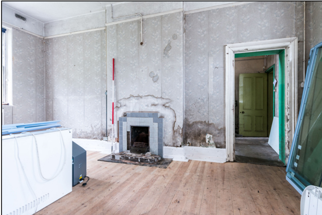
Appendix 2.42: Detail of north wall of room G15 ; note 1920s hearth and replaced flooring (2m scale). Photo No.51
