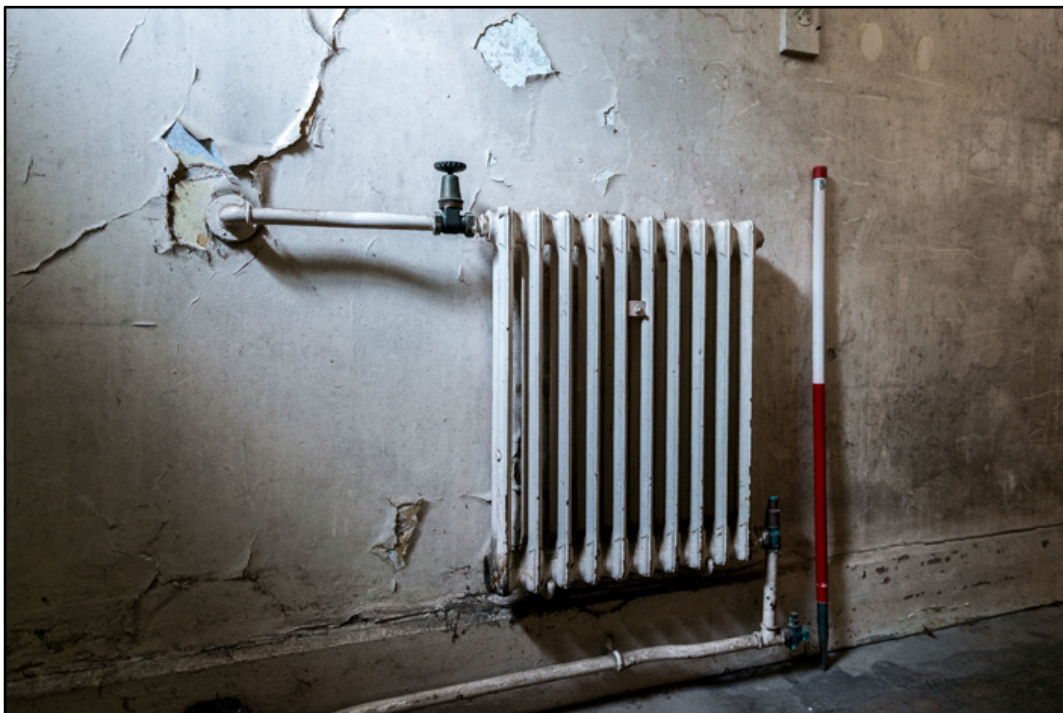
Appendix 2.35: Detail of cast-iron radiator in stairwell G12 (1m scale). Photo No.42
