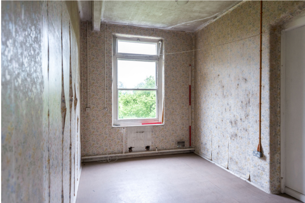
Appendix 2.65: General view of room F19 , looking east; note hopper style top-light on window (1m/2m scale). Photo No.78
