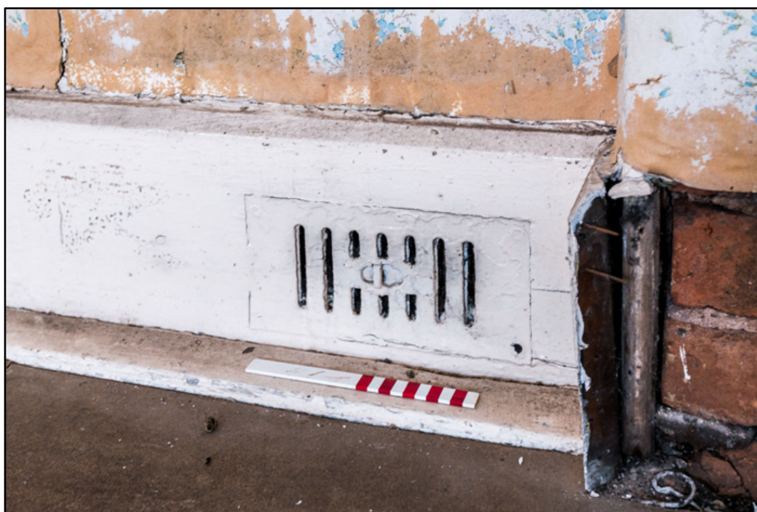
Appendix 2.82: Detail of skirting mounted cast-iron ventilation grill in room F10 (20cm scale). Photo No.101
