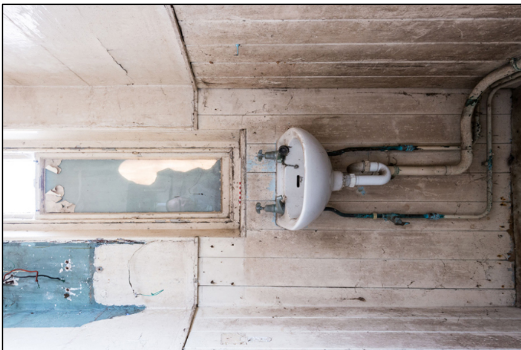
Appendix 2.29: Detail of timber match boarding in toilet G13 , looking north (20cm scale). Photo No.37
