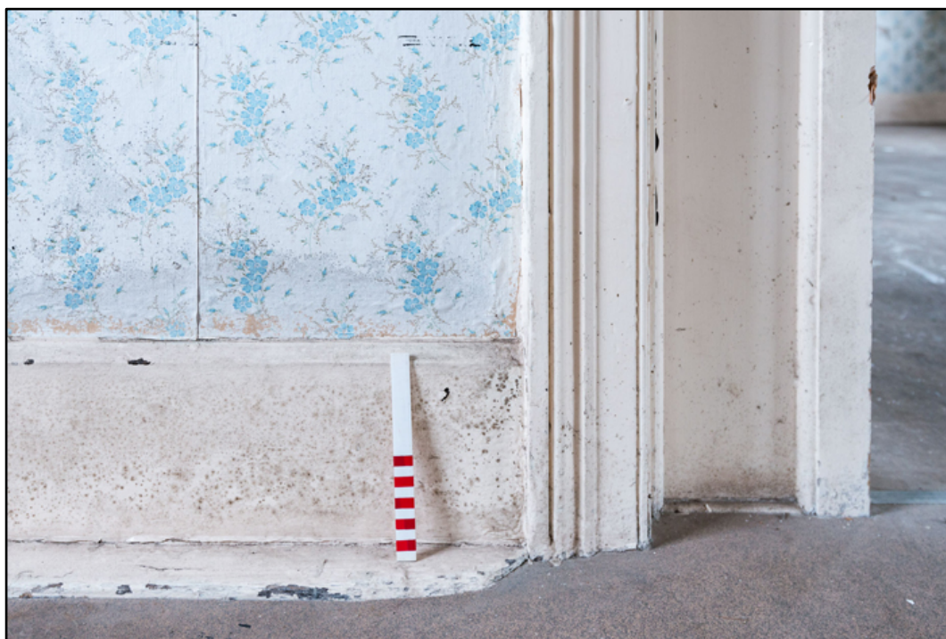
Appendix 2.81: Detail of skirting and door architrave in room F10 (20cm scale). Photo No.95
