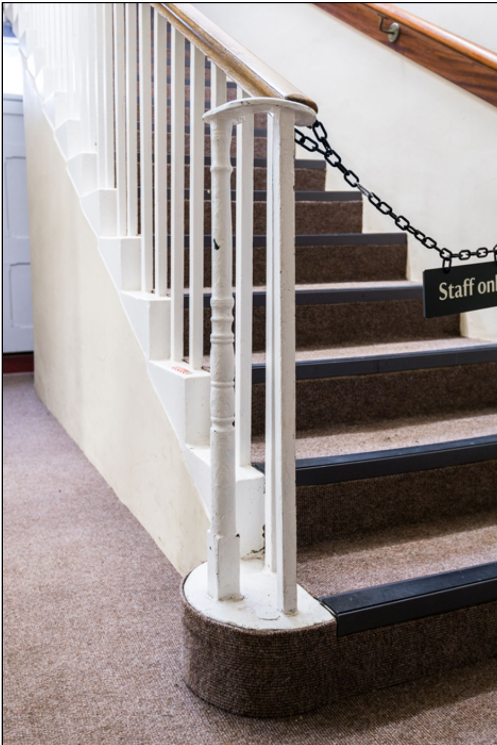
Appendix 2.25: Detail of original metal newel post at base of stairwell G3 (20cm scale). Photo No.31
