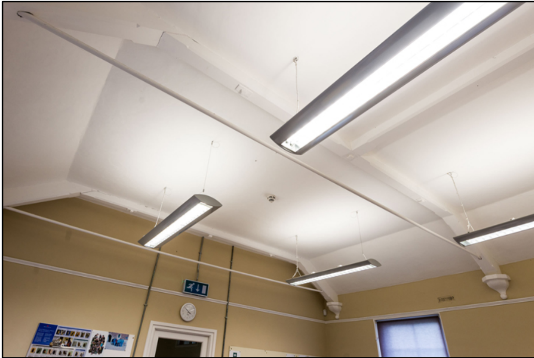
Appendix 2.96: General view of the ceiling in room FI looking north; note exposed trusses and tie rods. Photo No.115
