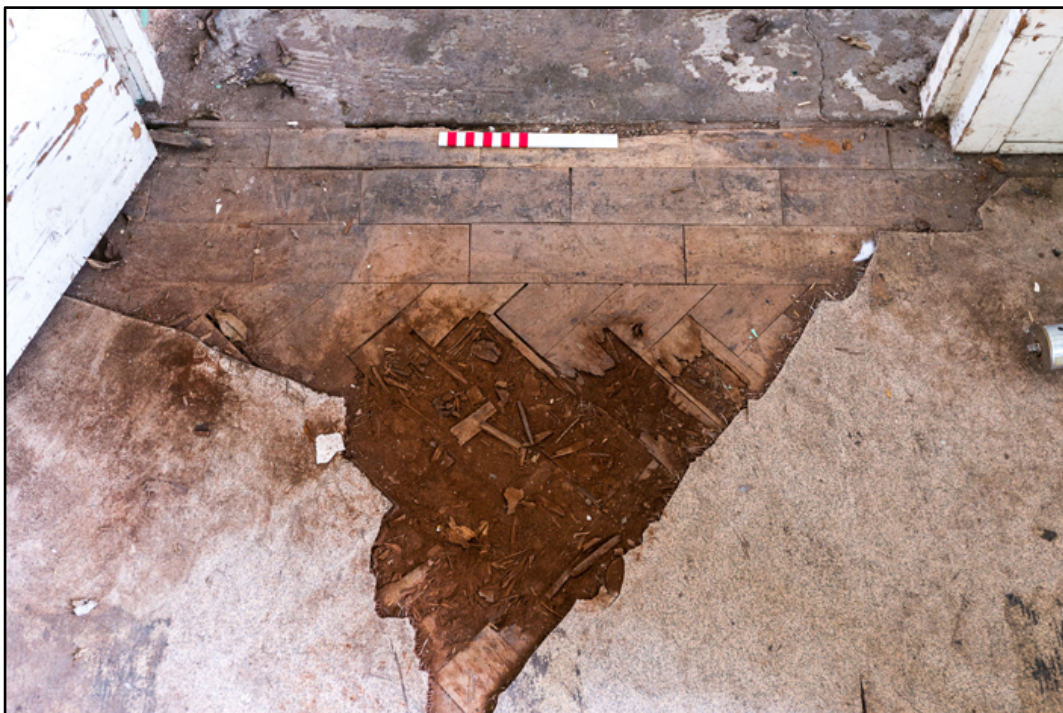
Appendix 2.51: Detail of original parquet (decayed) flooring in entrance of room G17 (20cm scale). Photo No.64
