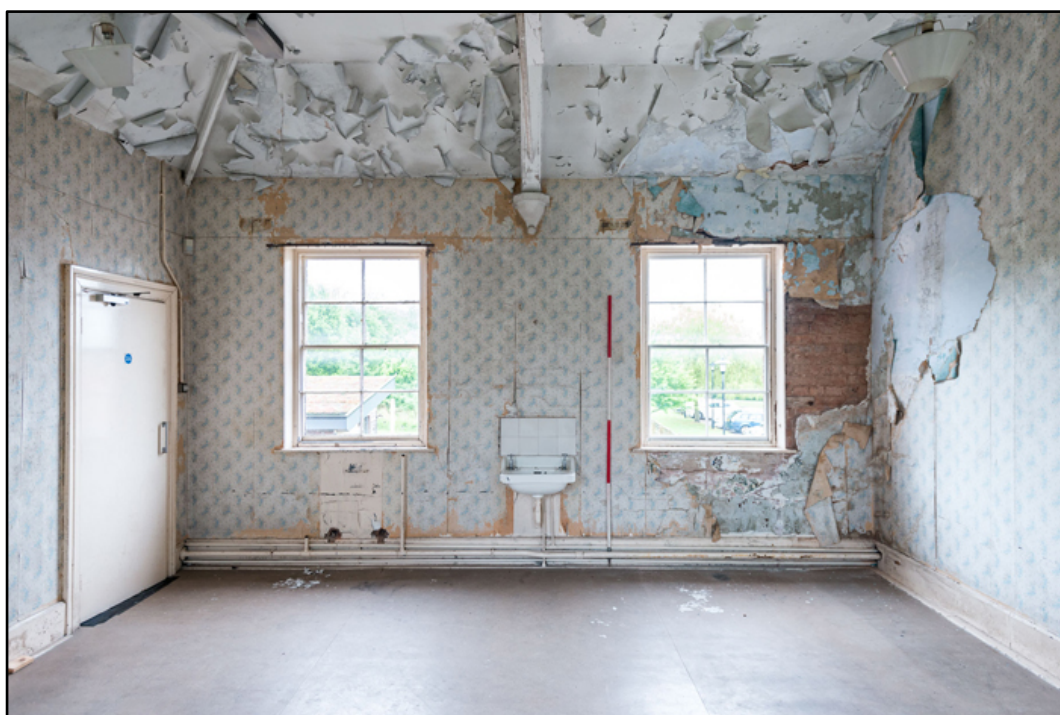
Appendix 2.78: General view of room F11, looking east; note inserted sink and pipes for heating. Photo No.94
