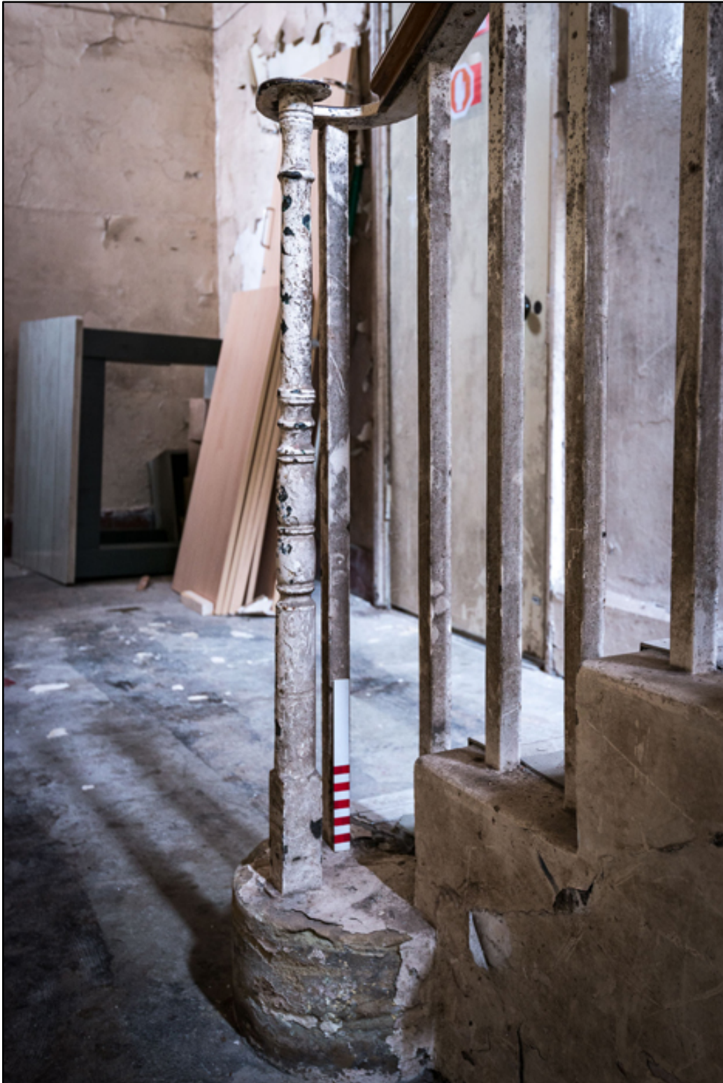
Appendix 2.33: Detail of original metal newel post at base of stairwell G12 (20cm scale). Photo No.40
