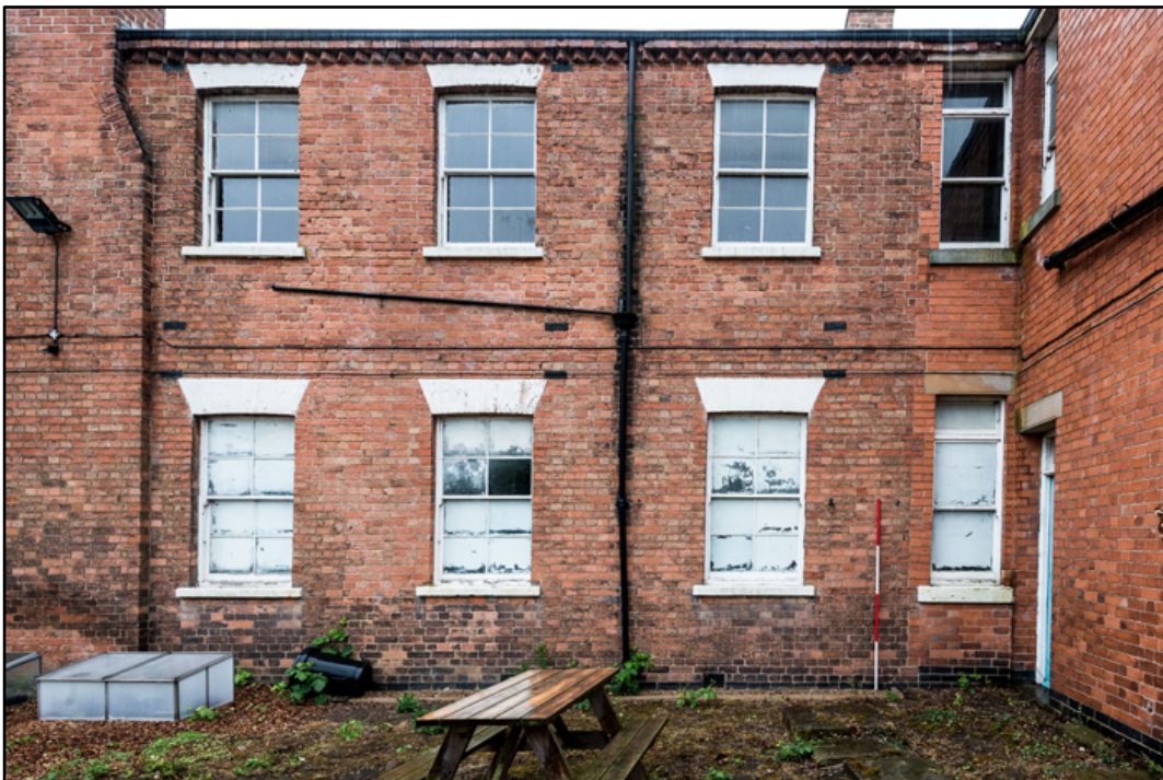
Appendix 2.18: General view of external east elevation of rooms G14/G15/F10/F11; note vertical construction joint (2m scale). Photo No.28
