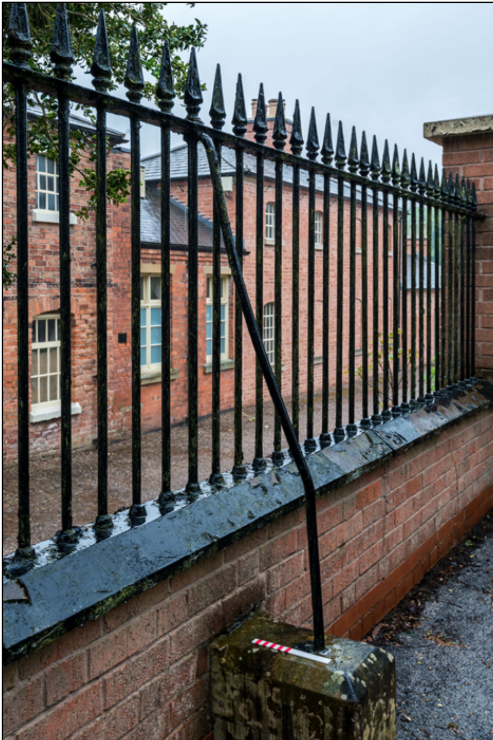
Appendix 2.10: Detail of original railings and stay around southwest boundary to Firbeck House (20cm scale). Photo No.15
