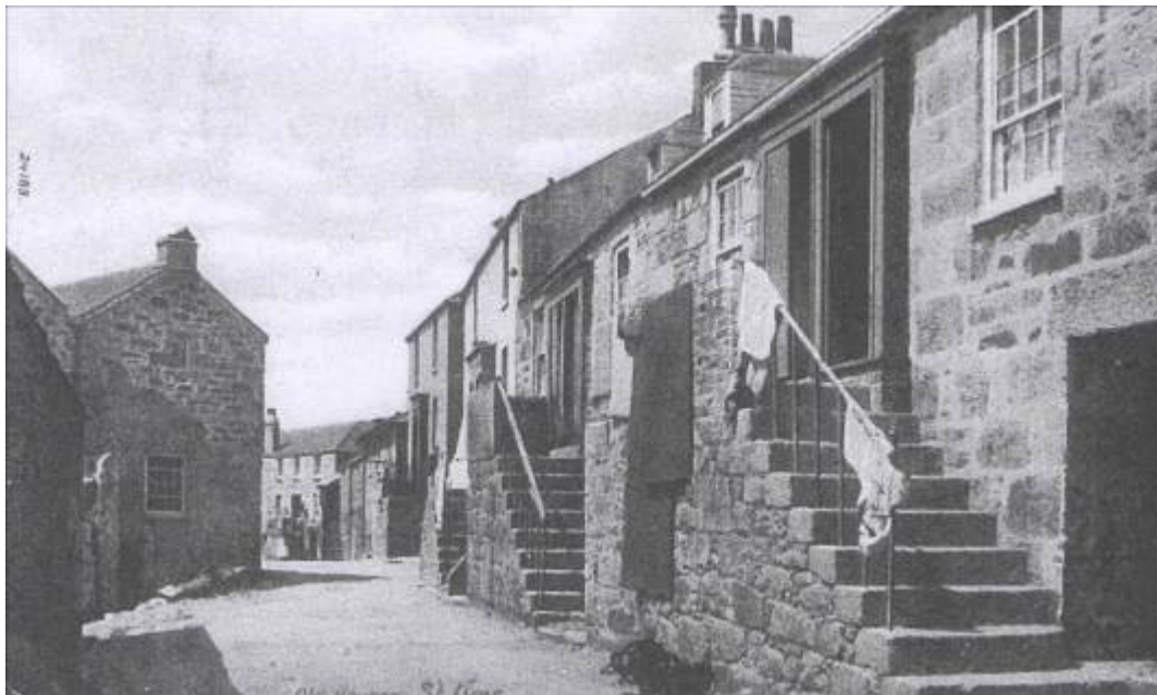
Figure 15. 'Old Houses, St Ives', with similar cellar arrangement and steps to adjacent first-floor rear (from St Ives Bay by J Holmes)
