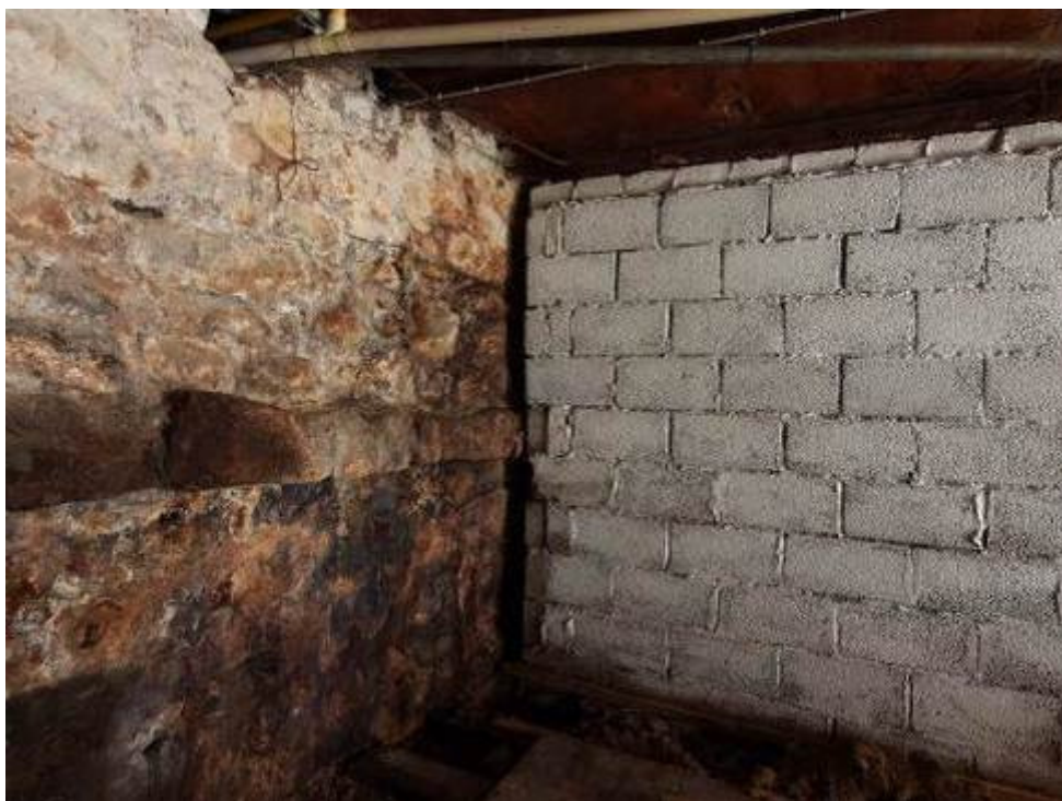
Figure 26. Pressing ledge of N cellar wall continuing beyond modern concrete block partition wall (indicating that cellar originally extended below No. 16/17 Teetotal St)
