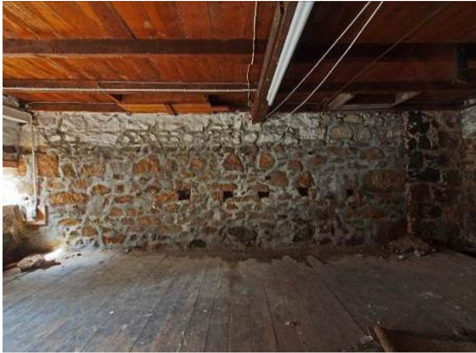
Figure 24. Pressing pole slots in W cellar wall; note also later wooden planked floor, laid over the original cobbled floor
