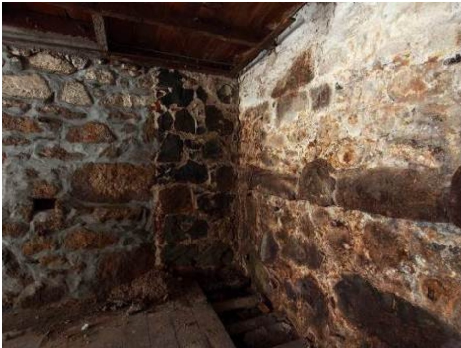
Figure 25. NW corner of cellar, with pressing ledge in N wall, pressing pole slot in W wall and blocked doorway in between
