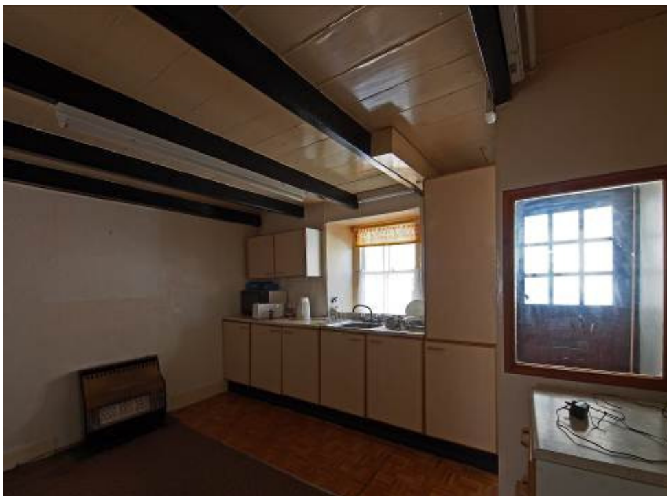
Figure 29. Ground floor N room (Teetotal St); traces of a larger fireplace in W wall, around the existing gas fire; note original wide-planked ceiling/second floor
