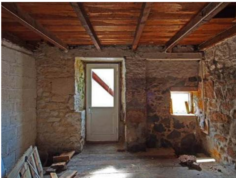
Figure 27. S wall of cellar, showing present doorway (originally a window) and window (originally a wide door opening); both have re-used ships timbers as lintels
