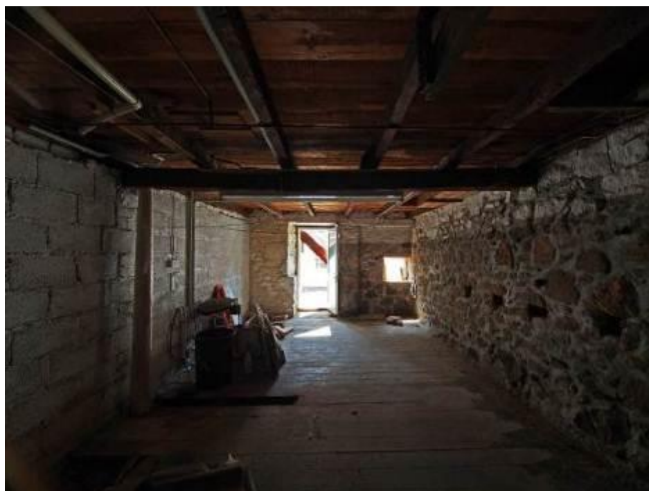
Figure 5. Cellar before removal of wooden floor; looking S to St Eia St entrance; note pilchard pressing pole slots in right hand wall, re-used ships spar supporting large cross beam (Eric Berry, Sept 2012)
