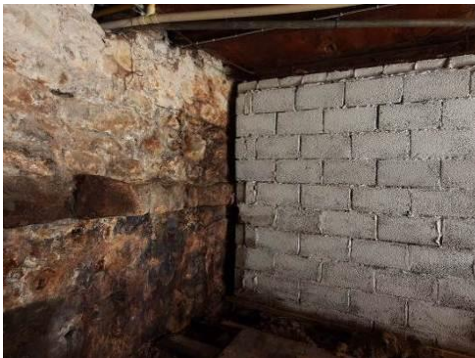
Figure 8. Cellar before removal of wooden floor; pressing ledge of N cellar wall continuing beyond modern concrete block partition wall, indicating that cellar originally extended below No. 16/17 Teetotal St (Eric Berry, Sept 2012)
