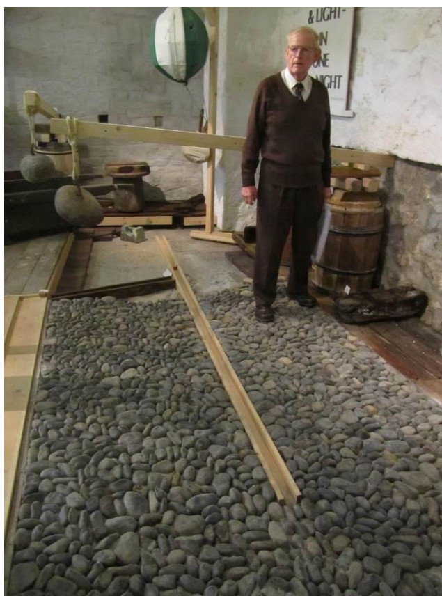
Figure 16. St Ives Museum (originally a pilchard pressing cellar); original pressing ledge and wooden barrel-base/drain along the bottom of the wall (cobbles and other wooden drains are reconstructions); with Curator, Brian Stevens (2012)
