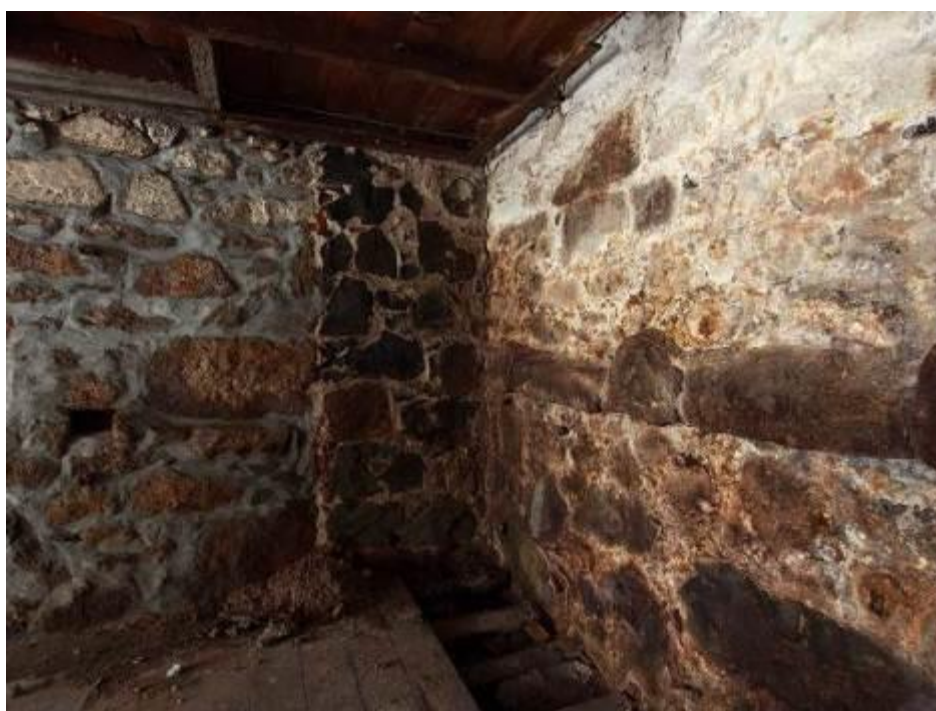
Figure 7. Cellar before removal of wooden floor; NW corner of cellar, with pressing ledge in N wall, pressing pole slot in W wall and blocked doorway in between (Eric Berry, Sept 2012)
