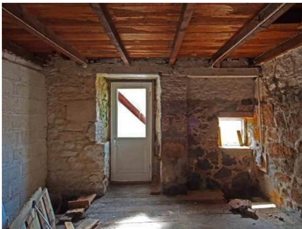
Figure 9. Cellar before removal of wooden floor; S wall, showing present doorway (originally a window) and window (originally a wide door opening); both have re-used ships timbers as internal lintels (Eric Berry, Sept 2012)
