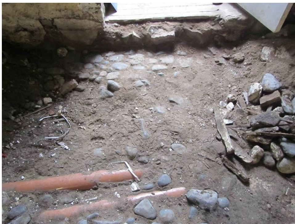
Figure 21. Cellar after removal of wooden floor; modern drain trench cut through cobbled floor across S end of room, looking S; fragment of cobbling surviving in front of doorway (March 2013)
