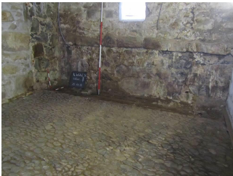
Figure 12. Cellar after removal of wooden floor; pressing ledge and wooden barrel-base/drain along N wall (March 2013)
