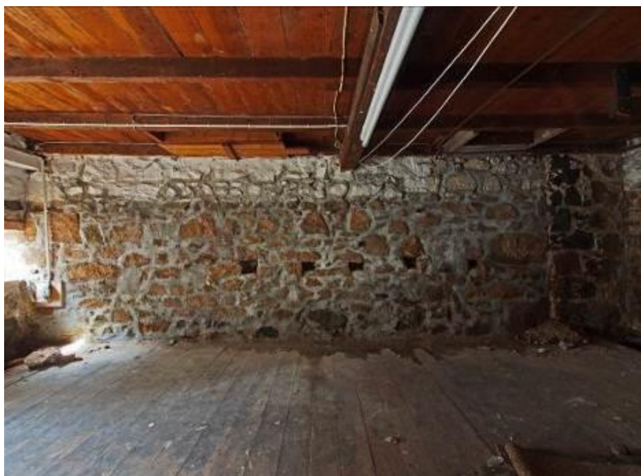
Figure 6. Cellar before removal of wooden floor; pressing pole slots in W cellar wall (Eric Berry, Sept 2012)
