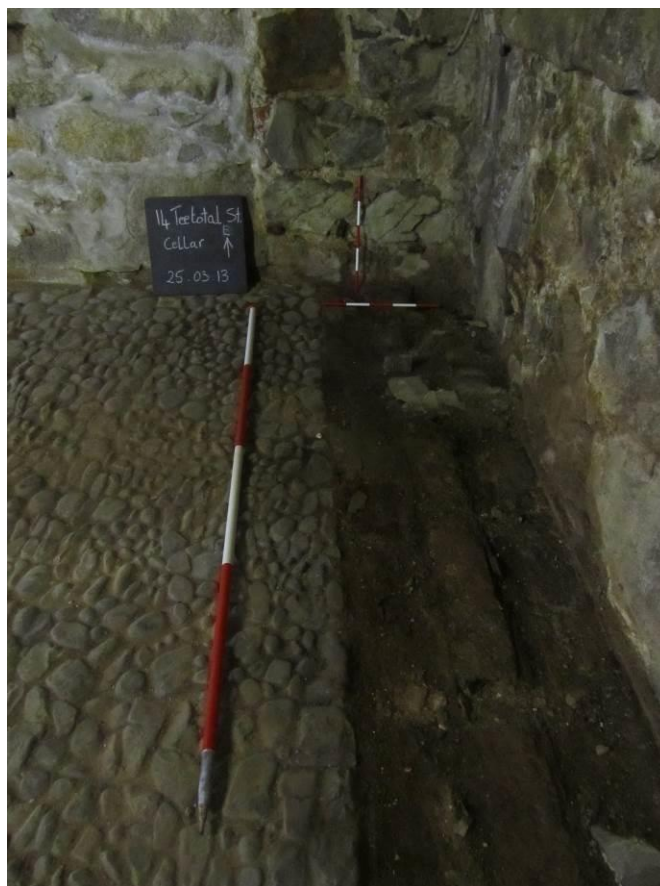
Figure 13. Cellar after removal of wooden floor; wooden barrel-base/drain along bottom of N wall, looking W (not E, as it says on board) (March 2013)
