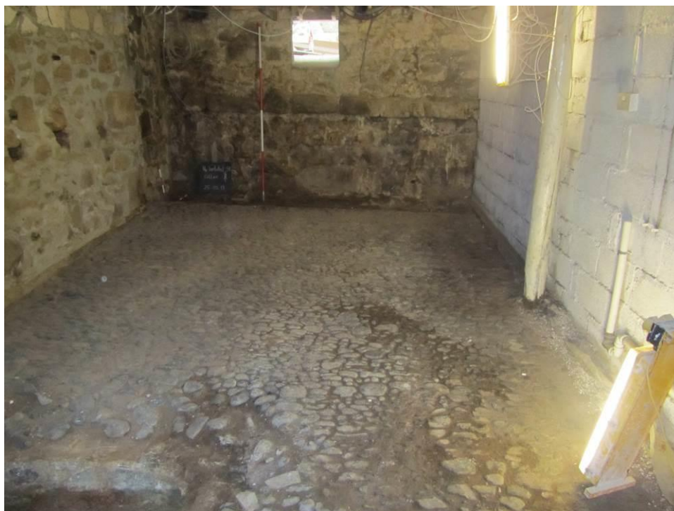
Figure 11. Cellar after removal of wooden floor; looking N across cobbled floor towards pressing ledge & wooden barrel-base/drain along N wall, and new window opening (March 2013)
