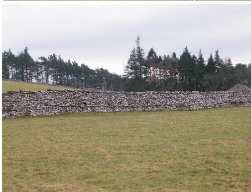
Plates 18 and 19: The deer park wall at Wharton just outside the Lake District National Park (top) has a quite different construction technique to 18-19 th century enclosure walls with through stones (© Archaeo-Environment Ltd)
