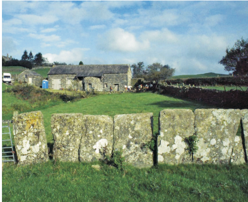
Plate 20: Shard fencing, made of simple upright stone slabs (© LDNPA)
