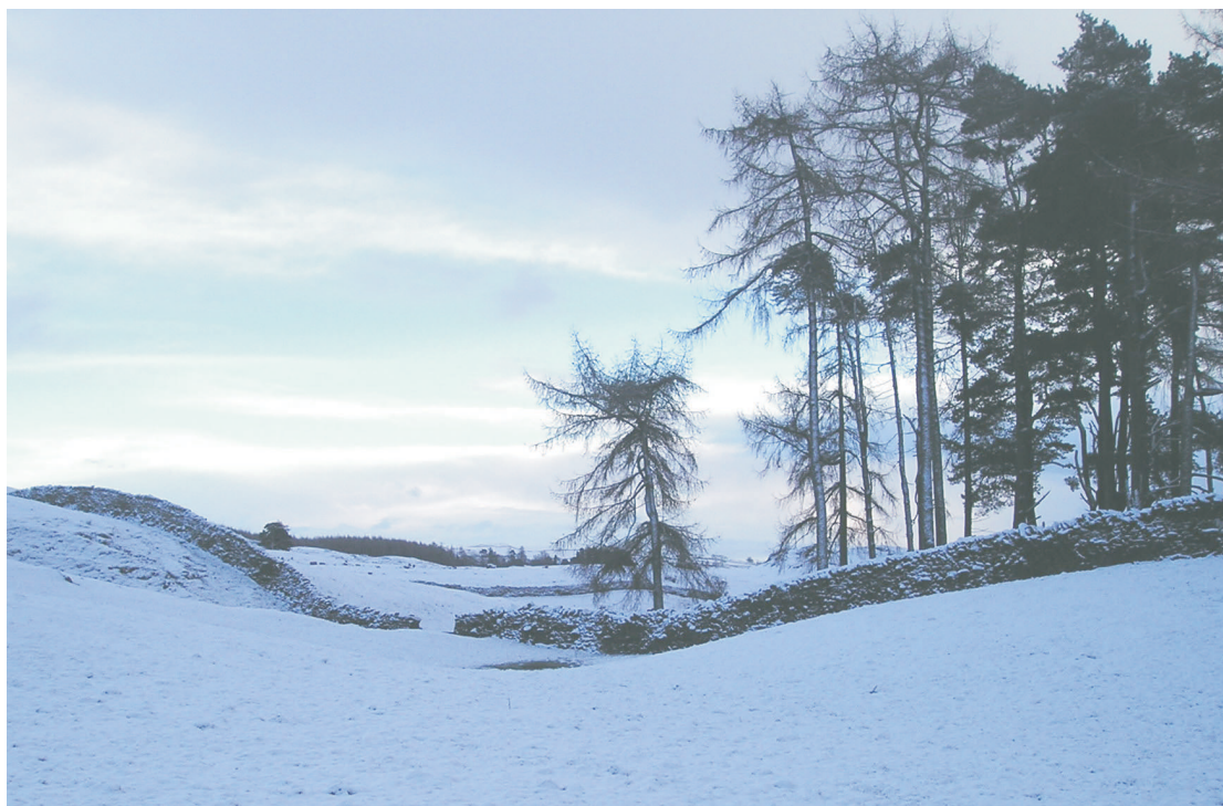
Plate 31: Stone enclosure wall, built to a minimum specification. A course of 'through' stones can be seen halfway up the wall. Beyond is a small stand of conifers, typical of small-scale enclosure-period plantations (© Lucy Drummond)
