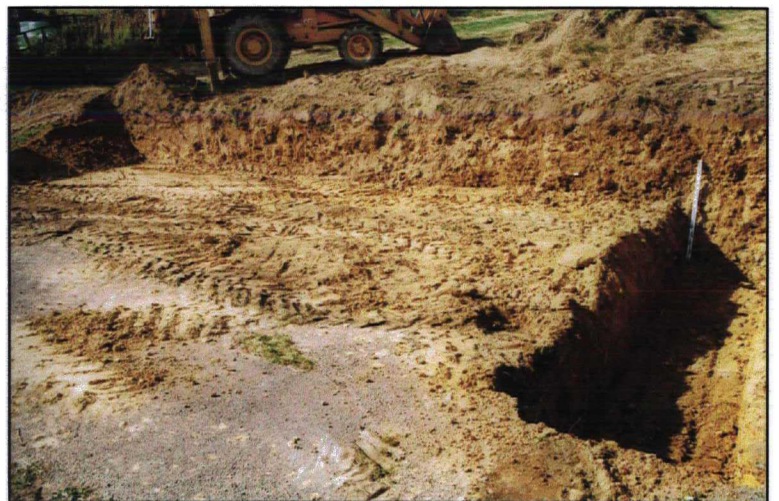
Plate 4: Completed groundworks and East footing trench, looking NW.
