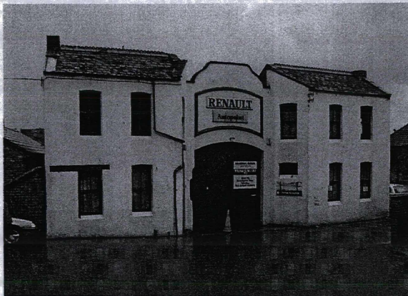
The street front; late 19 th century Stables/Coach House Entrance, with later alterations
