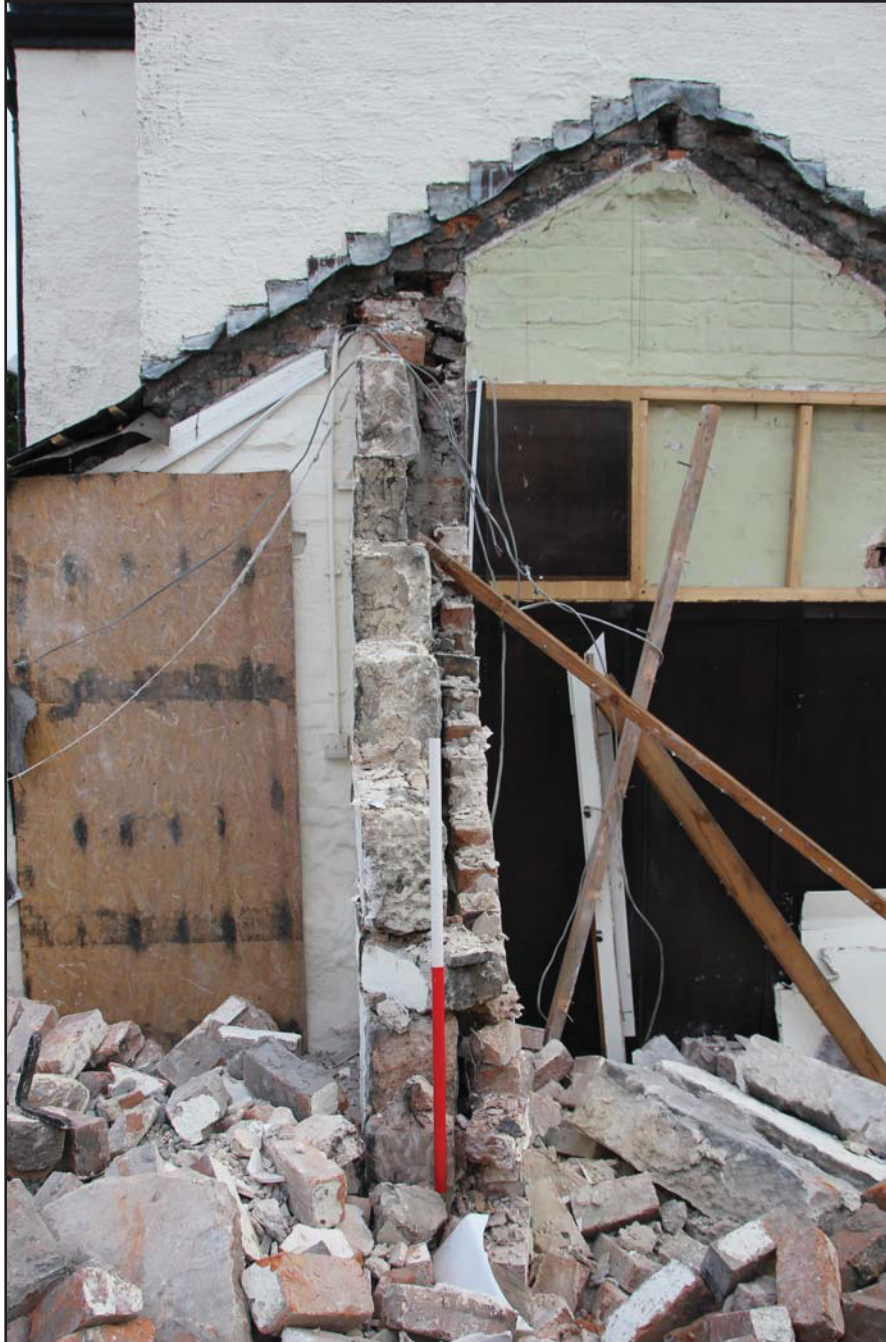
Plate 02: Sandstone wall with internal brick skin, from the northeast. Scale 1.0m.
