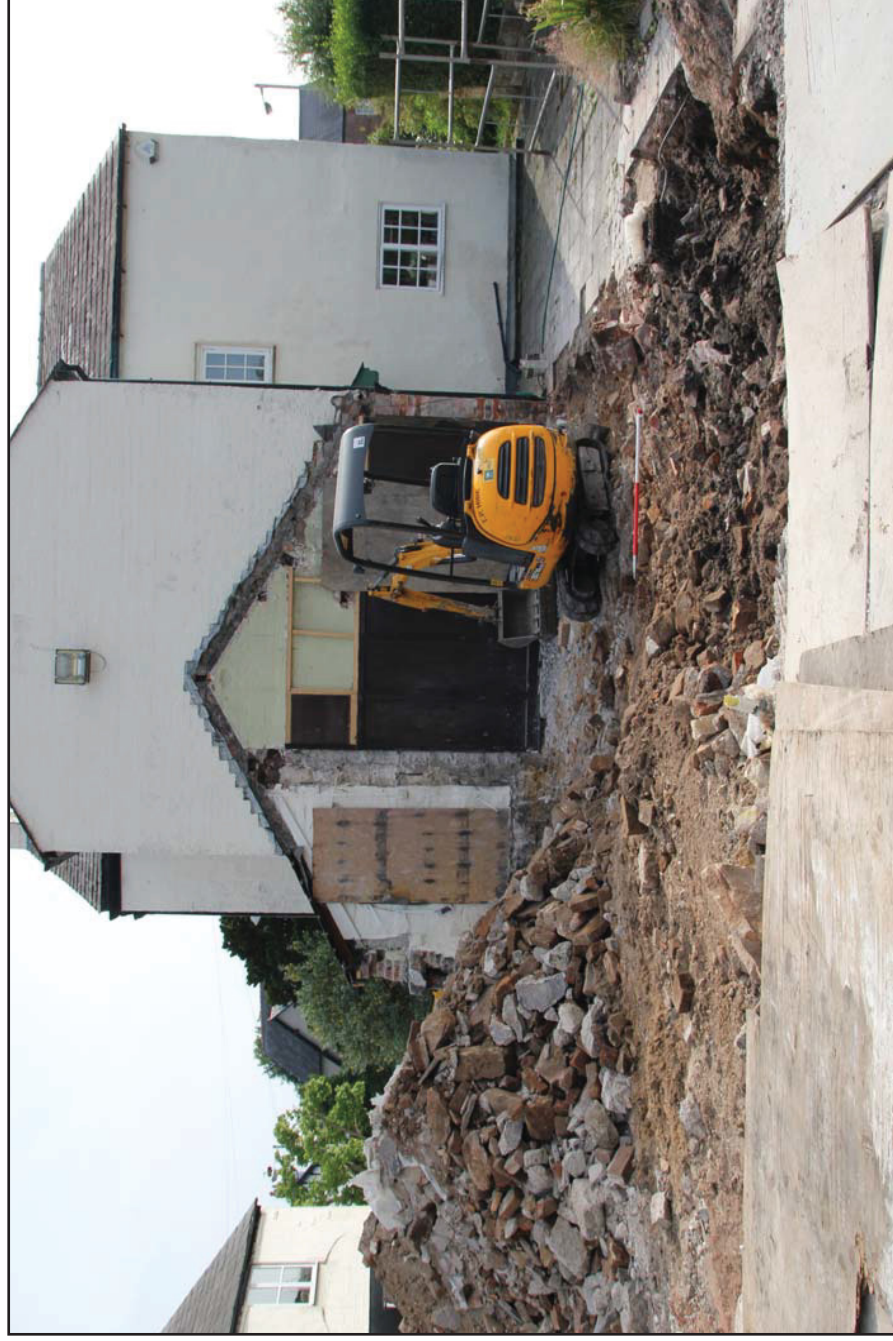
Plate 04: Ground reduction on to hardcore levelling layer (1002), from the northeast. Scale 1.0m.
