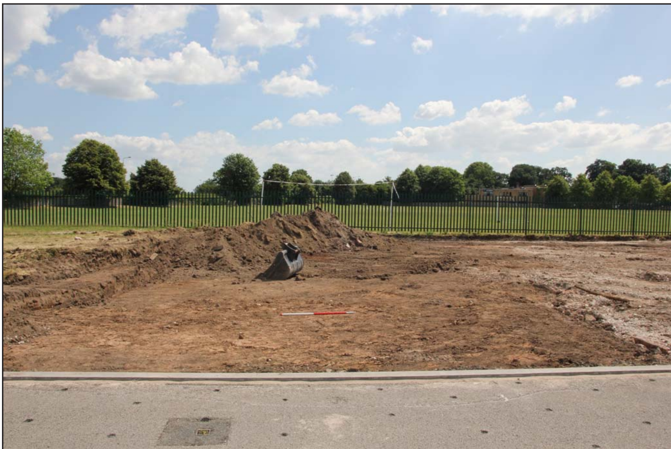
Plate 05: Removing the topsoil and subsoil layers within the grassed area, from the northwest. Scale 1.0m.
