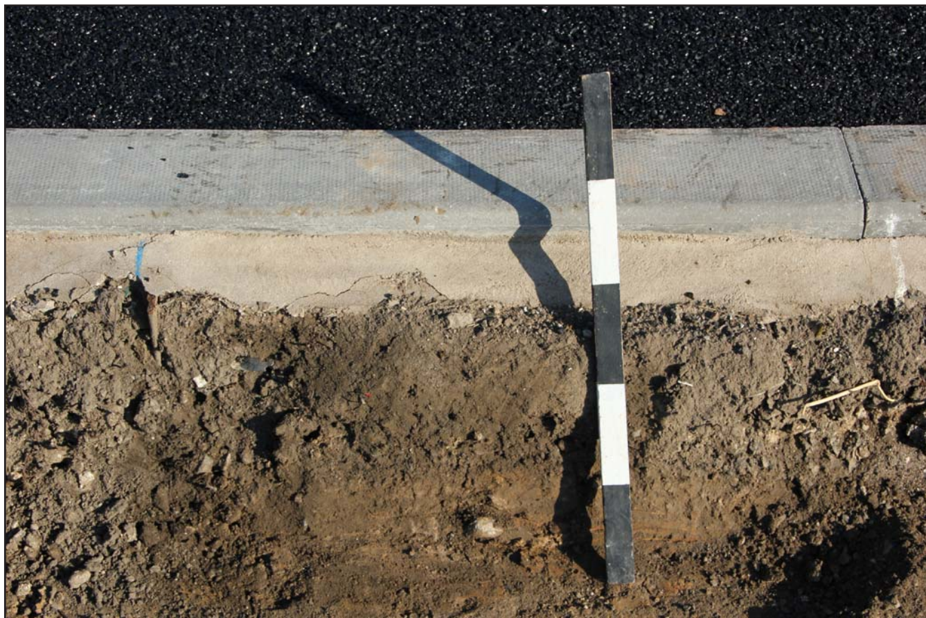
Plate 07: Trench section showing the ground reduction beneath the existing tennis courts, from the southeast. Scale 0.5m.
