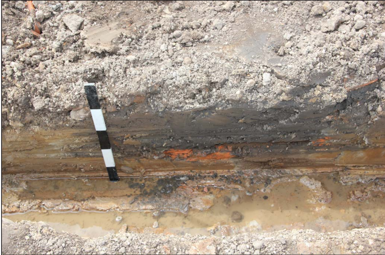
Plate 10: Section of new drain showing buried ceramic field drain, from the northeast. Scale 0.5m.
