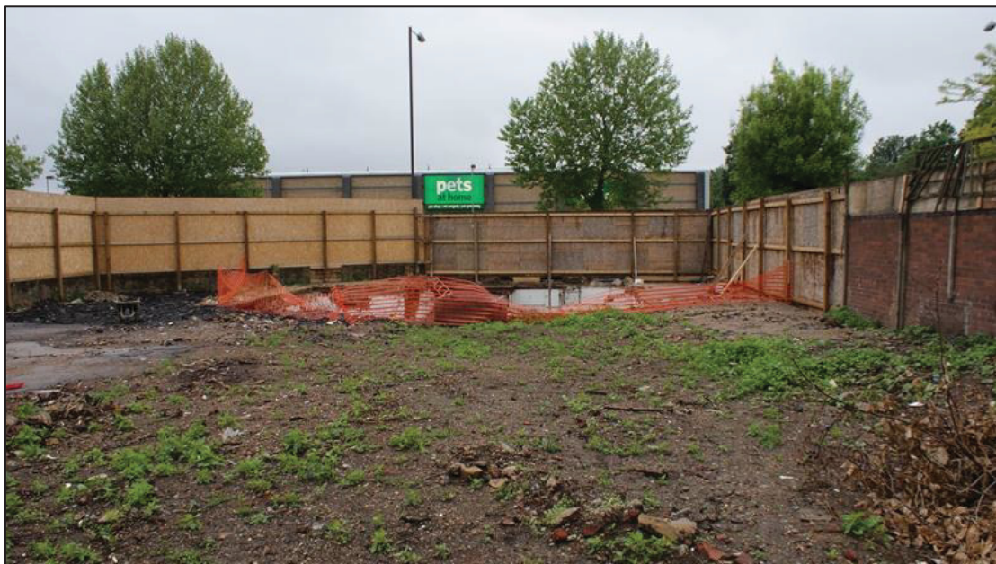
Plate 1 General view of the Site looking from the southeast towards the exposed cellar
