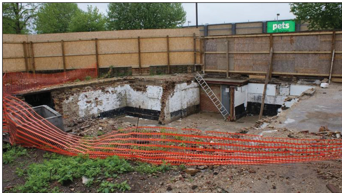
Plate 2: General view of cellar of the former George and Dragon, looking northwest
