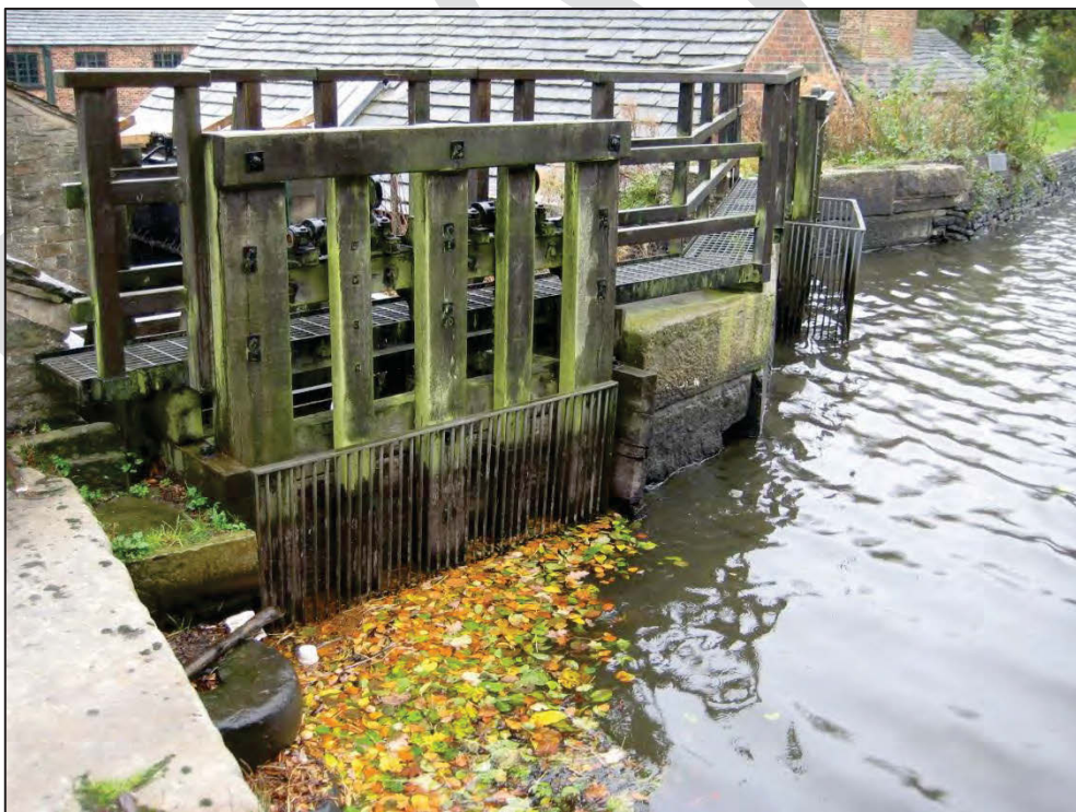
Plate 2: Detail of the sluice/penstock with mill pond steps at the bottom of the frame
